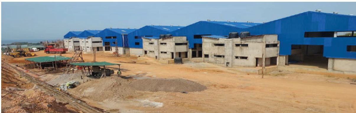
Construction works at UFZA at Entebbe Airport site.
