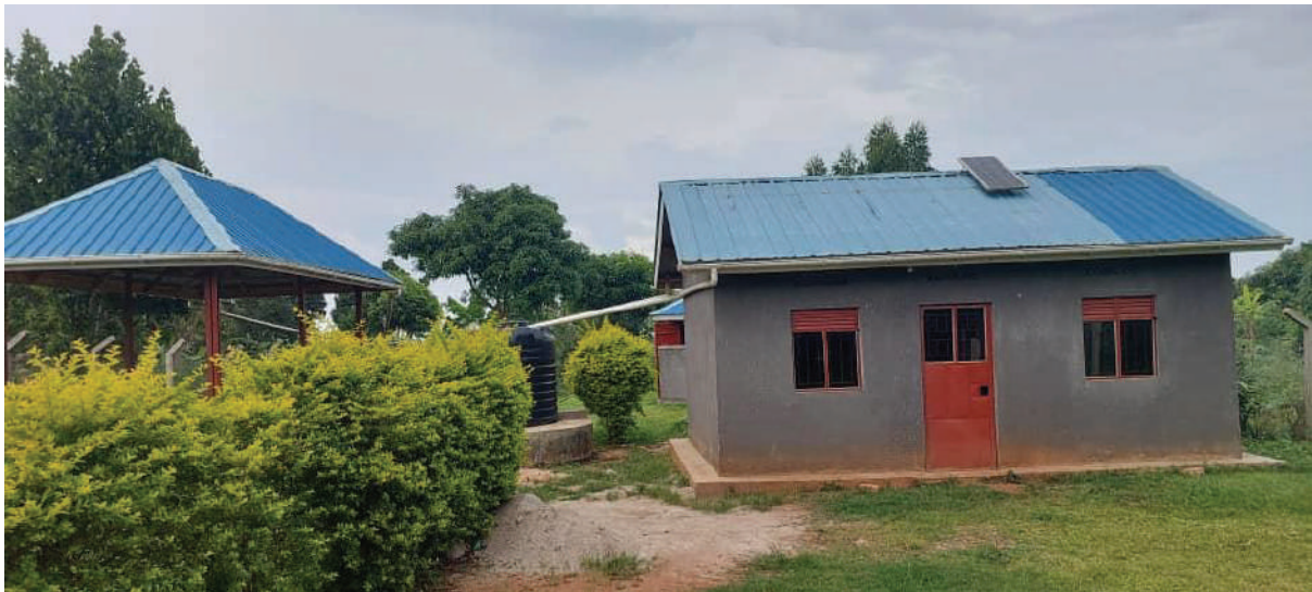
Police Post and detention cell at UFZA Buwaya site
