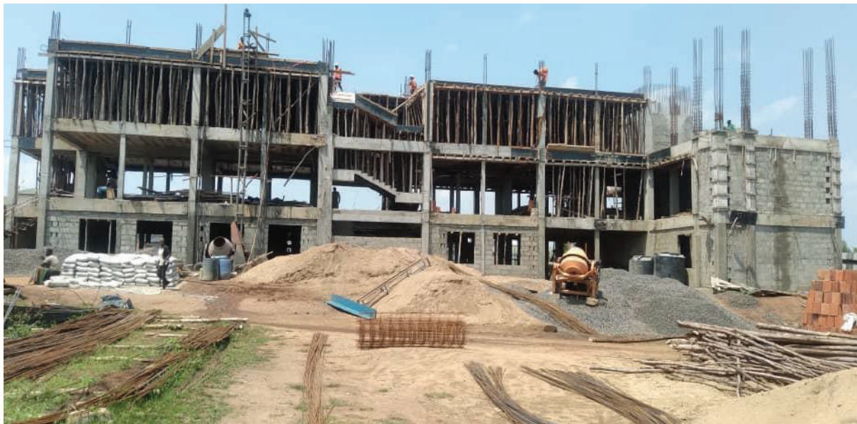
Administration block Annex under construction.
