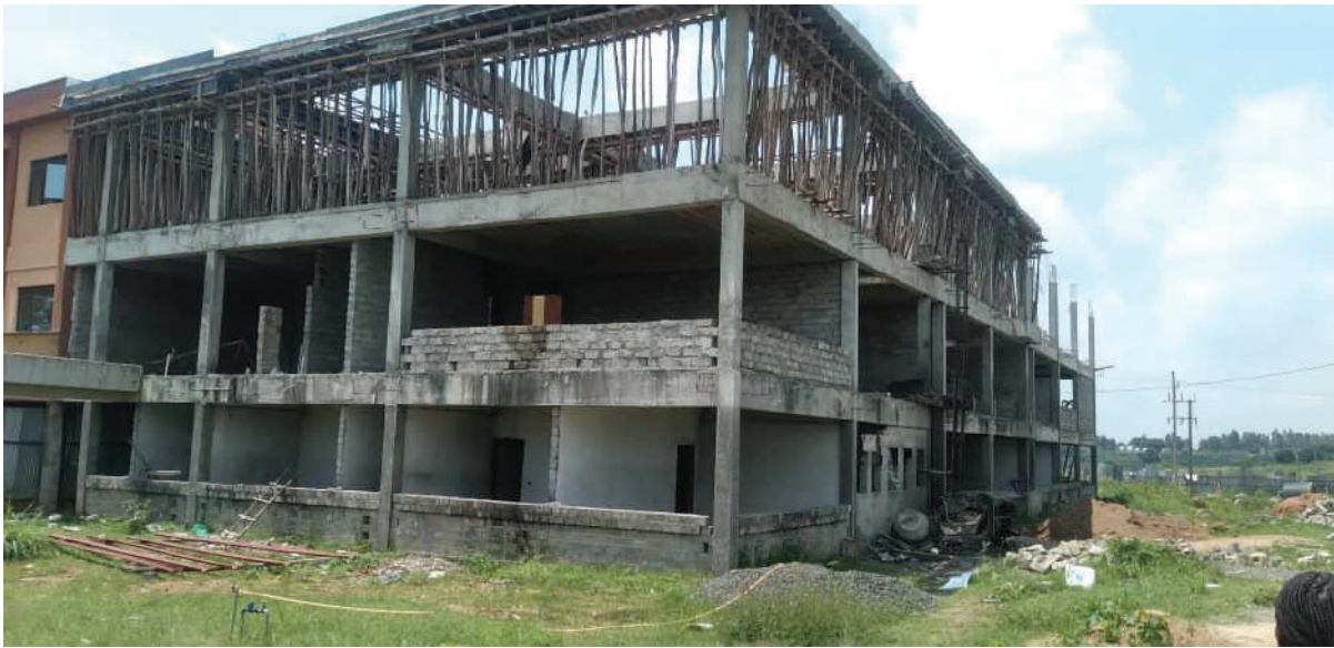
Health Science Laboratory phase II under construction.
