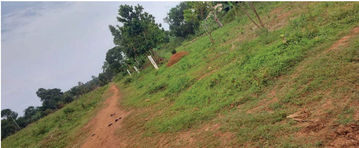
Concrete boundary markers installed at UFZA land in Buwaya.
