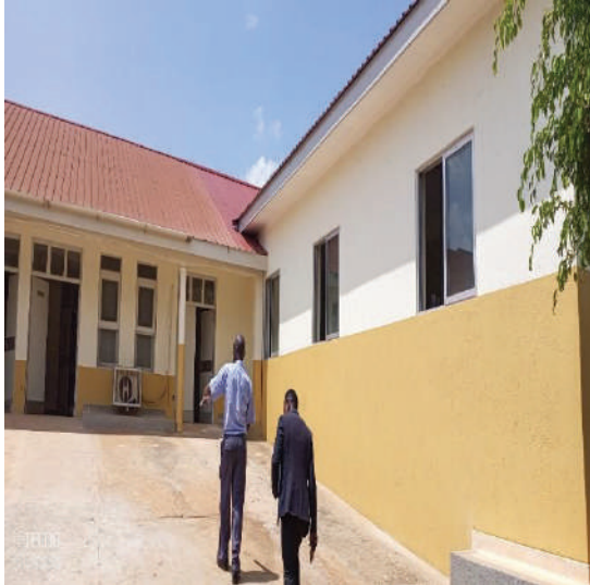
STORES UNDER RENOVATIONS
