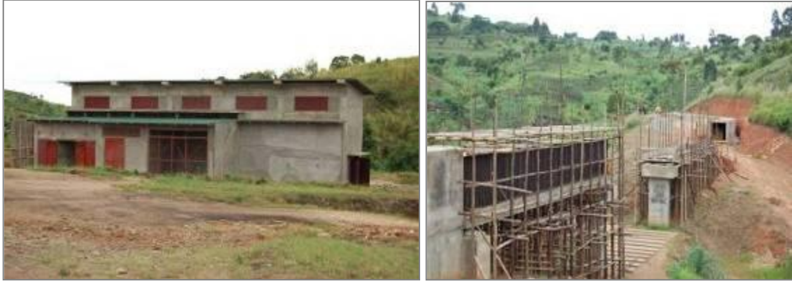
Power House and channel at the stalled Nyagak HEP dam construction
