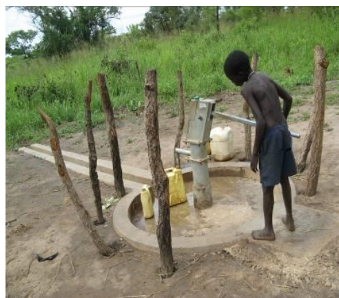
Citing done for borehole Kapo Village Abim Sc, Abim
