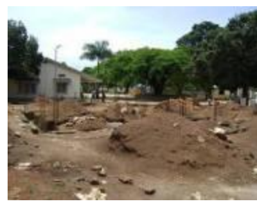
Excavation of information centre
