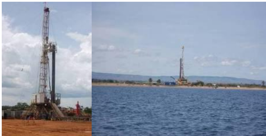
Oil rigs flow testing oil wells in the Albertine Garben
