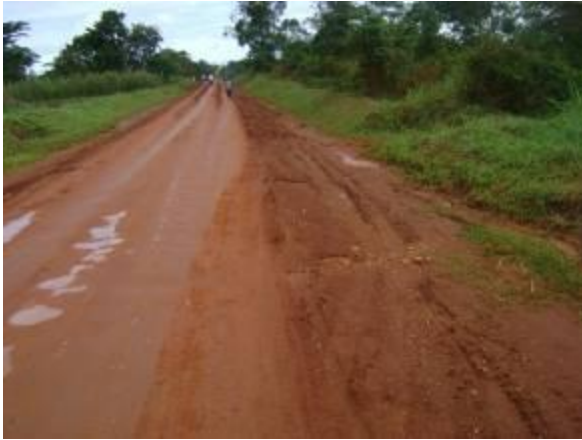
Picture shows a slippery section on Musita – Mayuge road maintained by force account
