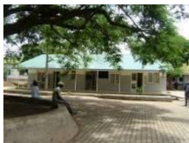
Rehabilitated Old Admin building
