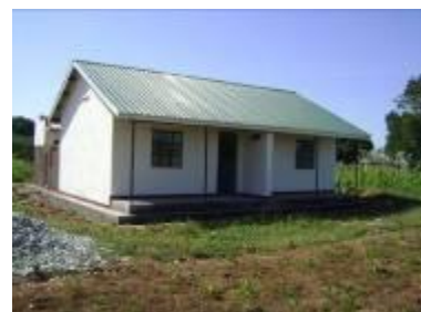
Two in one staff house at Budaka HCIV
