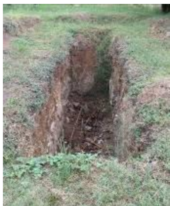
Collapsed latrine in Afere Primary School which has still not been rectified, Nebbi
