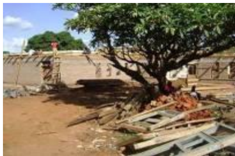
Medical ward under construction
