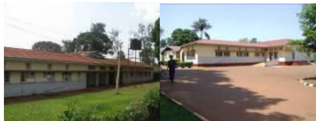
OPD before and after renovation
