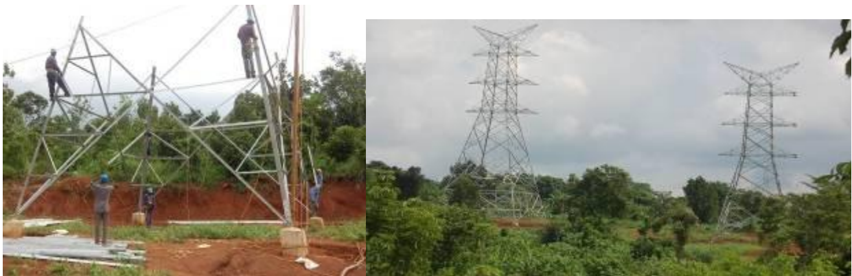
Construction of transmission towers on the Bujagali-Kawanda Transmission line
