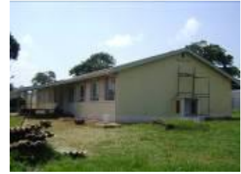
Laboratory under renovation
