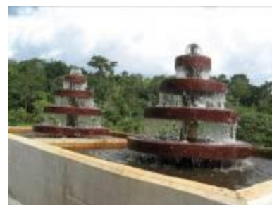
Piped water being treated and ready to be supplied, Kibaale
