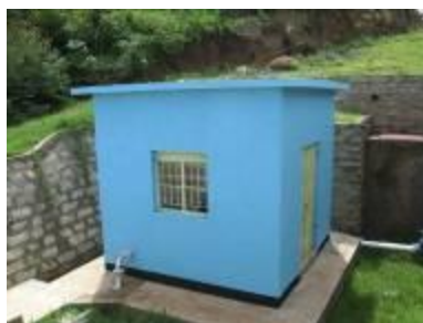
Untreated surface water is being supplied as the pump house still has to be connected to the grid to enable backwashing, Kapchorwa
