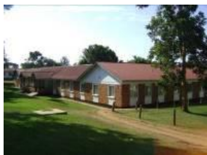
Rehabilitated interns' hostel
