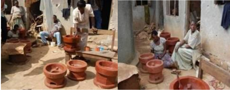
A women's cooperative in Bushenyi constructing energy saving stoves for sale.
