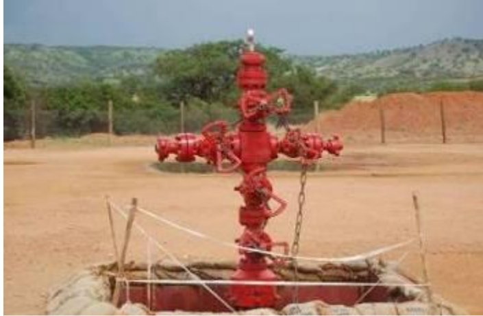
Flow tested and capped oil well in Kaiso-Tonya
