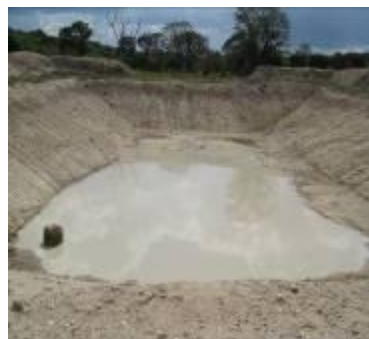
Construction of a valley tank; a shallow well will be constructed using the same water source for domestic consumption, Kiruhura
