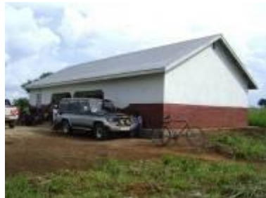
Completed OPD at Anyake HCIV
