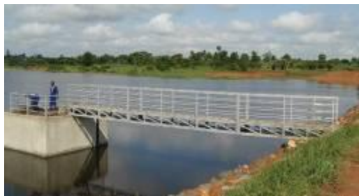
Contractor rectifying defects during the D&L period, Leye dam, Apac
