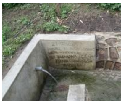
Making use of PAF funds for small spring construction, Bugiri district
