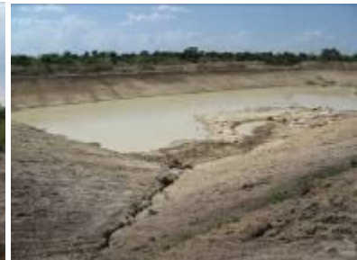
Olelpec dam under construction, Apac
