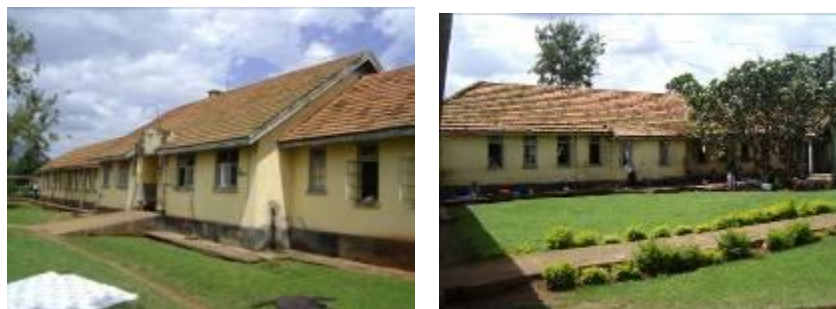
Some of the wards to be rehabilitated.
