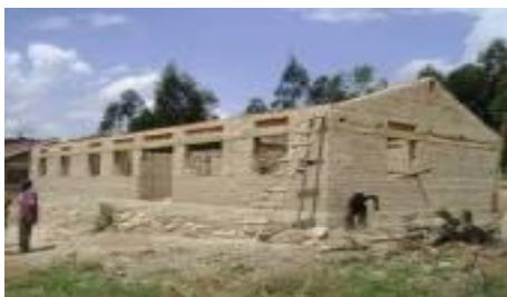
OPD at Biharwe- Nyabuhamba HC III
