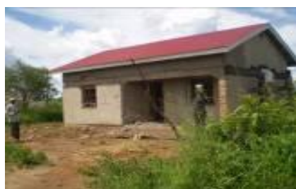
Incomplete staff house at Kungu HCII
