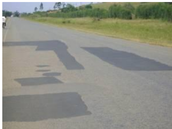
Picture shows pothole patching done on Mbarara – Ibanda road
