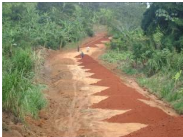
Picture shows on-going gravel works on an un-compacted section of Rutisi – Kigogo road in Wakiso district
