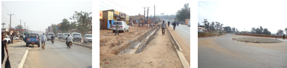
FIGURE 11: VEHICLES PARKED/DRIVEN ON PEDESTRIAN WALKWAYS AT KALERWE, DRAINAGE WORKS AND ROUNDABOUTS WERE INTRODUCED AT SOME SECTIONS OF THE ROAD AS PART OF THE DESIGN CHANGES
