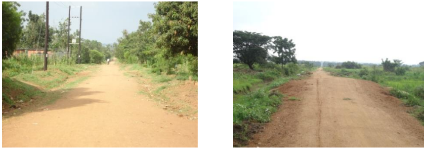
FIGURE 5 ROAD OPENED UP AT NAGONGERA (0+000) AND SWAMP CROSSING AT 3+600 LIKELY TO IMPEDE TRAFFIC IF DRAINAGE STRUCTURES ARE NOT PROPERLY INSTALLED AND SWAMP FILLED TO OVERCOME FLOOD SITUATIONS.
