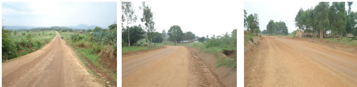
FIGURE 15 COMPLETED SECTIONS OF NAKIGO – BUSOWOBI STILL IN GOOD CONDITION
