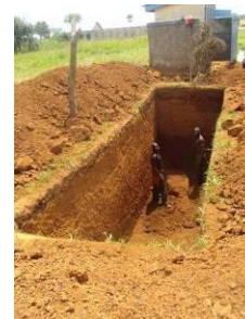
A 3 classroom block and a 2 classroom block at finishes level while the VIP pit latrine was at excavation level.
