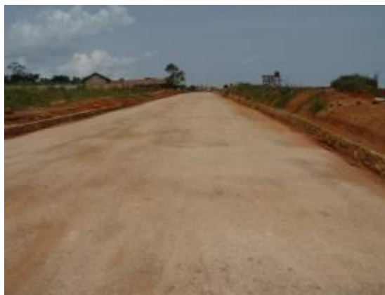
Incomplete By pass link, parked trucks (out of fuel), and primed Kyaliwajala road with stone pitched side drains below
