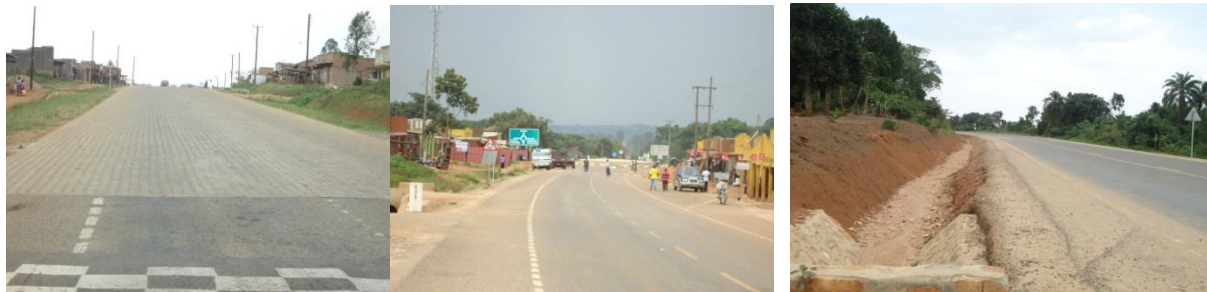
FIGURE 10 KM 22+100 TRIALS SECTION WITH CONCRETE PAVERS, SIDE DRAINS THAT ARE NOT STONE PITCHED ARE ALREADY SILTING AND END OF THE ROAD AT KM 41+000 KAPEKA
