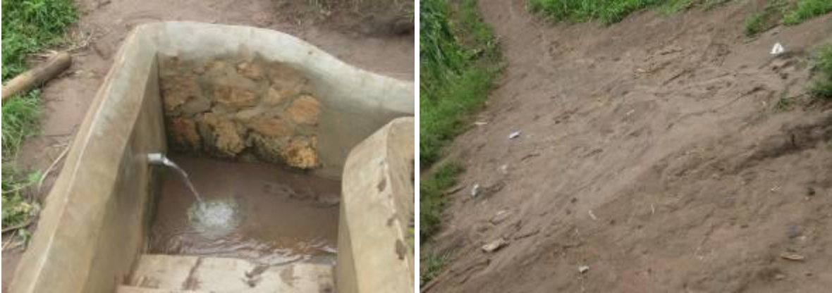
Photos 5&6: Protected spring in Kumi.it is yielding at less than 50% of design capacity due to degradation of the catchment area on the left.(photo taken 21/06/2011
