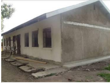
Classroom block under completion
