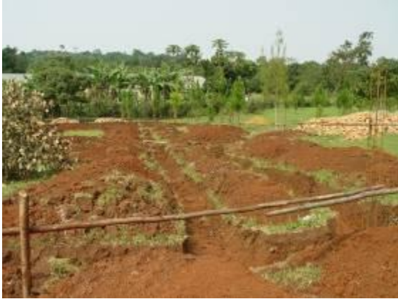
Excavation works at Kibibi SS ICT lab site
