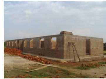
Dormitory block at ring-bim level
