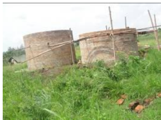
Photos 1&2: On-going construction works for The twin 90 cubic meters Reservoir Tank (on the left) at Nyamarebe piped water system and two Sand Filters (on the right) as part of the treatment plant. (taken on 30/06/2011)
