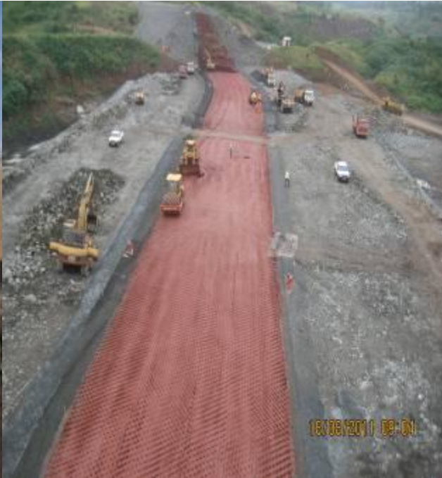
Earthworks, right Embankment
