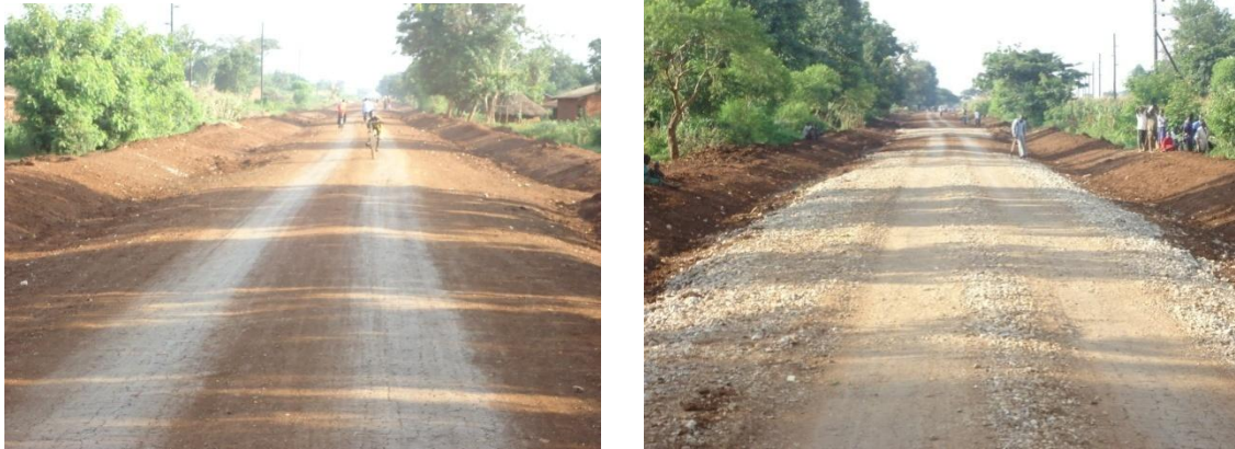
FIGURE 7 GRADING TO THE REQUIRED SLOPE ALONG MUYEMBE-NAMALU ROAD AND APPLYING OF STONE AGGREGATE ALONG MUYEMBE- NAMALU ROAD SO AS TO ACHIEVE A FIRM SURFACE.
