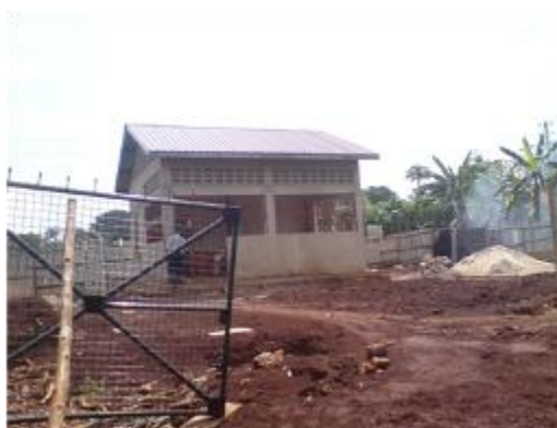
Jinja Regional Referral Hospital: renovated theatre (top left); new incinerator house (top right); works on staff accommodation (bottom left and right)
