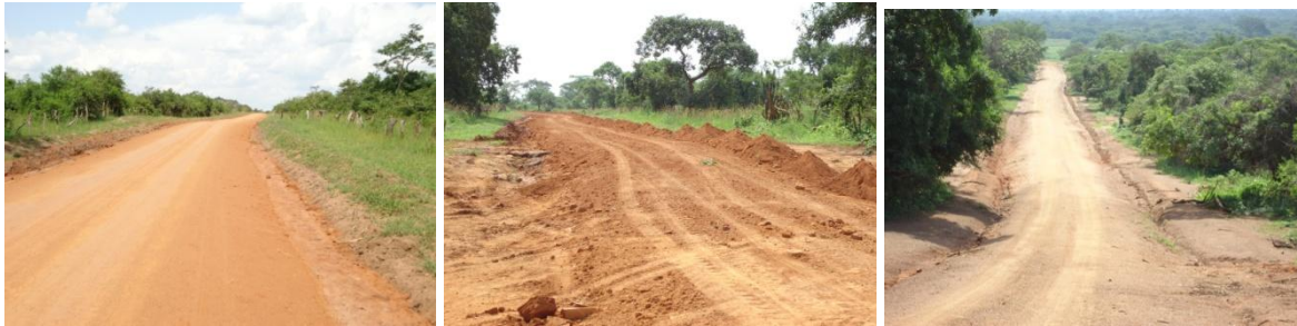
FIGURE 1 COMPLETED GRAVEL WORKS AT 25+200, DUMPING AND SPREADING OF GRAVEL AT 27+000 AND GRADED SECTION AT 29+500
