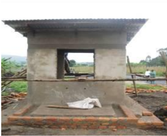
Photos 3&4: Water Kiosk (left) in the Kisoro Chuho-Bunagana project under construction and pipe- laying (right) partially back-filled in progress (Taken on 28/06/2011)
