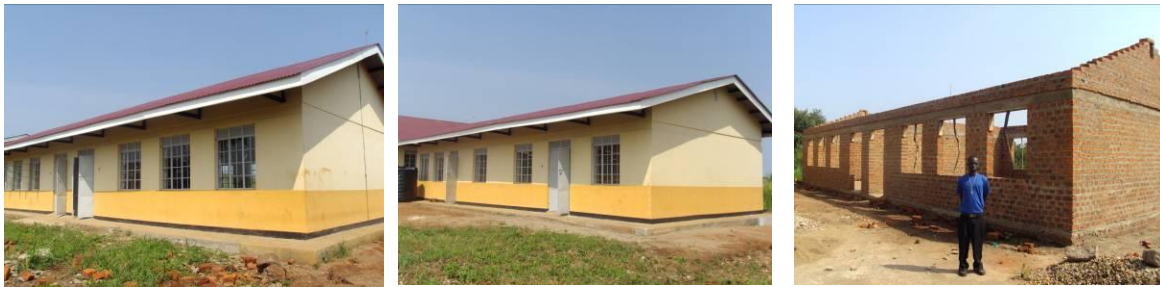
A classroom block, administration block and another 2-classroom block at roofing level
