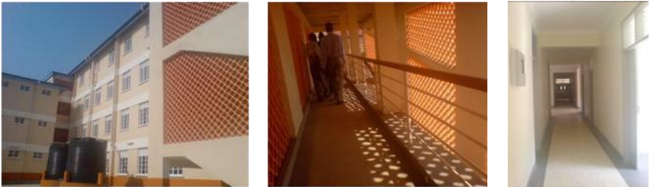
Arua Regional Referral Hospital: external works on the new ward building (left); disabled access ramp in the new ward building (centre); corridor inside new ward building (right)
