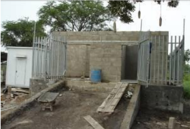
New Transmission Site under construction at Eregu
