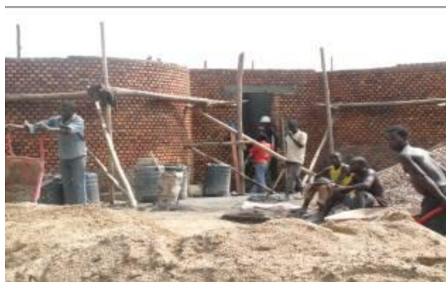
Photos 1&2: On-going construction works for The twin 90 cubic meters Reservoir Tank (on the left) at Nyamarebe piped water system and two Sand Filters (on the right) as part of the treatment plant. (taken on 30/06/2011)
