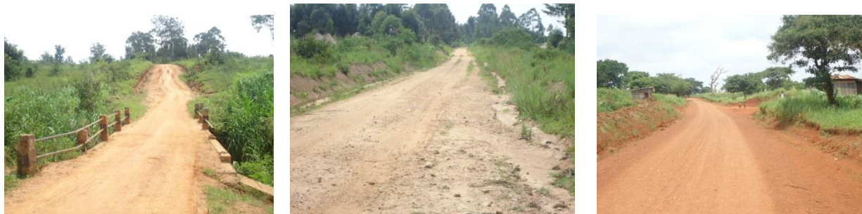
FIGURE 3 AYAVU BRIDGE AT 0+000, POORLY CONSTRUCTED SECTION AT 2+700 AND COMPLETED GRAVEL SECTION AT 25+300
