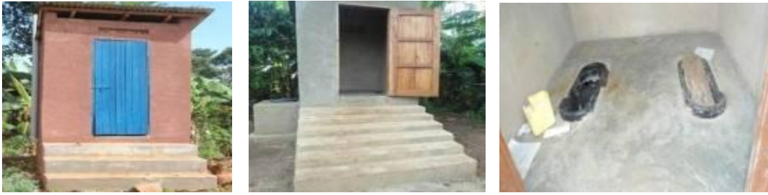
Ecosans constructed by WSDF-C in Kasanje - Wakiso and Ziobwe- Luweero respectively. Extreme left is 1 scot hole in use and another reserved
