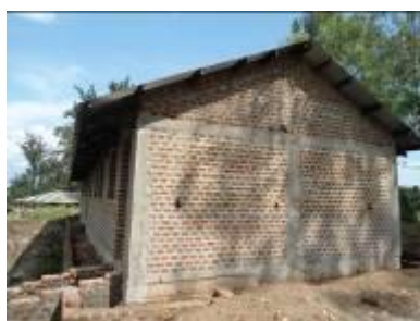
A 2 classroom block at finishes level at Kisomoro P/S
