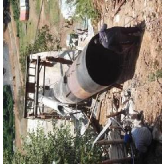
Ongoing construction works and alignment of penstocks at Buseruka
