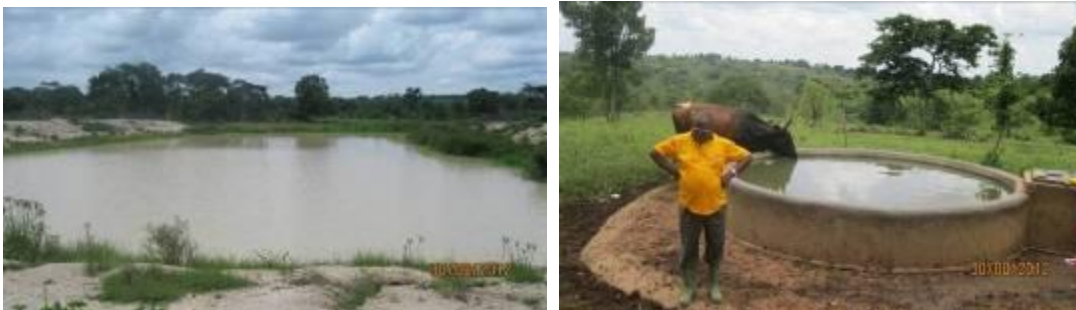
Newly constructed valley dam and newly constructed water trough
