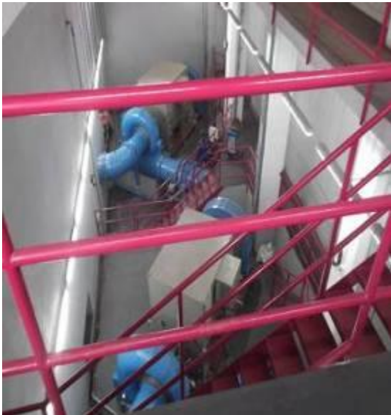
Dam construction at Nyagak HPP Complete and 2x1.75MW turbines at Nyagak HPP
