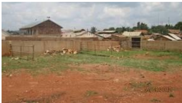
Nsooba market area under construction
