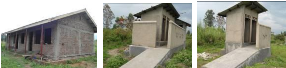
A 2 classroom block, a twin workshop, an MV workshop at roofing level, an administration block a 5-stance and a 2-stance VIP pit latrines constructed at Kisomoro Technical School under the Presidential Pledges
