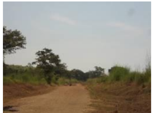
A SECTION OF ADJUMANI – SINYANYA ROAD, WHERE ROUTINE MAINTENANCE BY LABOUR BASED CONTRACTORS WAS ONGOING
