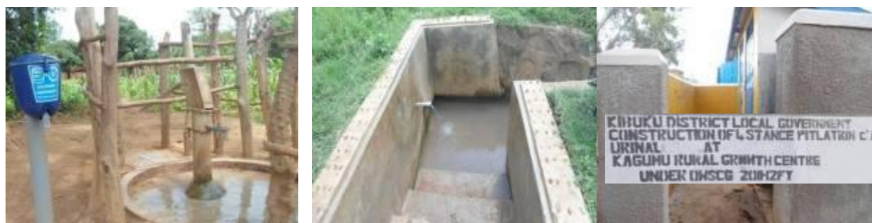
A borehole in Kagumu with a chlorine dozer (left), a spring in Bupalama Kagumu S/C made in 2010/11 and reported on in 2011/12(middle); a 4 stance latrine at Kagumu RGC. The O&M of the latrine is poor already.
