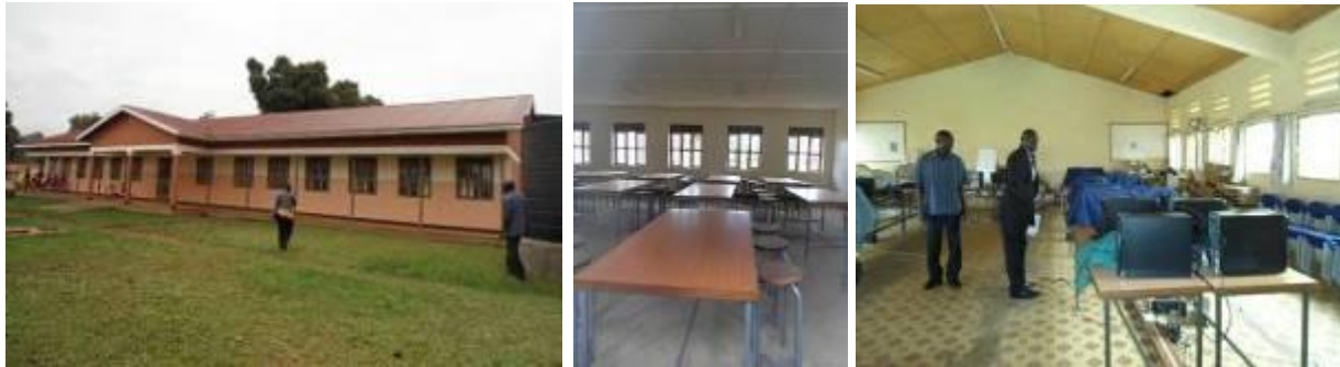
Completed structure, furniture and procured computers at Sacred Heart
