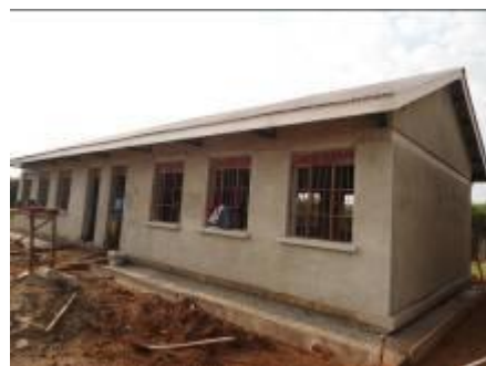
A 2 classroom block at finishes level Kacwekano P/S
