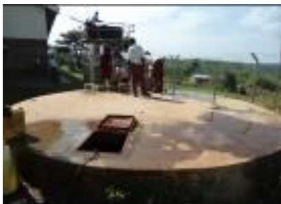
The underground water tank at Butoloogo Seed S.S.
