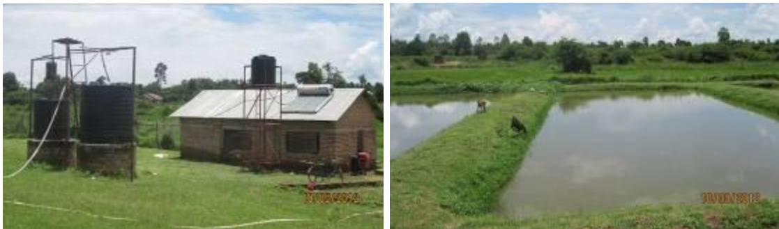
Left: Hatchery building with water heater on top of the roof Right: ACF fish ponds
