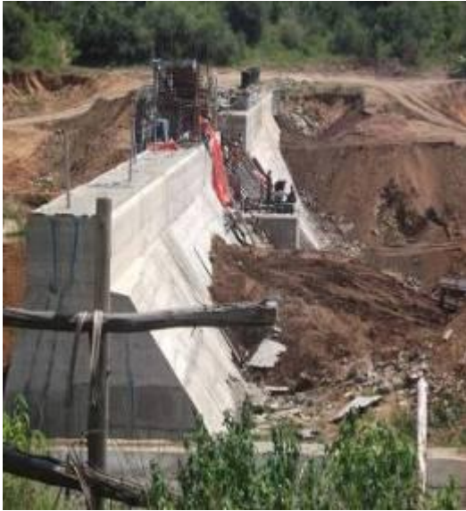
Ongoing construction works and alignment of penstocks at Buseruka
