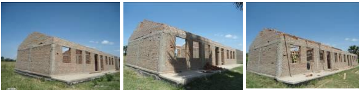
3 blocks of classrooms (2 & 2 & 3 classrooms) at roofing level at Rwebisengo S.S.
