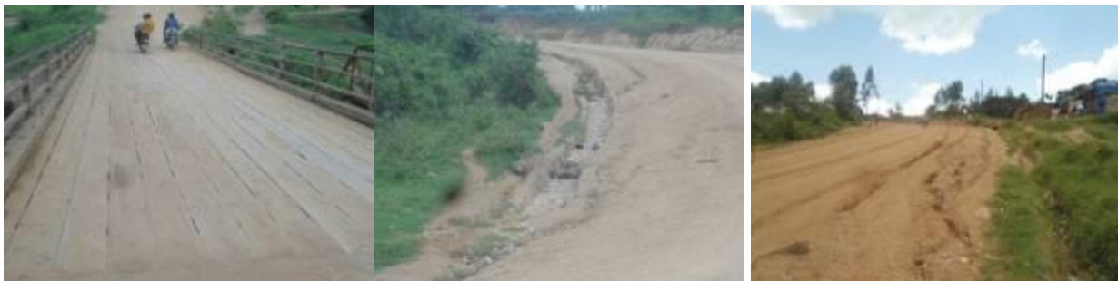
Timber decking on Katete bridge (left); open drainage channel with rubbish (centre); and gulleys forming on the road surface alongside the drainage. (right) on Rwizi Lane.
