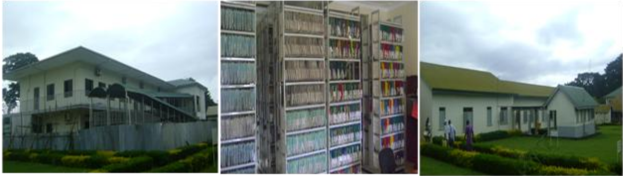
Lira Regional Referral Hospital: Intensive Care Unit (left); storage shelves for medical records (centre); renovation of female ward (right)
