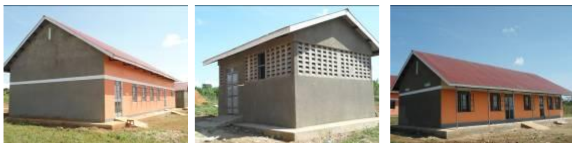
A dining hall, a kitchen and a staff house constructed at Lutunku CP
