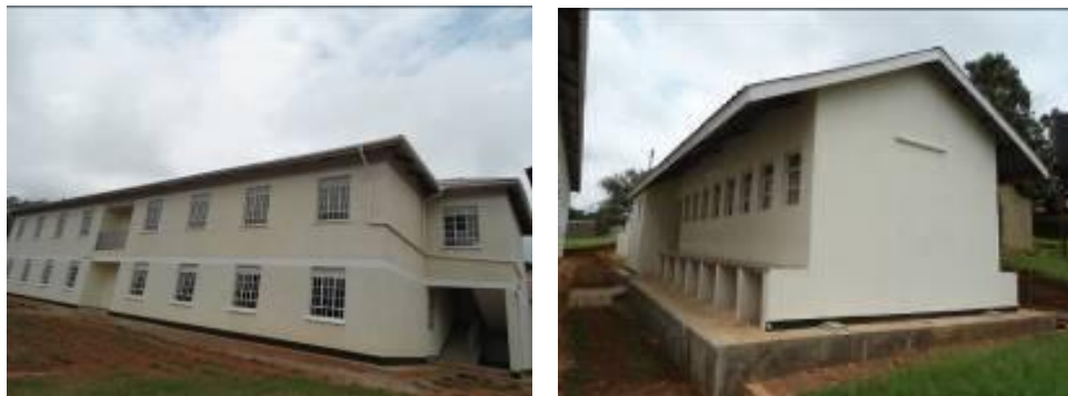
The storied dormitory block and water born toilets at Nkokonjeru PTC
