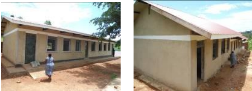
A 2 classroom block and a 3 classroom block at Kirowooza P/S
