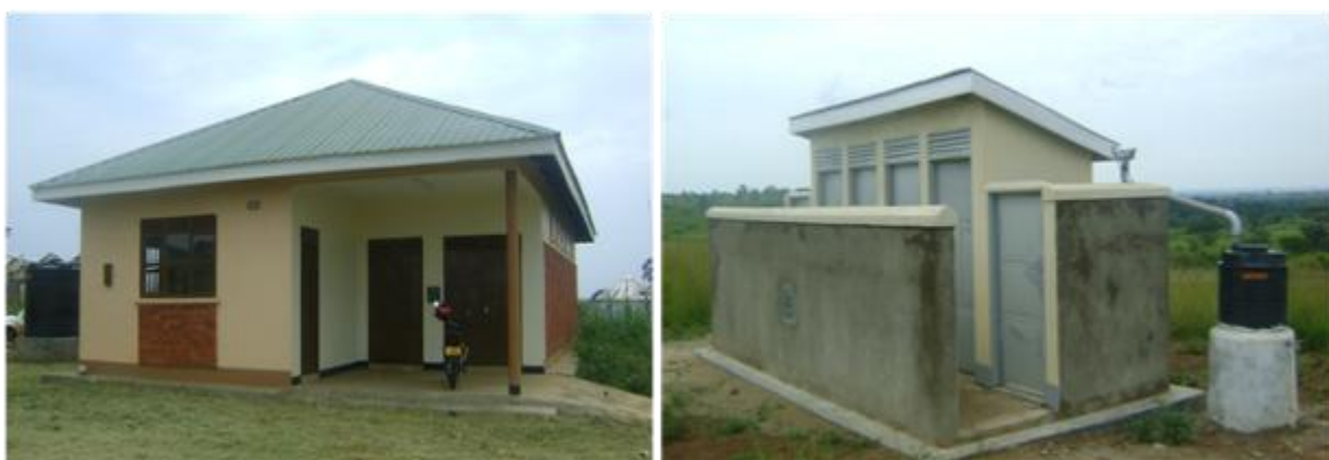
Nwoya district PHC development: cold chain store at the district headquarters (left); drainable pit latrine at Aparanga HCII (right)
