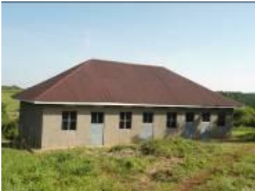
A completed staff house at Rusekere S.S.
