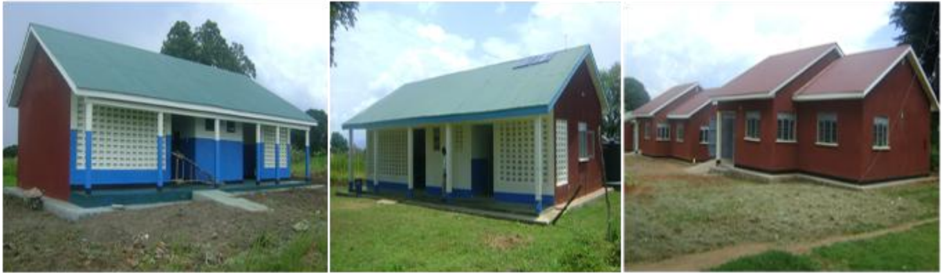
Adjumani district PHC development: Left to right: OPD Magburu HCII (left); OPD Nyumanzi HCII (centre); Doctors houses Adjumani Hospital (right)
