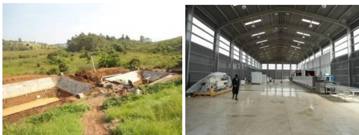
Lining of lagoons and installed biscuit and bakery lines at PIBID
