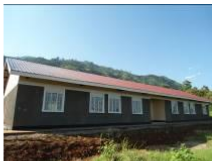
A completed dormitory block at Semiliki High under the Presidential Pledge
