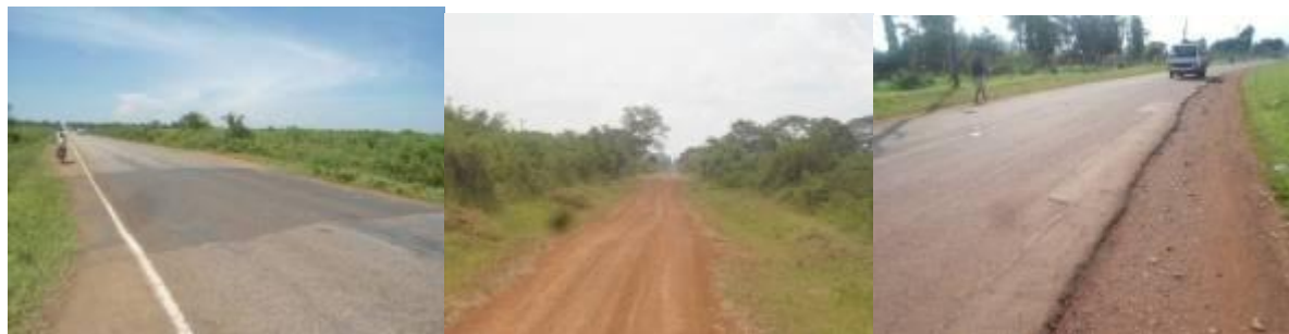
A patched section of NakalamaTirinyi road (left); Graded section of KamuliNamasagalil road. Note that LBC contracts of road side slashing had been implemented (centre); reinstating of the road edge on Kimaka Access next to the Jinja Airfield. (right)
