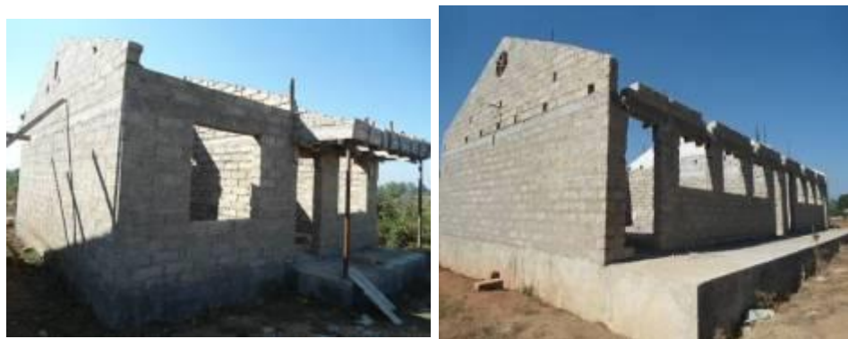
Another 2 bedroom housed abandoned at roofing level and another block abandoned at roofing level at Kalisizo S.S.
