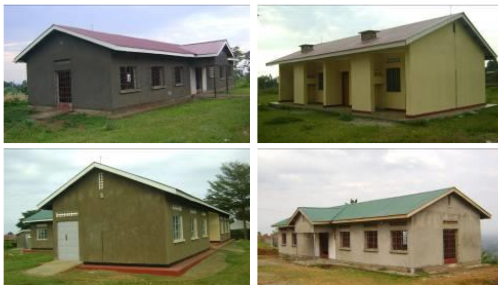
Clockwise, Maternity ward at Bungoho-Mutoto HCIII, Staff house at Namanyonyi HCII, Maternity ward at Naiku HCIII, and Maternity ward at Namawanga HCIII,
