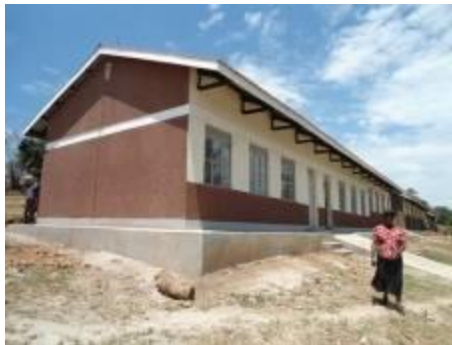
A 3 classroom block constructed at Bujubi P/S
