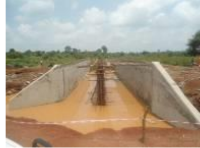
(Left); Spreading and compacting of stabilised subbase material (G7) at Km 5+000. (Centre); Box culvert with decking yet to be constructed at Km 67+00. (Right); Completed Box Culvert at Km 64+000
