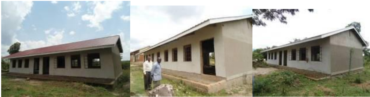
2 blocks each with 2 classrooms and a science laboratory constructed at Kinyogoga Seed with WB funding
