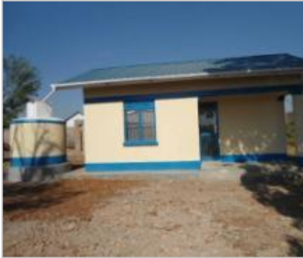
Tank and an office block
