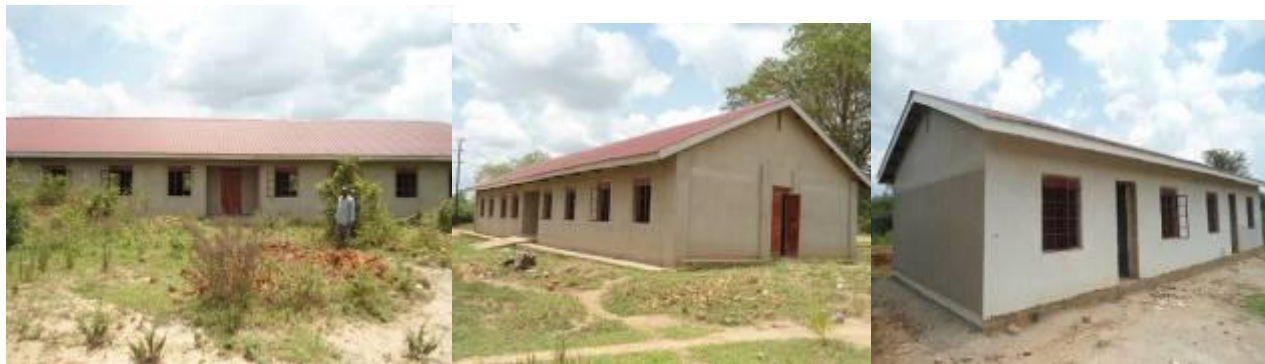
The 2 dormitories and a 4 unit teachers' house constructed under the Presidential Pledge at Kinyogoga Seed S.S
