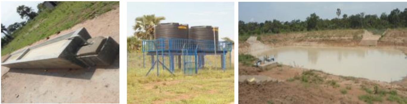
Clockwise: One of the 3 cattle troughs, tanks on 2 meter stands and the Nakakabal Valley Tank
