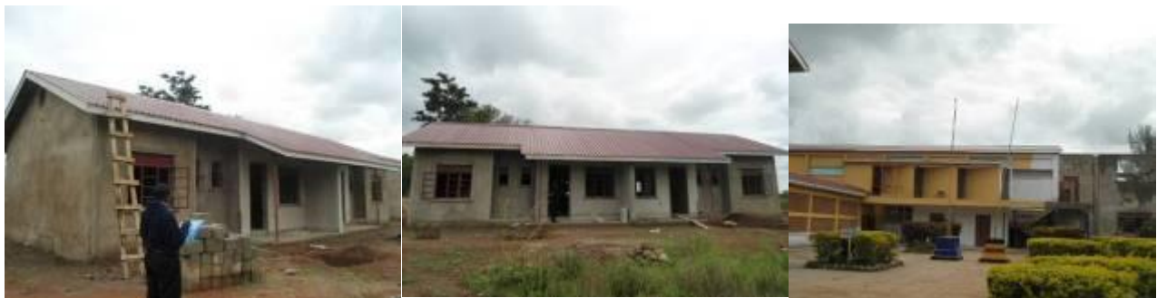
Two new blocks of teachers' houses and extension of the main hall at Teso College Aloet.
