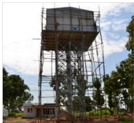
on going works at a reservoir tank
