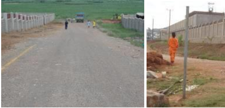
Completed 100 meter road extension and vandalized road furniture
