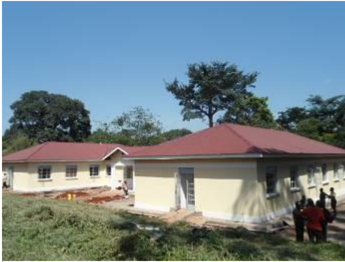
Students' hostel constructed at Nyabyeya Forestry College
