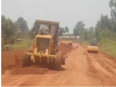
(Left); Spreading and compacting of stabilised subbase material (G7) at Km 5+000. (Centre); Box culvert with decking yet to be constructed at Km 67+00. (Right); Completed Box Culvert at Km 64+000
