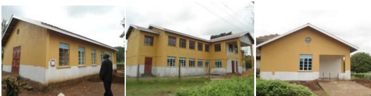
Structures under renovation at Teso College Aloet.
