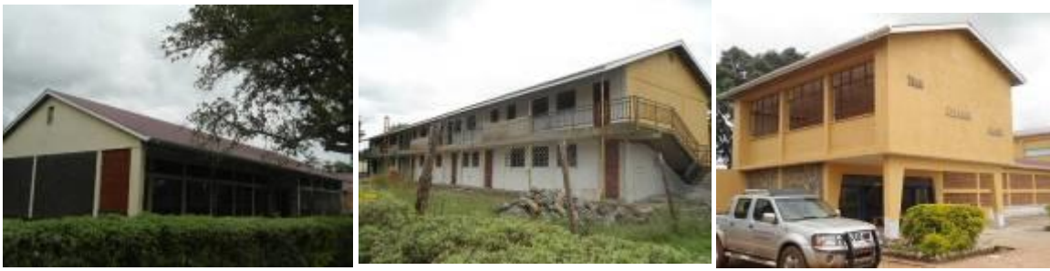
A new 300 seater library, a new storied block with two science laboratories, five classrooms and an ICT laboratory and an administration block renovated at Teso College Aloet.
