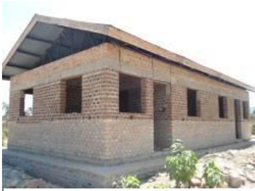
The teachers' house under construction at Kibaale S.S
