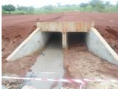
(Left); Spreading and compacting of stabilised subbase material (G7) at Km 5+000. (Centre); Box culvert with decking yet to be constructed at Km 67+00. (Right); Completed Box Culvert at Km 64+000
