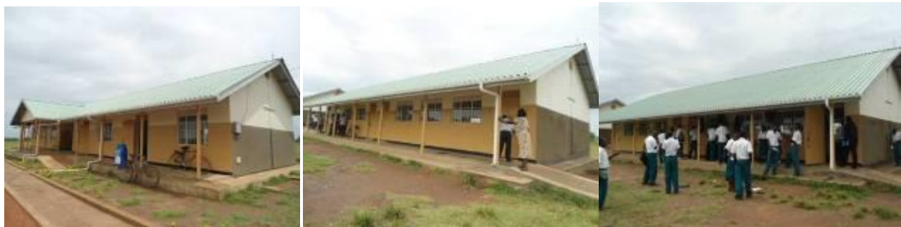
An administration block, a 2 classroom block and a multi-purpose room completed at Atatur S.S.
