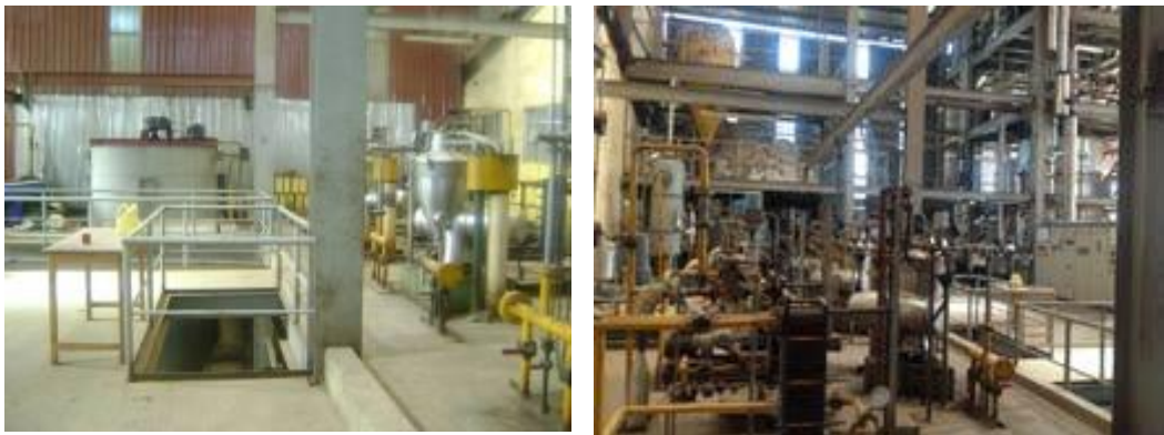
ACF funded Oil refinery at Mount Meru Millers factory Lira district
