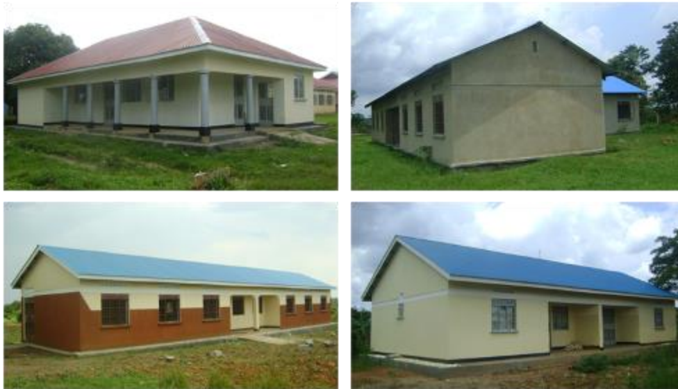
Clockwise: OPD renovation at Dokolo HCIV, Maternity ward construction at Anyacoto HCIII, Staff house construction at Bardyang HCII construction of maternity ward at Adok HCIII
