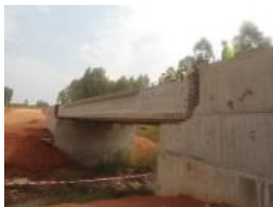
(Left); Completed first seal works at Km 22+400 -Manibe junction. (Centre); A bridge at Km 34+400 with decking works on going with the approaching sections not worked on. (Right); Concrete along the edge of the road at Km 45+625 to protect it from edge failure caused by motorcycles.
