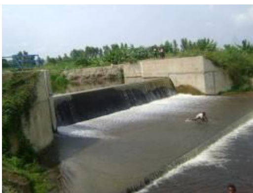
Mubuku completed Wier
