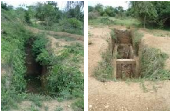
The 2 VIP pit latrines that stalled at excavation and ground-bim level respectively at Kinyogoga Seed under WB funding.
