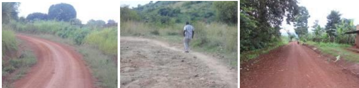
Kigorobya-Kibiro (6.5 Kms) (Left); A graded and re-gravelled section (Centre); A rock section at the escarpment. (Right); A graded and re-gravelled section at the beginning of Buliindi-Dwoli (17 Kms)road.
