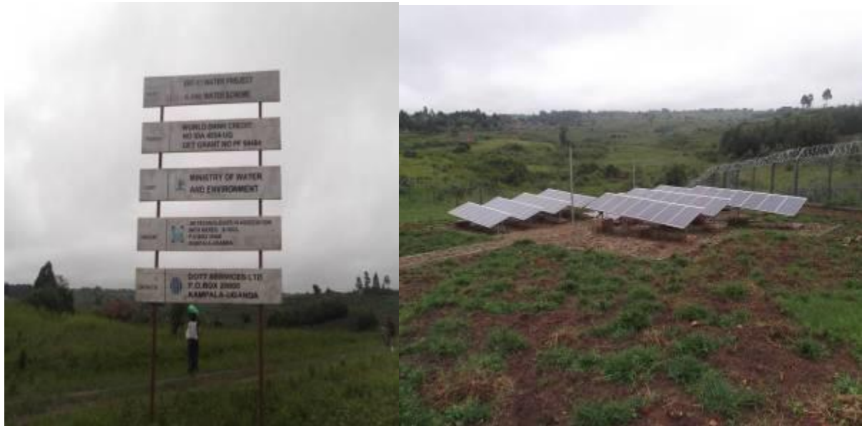
Installation of solar water panels in Alangi, Zombo district
