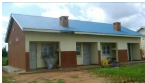
Bottom: completed staff houses at Agulurude HCIII and at Otwal HCIII.
