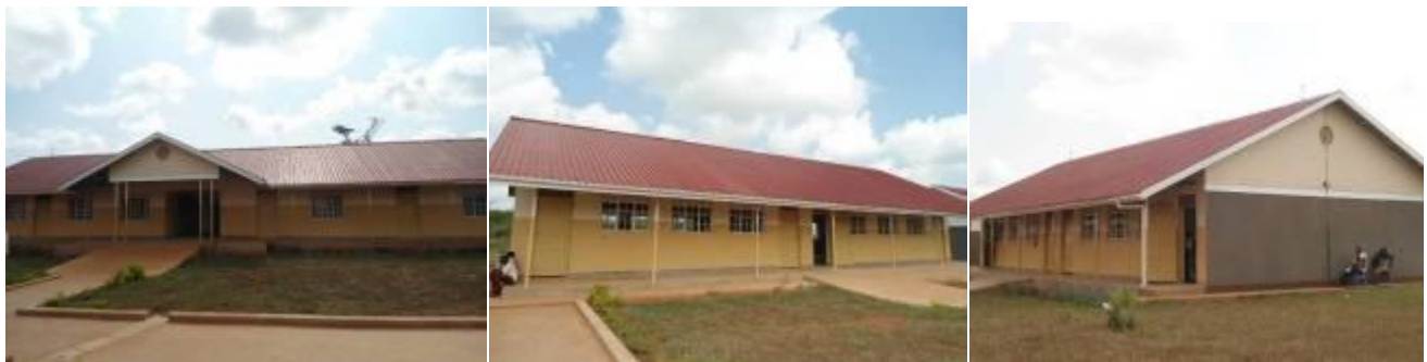
An administration block, Main hall and 2 classroom block completed at Wakyato Seed S.S under ADB IV
