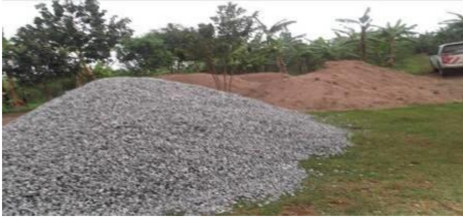
Materials for the construction of tower points on the Mbarara-Nkenda Project
