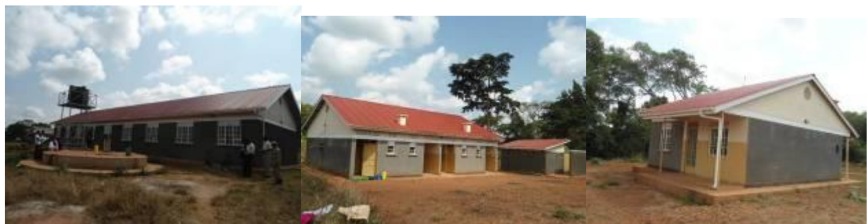
Science laboratory, a 4 unit teachers' house and the head teacher's house completed at Wakyato S.S under ADB IV
