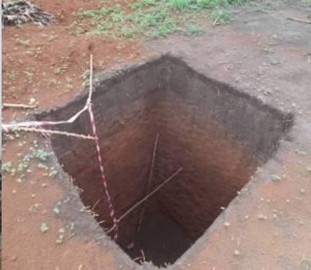
Initial excavation works for the construction of tower points on the Mbarara-Nkenda transmission line Project
