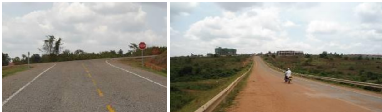
Installed road signage and road marking on First Street and silted surface of the by-pass link with UNBS and Bweyogere hospital structures in the background
