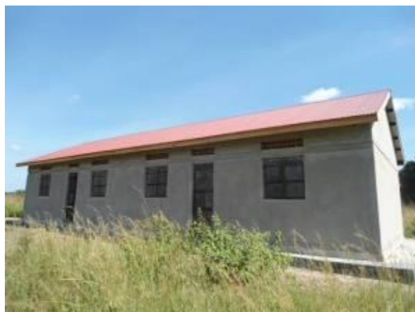
A 4 unit teachers' house constructed at Ngariam Seed S.S.
