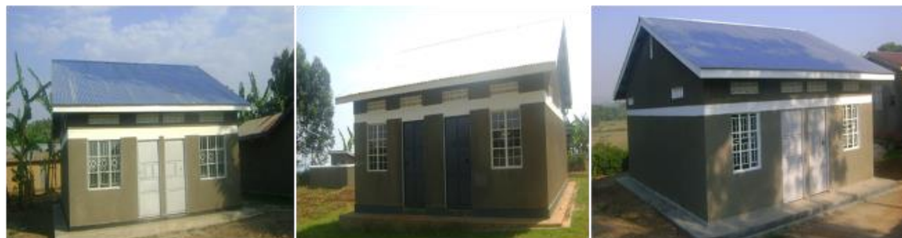
Left to Right: Completed staff junior houses at: Kigaga HCII, Nyakabale HCII and Bwizibwera HCIV
