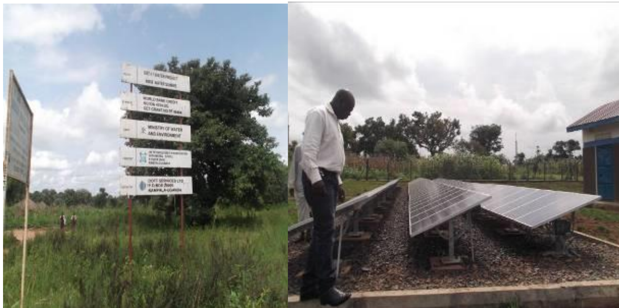
Installation of solar water panels in Midogo (Yumbe district)
