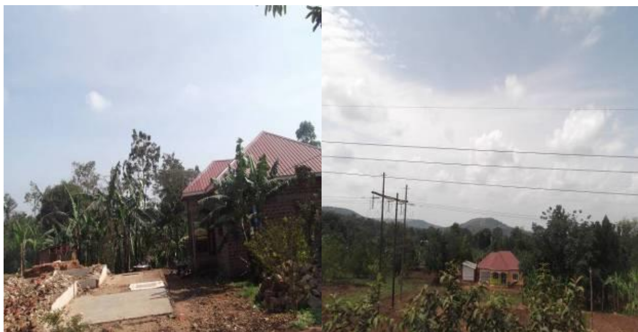
Resettlement houses constructed by the PAPs on Masaka-Kawanda Transmission line after they received their compensation package
