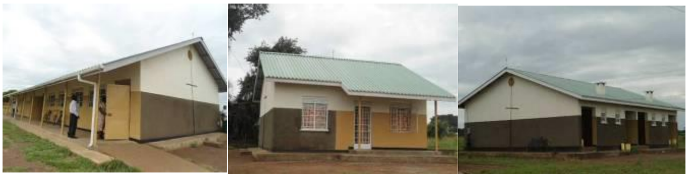
A science laboratory, head teacher's house and a 4 unit teachers' house constructed at Atatur S.S
