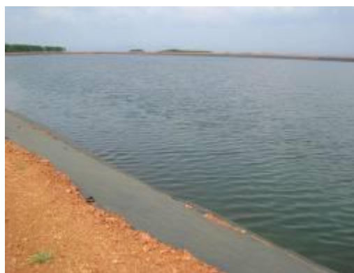
Mubuku water storage reservoir
