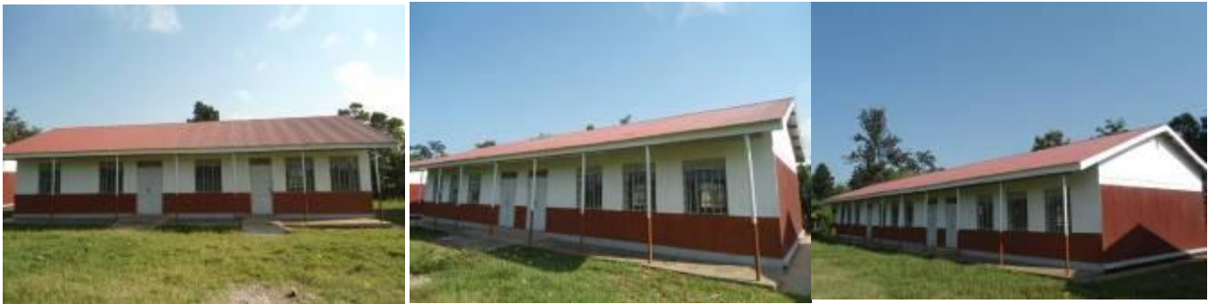
An administration block, a 2 classroom block, a 3 classroom block constructed at Walibo S.S. under the Presidential Pledge.
