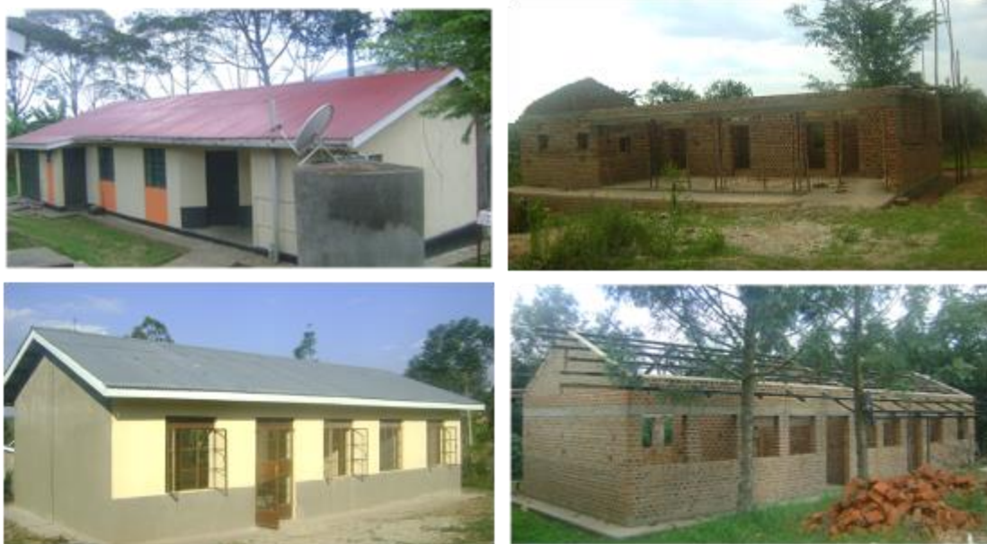
Top: Rehabilitated doctor's house Ruhoko HCIV, and OPD Rwensambya HCII
