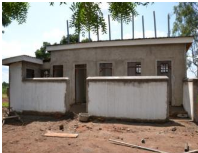
Construction works for a 5 stance Ecosan at a primary school
