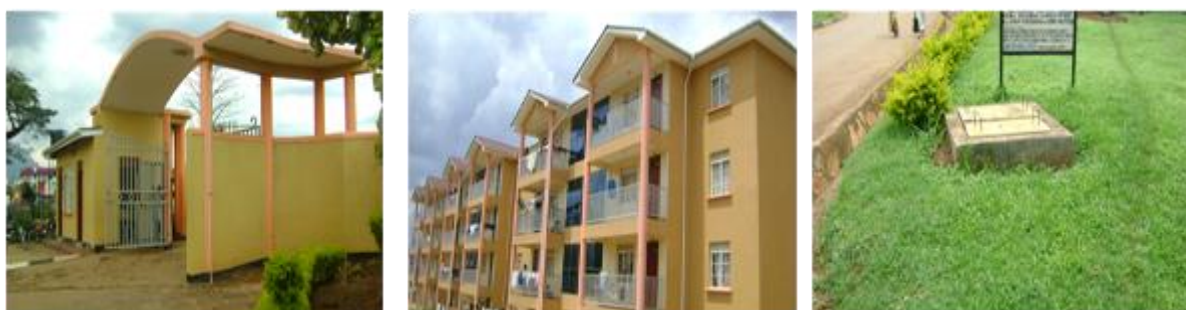
Left to right: Completed gate, Staff quarters and sewerage line Mbale Regional Referral Hospital
