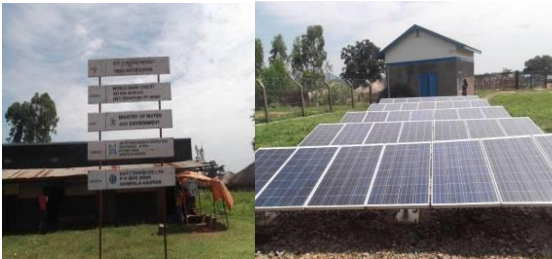
Installation of Solar Water Pumping System in Kubala (Arua district)
