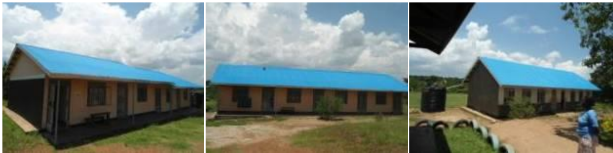
The 2 blocks of teachers' houses and the 2 classroom block constructed at Nabalanga P/S
