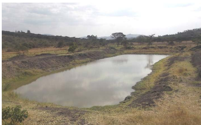
A valley tank excavated at Kakama & Farm Ltd in Masha Sub County in Isingiro district
