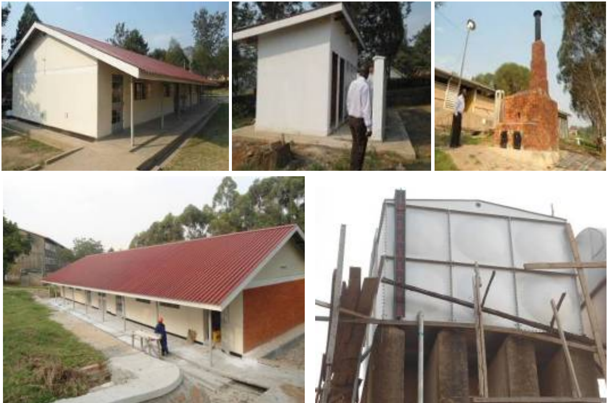
Clockwise; a completed two classroom block, a five stance VIP latrine at finish level, an incinerator, a science laboratory and a 50,000 litre water tank at Bweranyangi Girls
