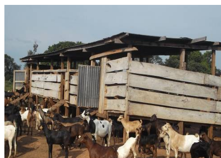
Newly constructed goat house at Kasolwe farm
