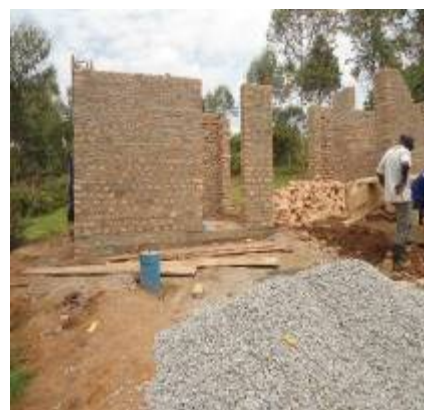
Left to right: Construction works of a twin reservoir tank of 220m 3 , a water office block, and a pump house
