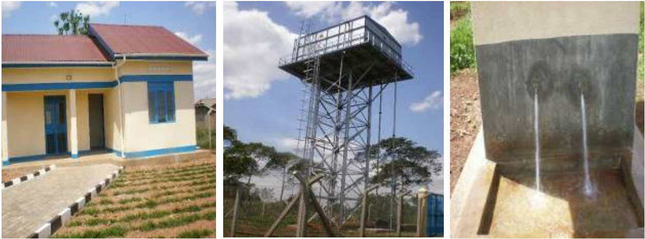
Left to right: A completed water office, reservoir tank, and water flowing at one of the kiosks
