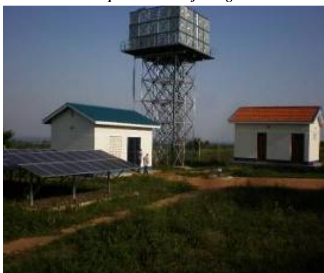
Left to right: Installed solar panels, pump house, reservoir tank, and attendant's house. Completed water office block in Singila RGC in Nebbi district
