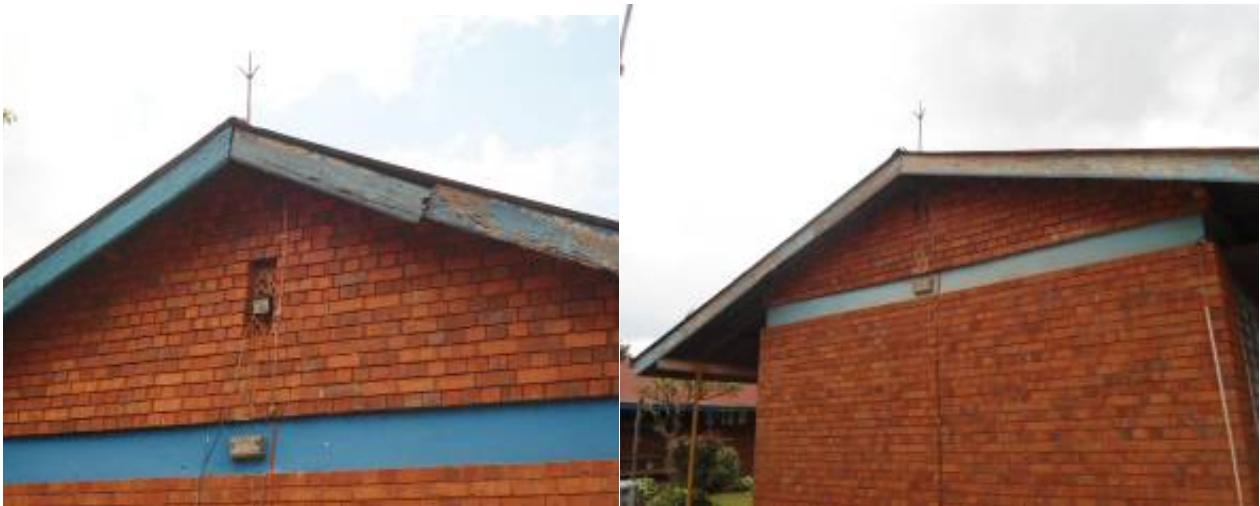
Lightning conductors installed on two of the blocks at Ntinda School for the deaf
