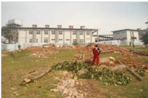
Site clearance for the maternity ward complex
