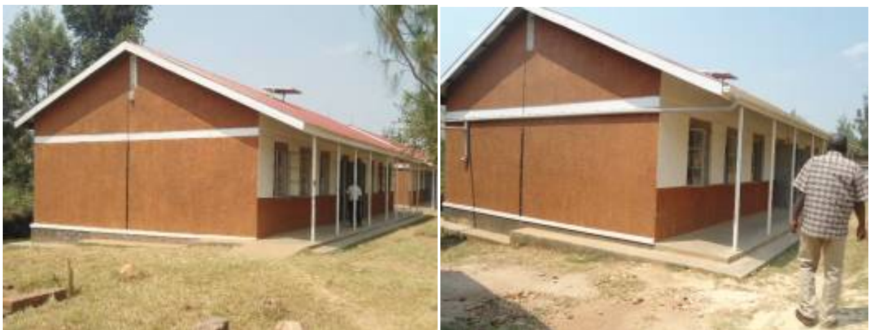
Two blocks of two classrooms each completed at Bwanga S.S.
