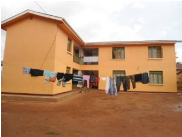
A four unit storied staff house completed at Kawempe Church of Uganda P/S
