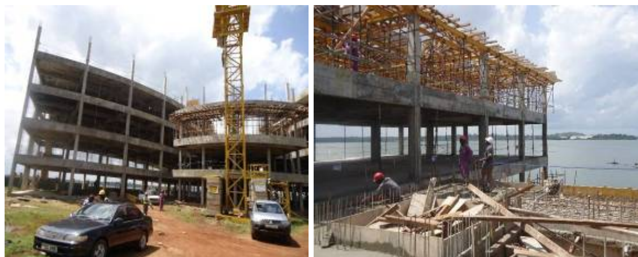
L-R: Completed Building frame; ongoing construction works of the data center
