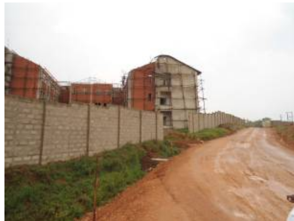
L-R: Stabilised sub base section and graveled section of road around the factory complex, in the background is the fence of the quality assurance block at Nyaruzinga, Bushenyi district
