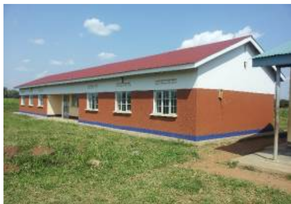
Completed maternity ward Kitgum HCIII
