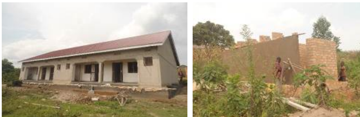
Staff house pit latrine under construction works at Kitanga HCIII
