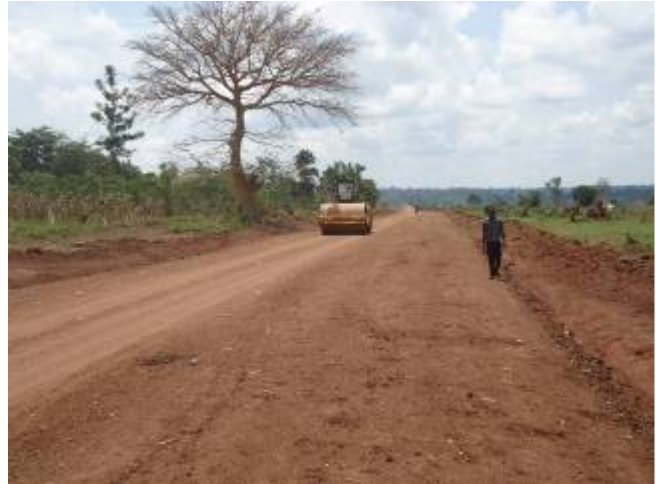
Right: Levelling of access road
