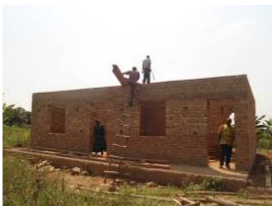
The staff house at roofing level at Lutunku Community Polytechnic
