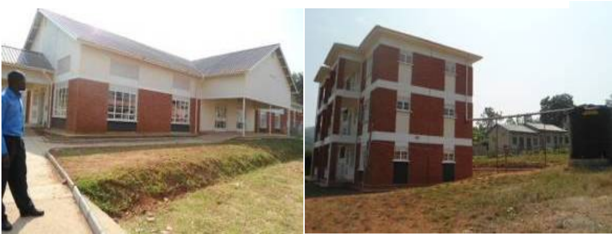
Left: A multipurpose block and Right: a storied self contained staff house completed at Muntuyera High School
