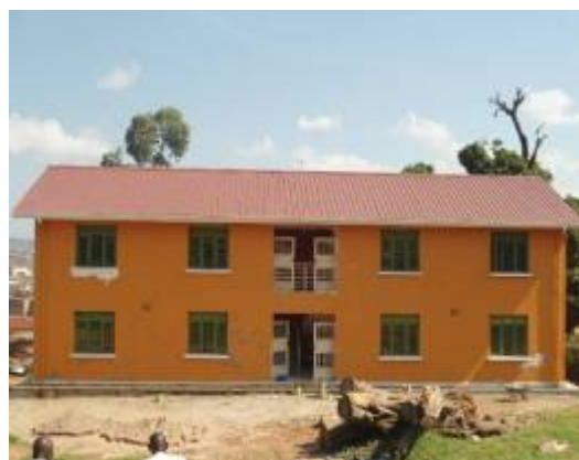
The staff house at Naggulu-Katali P/S at finishes level
