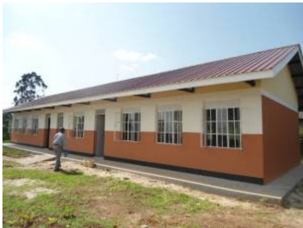
The completed classroom block at Mukumbwe P/ S
