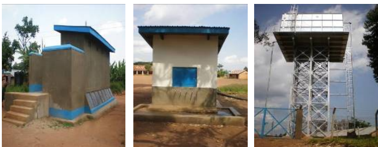
Left to right: completed school eco-san toilet at Assumptio Catholic school in paidha town, water kiosk and reservoir
