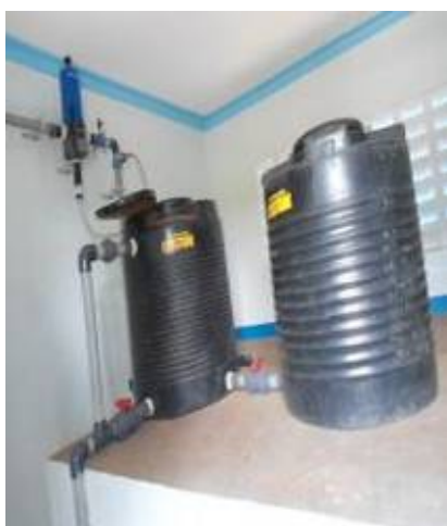
Left to right: Chlorine dozing equipments, tools supplied by the contractor for O&M, and household connection
