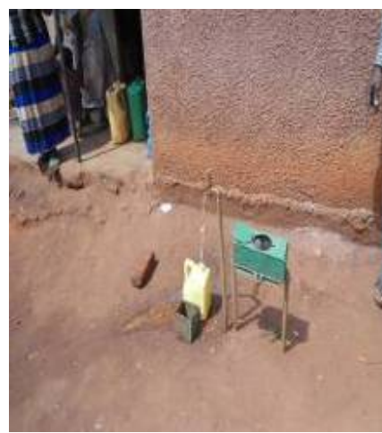
Left to right: Chlorine dozing equipments, tools supplied by the contractor for O&M, and household connection
