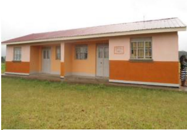
The completed two unit staff house at Kaabong Nursing Training Institute
