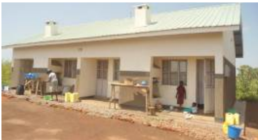
Four-in-one staff house at Lalogi HC IV, Gem Parish, Lalogi Sub County in Gulu District
