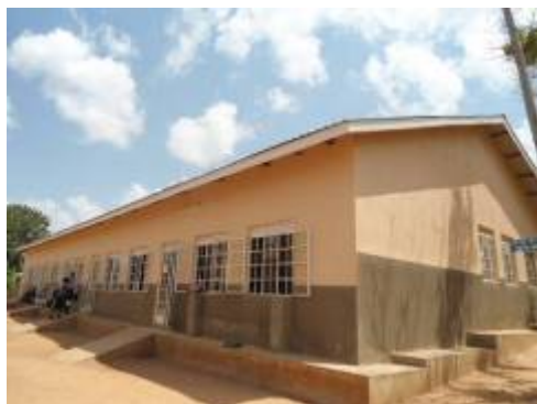
The renovated seven classroom block at Kisugu C/U
