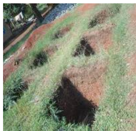
Left to right: Connections awaiting pressure testing, a booster station house, and foundation Excavations for installation of the 40m 3 reservoir tank
