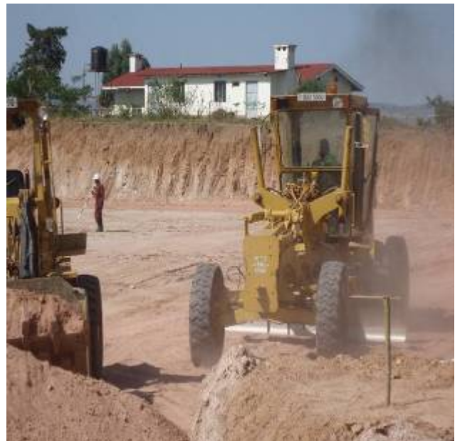
Left: Completed leveling works Right: Ongoing earthworks on new Mbarara North Substation
