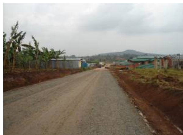
L-R: Stabilised sub base section and graveled section of road around the factory complex, in the background is the fence of the quality assurance block at Nyaruzinga, Bushenyi district
