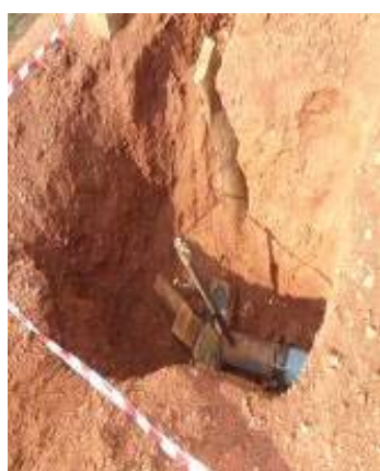
Left to right: Connections awaiting pressure testing, a booster station house, and foundation Excavations for installation of the 40m 3 reservoir tank
