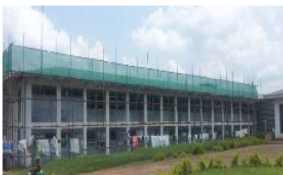
Ongoing renovation works on the existing T-block at Kiryandongo Hospital
