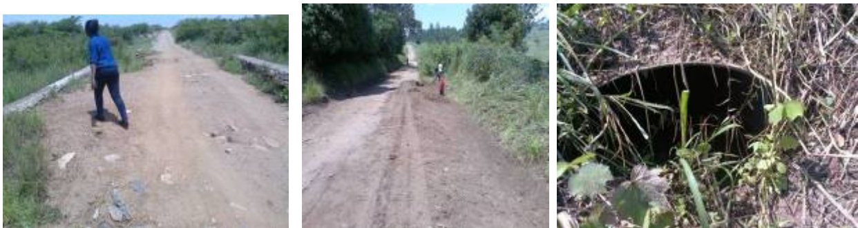
Nebbi District: Left; A completed section of Achwera bridge approach; (centre): Routine manual maintenance works on going along Nebbi-Kei-Goli road; Right: An Armco culvert along Nebbi-Kei-Goli road covered with bush
