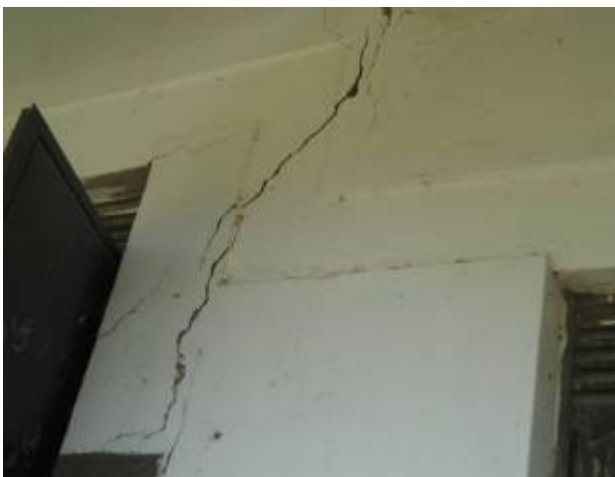
Some of the structural cracks on the three classroom block at Packwach S.S. indicating that the contractor did shoddy work
