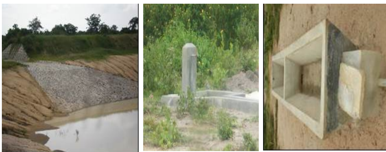
Left to right; Spillway, public tap stand, and cattle trough at Nyamiringa
