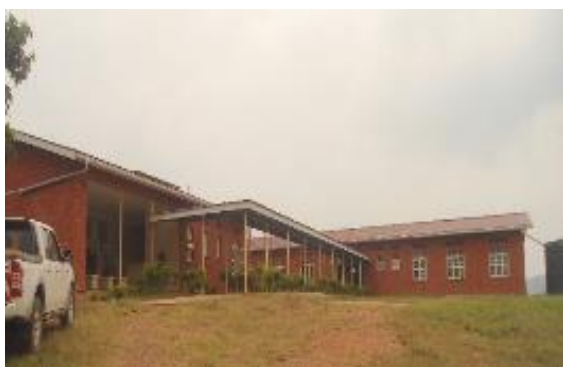
Newly constructed Kisozi HC III
