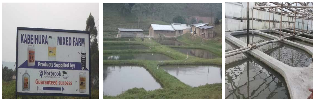
Middle; Rehabilitated fish ponds, right; newly constructed tanks at Kabeihura Mixed Farm Bushenyi district
