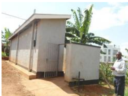
The 10 stance VIP pit latrine completed at Summit View Army P/S
