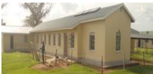
General ward at Awach HC IV in Gulu District under renovation
