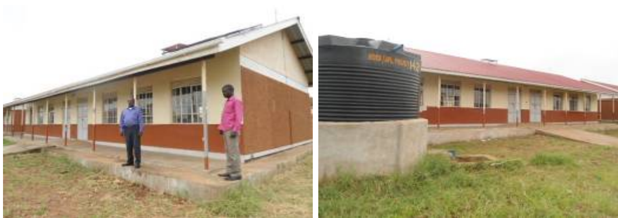
The new classrooms that were completed at Kaabong S.S
