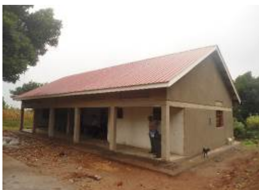
OPD under construction at Mpugwe HCIII
