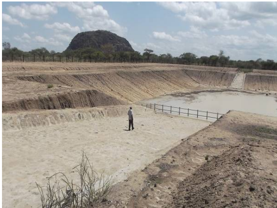
Waliwal valley tank in Kotido district
