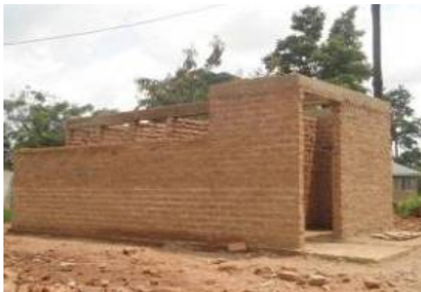
From Top left: The two classroom block at slab level, the two girls' dormitories at ring beam level, and one of the six stance VIP pit latrines at Canon Lawrence PTC - Lira
