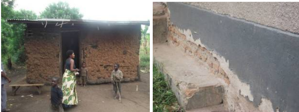
Left: A PAP in Kitwamba Sub County, Kasese district cannot make developments on the house and yet payment has delayed to enable her relocate. Right: Shoddy resettlement house in Rwimi Sub county, Kabarole district
