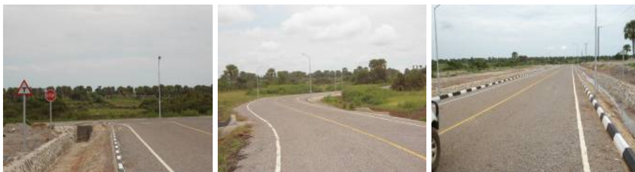
L-C: Completed Temele road, with side drains, road marking, signage and lighting infrastructure.
