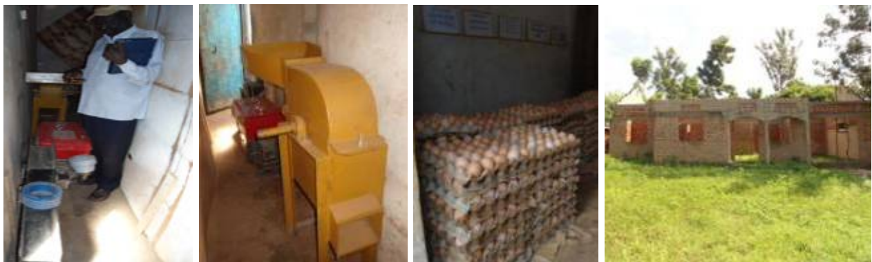
L-R: Vice chairperson showing a diesel engine, mixer and some of the eggs from the members. Far right is the shell to house the equipment awaiting roofing
