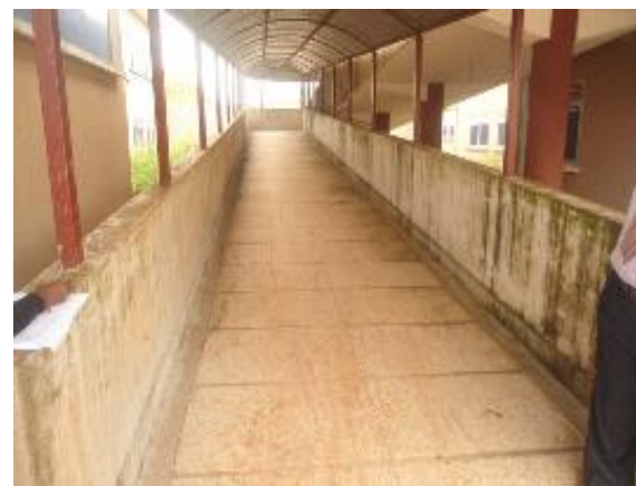
Newly constructed Private wing at Jinja RRH (Left) Walk way of the private wing with green algae growing on the walls
