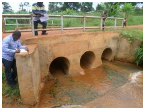
Left: Twaha Multiple culverts Left; Right: Bushy section of the road along Kasingo – Kalyabuhire road
