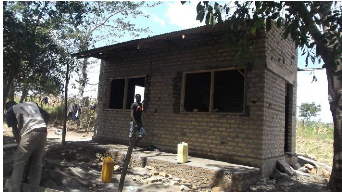
Construction of a two unit market stalls at Kyawagonya Market
