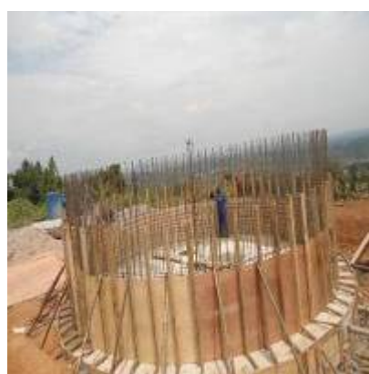
Left to right: Construction works of a twin reservoir tank of 220m 3 , a water office block, and a pump house
