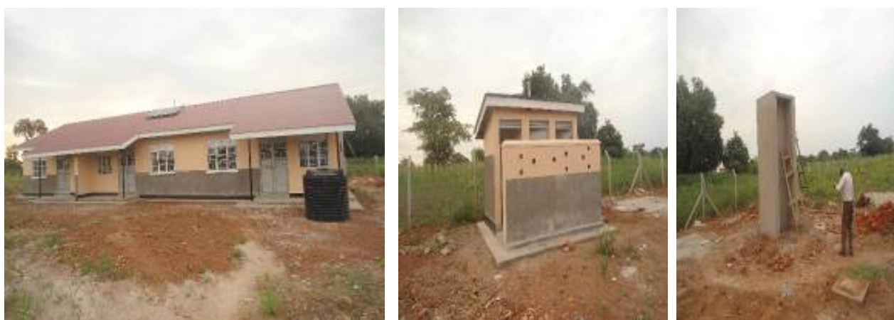
Completed staff house, Pit latrine and tank stand at Tiriri HCIV
