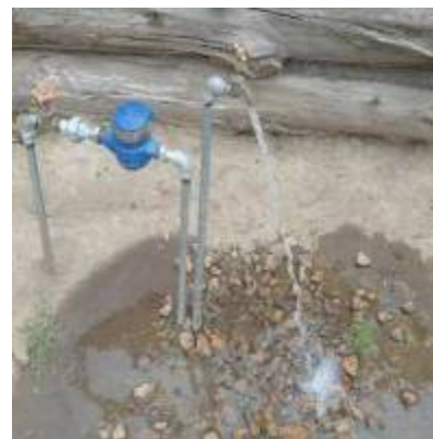
Left to right: Water office, a short term provision by community to avoid airlocks, and household connection
