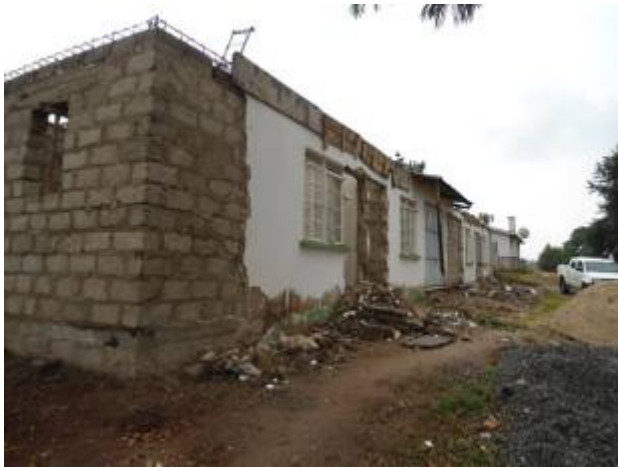
L-R: Remodeled 12 unit staff house at ring beam level and sub structure of the hostel at Nyaruzinga Bushenyi district.
