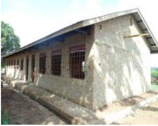
The three class room block still under construction at Wampewo P.S
