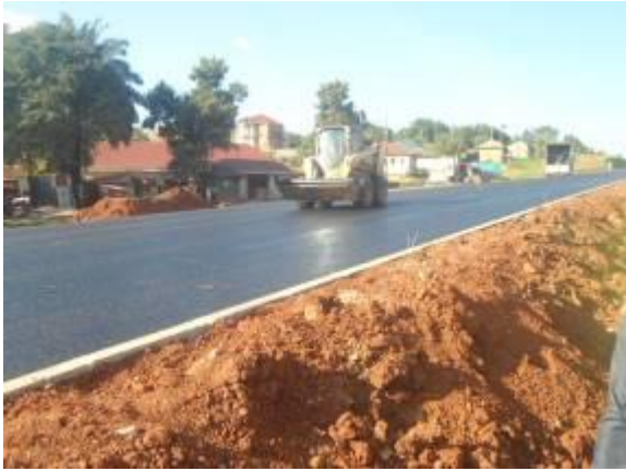
Kampala –Entebbe Expressway : Asphalt works
