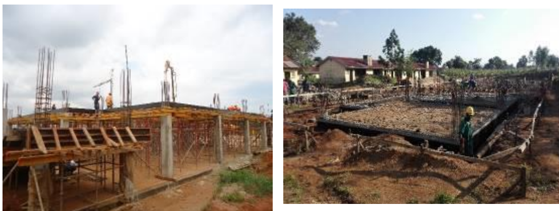
L-R: Ongoing construction works at Kayunga Hospital; Works at Yumbe Hospital
