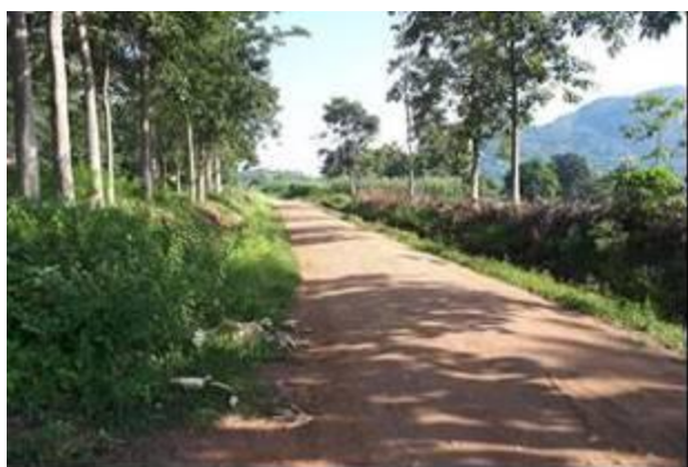
A section of Koboko-waniza (11.3km) that received routine mechanized maintenance in Q2
