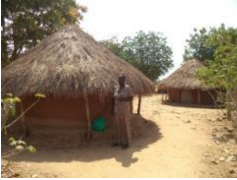
Old huts occupied by Teachers in Ájoba Primary School, Olio sub-county, Serere district
