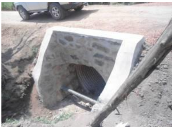
An armco culvert on Rutoto-Ndangaro road at km 0+800
