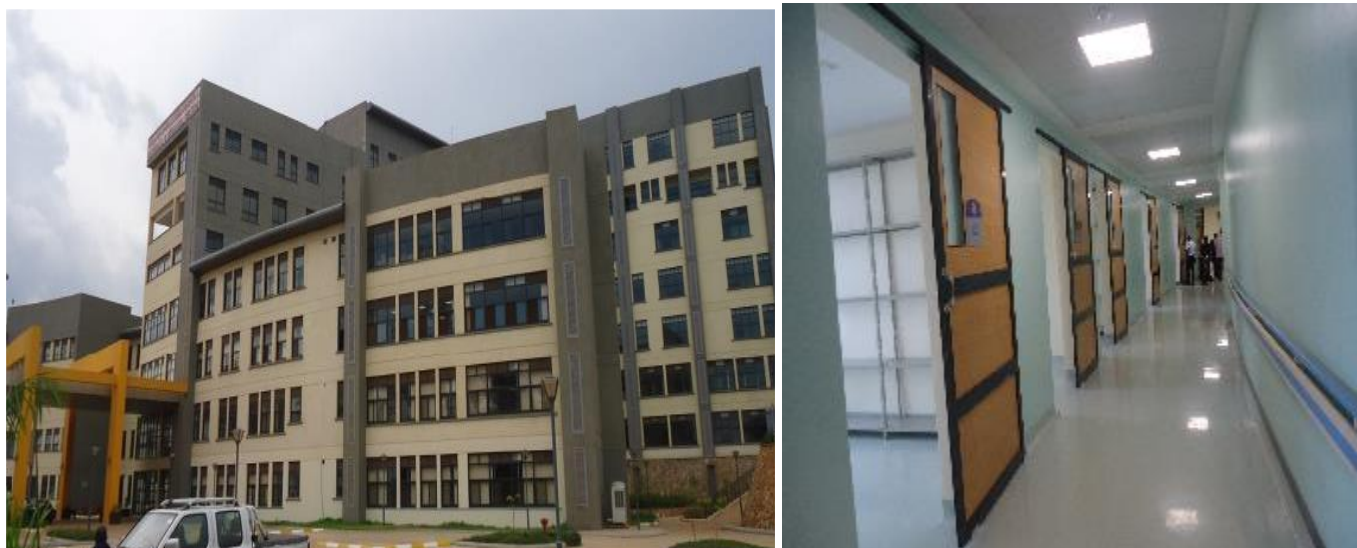
Completed section of the Neonatal and Maternal Hospital at Mulago
