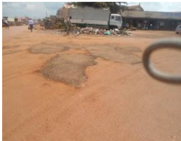
Patch works along Kinyoro-Church road
