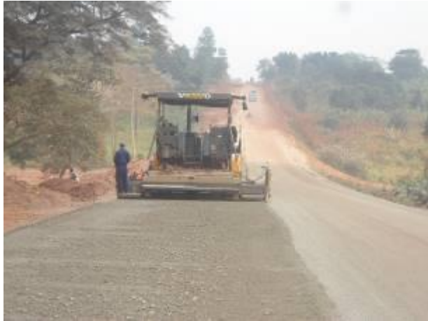
Nansana-Busunju Road: Laying of base course at km 35+480
