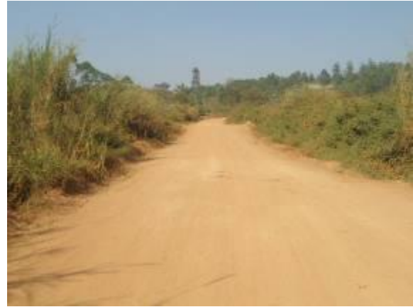
A section of Lusailira-Nkonge road at km 15+500
