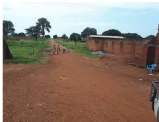
Acholibur – Latanya Road (17.4km) after Routine Mechanised Maintenance
