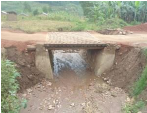
Emergency works of a timber deck bridge on Butambi-Mparo road at km 0+200
