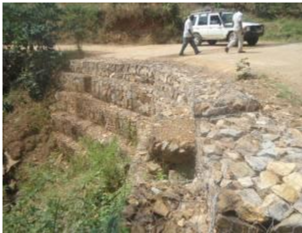
Gabion Embankment works along Ruhumuro-Burungira-Kikorijo-Nyeibingo-Buhimba road
