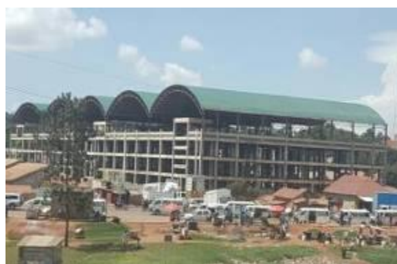
Roofing and external works in progress on Busega Market
