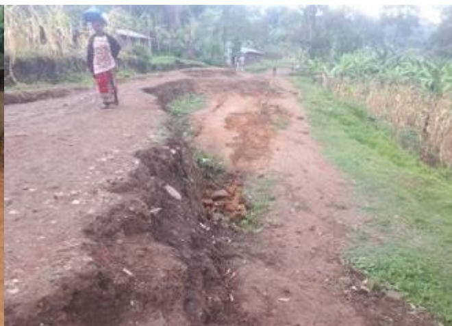
Kufu-Magale Road (16.7km); A bottle neck at km 13+100 following a landslide
