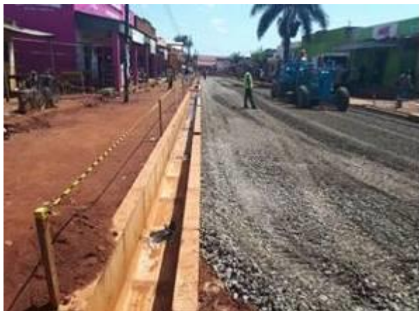
Processing base layer on Gulu municipality roads
