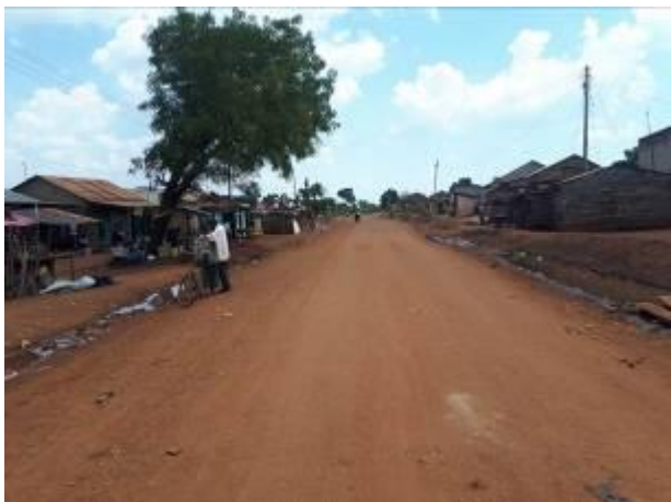
Kamuli-Namasagali Road (23km) after routine mechanized maintenance in Q3 FY2017/18
