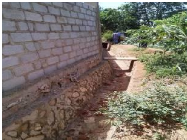
Stone pitching works of the off-shoot drain for Sebugwawo road
