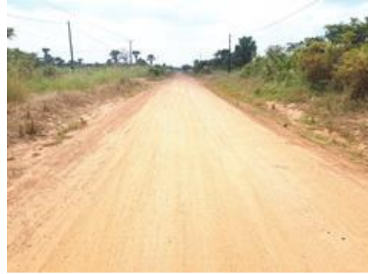
A well graded section of Gweri-Awaluwili-Amukaru Road after routine mechanised maintenance
