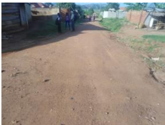
A section of Access to Kajjansi Airstrip Road
