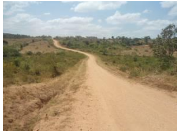
A road section of Kitenga-Ikula-Kanyogoga road at km 18+400
