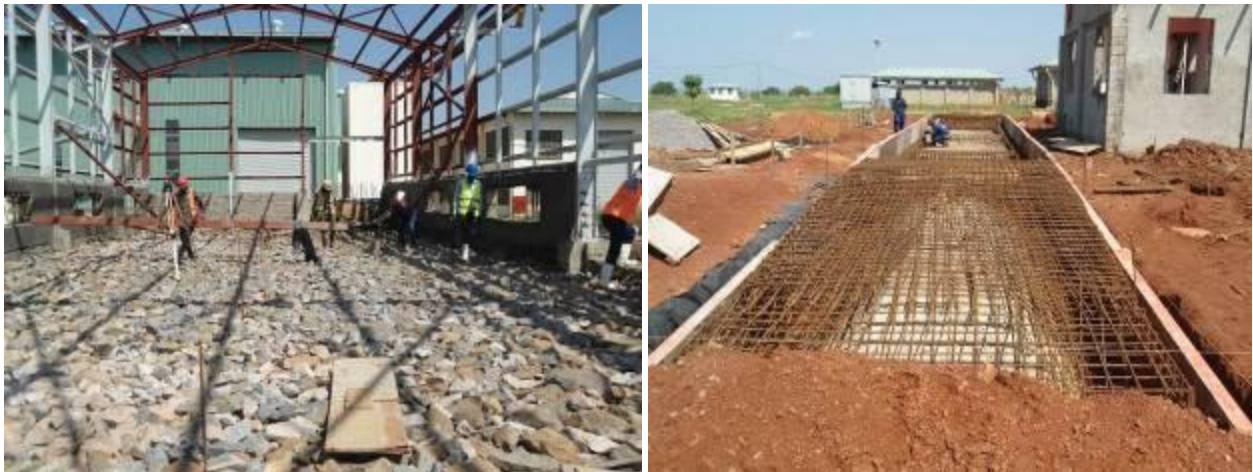
Ongoing construction works at CDO cotton seed dressing station in Pader District
