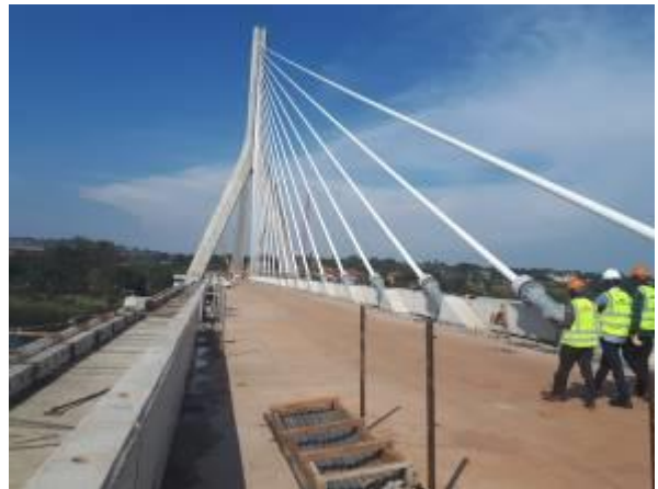
New Nile Bridge(525m long)
