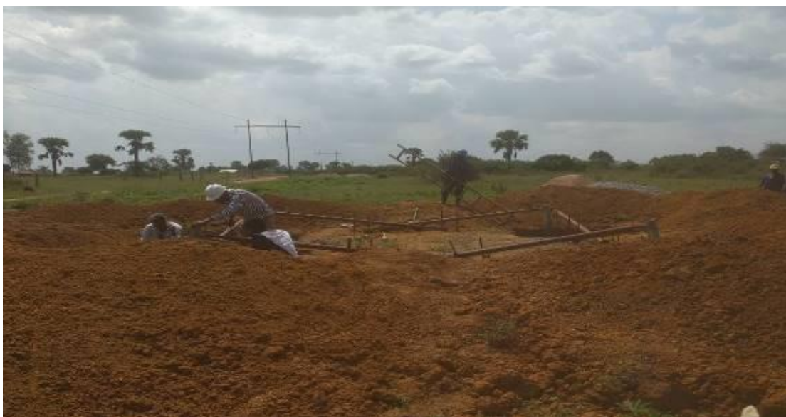
On-going Tower foundation works at Soroti Airfield, works at this location area as a result of transmission line diversion at Soroti Airfield
