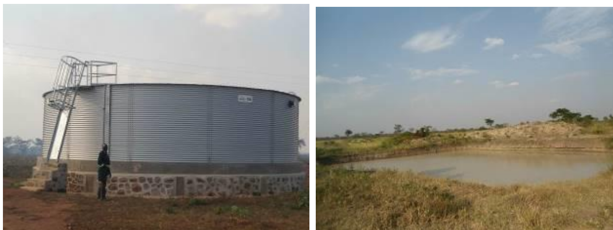
350,000 litre reservoir tank (left) and one of the six valley tanks constructed at the National Leadership Institute by MAAIF under the Meat Export Support Services sub-programme
