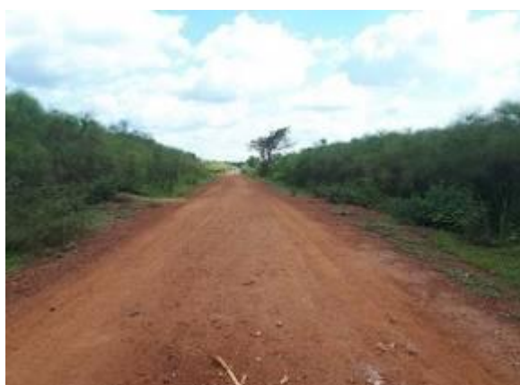
A well gravelled swamp section on Nsinze-Naigobwa road(5.3km)
