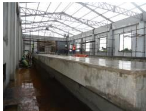
L-R: Sludge Digester under construction in Bugolobi, Kampala; Grit removal chamber at roofing stage in Kinawataka Kampala
