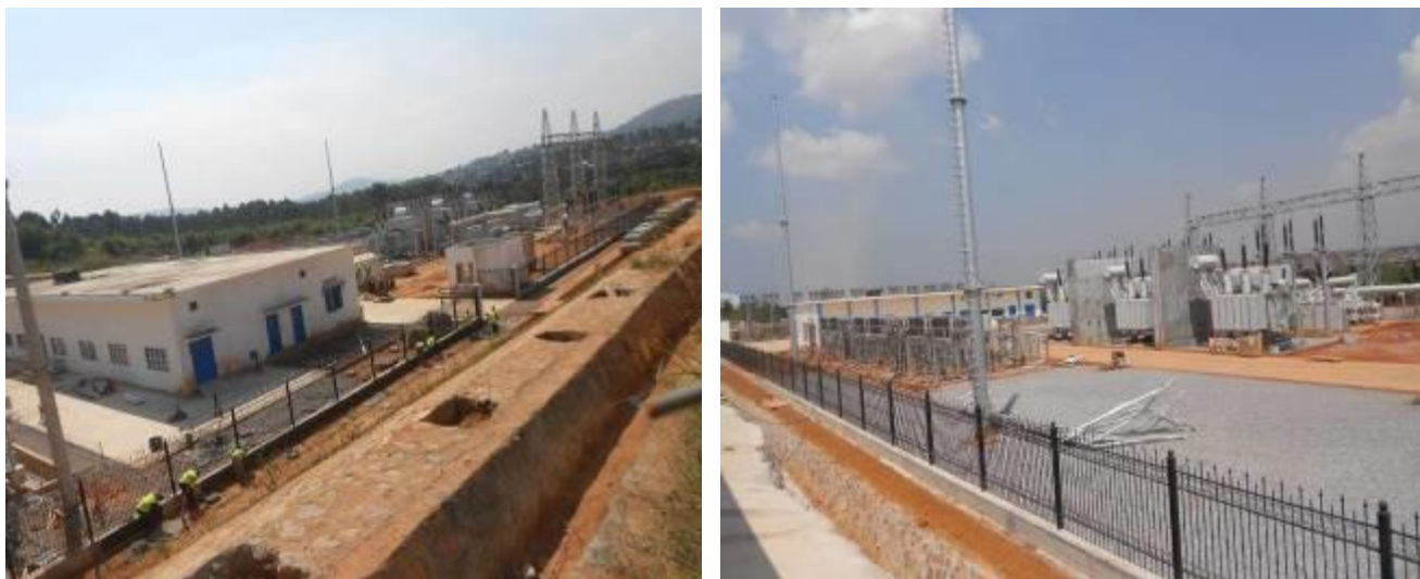
L-R: Fencing works at Mukono substation; Final works at Namanve Substation
