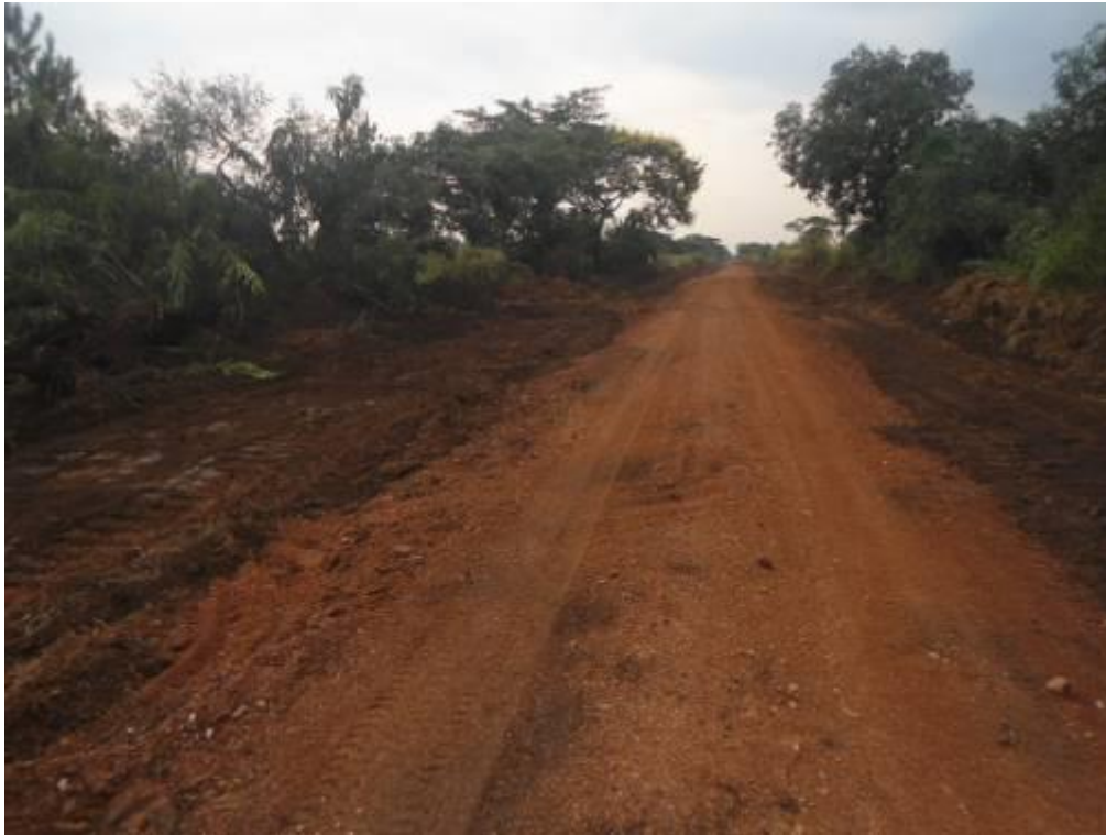
A section of Ikooba-Ntooma road where bush clearing had been done
