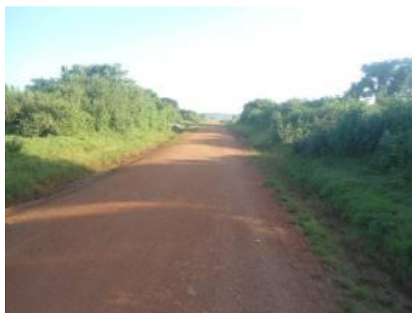
A well graded and shaped section of Kawuku-Bwerenga Road at km 6+600
