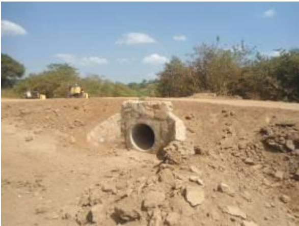
A culvert at km 10+700 on Kasambya-Nabakazi road
