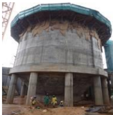
L-R: Sludge Digester under construction in Bugolobi, Kampala; Grit removal chamber at roofing stage in Kinawataka Kampala
