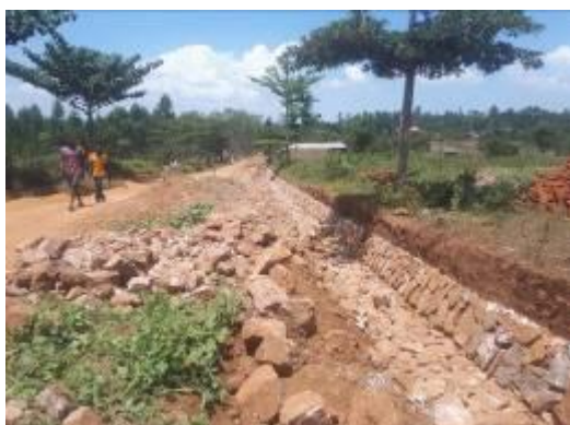
Nangwe Road (0.5km)-stone picking works were ongoing
