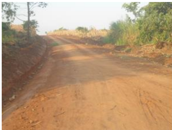
A section of Kidunumya-Muwoko-Nsira-Kyamasinde at 0+000
