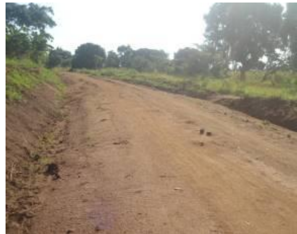
A graded and shaped ssection of Mabuye-Nakakono road with loose material
