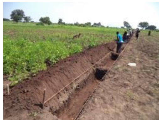
Soil and water conservation trenches
