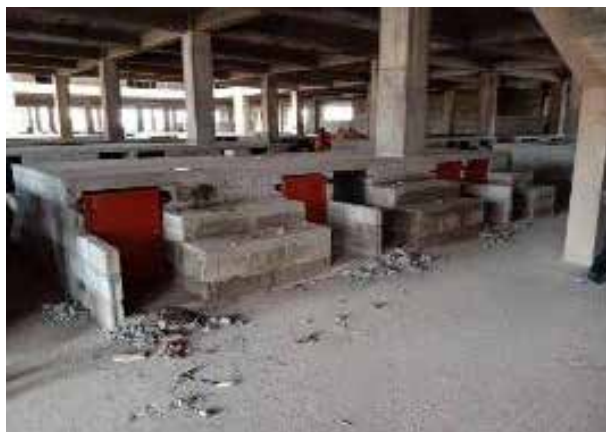
Constructed produce stalls in Busega Market
