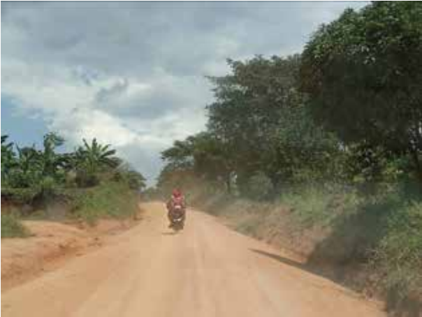
A section of Kassanda-Kalambe at 2+500
