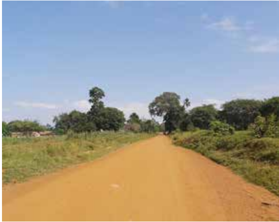
Nagongera-Busolwe-Busaba Road (28km) received routine mechanized maintenance in Q2 FY2018/19
