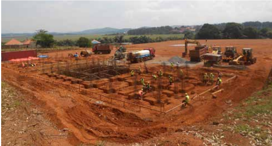
On-going civil works at the Entebbe 132kV substation site
