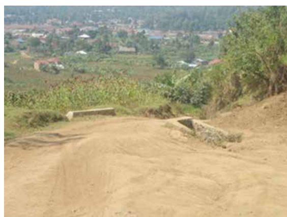
A culvert on Nyagashinge road at km 0+400
