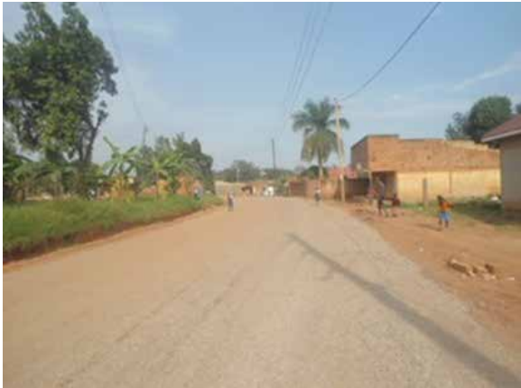
First level works on Kawanda-Senge Road
