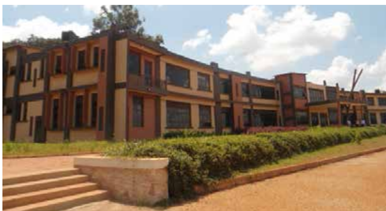
The central lecture block phase I completed at Kyambogo University
