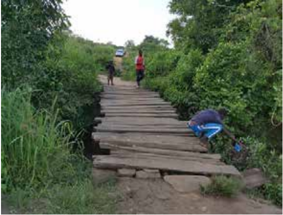
Lamola-Gweng Pamon-Lanydyang (3.3km): A bottleneck on the road that prohibits connectivity of motorized traffic between Kitgum District and Pader District
