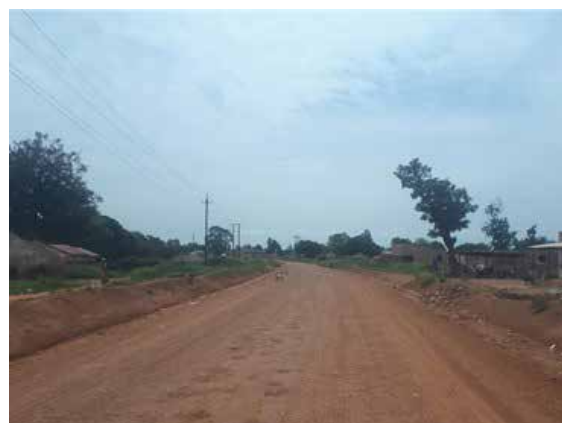
Koboko-Lodonga Road after gravelling done in Q4 FY 2018/19
