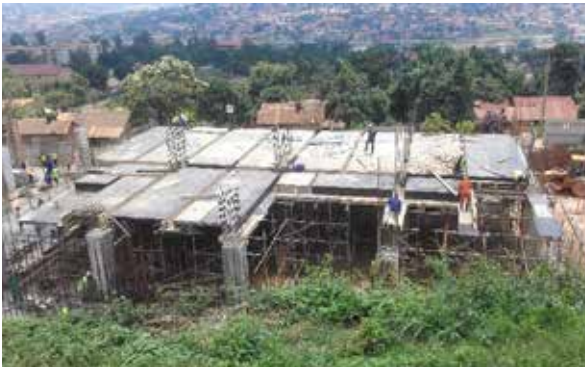
Auxiliary buildings under construction at Uganda Cancer Institute, Mulago
