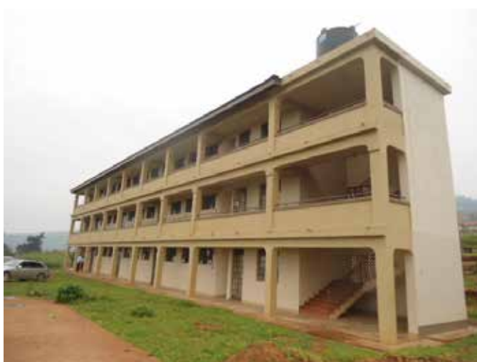
Lecture block completed structure at Kabale University
