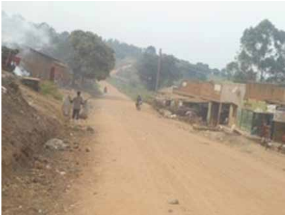
A section of Bukomansimbi-Bulenge Road at 0+000
