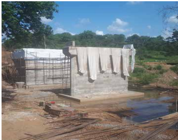
One completed abutment and pier of Ayugi Bridge in Amuru district
