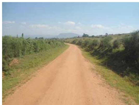
A section of Rwashamire-Kyafora-Kiyenje at 12+200
