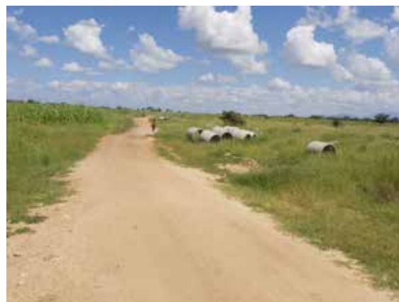
Delivered culverts yet to be installed along the Lopei – Kokeris Road
