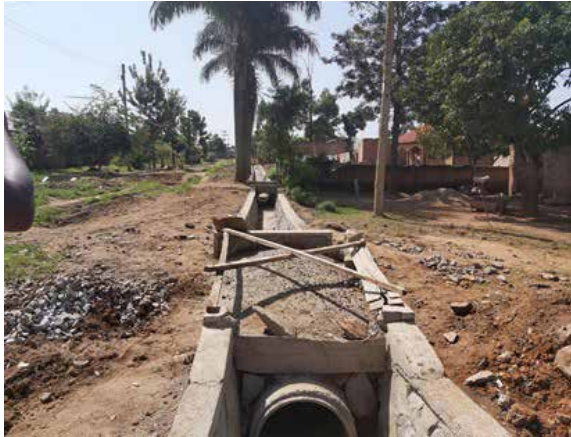
Stone pitching works for side drains on Economic road (0.3km)
