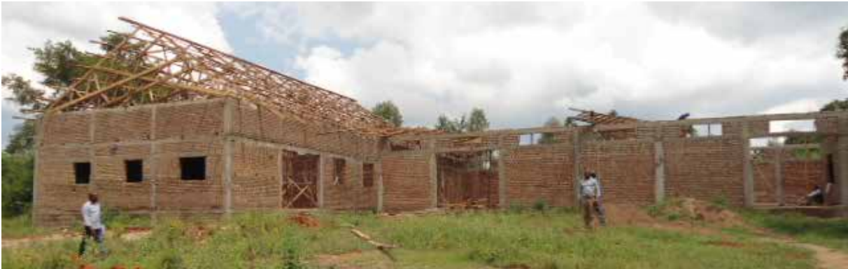
Warehouse under construction at Sihubira Area Cooperative Limited in Busia District
