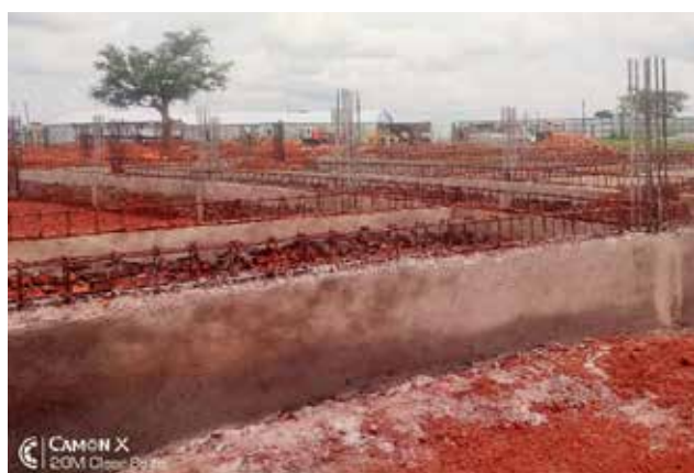
Construction of administration block still at foundation level at Lira University
