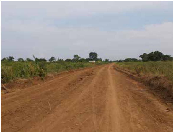
Omolokonyo Road after grading works in done in Q4
