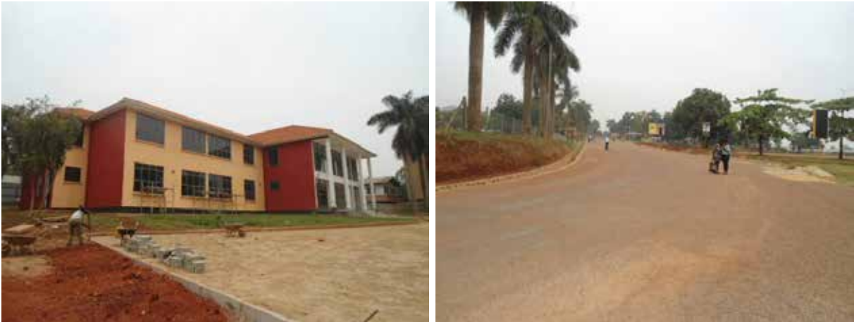
L-R: Block one/bursar's office; Part of the tarmacked 600 metres of the road at MUBS
