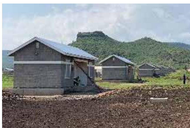
Connections to UMEME on completed housing units in Bunambutye sub-county, Bulambuli district
