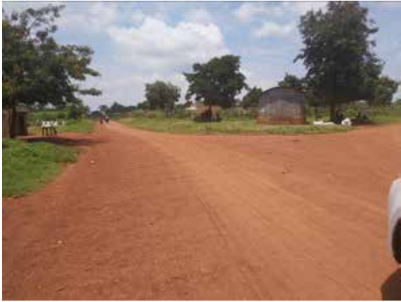
Part of the finished Okwir-Goro TC(10km) road in Nwoya District
