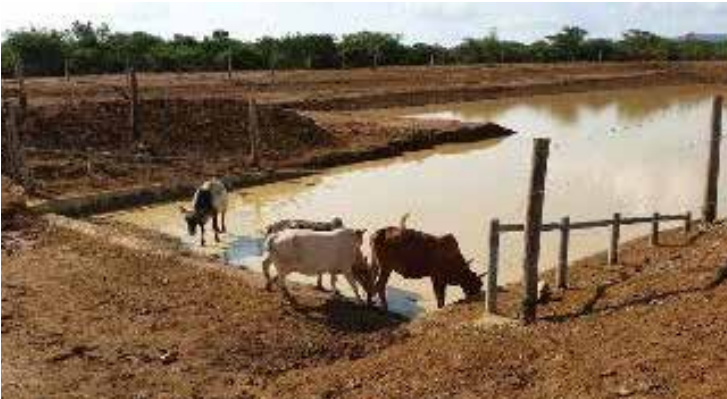
Completed Nakigwangret valley tank in Kataboke Parish, Amudat sub-county
