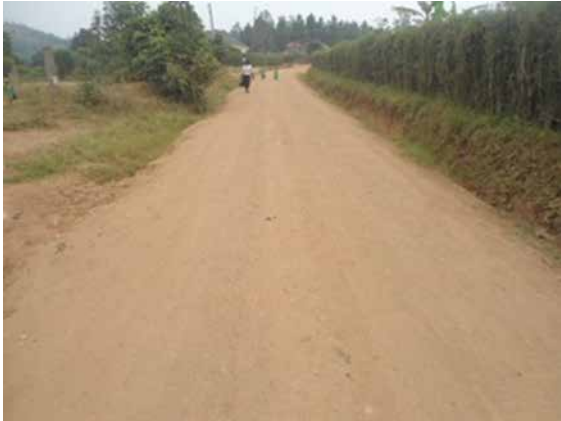
A section of Karugangama Road at km 1+600
