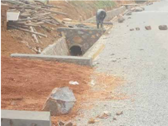
Stone pitching works along the sealed section of Rwizi road
