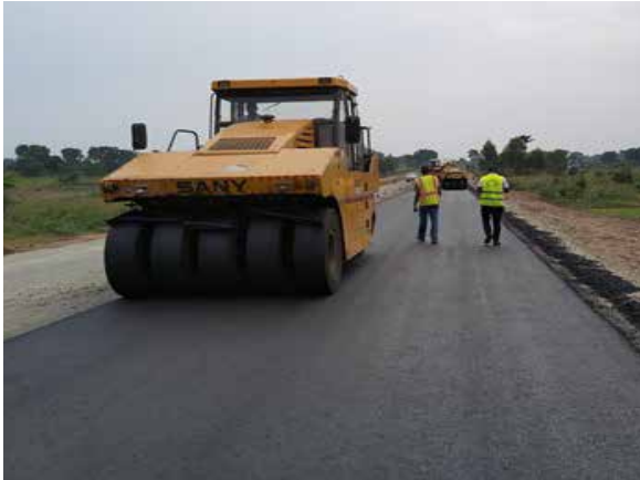
Asplat works on Nakalama – Tirinyi – Mbale road Road at km 37
