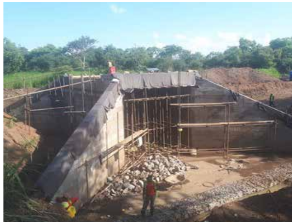
Construction of a one cell box culvert on Nakalama – Tirinyi – Mbale road Road at km 44 + 309
