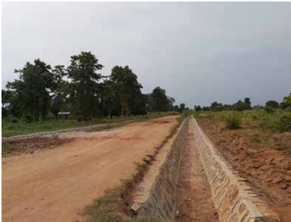
Stone pitched side drains on Kakungulu Road
