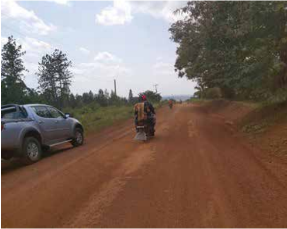
Bugiri-Muterere (18km) received periodic maintenance
