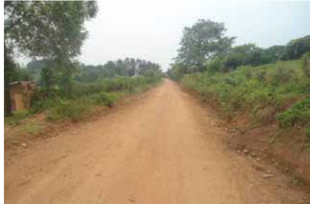
A section of Kigarama-Kobuzizi at 7+400 in a good motorable condition
