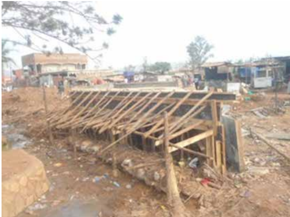
A box culvert under construction on Nansana-Nabweru-Kawala Road
