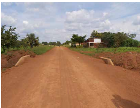
Left: Graveled section of Kitgum-lukung road (34 km) after mechanised maintenance done in the first call off order. Right: One of the cross culverts installed on the road
