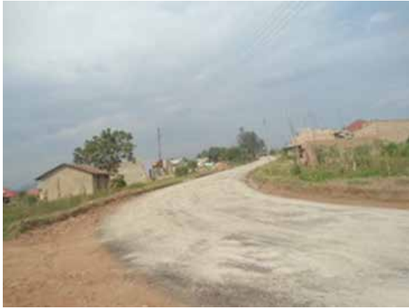
Sealing of Bigyega road at priming stage
