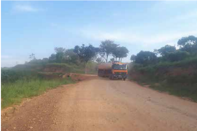
Nebbi–Goli Road (17km) after mechanized maintenance under the framework contract
