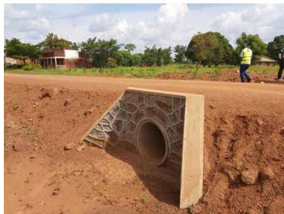
Left: Graveled section of Kitgum-lukung road (34 km) after mechanised maintenance done in the first call off order. Right: One of the cross culverts installed on the road
