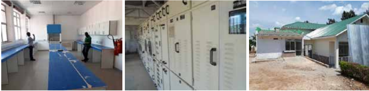
L-R: Research Laboratory being equipped, power stabilizers and director general's residence under renovation at PIBID in Bushenyi District
