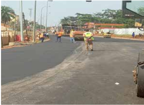
Priming works at km 31+150 on Kampala Entebbe Expressway
