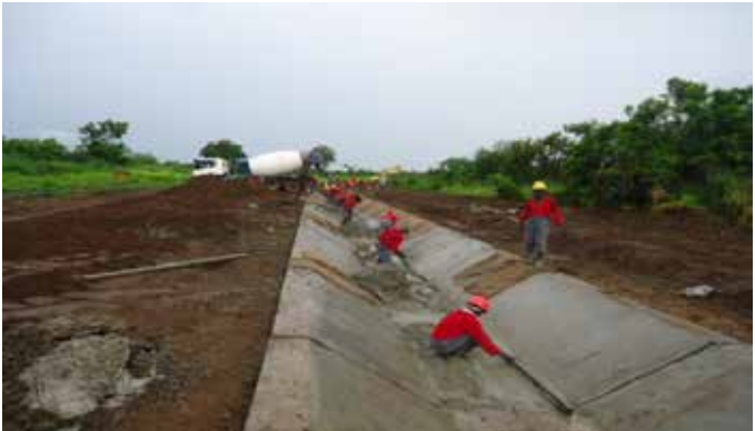
Main canal construction for Wadelai Irrigation Scheme in Pakwach District
