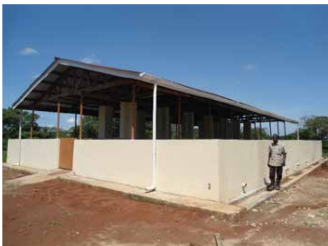
Completed pig sty at Kasolwe Stock Farm in Kasolwe Bulagala B village in Kamuli District
