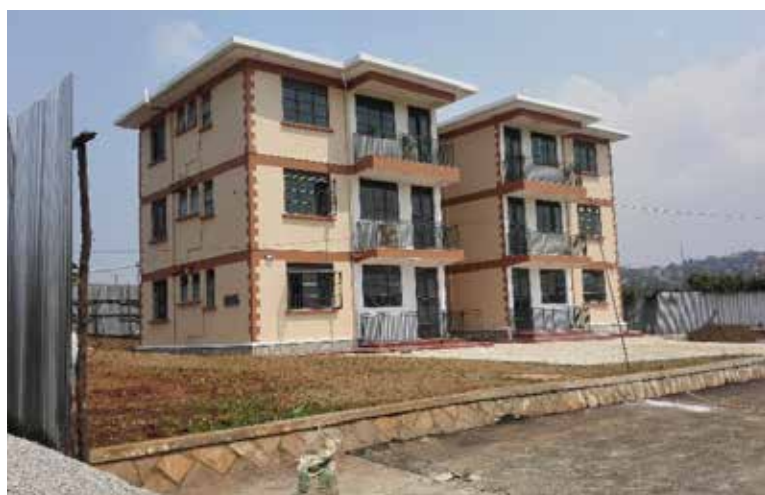
Six Storey Staff house at substantial completion at Butabika Hospital
