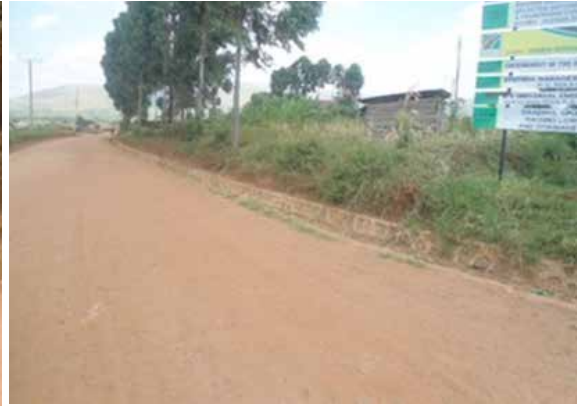
A stone pitched drain at the start of Rwentobo-Ngoma-Kizinga road
