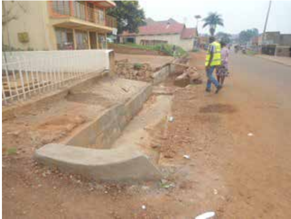
Resealing and draingae works on Kibuura road
