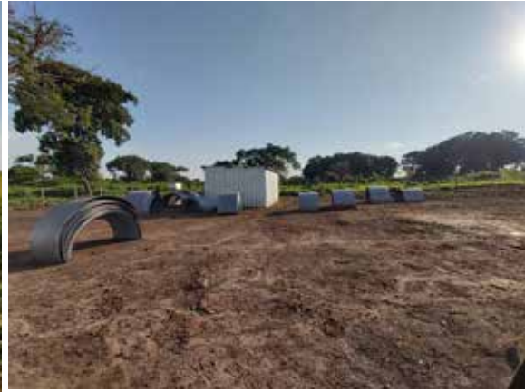
Mobilised materials for the Armco culverts- Kangai swamp crossing, Dokolo District
