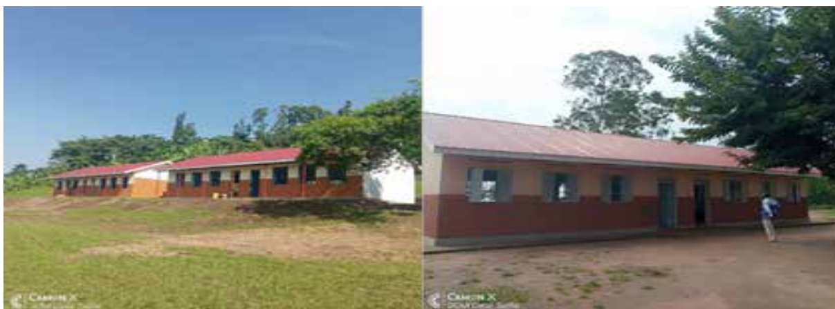
L-R: Completed 2 classroom block at Awadri P/S; Arua District and 4 classroom block at Buyobo P/S; Sironko district
