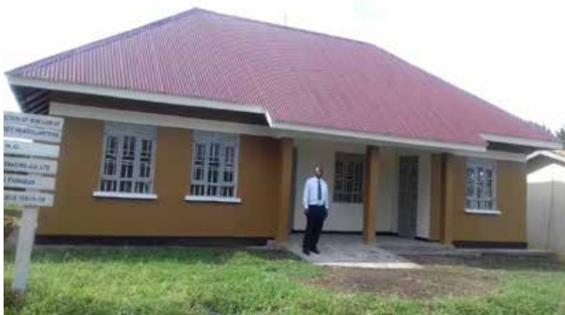
Mini-laboratory completed from slab level in Central Division Ntungamo Municipality, Ntungamo District
