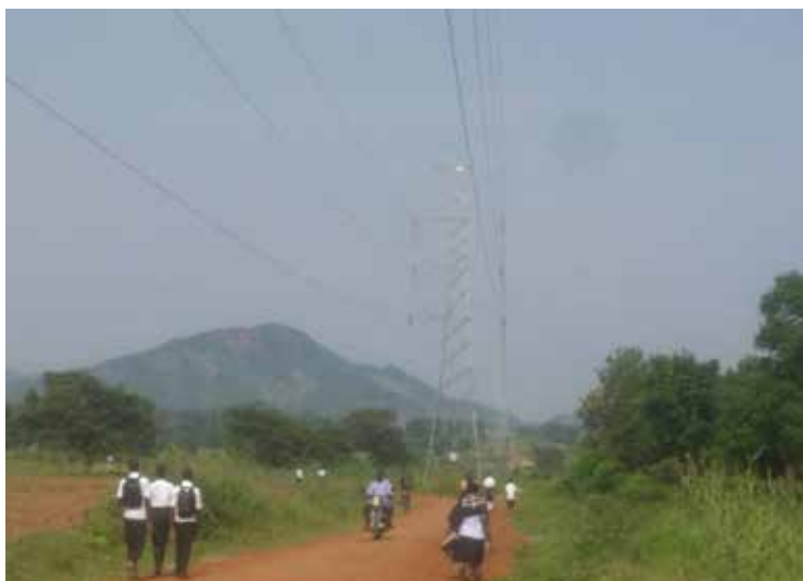
Completed section of the Tororo-Opuyo-Lira transmission line at Katerema, near Tororo substation
