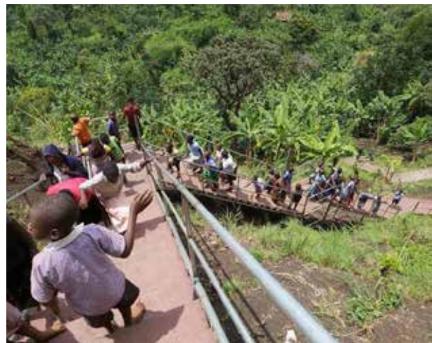
School going pupils already making use of the ladder at Sigwa Hill- Sironko District
