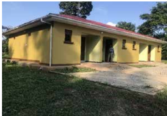
One of the staff blocks completed at NACORI in Mukono District
