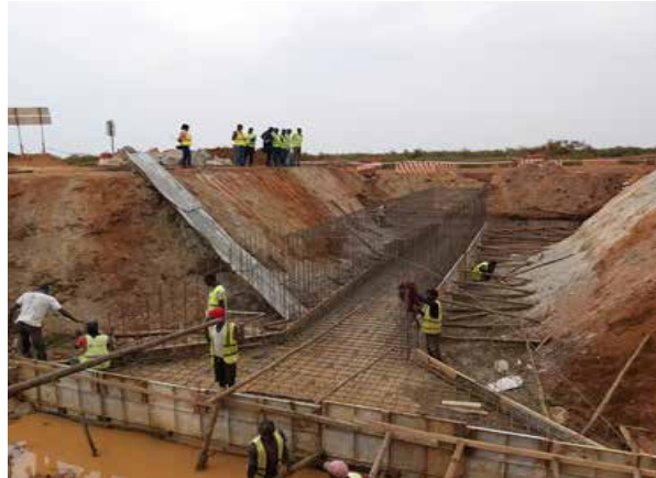
Construction of a one cell box culvert on Nakalama – Tirinyi – Mbale road Road at km 44 + 309
