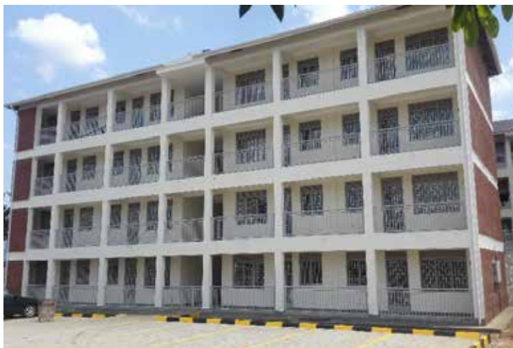
Newly constructed staff house at Fort Portal RRH
