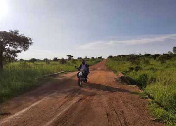
YY Okot-Ocettoke (11km) after Routine mechanised maintenance in Q2 FY2018/19
