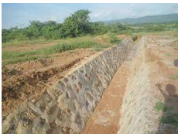
Left: Drainage Works on Kyehoro link along Hoima-Kaiso-Tonya road
