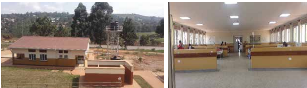
Left: View of the completed Mortuary. Right: Female Ward already in use at Kawolo Hospital
