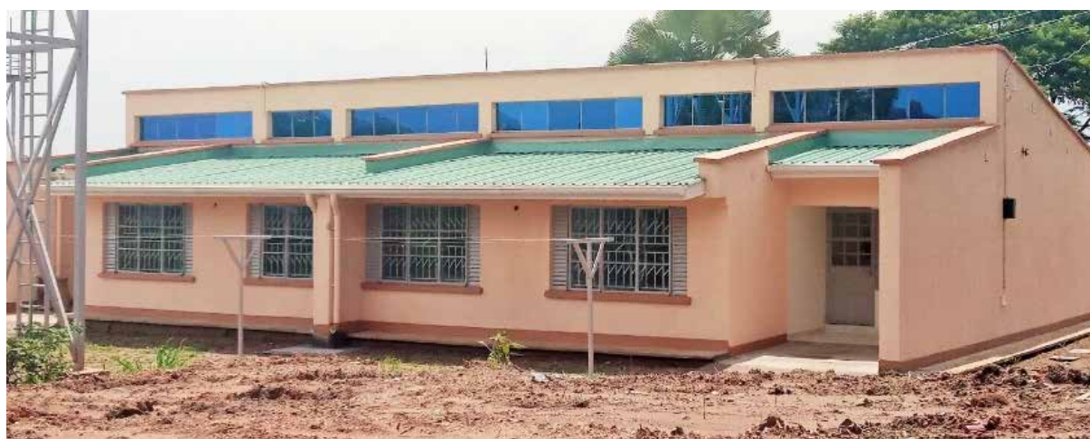
Completed staff house by Ambitious at Muni NTC
