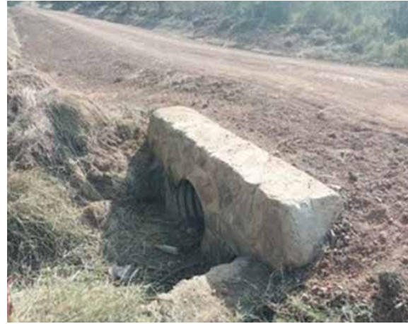
A culvert installed on Kaberebere-Nyarubungo-Nyamitsindo
