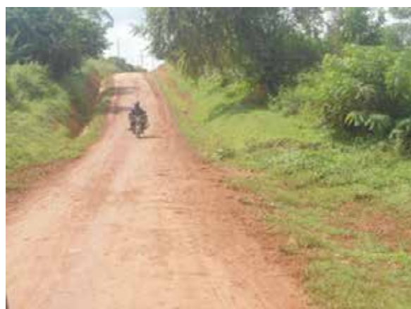
Right: A section of Katsiha-Waaki Road at 5+200
