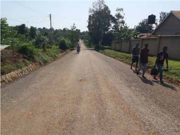
Surface dressing done on Balunywa road under Periodic maintenance
