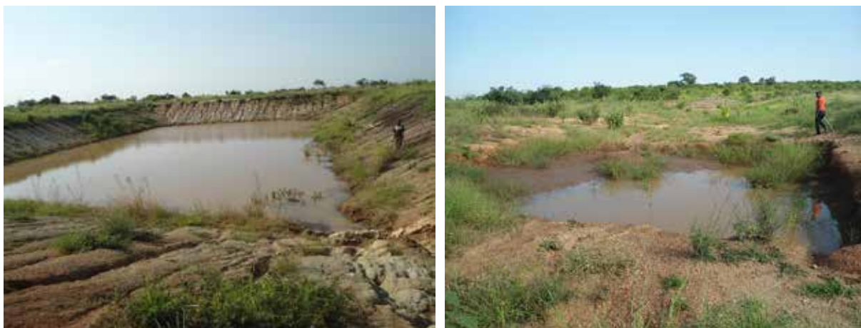
Non-operational Lojudongu community dam (left) and desilted small dam in Lojudongu village Nebbi District
