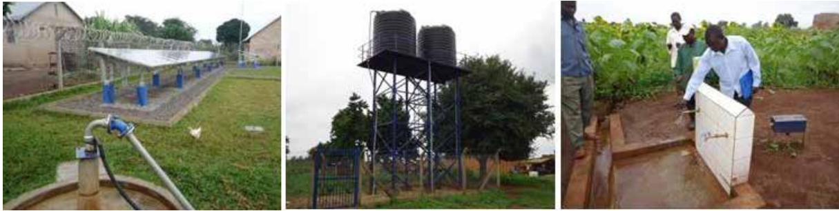
L-R: A water source and solar array; Reservoir tanks; and community PSP of Kalwala mini solar powered scheme in Kiryandongo District
