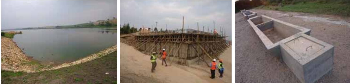
L-R: The dam/water source; a 1200m 3 reservoir tank; and cattle troughs of Mabira dam in Mbarara District
