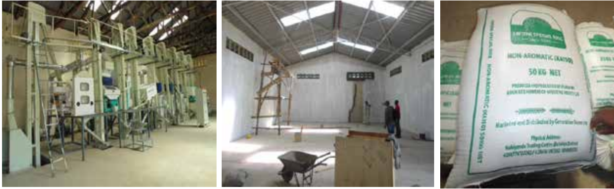
L-R: Installed rice processing equipment, a 500MT store and processed and bagged rice in Manafwa
