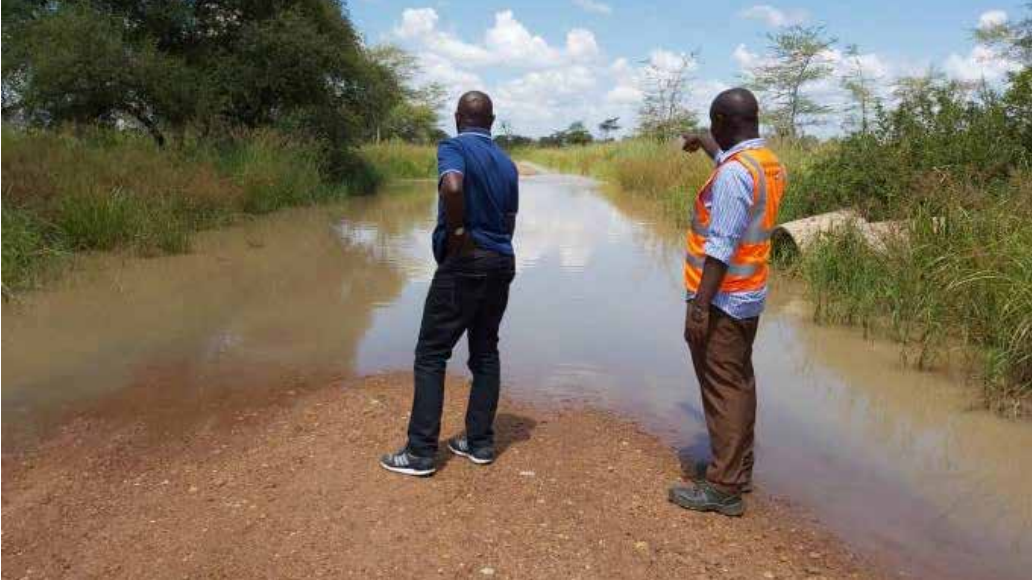
Flooded/impassable section along the Matanyi – Lokopo – Turutuko Road
