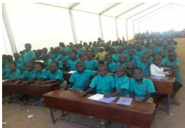
Erected tarpaulin being used as temporary classrooms for learners in Bulambuli District as at July 2019
