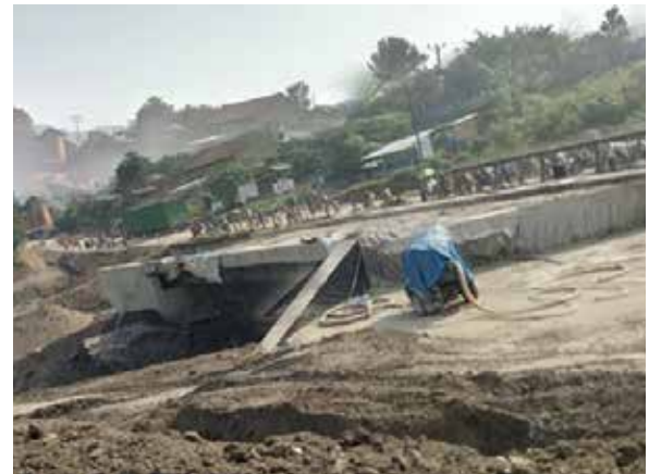
Mpondwe Bridge works at the Uganda-DRC Border in Kasese
