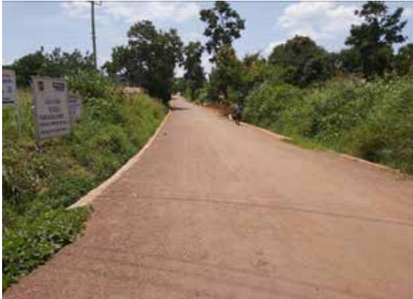
A completed section of the Gulu High School road
