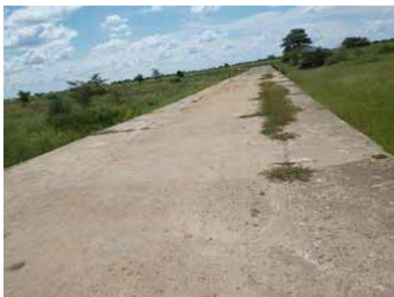
Repaired drift along the Lopei – Kokeris Road
