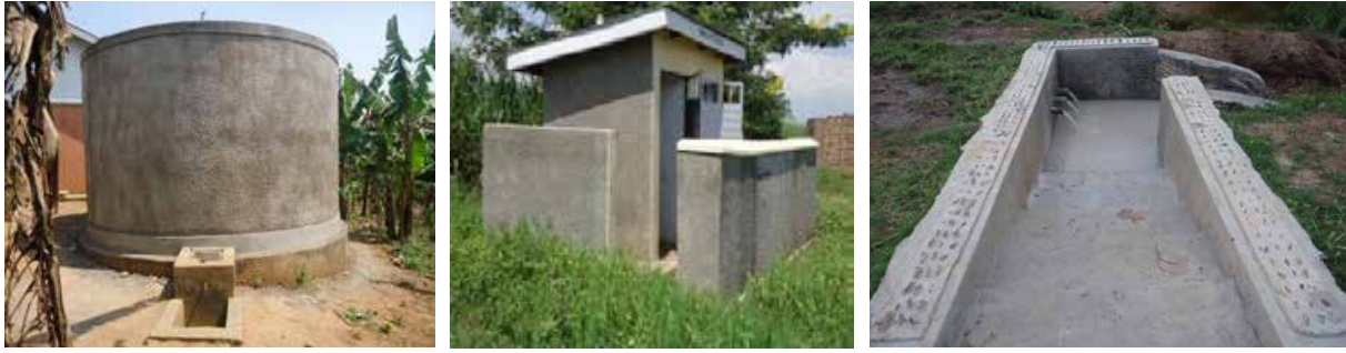
L-R: A rain water harvesting tank at Bulungibwabakadde P/S, Kalungu DLG, a public toilet at Lubaizi landing site, Kamuli DLG and a protected spring at Kocheke village, Bukedea DLG
