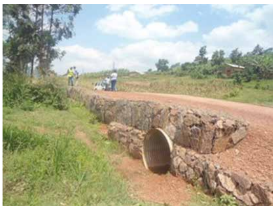
A culvert installed and gabion works on Butobere-Muyomba-Rwamcucu at 16+500
