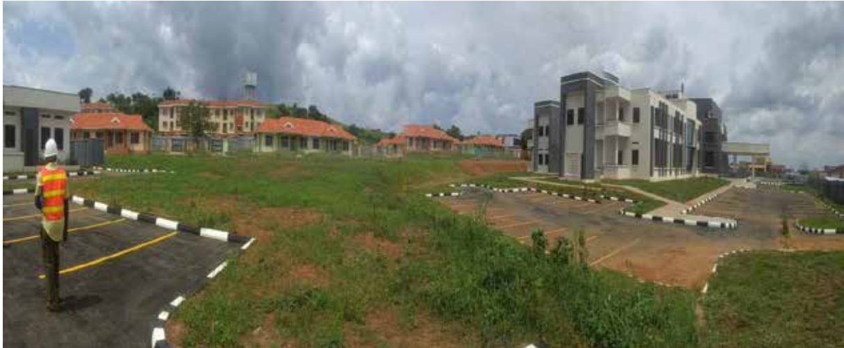
Newly constructed office block ( Far right) , staff houses(Center) and laboratory building(Left) at Karuma HPP
