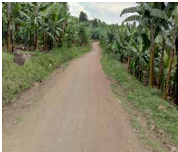
A section of Kibiito-Kabonero – Kasunganyanja Road
