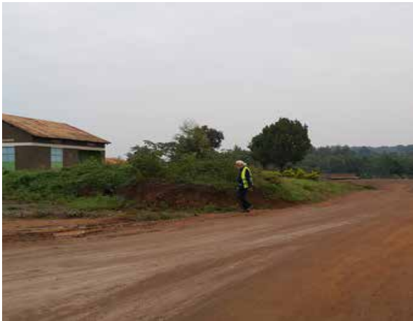
One of several sections (at km16+00) of Bumbobi – Lwakhakha road skipped due to compensation issues
