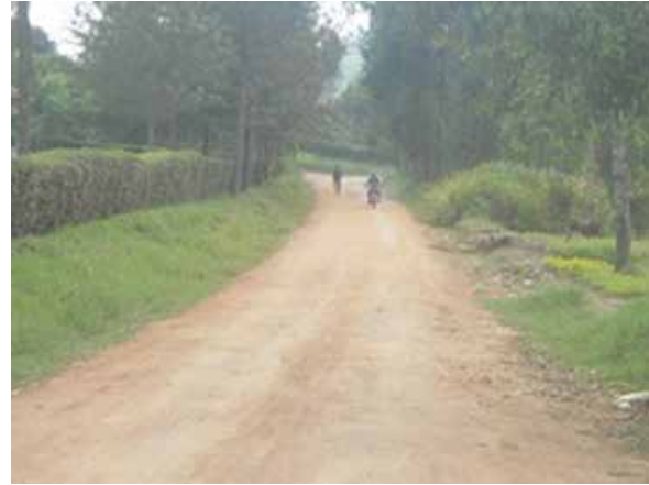
A section of Binyerere Road at km 1+900 in good condition
