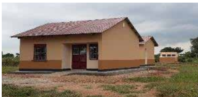
Newly constructed house , kitchen and bathroom facilities at Kwarikwar Primary School in Kumi district
