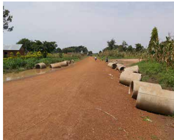
Culverts dumped on Hahoola-Maluku road awaiting installation
