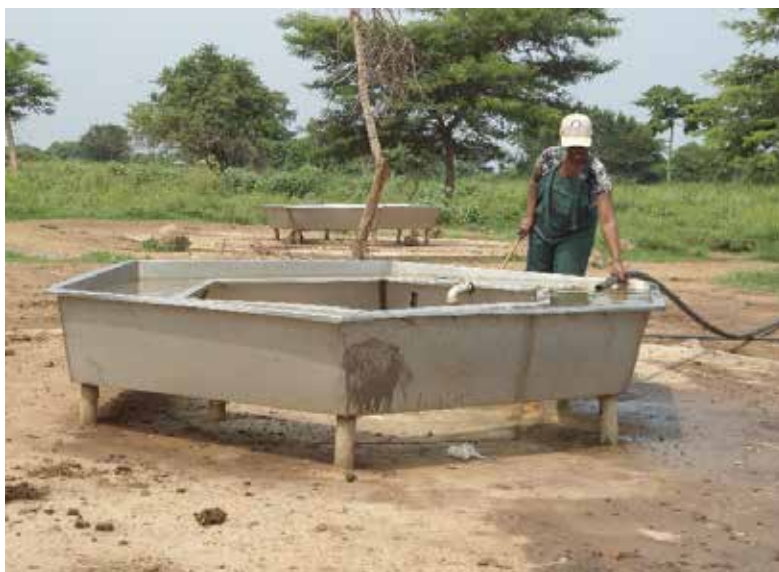
Completed and functional water troughs at Maruzi Ranch in Apac District
