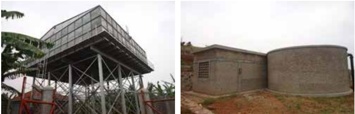
L-R: 500m 3 main reservoir; 100m 3 sump and pump house of Nyamiyonga-Katojo water supply scheme in Isingiro district.
