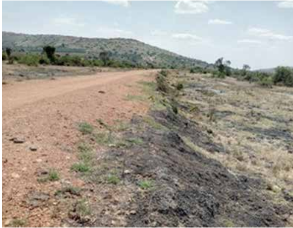
A swamp rased section at km 3+800 along Remibiribwa-Kendobo-Mirambiro road
