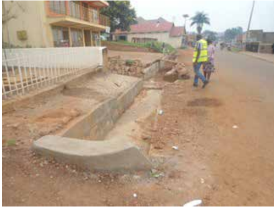
Resealing and drainage works on Kibuura road
