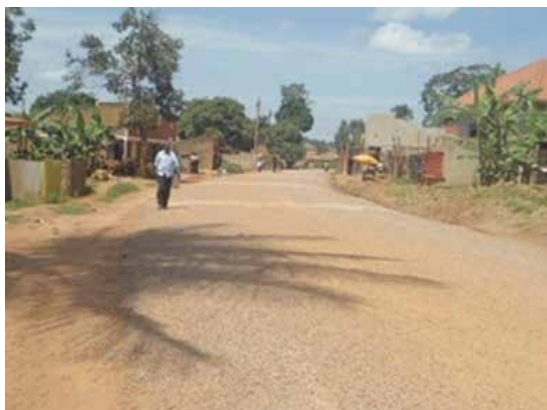
First seal works on Serado-Bajjo-Nantabulirwa
