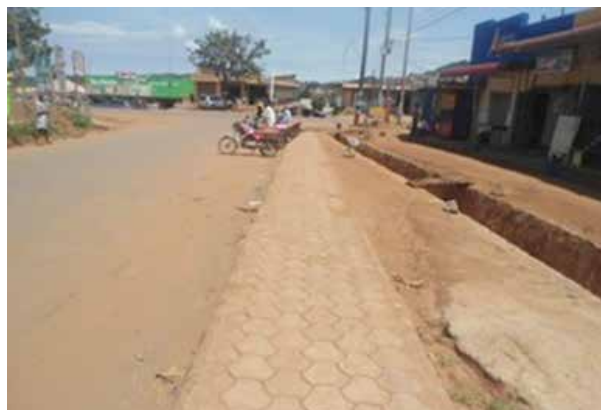
A pedestrian walkway on Mulyanti Road
