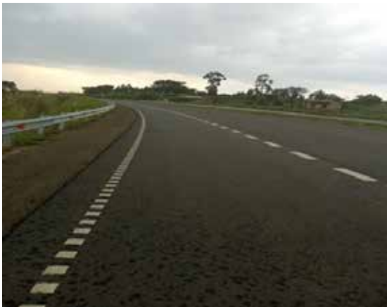
A completed section of Mubende-Kakumiro-Kagadi road at km 56+000
