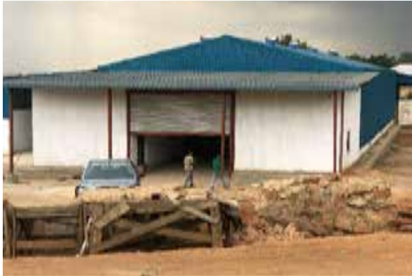
Warehouse whose construction was partially financed with the ACF at New Kakinga Millers Enterprises Ltd in Ibanda district
