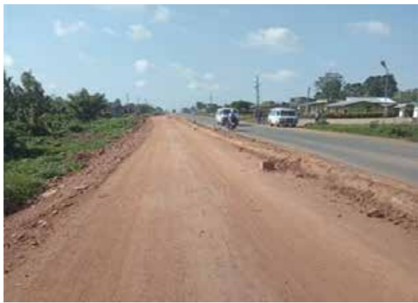
A section under widening on Fort-Hima road.
