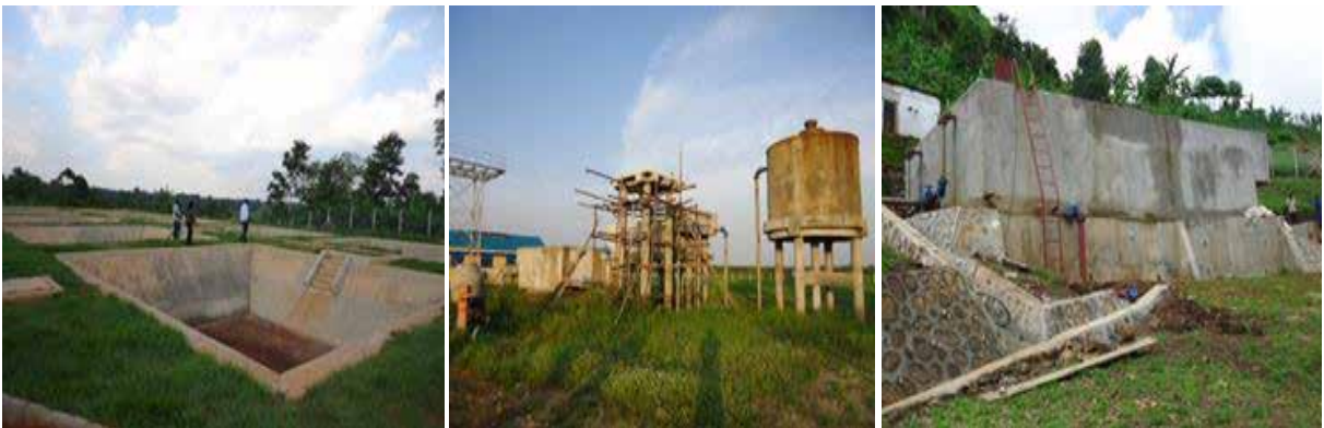
L-R: Facultative ponds of Kamuli Faecal Sludge in Kamuli District; Water treatment structures for the Namwiwa WSS in Kaliro District; and Sedimentation tank of Bulegeni WSS in Bulambuli District
