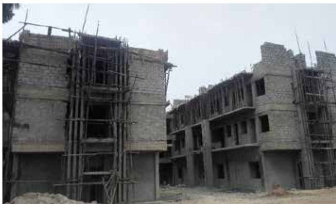
Intern's Hostel under construction at Kabale RRH
