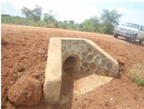
A culvert installed on Bukomero-Dwaniro-Kyankwanzi Road at 28+700
