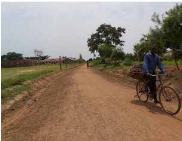
Busibira -Butesa (9km) received routine mechanised maintenance in Q2-Q4 FY 2018/19
