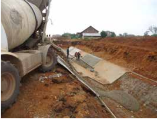
Main canal construction for Mobuku Irrigation Scheme in Kasese District
