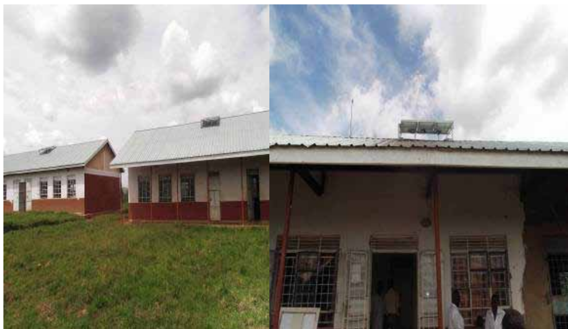
Installation of solar panels at Jangokoro Seed Secondary School and Ora Technical Institute Zombo district
