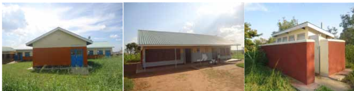
From left: Completed general ward at Labworomor HCIII, completed OPD Lujorongole HCIII, and completed latrine at Lukwir HCII
