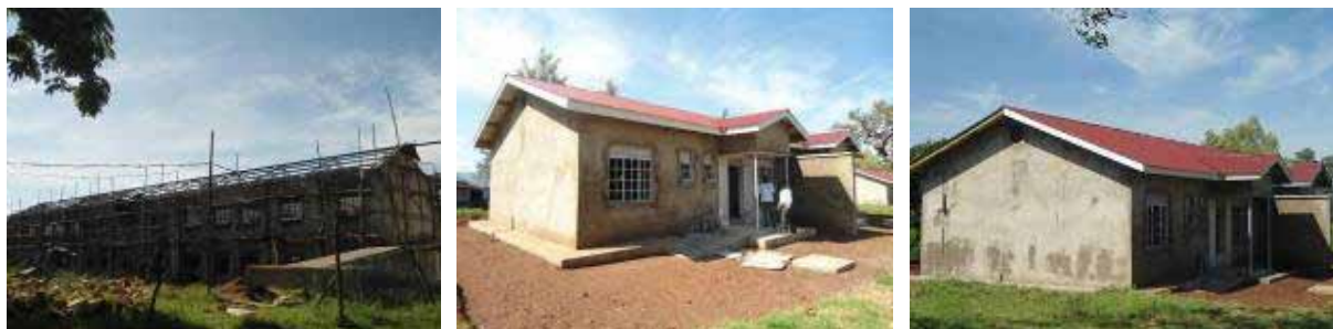
From left: The multi purpose block at roofing level, and 2 semi detached houses at finishes level at St Peter's College Tororo
