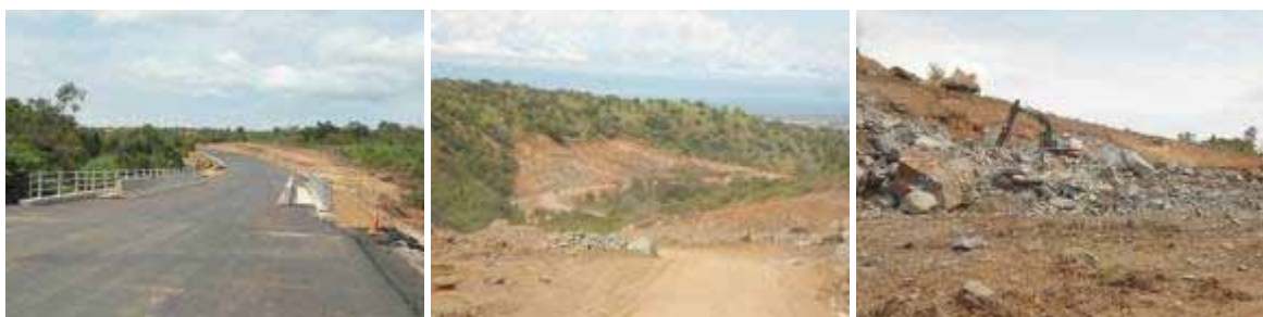
(Left): Completed Wababya Bridge with walkways at Km 34+000; (Centre): New alignment of the road at Km 59+480 with a 28m fill; (Right): Rock excavation along the escarpment.
