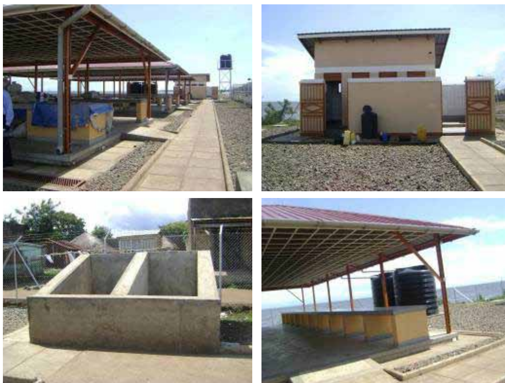
Rehabilitated Panyimur fish market in Nebbi district
