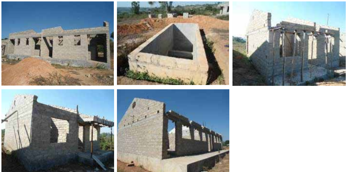
From the top left, A 4 unit teachers' house, a 5 stance VIP abandoned at slab level and a 2 bed roomed house, 2 bedroom housed abandoned at roofing level and another block abandoned at roofing level at Kalisizo S.S.
