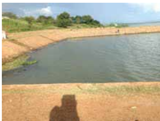
UEAWCP funded jetties at Masese landing site Jinja
