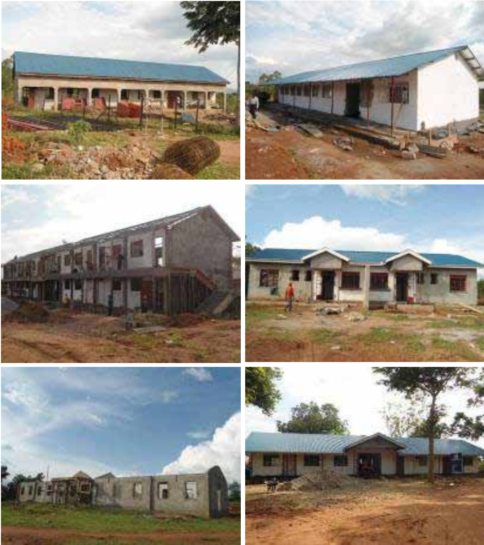
From the top left: The renovated boy's dormitory, a library and the storied six classroom block at roofing level. From bottom left: The semi-detached house at finishes level, a girls' dormitory at roofing level and the administration block at finishes level at Lumino High School.
