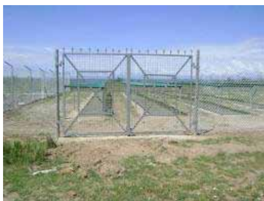
Fenced off MAAIF funded mukene drying racks not yet operational at Walukuba landing site.
