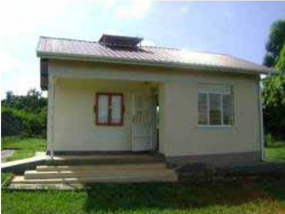
New office block for Hoima DFO
