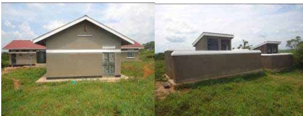
Nearly completed maternity ward at Lukolo HCIII and adjacent pitlatrines
