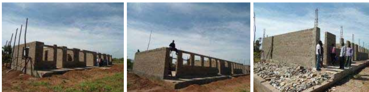
From left: The administration block and the 3 unit science block at ring beam level while the storied 6 classroom block they were beginning shuttering for the 1 st floor slab at Apo Seed S.S. Other structures were at the same level.
