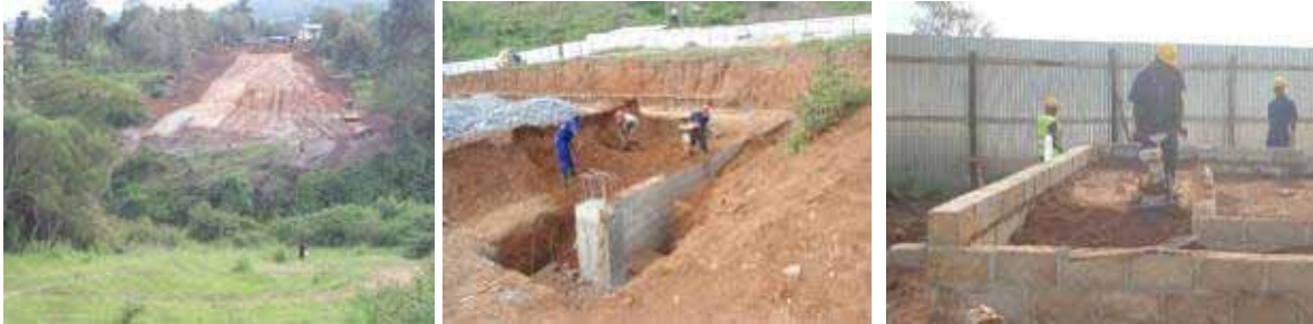
(Left): Road works ongoing on the Rwandan side but have yet commenced on the Uganda side; (Centre); Return, filling and ramming of soil into the excavations of the Customs and Immigration Block substructure; (Right) Compaction of murrum to make part of the floor of the Proposed Clearing Agents Building.
