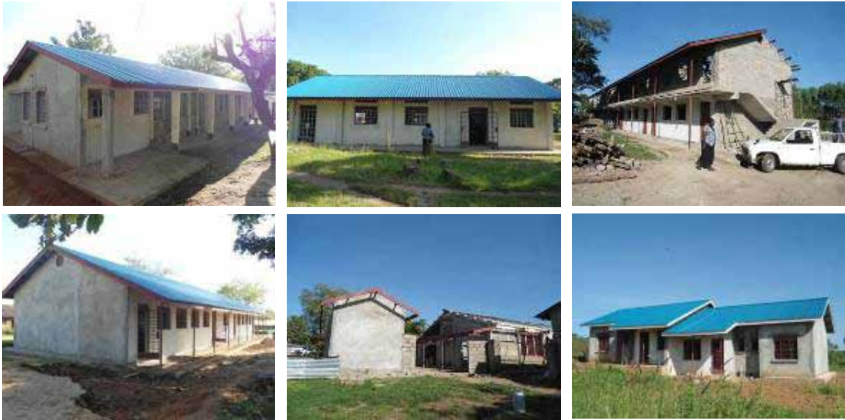
From the top left, a renovated staff room, ICT block and the 8 storied classroom block. From bottom left, the new science block, semi detached 2 bedroom house, and the dining hall/kitchen complex being rehabilitated at Mvara S.S.
