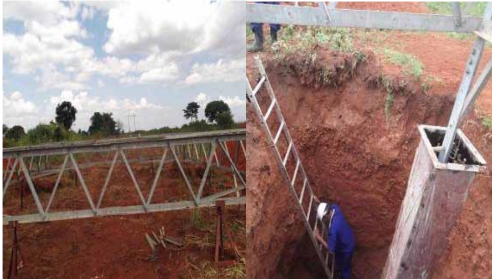
Foundation works for tower installation on the Tororo-Lira Opuyo transmission line
