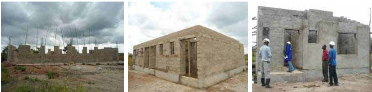
From left: The storied 4 classroom block going to first floor slab, a 4 unit teachers' house and the 2 bedroom house at wall plate level at Ramogi Seed S.S.
