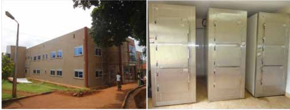
Left to right: Private wing under construction and repaired Mortuary fridges at Jinja RR Hospital
