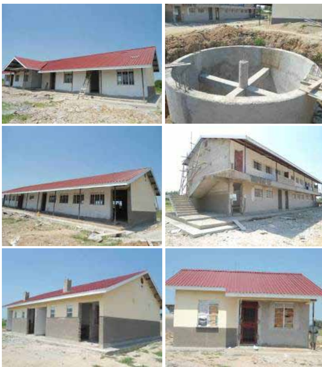
From top left the administration block at finishes level, the under ground tank, a 2 unit science laboratory at finishes level, From bottom left: a storied 6 classroom block at finishes, a 4 unit staff house and a 2 bed room house at finishes level at Kanara Seed S.S The other structures were also at finishes level.
