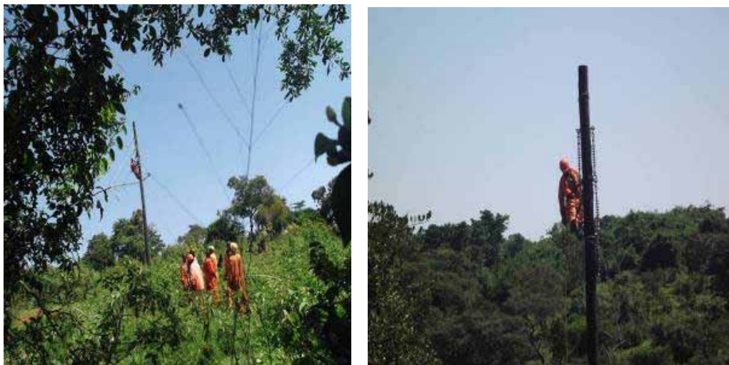
Stringing works ongoing on the Nkoge-Kashozi line
