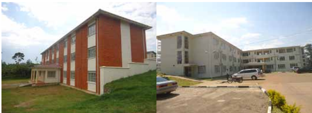
Left to right: Completed private wing and Interns and doctors house Fort Portal RRH
