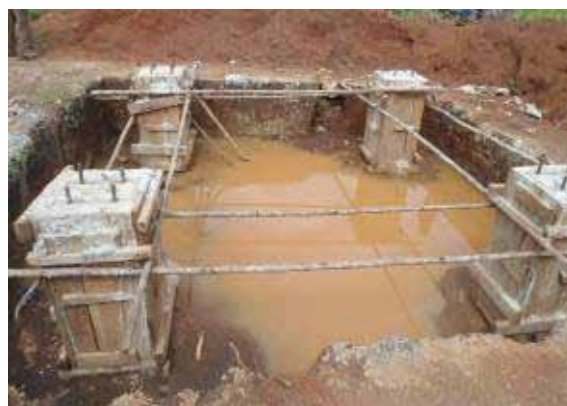
Tank basement for erection construction works
