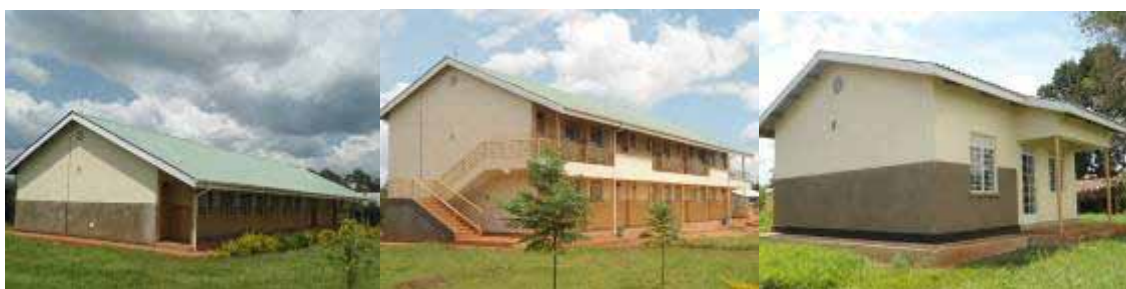
A library/computer laboratory completed, a storied 6 classroom block completed and 2 bed room house completed at Bukanga S.S
