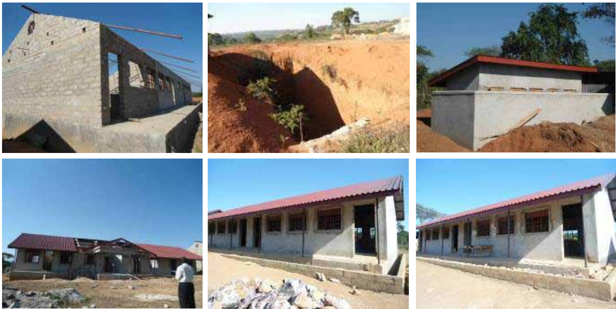
From top left: An administration block, 2 blocks of 2 classrooms each left incomplete From bottom left: A science laboratory at roofing level, a pit latrine behind the laboratory abandoned at excavation level and another VIP latrine left finishes level at Kalisizo S.S.
