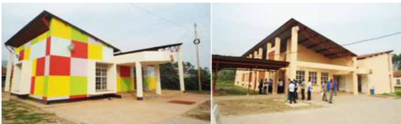
Left: Renovation of the ECO centre completed, Right: Renovation of the administration block completed at NTC Kabale under FNARI-F project.
