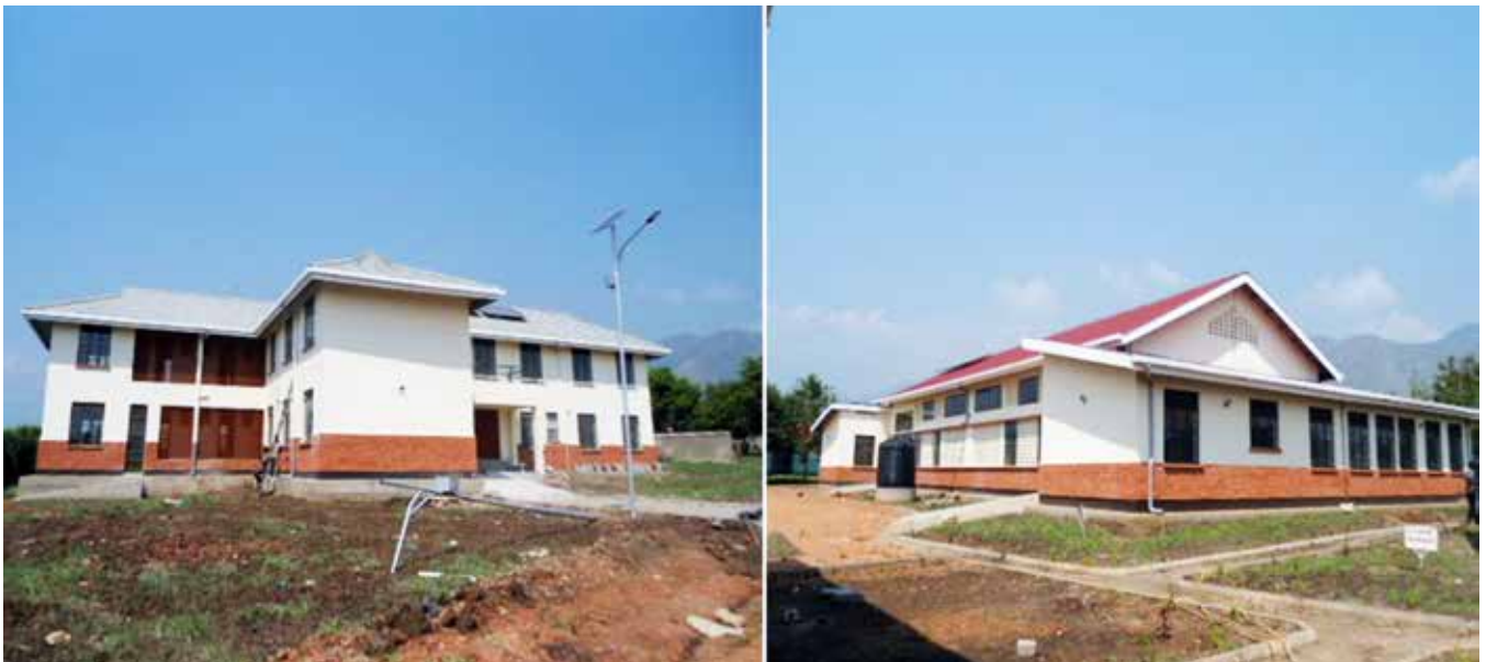
Left: A boy's dormitory completed, Right: an Electrical renewable Energy Workshop completed at Kasese Youth Polytechnic under BTC
