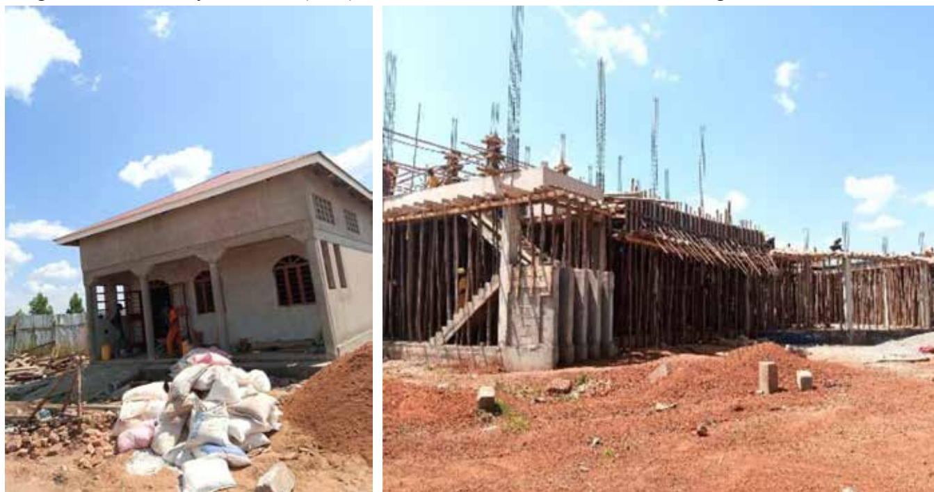
L-R: Medical store at plastering level; Multi-Purpose building
