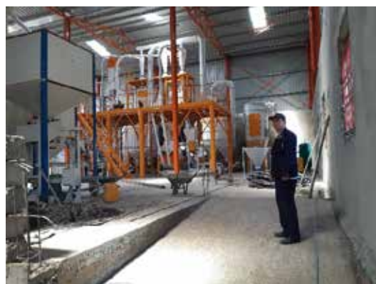
Machine installation in progress at Arua Agro Processing Facility
