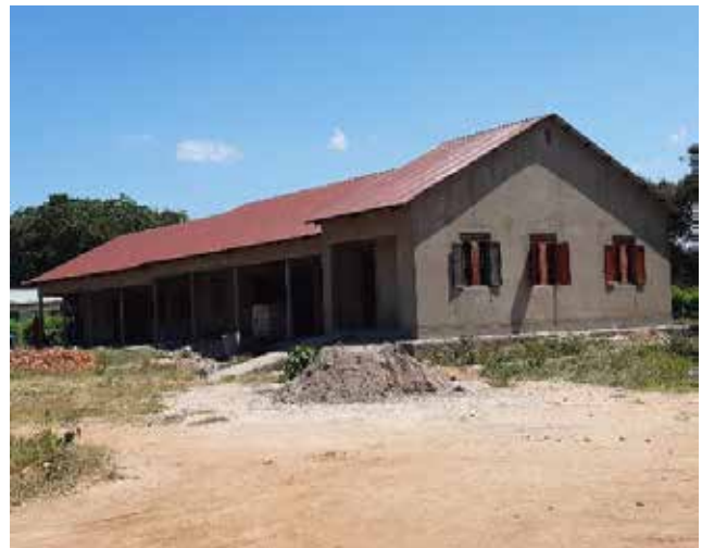
Completed classroom block at Kaler Primary School in Ngora District
