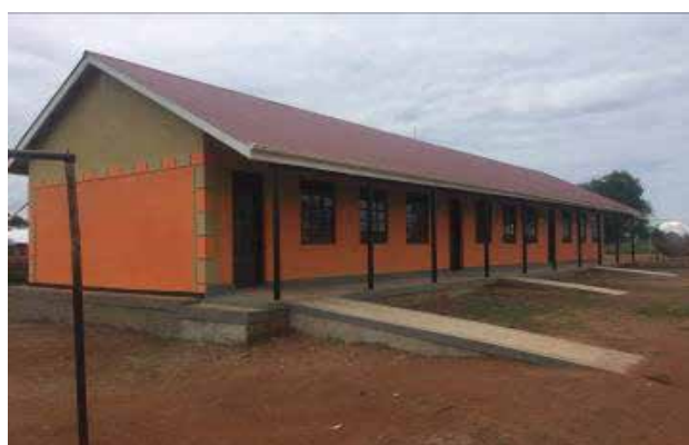
Newly constructed three in one classroom block in Kasenyi Lyato Primary School, Hoima District
