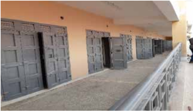
Completed lockup shops in the market in Kasese Municipality
