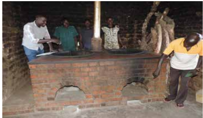
Twin kitchen improved energy cooking stove constructed at Alero Senior Secondary School, Nwoya District
