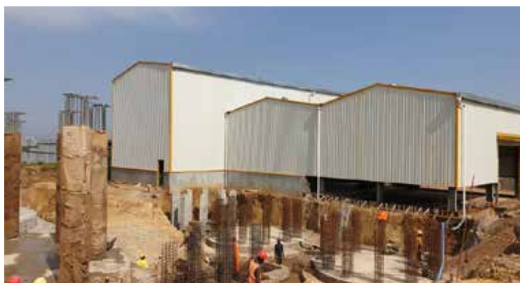
Ongoing works at Busia High Value Addition Facility
