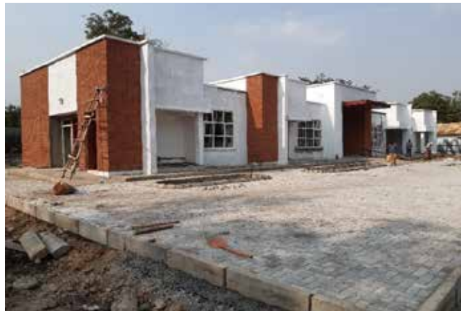
Ongoing civil works at Kasese Service Centre, Kasese Municipality
