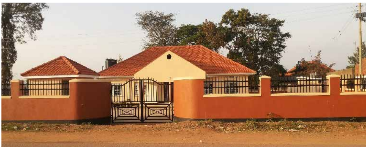
Vacant Support to Luwero-Rwenzori Regional Office at Luwero District headquarters
