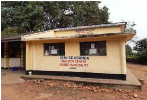
Current residence of the Kasese One Stop Centre
