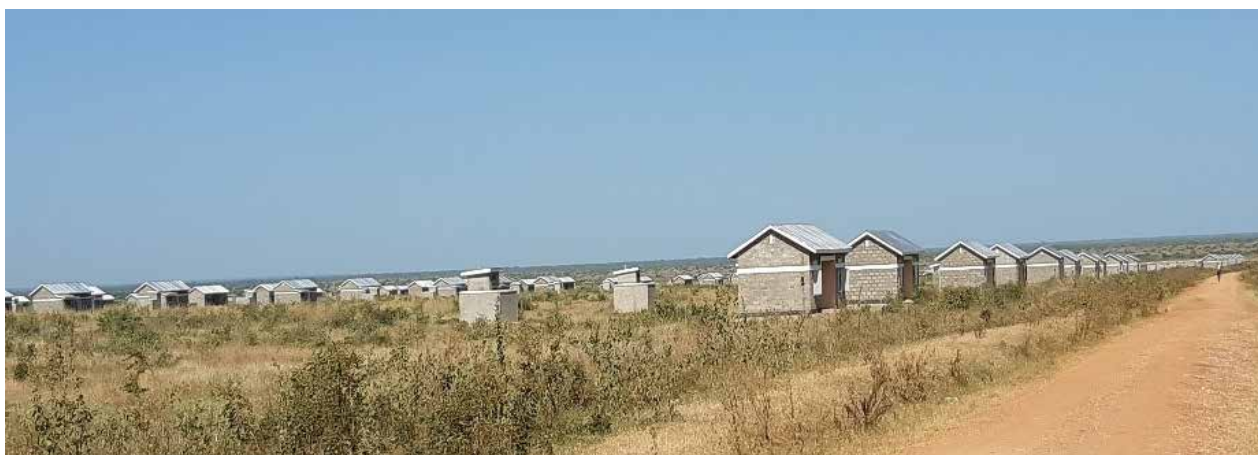
Completed housing units under Phase II in Bunambutye Town Council, Bulambuli District
