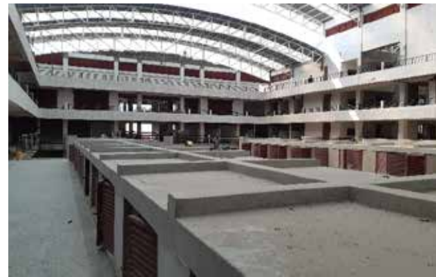
Internal finishes on Soroti Main Market
