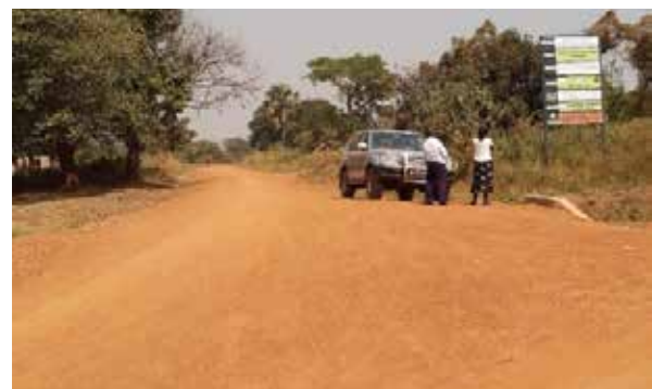
Rehabilitated Ocim Corner-Agula-Dino Community Access Road in Omoro District
