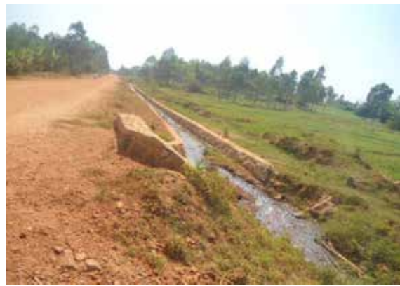
A stone pitched drain at swampy section (9+700) along Kadoto-Butebo-Kabwangasi Road
