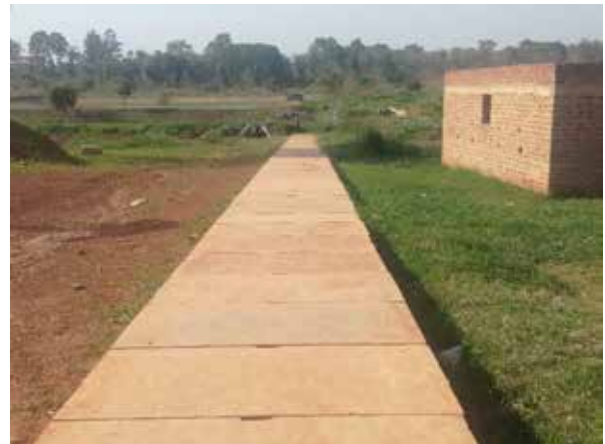
Part of the U-drainage channel covered with slabs
