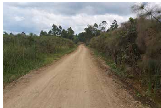
Swamp raising done on Butebe-Karambi Road under RMeM in Q2 FY 2019/20
