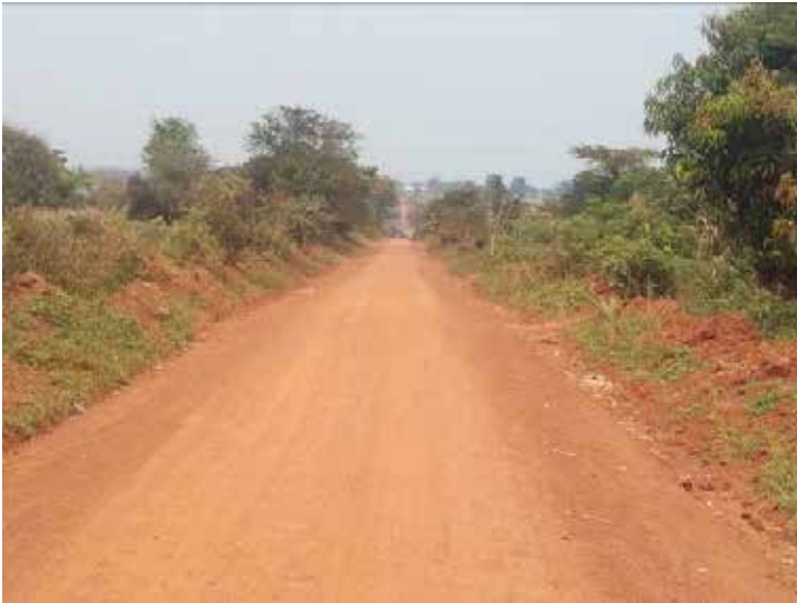
A section of Otwal-Railway-Ojwi road at 9+400
