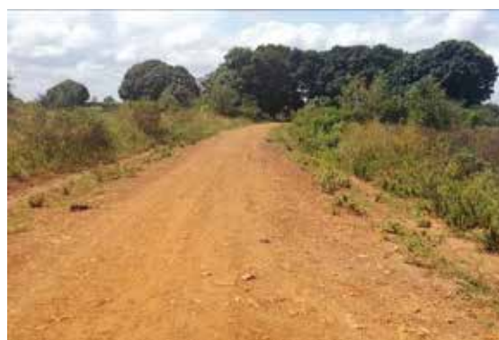
A section of Aterai-Abubur-Kelim at 1+800 section II
