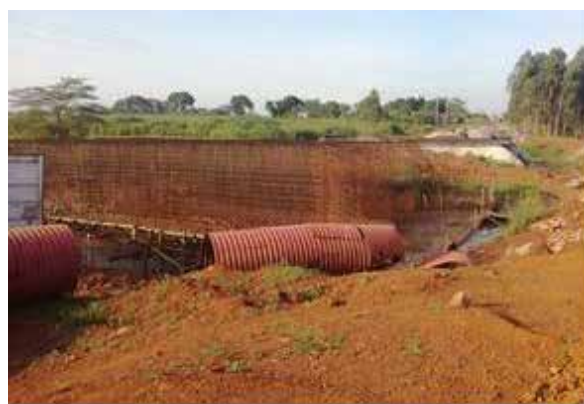
Fixed reinforcement for the abutment at Kiko 2 swamp
