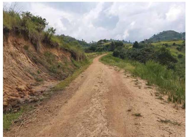
Kashenshero-Kati-Kibungo road (14km) after routine mechanized maintenance in Q1
