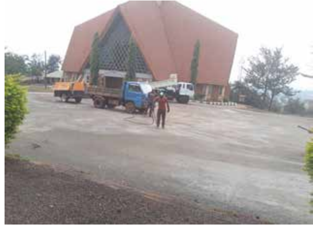
Priming of the parking area at Bugembe Cathedral in Bugembe Town
