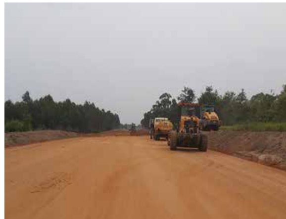
Processing of fill layers on Rukungiri-Kihihi Road
