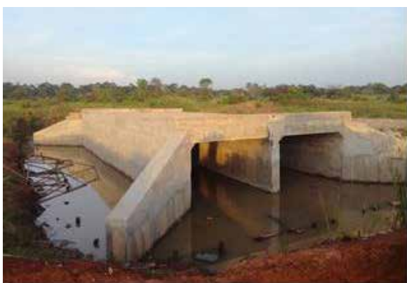
A double cell box culvert at 13+100 at the Nalwekomba Swamp Crossing
