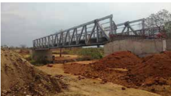
The abutment and decking of the 39.6m span Ora bridge in Okollo subcounty, Madi Okollo District
