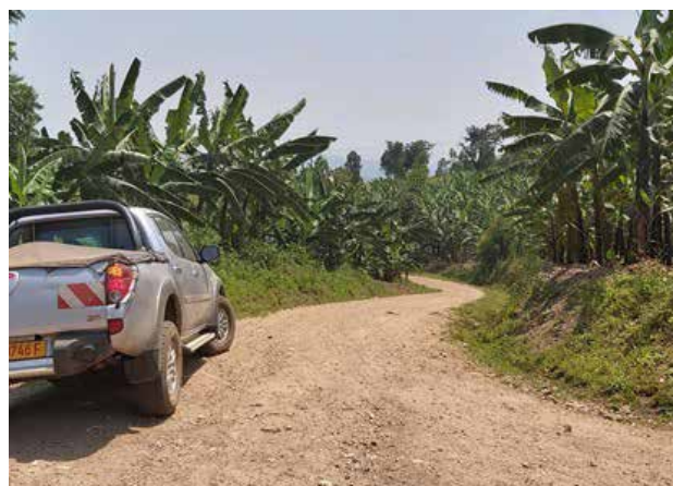
Mubanga-Kahengye Road (5.3km) after routine mechanized maintenance done in Q1 FY 2019/20
