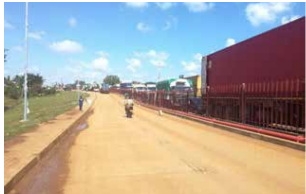
Entry road to Uganda from Kenya: Landscaping, walkway, street light posts, concrete pavement, fire hydrant pipe and fencing separating of the exit and entry roads
