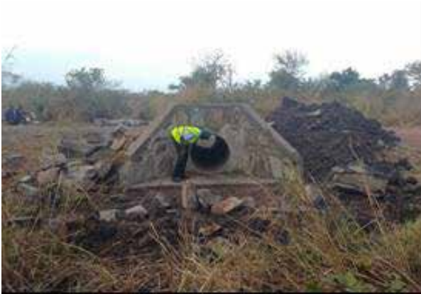
An installed culvert at km 12+900 along Bibia-Nimule section
