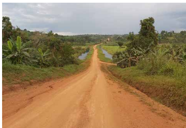
Kasambya-Nabakazi Road (23.5km) after routine mechanized maintenance in Q2 FY 2019/20
