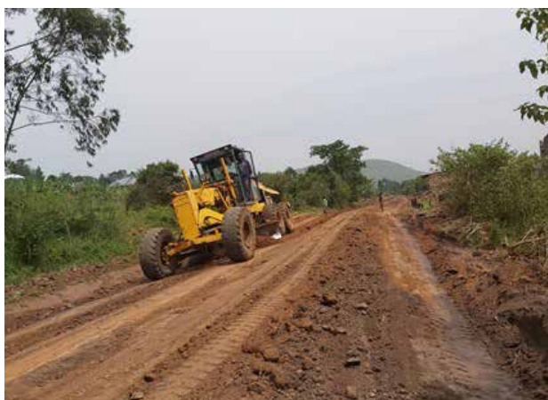
Grading works on Rwagaju-Kikade (4km), part of periodic maintenance
