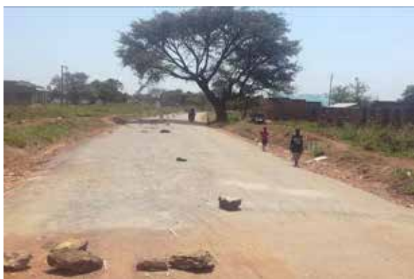
A section of Opit-Awoo Road that is being tarmacked
