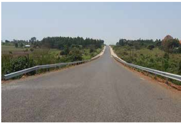
A completed section of Bulima – Kabwoya Road (66km) with guard rails at km 121+240
