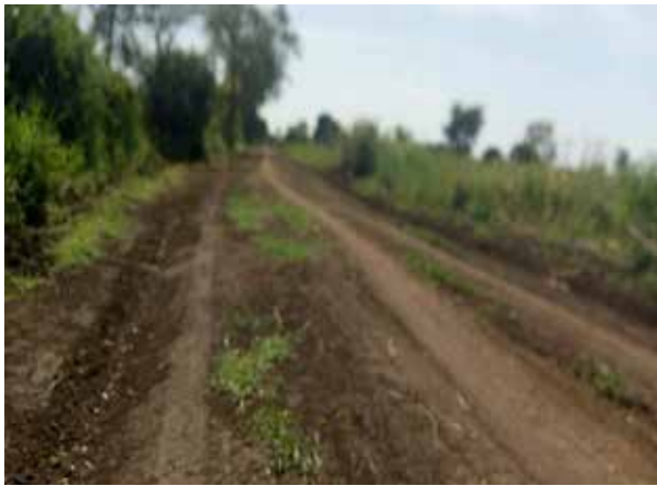
A graded section of Alyeki-Atopi at 0+000
