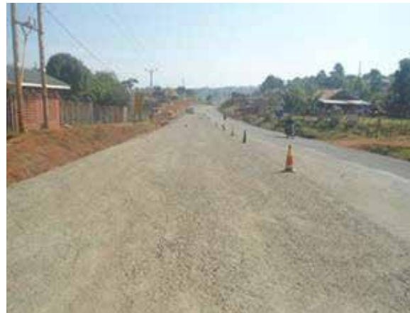
A primed section at the start of the Kapchorwa Suam Road
