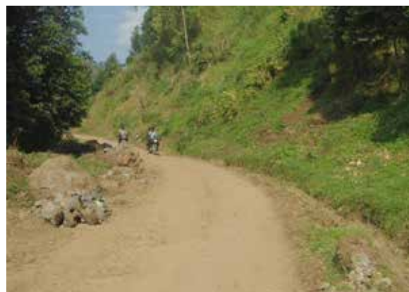
A section of Mbale - Nkokonjeru Road at km 9+100
