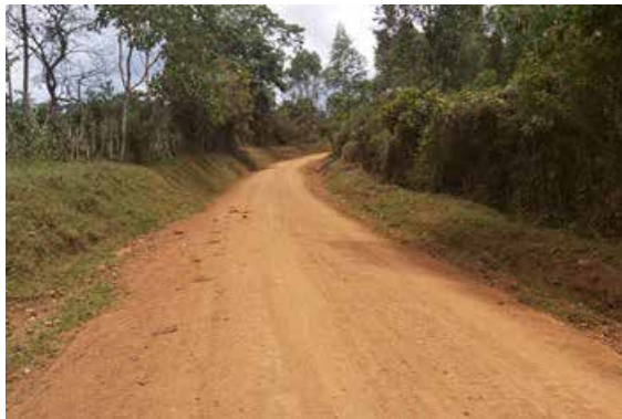
A gravelled section of Kasusu-Mahoma-Kabahango road after Routine Mechanized Maintenance (RMeM) in Q1
