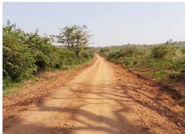
A graveled section of Kigorobya-Kibiro Road (6km)
