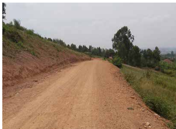
Koranorya-Rwemikunyu-Katamba-Rwagaju Road worked on under periodic maintenance in Q2
