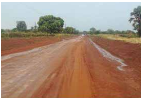
A section of Laropi-Ayugi Road at km 30+100 that was graveled
