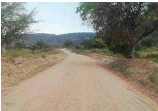
A section of Moyo-Laropi Road at km 19+000
