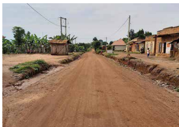
Kinoni-Nakalembe Road (3km) was gravelled under RMeM in Q2
