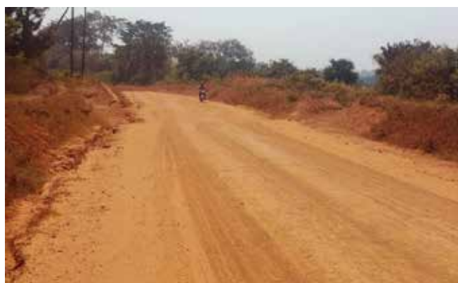
A section of Apala-Ngetta Road at km 17+600
