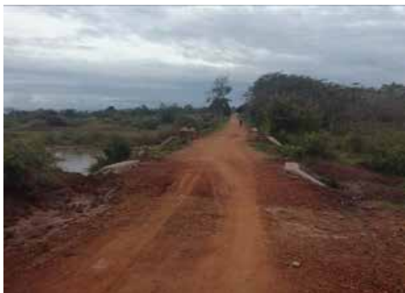
A culvert installed at 2+500 on Agule-Nyago
