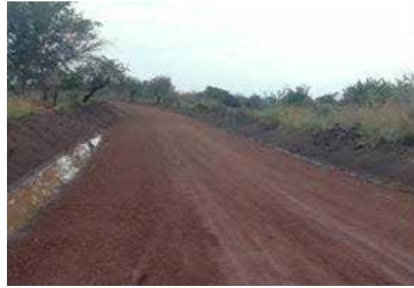
A gravelled section of Pakele-Pabbo Road at km 7+000
