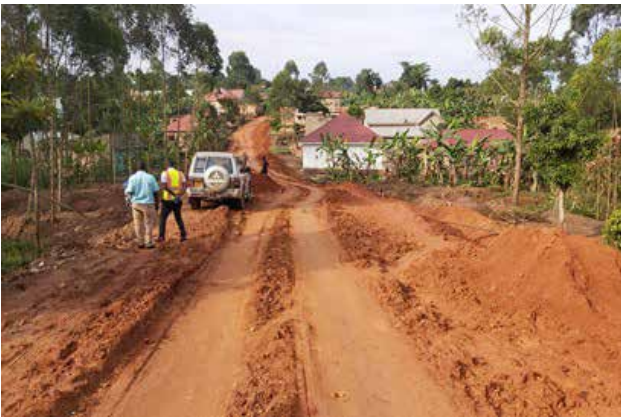
Swamp filling along Kiyudaya – Katovu Circuit roads in Mityana Municipality
