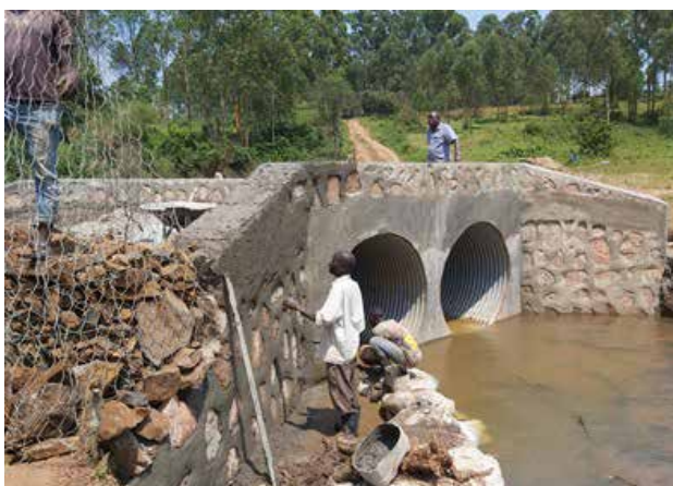
Kabaale river crossing along Ruhinda – Kabaale Road
