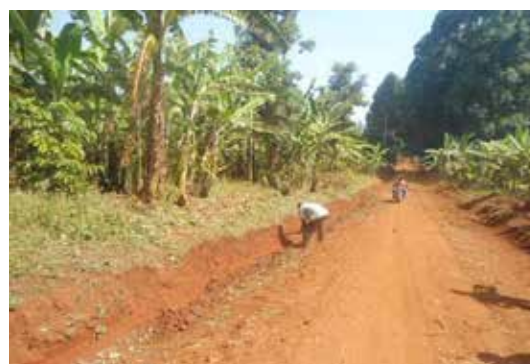
A casual carrying out manual maintenance on Kapteret-Teregres road at 3+500
