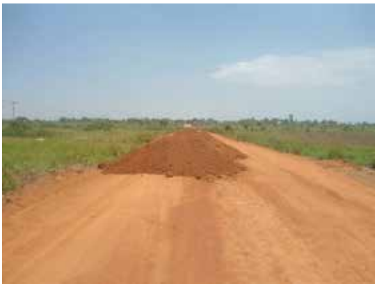
A section being gravelled along Kachumbala-Kolir-Malera-Kumi at km 45+100
