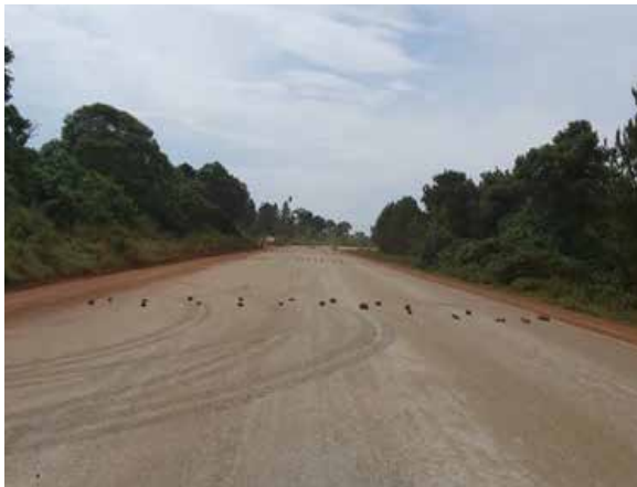
Top of base layer on Kitala-Gerege at km 8+200
