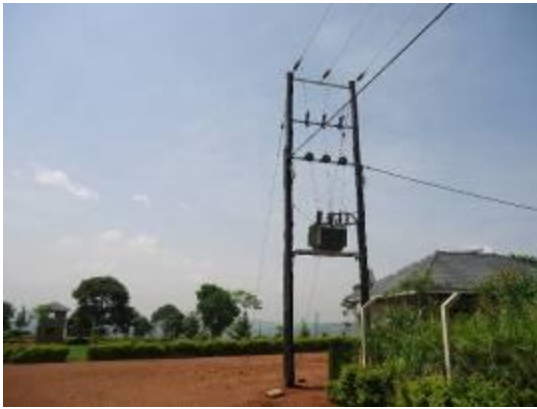
L-R: Completed transformer installation and completed construction Low voltage network at Maya Resort in Wakiso district
