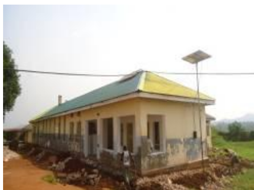
Ongoing rehabilitation of the maternity ward at Masindi Hospital
