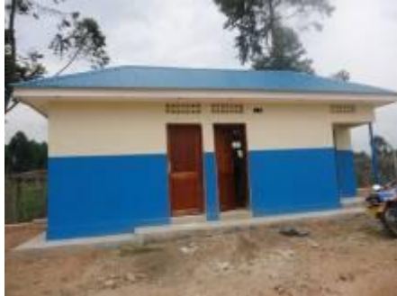
L-R: Sludge drying beds; PVC pipes; Store/Guardhouse/Water borne public toilet in Ntungamo town
