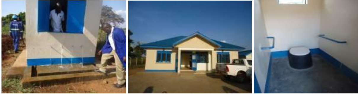
L-R: Functional water kiosk; Water Office; PWD stance at Pajule P/S all in Pajule Town Board
