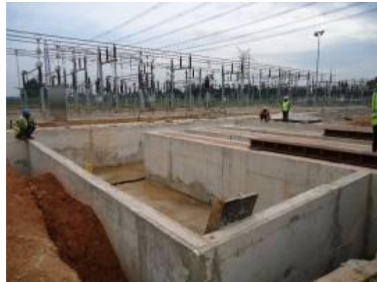
L-R: Form and steel works in preparation for concreting; Transformer foundation in advanced completion stages at Kawanda substation for the ESDP project
