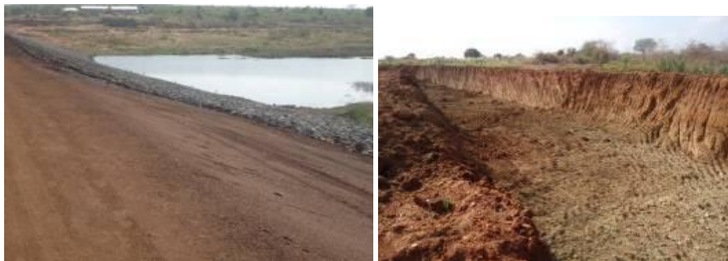
L-R: Riprap rock embankment protection upstream; Excavated spillway in Panyango sub-county
