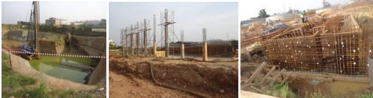
L-R: Pile foundation excavation for inlet pumping station; Columns for the pretreatment structure/chemical house; and Reinforcement bars for the trickling filter pumping station walls at Bugolobi, Kampala district
