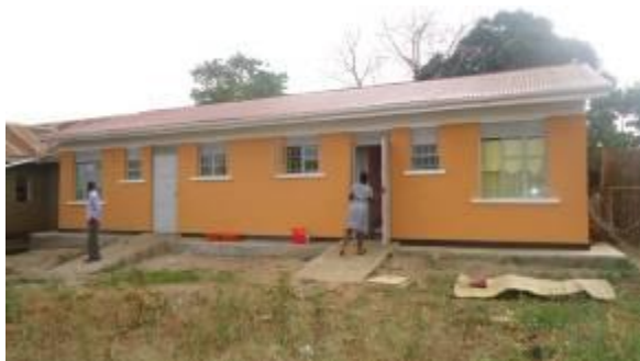
Completed staff house at Biiso HCIII, Buliisa district
