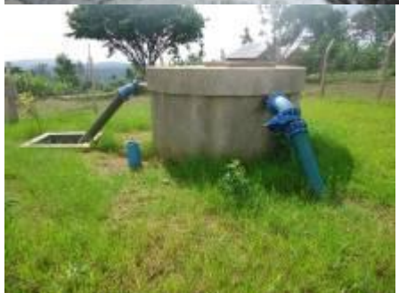
L-R: Part of the protected water source; Chemical house with office and laboratory; 10m 3 BPT in Manafwa district
