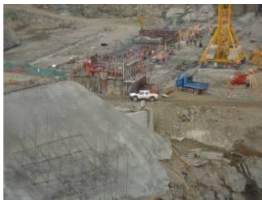
L-R: Form, steel and concreting works at the dam area in Karuma HPP in Kiryandongo district
