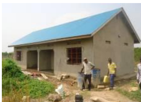
Construction of the staff house at Buliisa general hospital
