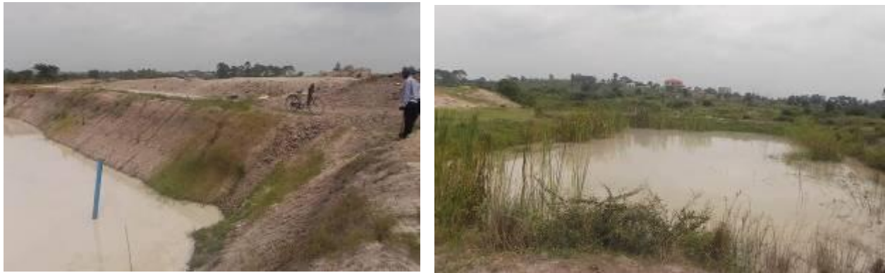
L-R: Adjustable water pipe was installed in valley tank to drain water into the fish ponds, and valley tank were the tilapia were being raised at MBAZARDI in Mbarara district
