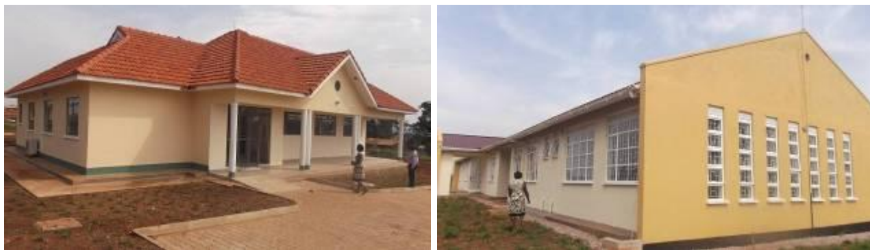
L-R: Completed nutritional laboratory and administration block at Nakyesesa Centre in Wakiso district
