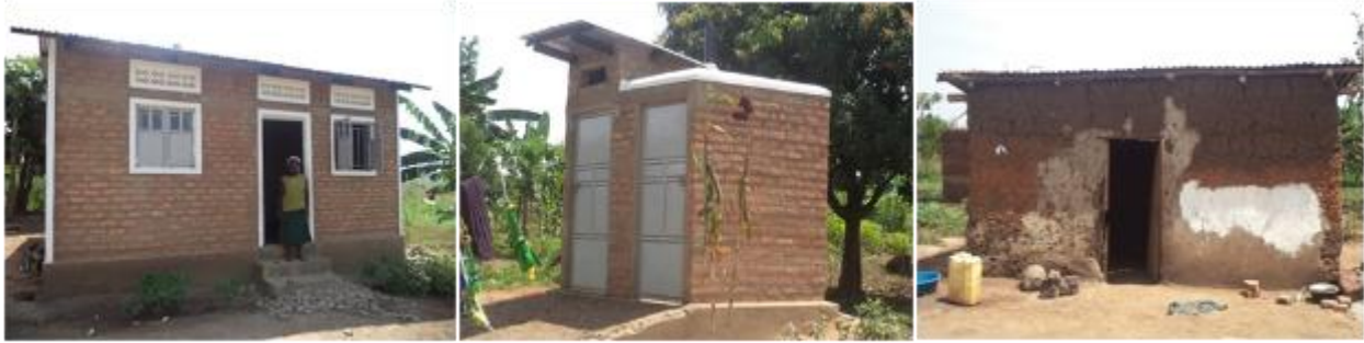
L-R: Robinah Nekesa’s house; the bathroom facilities; house where beneficiary is currently residing as the floor of the new house is being completed in Zone A2, Kiryandongo district
