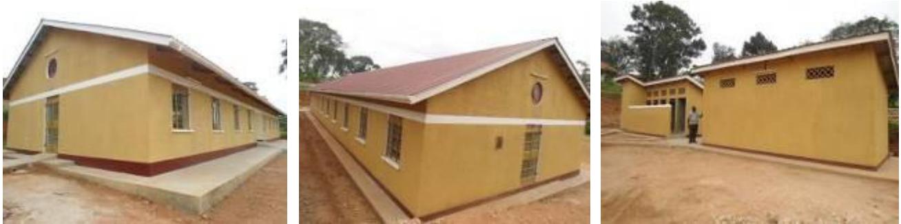
Left: A girls' dormitory, Right: A boys' dormitory; and a boy's six stance VIP latrine and a shower block completed at Kabukunge PTC
