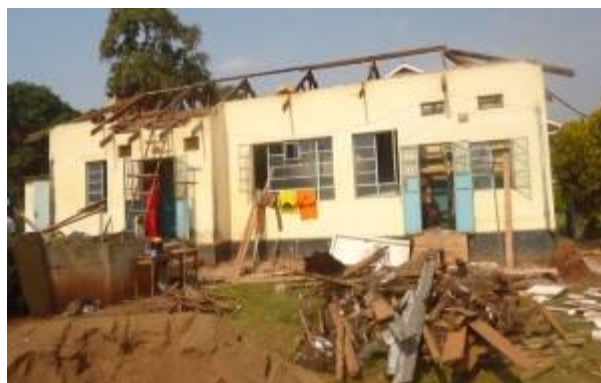
Ongoing renovation of the operating theatre at Masindi Hospital
