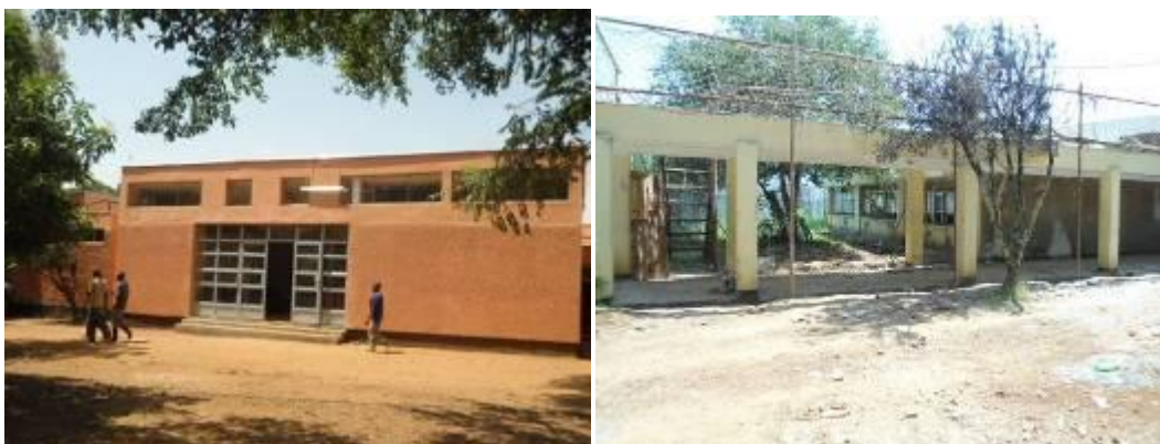
Left: Block 'Y' renovated, Right: Renovation of block 'X' on going at Kaliro NTC
