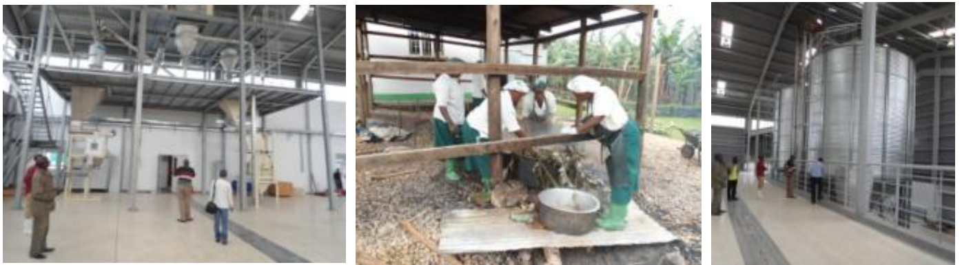
L-R: Partially installed Hammer mill, ladies preparing instant Tooke and installed Silos at Nyaruzinga-Bushenyi
