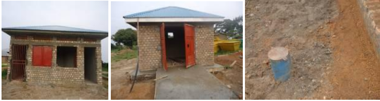
L-R: 13 stance water borne toilet at the sub-county; Pump station 1 at Kabasese; Unmotorized production borehole of pump station 2 in Kabasese A cell Bukakata sub-county, Masaka district
