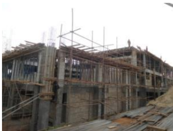
Construction, of the new faculty of Business Computing at MUBS
