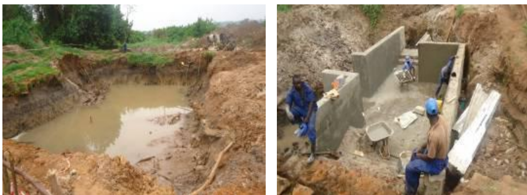
L-R: Excavation of the reservoir and construction of the community well at Kiboga Hospital
