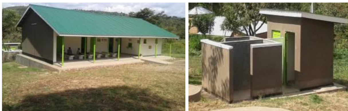
L-R: Completed OPD and pit latrine at Bukiende HCIII, Mbale district
