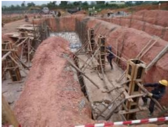
L-R: Form and steel works in preparation for concreting; Transformer foundation in advanced completion stages at Kawanda substation for the ESDP project
