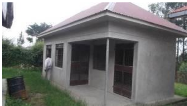
The crop mini laboratory under construction at Bushenyi DLG headquarters
