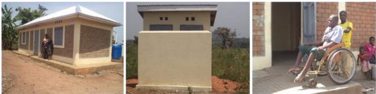
L-R: Sam Watendo with his four children standing by house he received; toilet and bathroom;, Weleka Clement with his three children in front of the house he received in Zone B1 in Kiryandongo district
