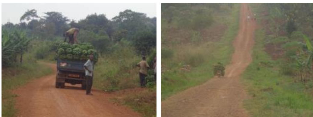
Left: Produce being loaded for transportation to Mubende town from farms and main roads along the rehabilitated Kansotoka–Buta 14.8km road
