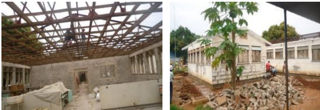
Different rehabilitation works ongoing at the maternity ward of Apac Hospital
