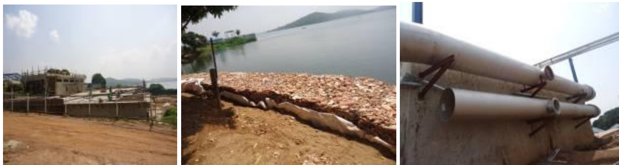
Left: New reservoir and pumping station; Center: Gabions on the lake shores; Right: Sludge recirculation pipes at Ggaba I water treatment plant
