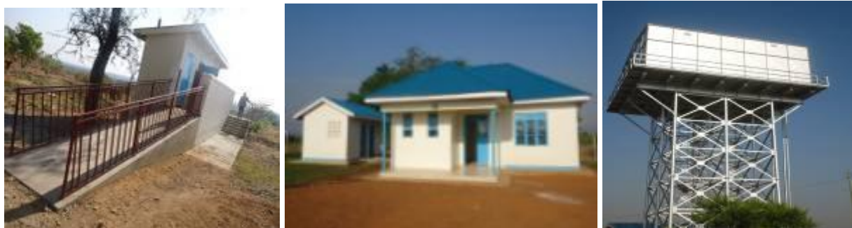
L-R: Institutional Ecosan Toilet at Okollo P/S; Water Office; 200m 3 reservoir tank in Okollo town
