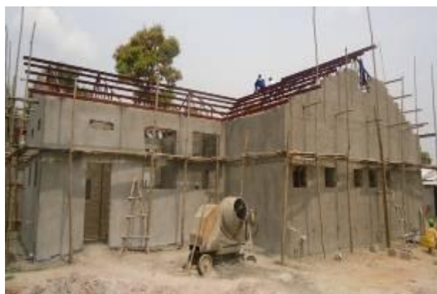
Ongoing construction of the theatre block at Aboke HCIV, Kole district
