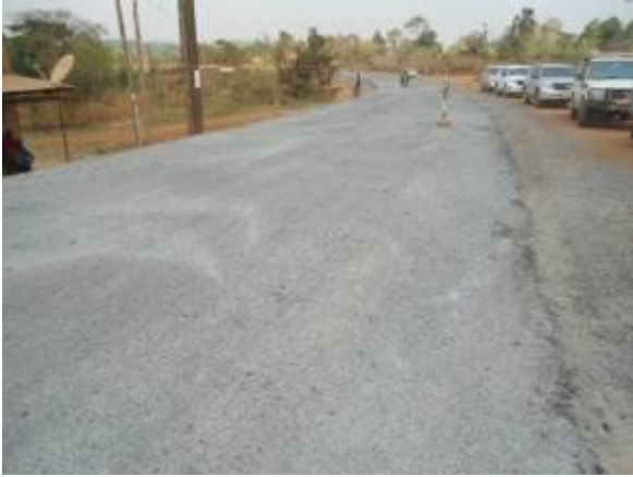
First seal works at Km 90+145 at Kyenjojo-Kagadi-Kabwoya (100km)
