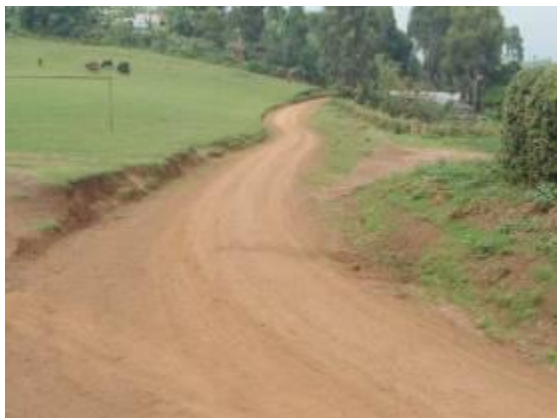
A well graded section of Kagarama-Rubare Road at Km 5+000
