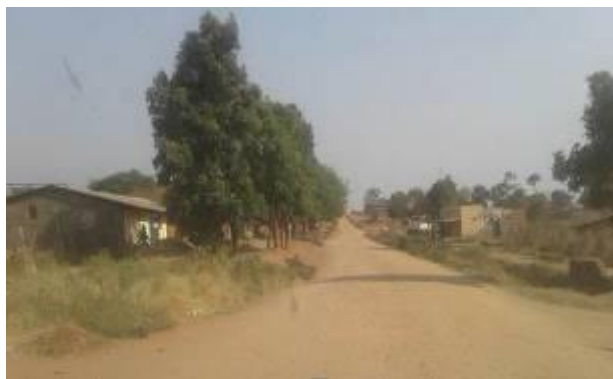
A graded section of the Kanawat–Kabong Road within Kabong trading centre
