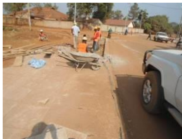
Ongoing drainage works along Rukurato Road (USMID)
