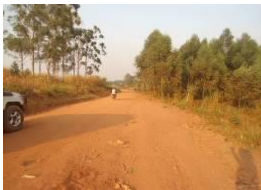
A section of Isunga-Bugwara-Kikwaya Road at km 14+900
