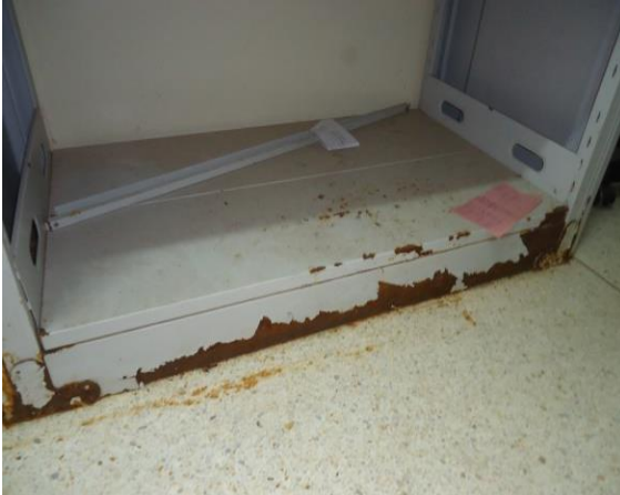
L-R: Rusted metallic shelves and a clogged broken drainage channel at the Services Block, Kawempe Hospital
