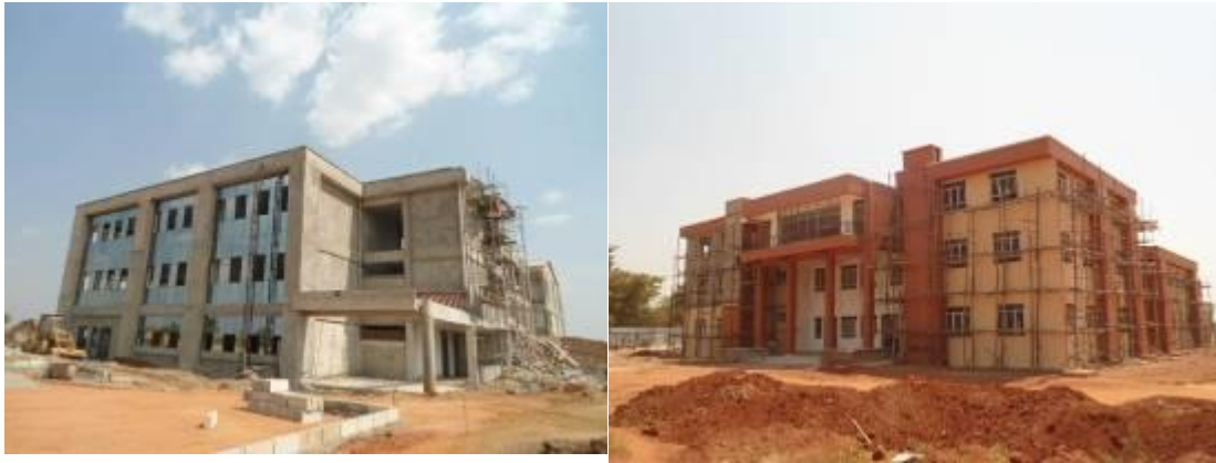
L-R: The agricultural block at 88% and the library block at 90% progress at Gulu University
