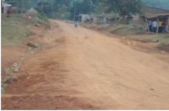
Mugalike-Kyanaisoke Road section at Km 0+000
