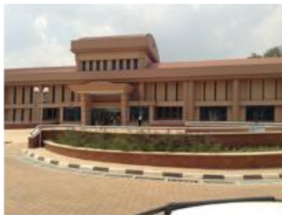
Completed but not fully functional NARC Building at Nakasero, Kampala
