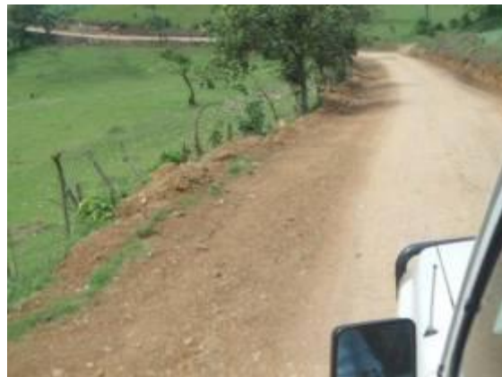
A section of Nyakishana-Engaju Road at 0+000
