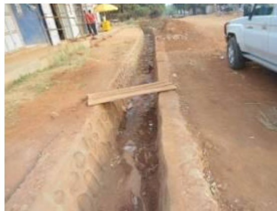
The stone pitched drain on Buzabo Road
