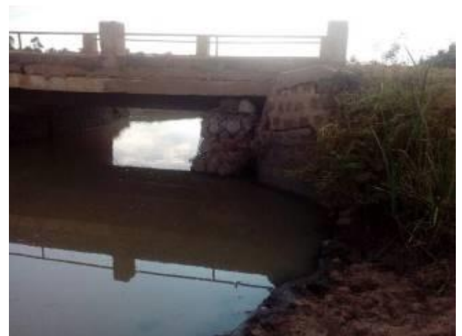
A dilapidated Kaboloi bridge that was constructed in 1960s requires immediate replacement along Agule-Pallisa Road in Pallisa District
