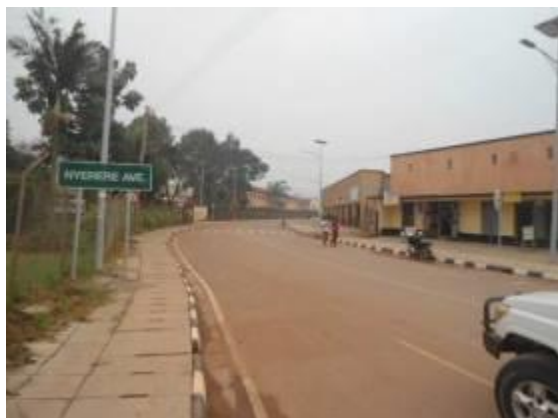
Completed Nyerere Avenue (0.42 km) in Central Division rehabilitated under the USMID Project
