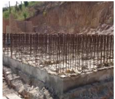
L-R: Water borne public toilet at Sekanyonyi health center IV; Excavations for distribution mains; Steel reinforcement for reservoir tank studs in Sekanyonyi Town, Mityana District
