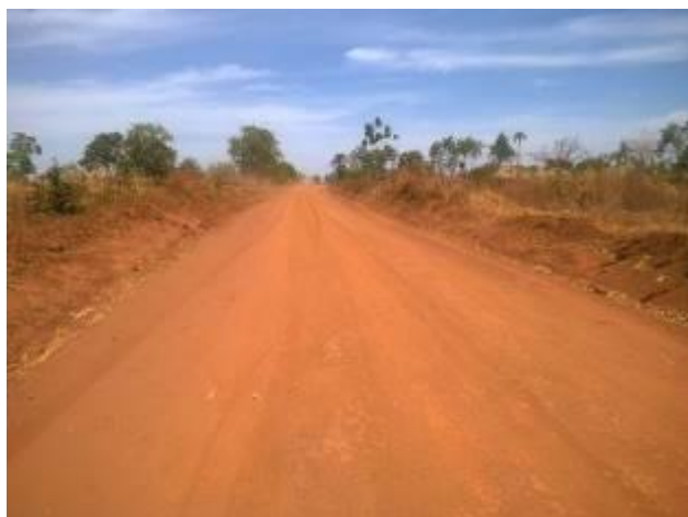
Well graded section along Allidi-Awangi Road
