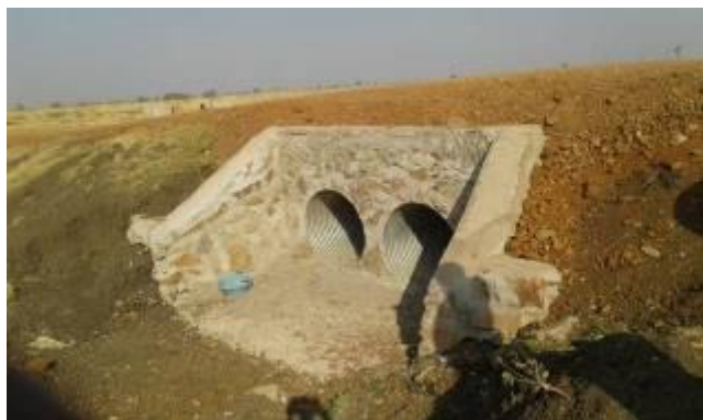
Constructed two cell culverts along Kotido–Abim Road
