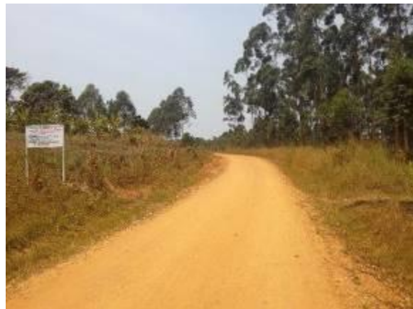
A well graded but not gravelled section at Km 8+000 which is the end of the project road
