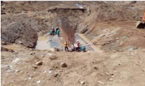
Ongoing foundation works at Nalakasi bridge in Kaboong District
