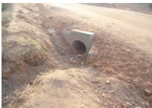
A culvert of 600mm encased in concrete at km 14+900 Isunga-Bugwara-Kikwaya Road
