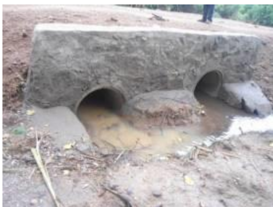
A culvert installed at km 3+200 along Harunyinya-Kyarugumba-Mukagera-Kesonbiire-Kasansa-
