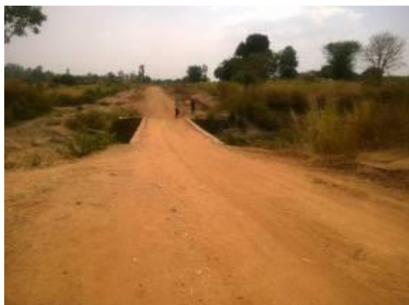
A graded section along Konzi-Onzilabori Road
