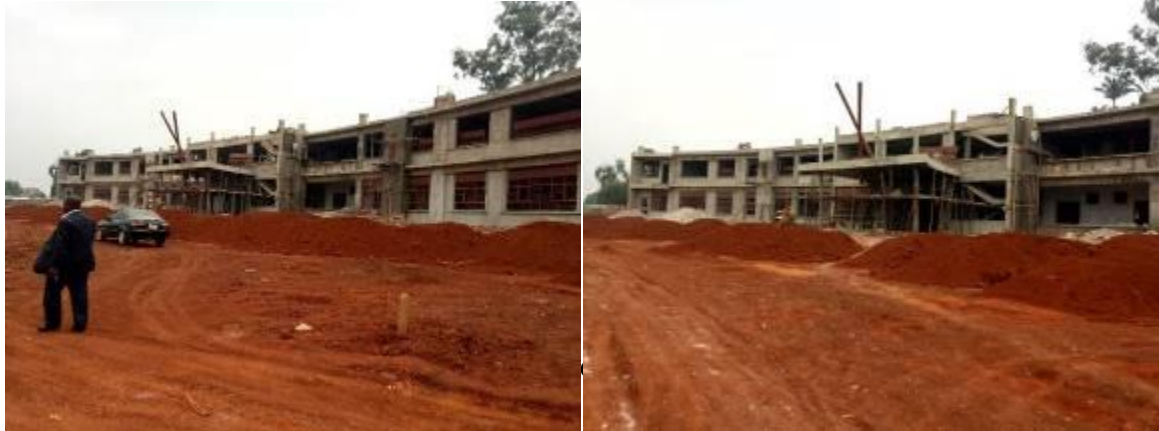
Ongoing construction works on the Central Lecture Block at 75%
