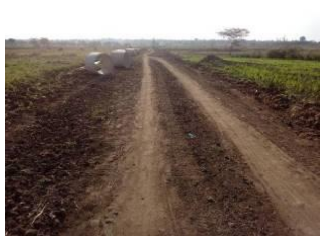
Gravel stock piles (L) and a graded section waiting culvert installation (R) along Agulo-Ogonyo Road in Pallisa District
