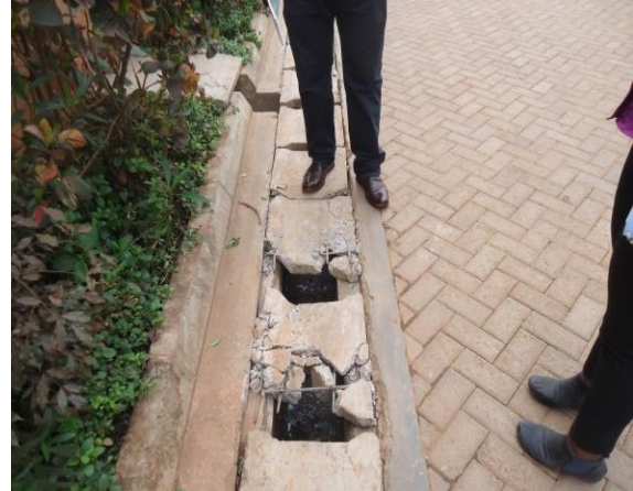
L-R: Rusted metallic shelves and a clogged broken drainage channel at the Services Block, Kawempe Hospital
