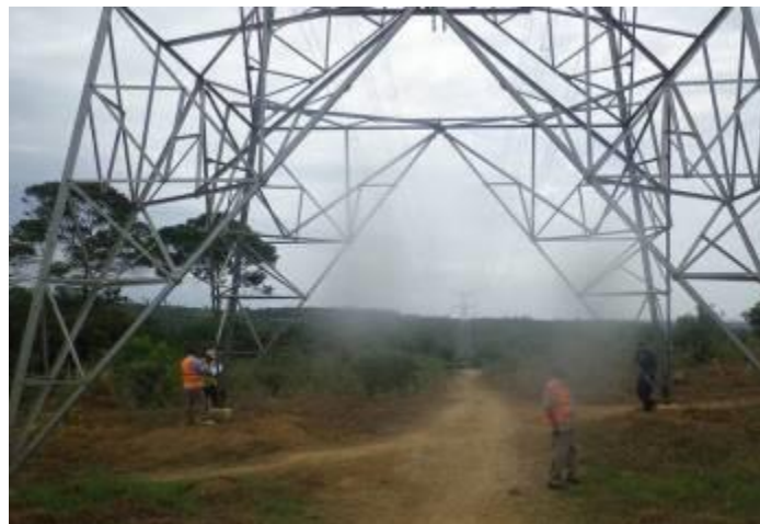
Engineers inspecting a newly completed section on the Kawanda-Masaka Transmission line
