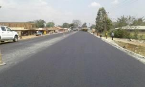
Asphalt surfacing works ongoing at KM 30 in Bulambuli Trading Center along Sironko-Muyembe Road
