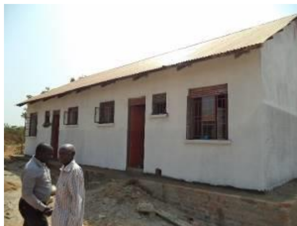
Newly constructed residence for teachers in Serere District
