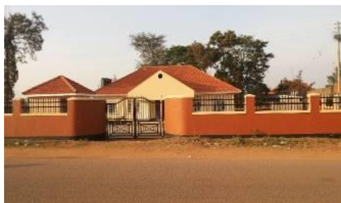
Completed Regional Office at Luwero district Headquarters under Support to LRDP
