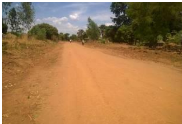
Graded section of the Anaka TC-Amuru TC Road
