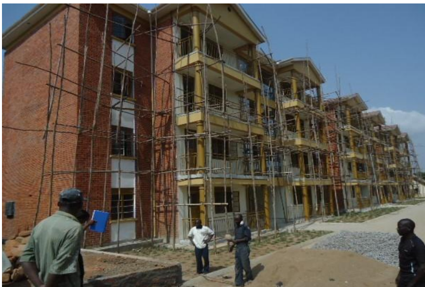
A 24-unit staff house at Soroti RRH at substantial completion
