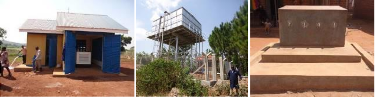
L-R: Iziru Pump station; 109m 3 reservoir tank; Public water kiosk at Buyengo sub-county, Jinja District
