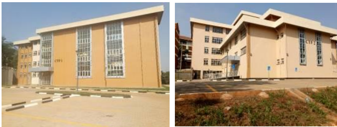
L-R: Central Teaching Facility I, Central Teaching Facility II completed at Makerere University
