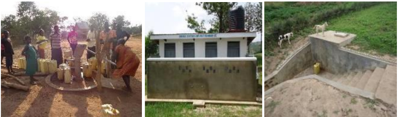
L-R: New borehole at Bulungana village, Kagulu sub-county in Buyende District; School toilet, a spring in Kibunda Cell, Buyanja sub-county, Rukungiri District
