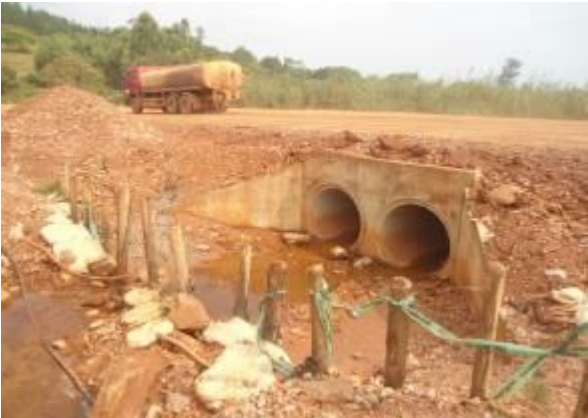
Double cell culverts of 900mm laid at km10+500
