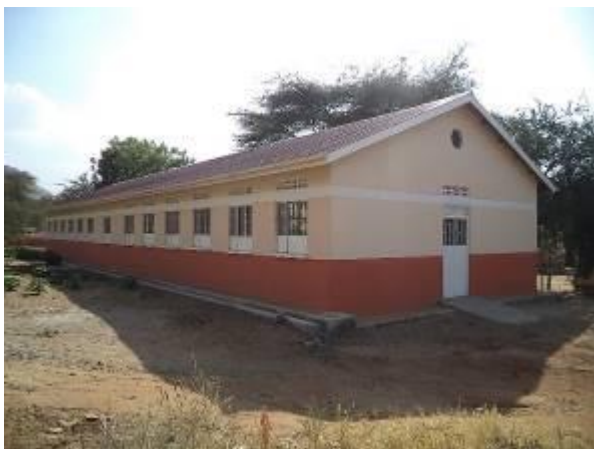
Completed girls dormitory at Moroto High School in Moroto District
