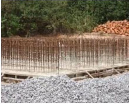
L-R: Steel reinforcements for the reservoir tank studs; Water office; Public toilet at Kikonge trading center all in Zigoti Town, Mityana District
