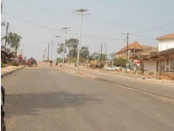
A two line culvert bridge structure at km 1+500 along Kasasa-Kasingo Road
