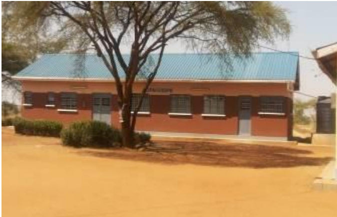
Completed Operating Theatre at Nadunget Health Centre III in Nadunget sub-county, Moroto District
