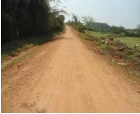
A section of Ruhumba-Byanamira-Kashwa at km 0+000
