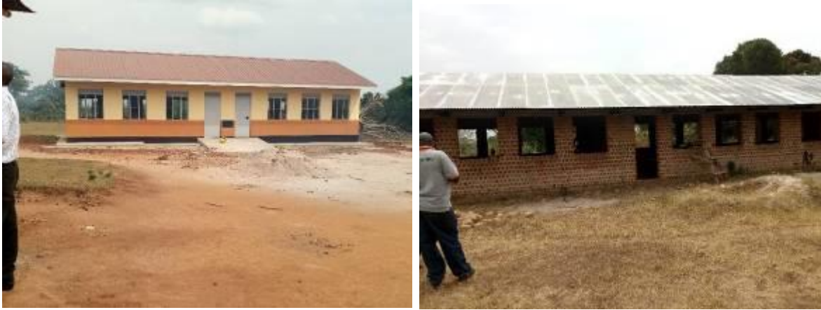
L-R: Completed classroom block at Kakubansiri Primary School in Gomba District; Classroom block at Wakayamba Primary School in Nakaseke District awaiting plastering
