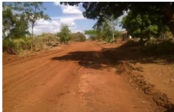
Graded and shaped section of Laminakulu Road
