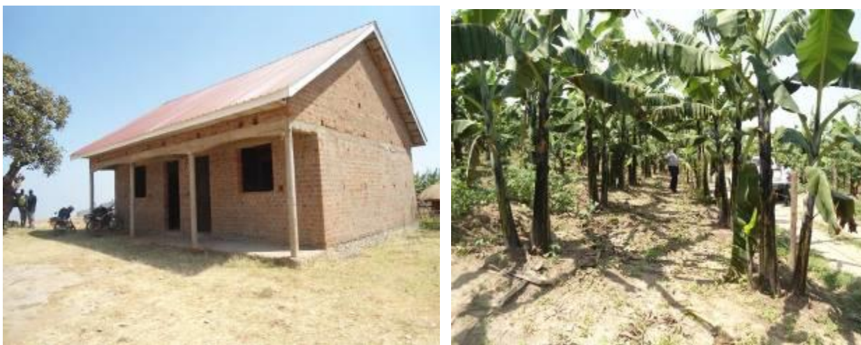
Plant clinic and animal laboratory building under construction at Kween District Headquarters (left) and banana demonstration garden in Bushenyi Municipality (right)
