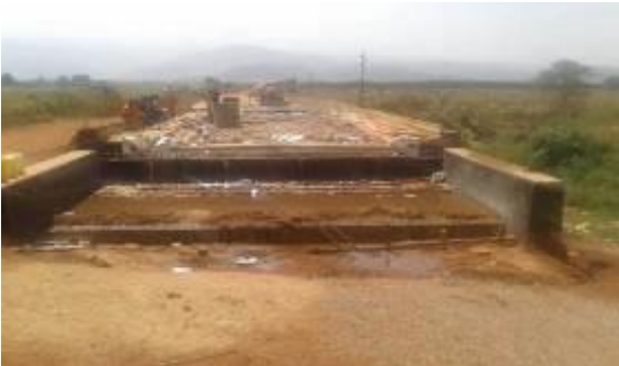
Finished deck for the Seretiyo Bridge along Muyembe – Nakapiripirit road
