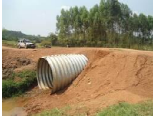
An armco culvert installed along Kashongi-Kantaganya Road at km 11+700
