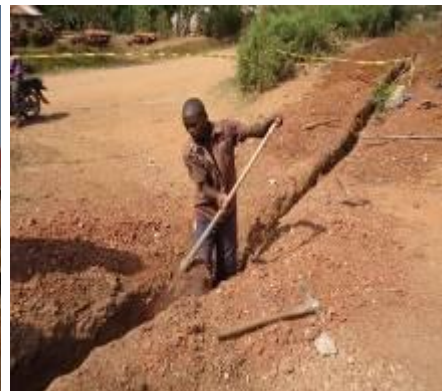
L-R: Water borne public toilet at Sekanyonyi health center IV; Excavations for distribution mains; Steel reinforcement for reservoir tank studs in Sekanyonyi Town, Mityana District
