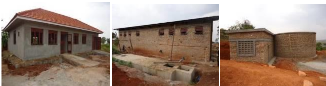
L-R: Water office; Public water borne toilet; Sump and pump house of Nyamiyonga WSS in Rugaga sub-county, Isingiro District
