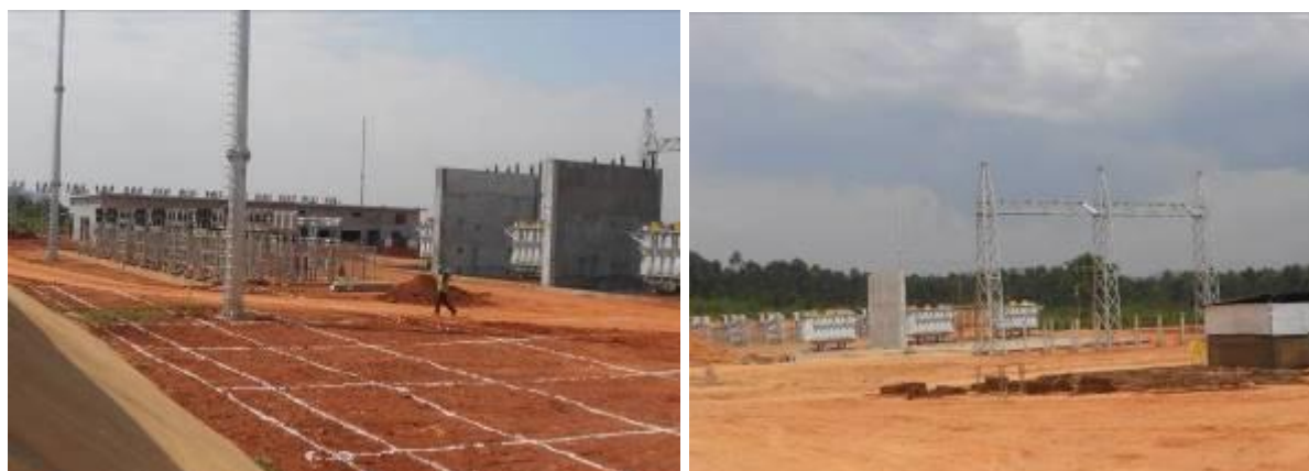
L-R: Partially completed Namanve South substation; On-going works at Mukono substation
