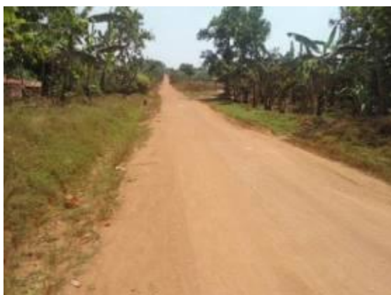
A section of Kibibi-Butaka Road at 0+000
