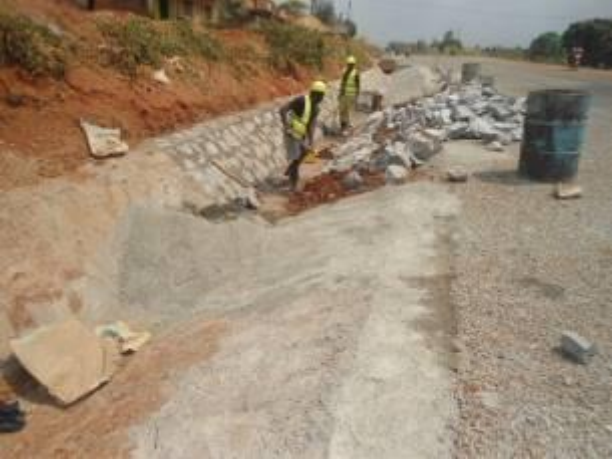
Stone pitching works at km 6+702 at Bulima-Kabwoya Road (66km)
