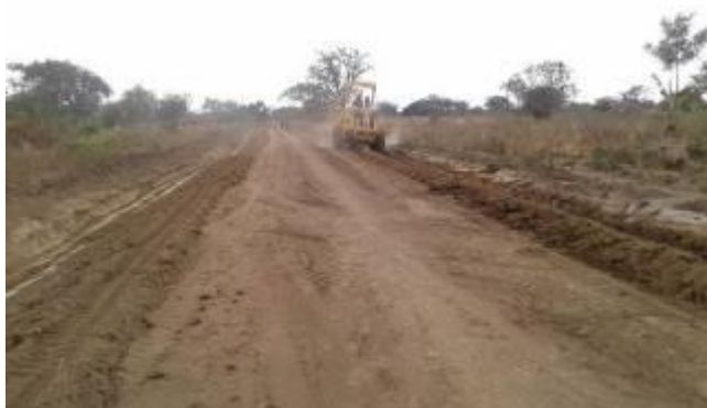
Grading and shaping ongoing along Ochen – Araso Road
