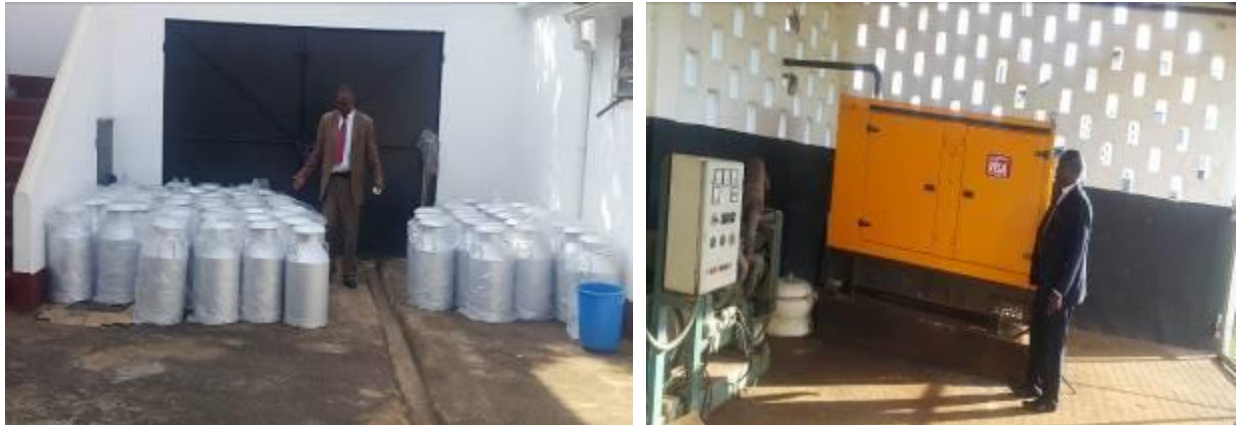
L-R: Part of the milk cans consignment at DDA Head office awaiting distribution and a 60KVA generator procured and installed at Entebbe Dairy Training School in Entebbe Municipality, Wakiso District
