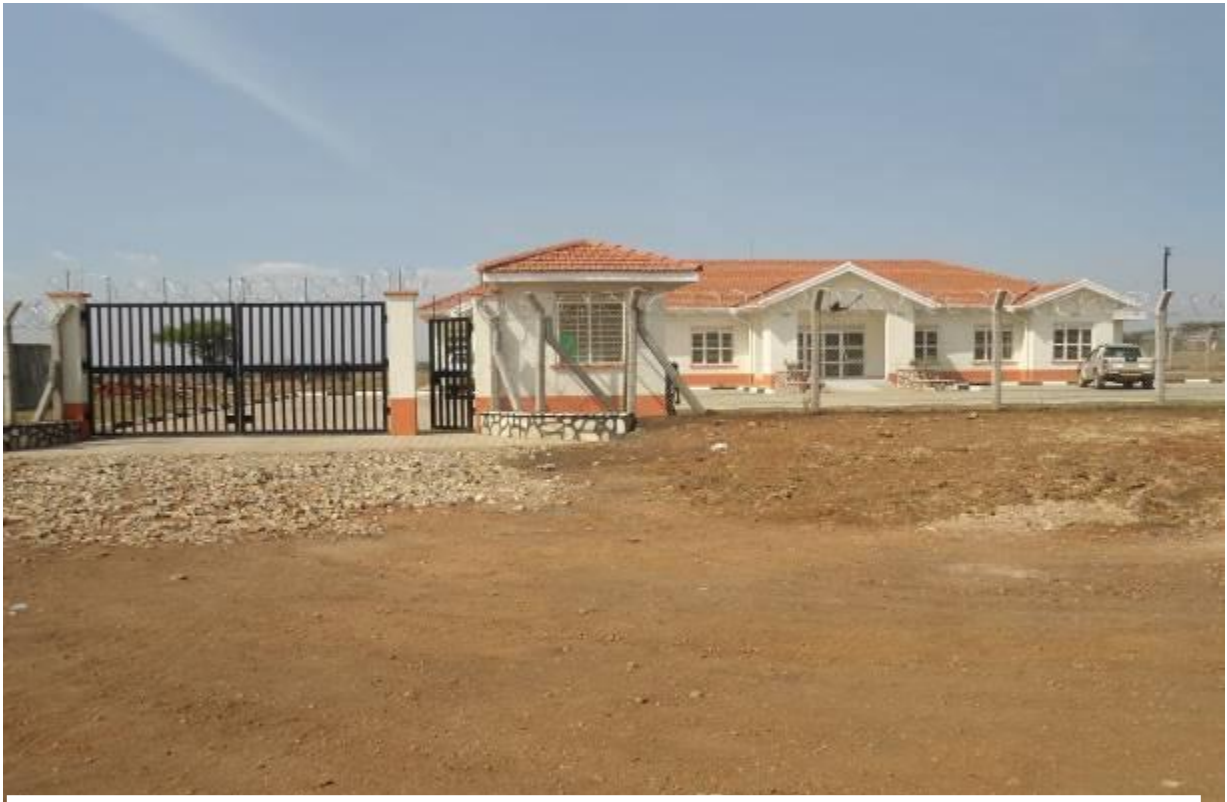
Completed Regional Mineral Beneficiation Center in Moroto District
