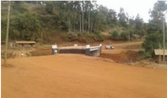
Finished deck for Nyalit Bridge in Bukwo District
