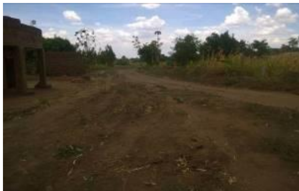
Part of the opened up Kiguka Road
