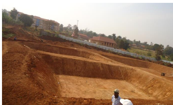
L-R: Section of the completed fence and excavated chambers of the lagoon at Hoima RRH
