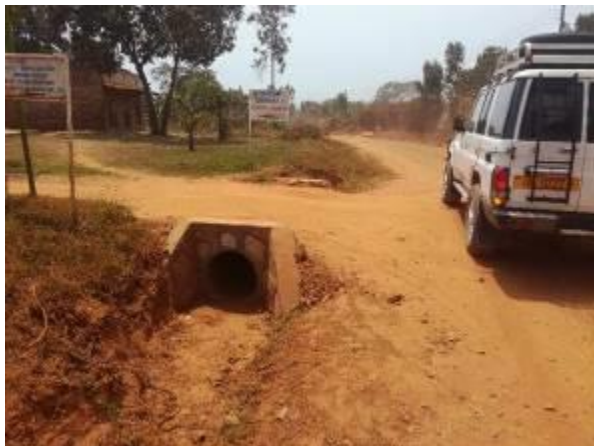
A 600mm diameter access culvert at Km 0+700 on Wabigalo-Busuubuzi-Wabiyinja Road
