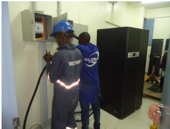
L-R: Installation of the UPS for the imaging equipment; Broken shelf at Kirruddu Hospital
