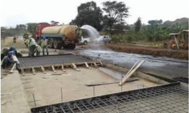
Preparation of a reinforce concrete surface works at KM 36 along the Muyembe-Kapchorwa Road
