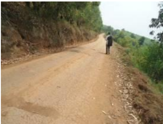
A section of Kitega-Mushasha-Buhuga Road at km 1+500
