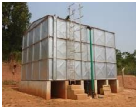
L-R: Surface pumps; 100m 3 reservoir tank; Water office block in Gombe Town, Mpigi District
