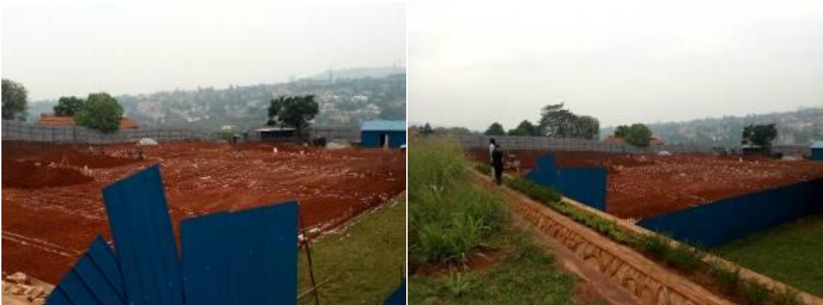
Department of Lands and Architectural Science block at foundation level
