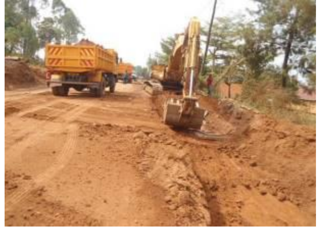
On-going clearing works along Katwe Road (USMID-Batch 2)
