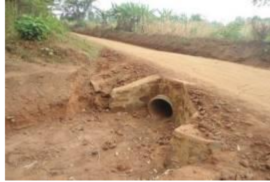
A culvert laid along Mugalike-Kyanaisoke at Km 6+000
