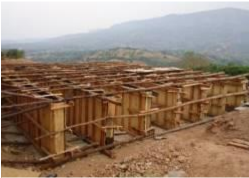
L-R: Shuttering for stud columns of the 222m 3 reservoir tank in Nyabuhikye sub-county; Site clearance at the treatment plant in Igorora Town Council, Ibanda District
