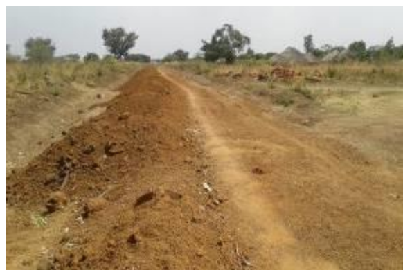
Dumped gravel yet to be spread along Aberani – Yalakwai Road
