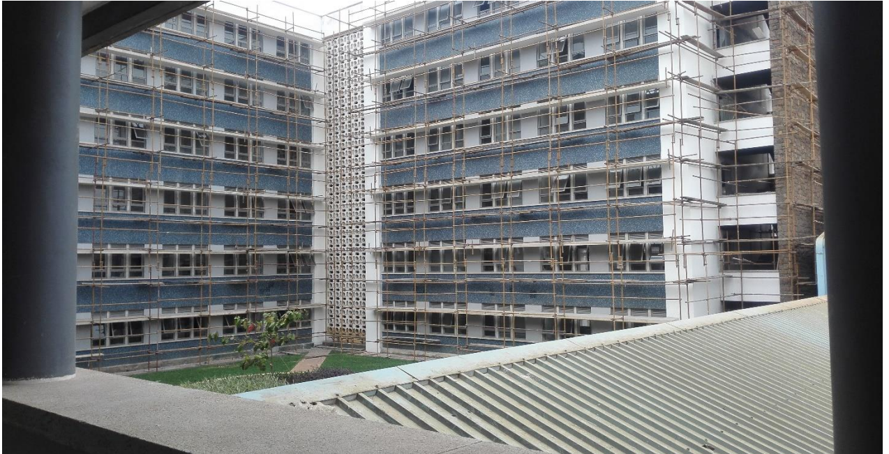
Ongoing works at Mulago Hospital Complex
