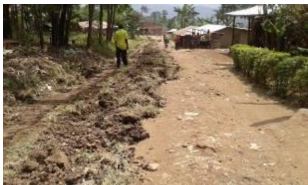
Bush clearing of Bugibuni – Kidega Road in progress
