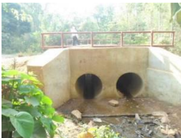
A two line culvert bridge structure at km 1+500 along Kasasa-Kasingo Road
