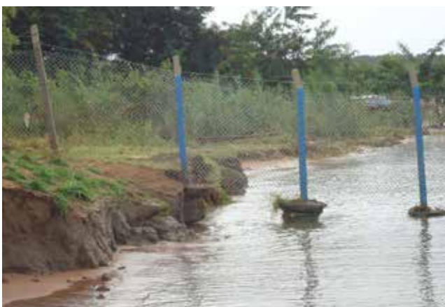
L-R: Fish handling surface sand fencing destroyed by waves from the lake at Mbegu landing site in Hoima DLG
