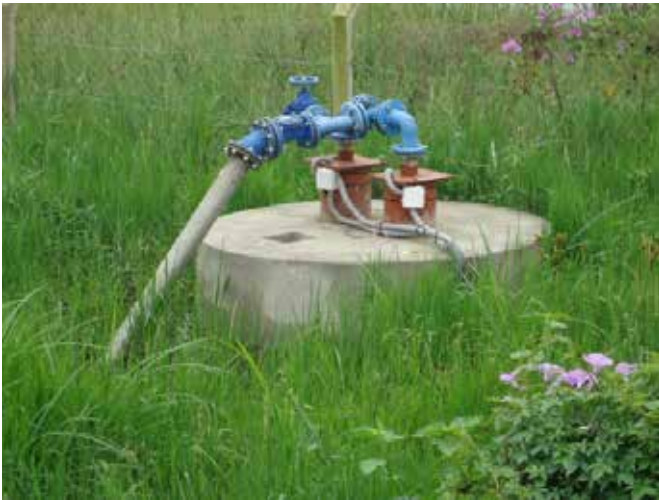
L-R: Production borehole; and surface pumps of Buyamba Water Supply System in Rakai District
