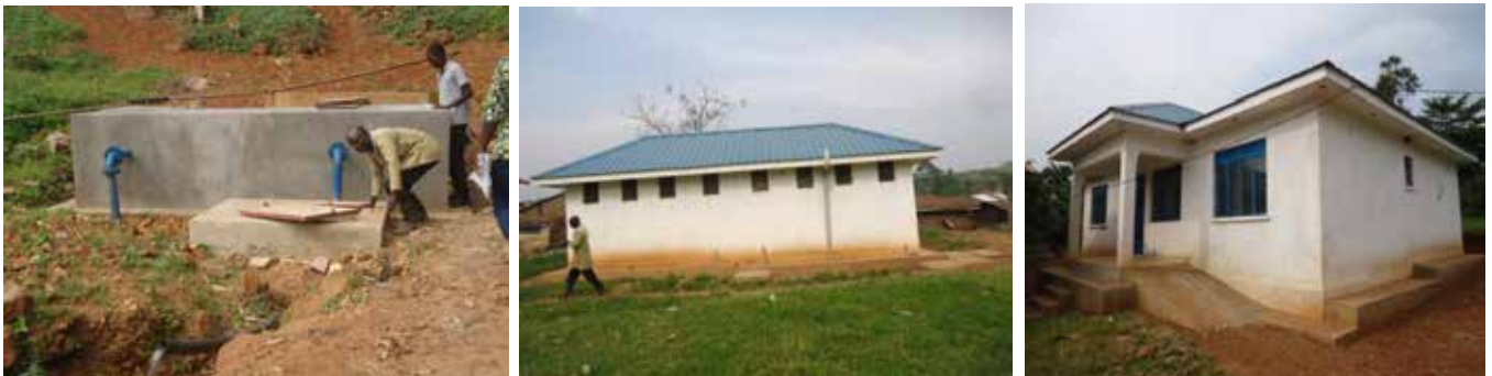
L: Collection tank at the spring source; C: Public water borne toilet; and R: Water office of Lukalu-Kabasanda WSS in Butambala District
