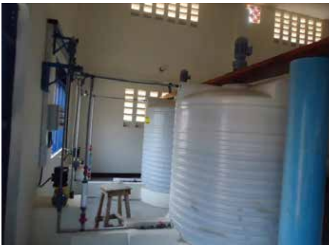
L: Chlorine dosing unit at the treatment plant; and R: A service connection at Kanara Town Council
