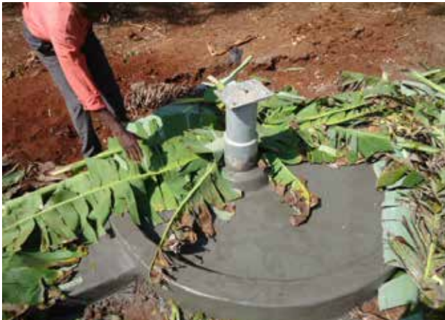
Borehole casting after drilling at Khabutola and Naukhaya villages in Manafwa District
