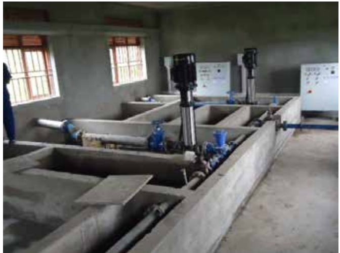
L-R: Production borehole; and surface pumps of Buyamba Water Supply System in Rakai District
