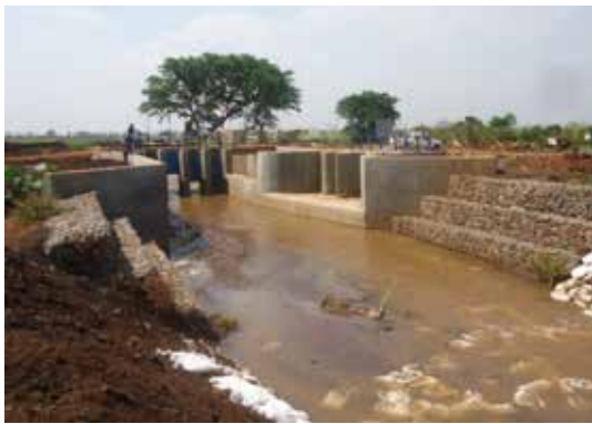
L-R: Headworks on R. Ngenge; and Cross head regulator of Ngenge Irrigation Scheme in Kween District
