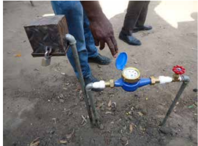
L: Chlorine dosing unit at the treatment plant; and R: A service connection at Kanara Town Council
