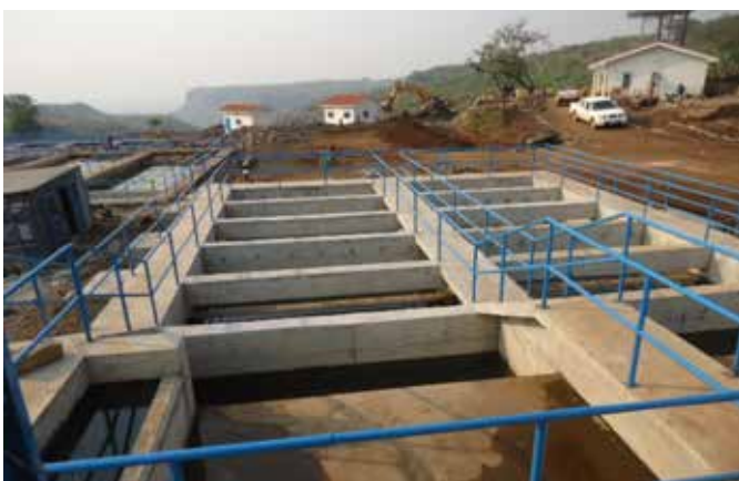
L: Flocculator/Clarifier; R: Rapid sand filter at the treatment plant of Bukedea WSS in Kapchorwa District
