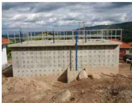
L: An Aerator; C: Rapid sand filter; and R: 500m 3 main reservoir tank of Shuuku-Matsyoro GFS in Sheema District
