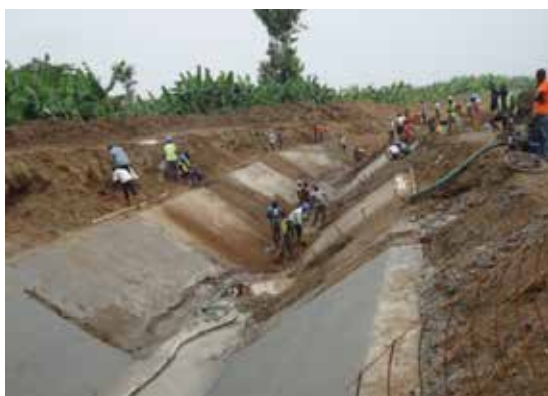
L-R: A section of the main canal under construction; and a cross head regulator of Doho II Irrigation Scheme in Butaleja District
