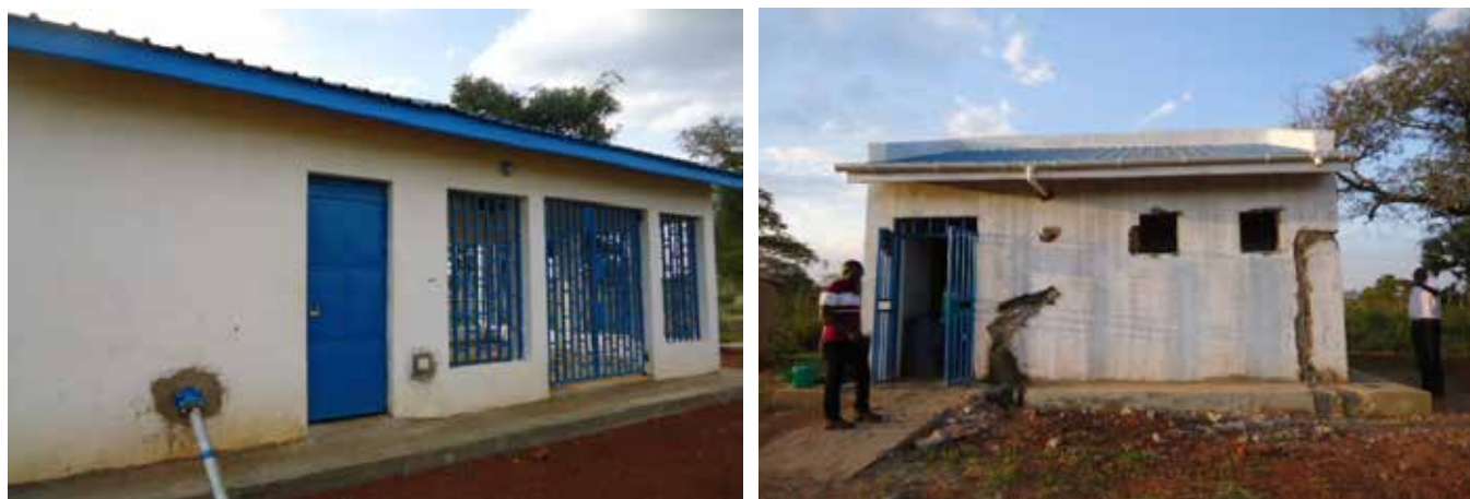
L-R: Pump house and generator house; VIP latrine of Agago Town Council Water Supply System in Agago District
