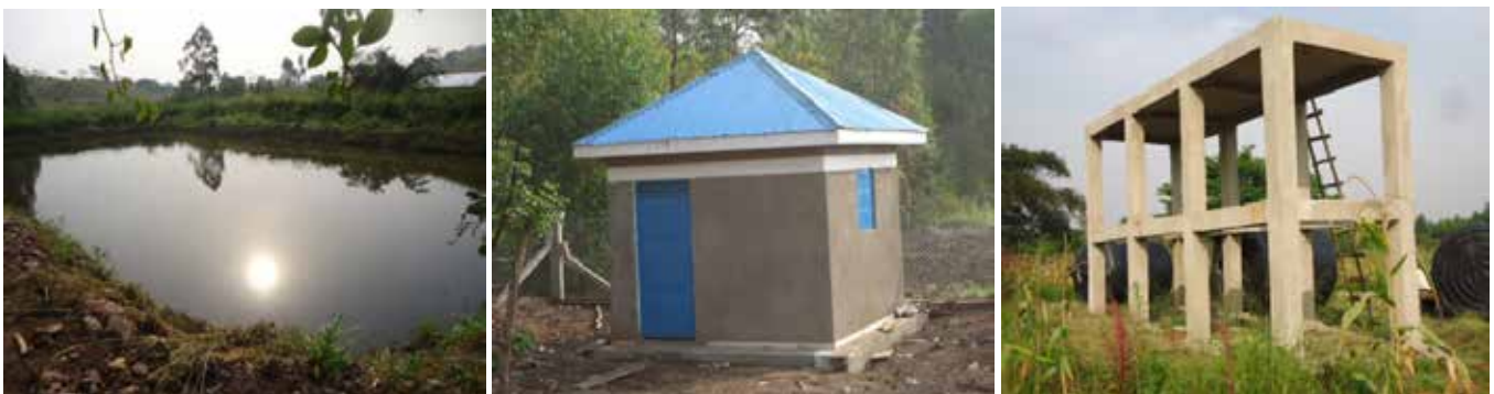
L-R: Valley tank for water source; Pump house; and reservoir tank stands of Kyakayondo Small Scale Irrigation Scheme in Kasanda District
