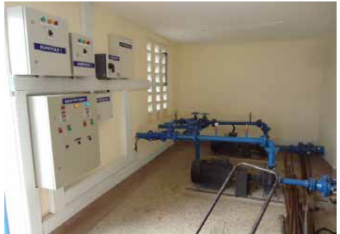
L-R: The water office; and pumps and pump control units of Kiwoko-Butalangu Water Supply System in Nakaseke District
