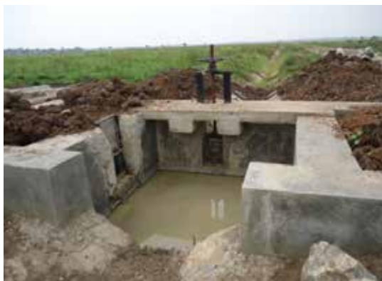
L-R: A section of the main canal under construction; and a cross head regulator of Doho II Irrigation Scheme in Butaleja District
