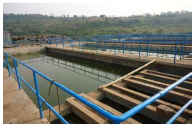
L: Flocculator/Clarifier; R: Rapid sand filter at the treatment plant of Bukedea WSS in Kapchorwa District
