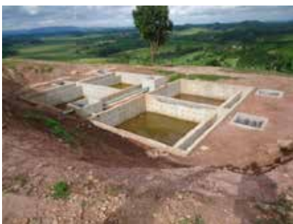
L: Sludge drying beds; C: VIP toilet; and R: Power extension to the treatment plant of Shuuku-Matsyoro GFS in Sheema District
