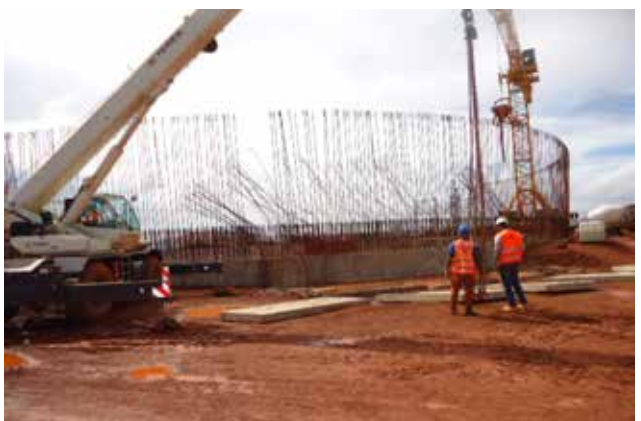
L-R: Staff houses; and casting wall for one of the Nsumba reservoir tanks of the Katosi-Kampala water treatment plant in Mukono District
