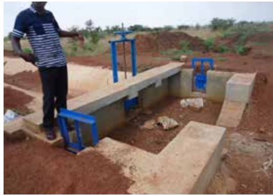
L-R: Headworks on R. Ngenge; and Cross head regulator of Ngenge Irrigation Scheme in Kween District
