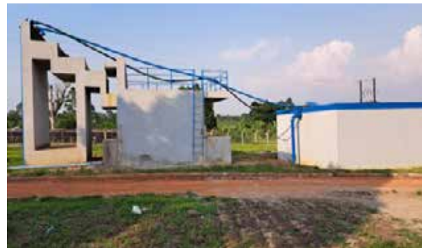
L-R: Water pipes bypassing treatment to the sump at Kyenjaju Station; Leakages on the installed pipes at Luswiga Pump Station 2 for Kagadi WSS in Kagadi District
