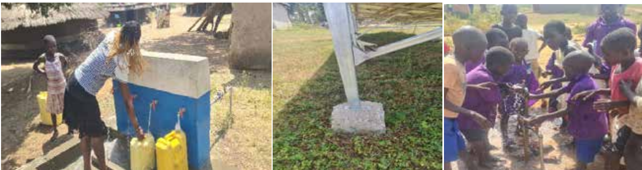
Institutional tap at Bulumba P/S in Kibuku, Eroded solar base of Budumba WSS in Butaleja District; and a PSP of Mutir WSS in Packwach District
