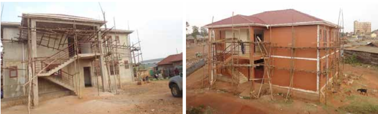
L-R: Staff houses and laboratory at Busia Port Health Facility
