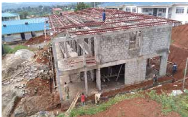
Ongoing works at the MCH building at Gombe
