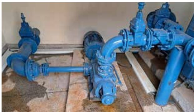
L-R: Water pipes bypassing treatment to the sump at Kyenjaju Station; Leakages on the installed pipes at Luswiga Pump Station 2 for Kagadi WSS in Kagadi District
