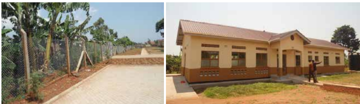
L-R: Completed maternity ward and external works at Malongo HCIII Mayuge District
