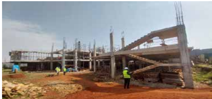
Ongoing construction of the UBTEB Assessment Center at Kyambogo in Kampala
