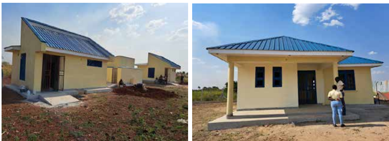
L-R: Lacekocot water office, and three toilets for pupils (male and female) and teachers at Lawiyeadul Primary School, Pader District
