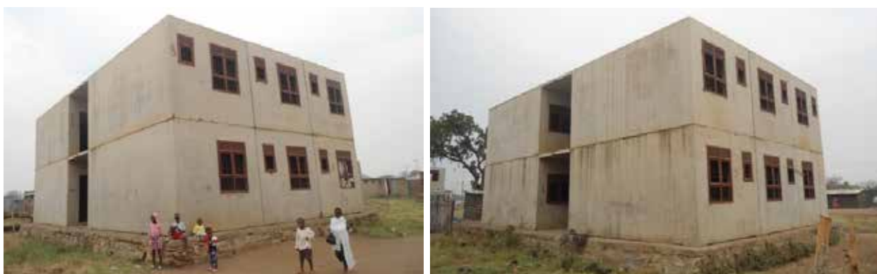
Prefabricated units installed for the staff house and laboratory at Elegu Port Health
