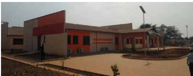
Substantially completed structure of the northern oncology center
