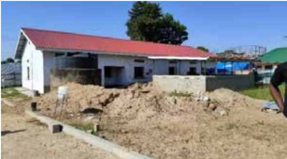
Ongoing renovation of OPD at Bukakata HCII under Lot 3
