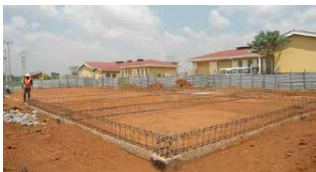
Left: Construction of a multi-purpose block at walling level, Right: Construction of a girls' dormitory at ground beam level at Basoga Nsadhu TI under OFID
