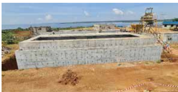
L-R: Intake structure (pumps and control rooms); Clarifier structure at the Water Treatment Plant in Busia district
