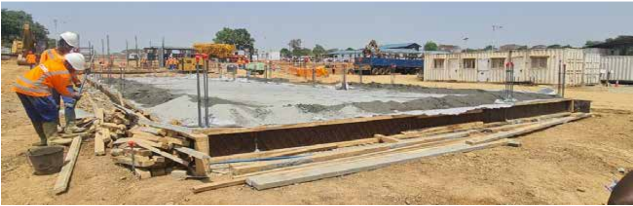
Ground floor concrete slab of administration and control room
