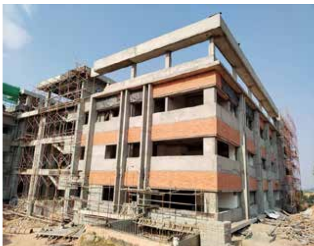
Progress of works at the multipurpose building-UCI
