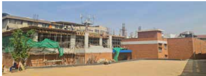
Ongoing works at the auxiliary building at the UCI Mulago
