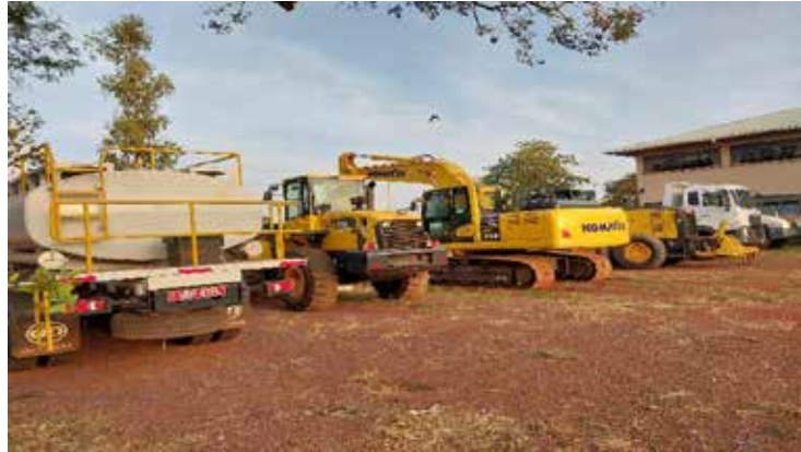
Assorted road construction equipment and plants at UTC-Lira
