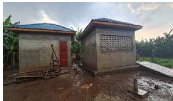
Second pumping station
