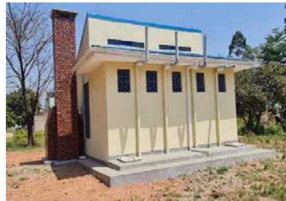
An institutional VIP girl's toilet at Mingoro P/S Ayivu Division, Arua City
