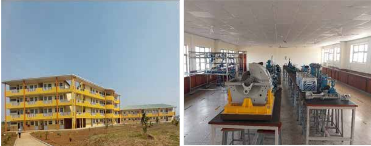
Left-Right: Newly constructed, furnished and equipped Multi-purpose block, and Down-stream Equipped Laboratory at UPIK
