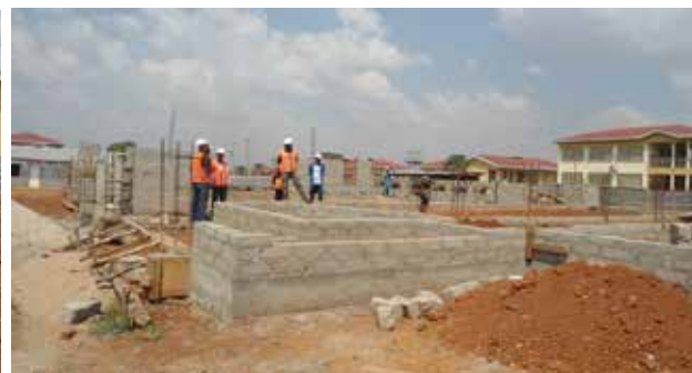
Left: Construction of a multi-purpose block at walling level, Right: Construction of a girls' dormitory at ground beam level at Basoga Nsadhu TI under OFID
