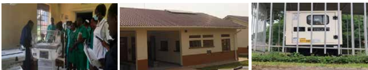
L-R: Generator installed at Kajjansi HCIV, solar panel and Namugongo HCIV and equipment at Maddu HCIV
