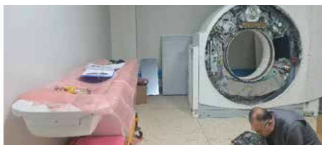
L-R: CT Simulator installation works; Delivered equipment awaiting installation
