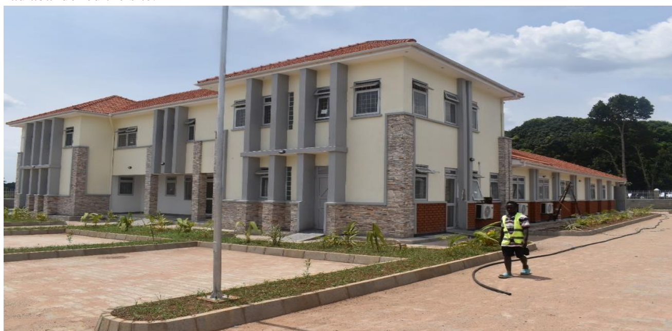
Substantially completed construction of Hoima Regional Blood Bank
