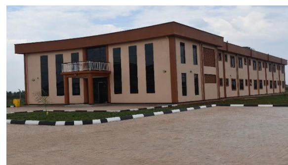
Complete medical intern residence at Lira University, Lira District
