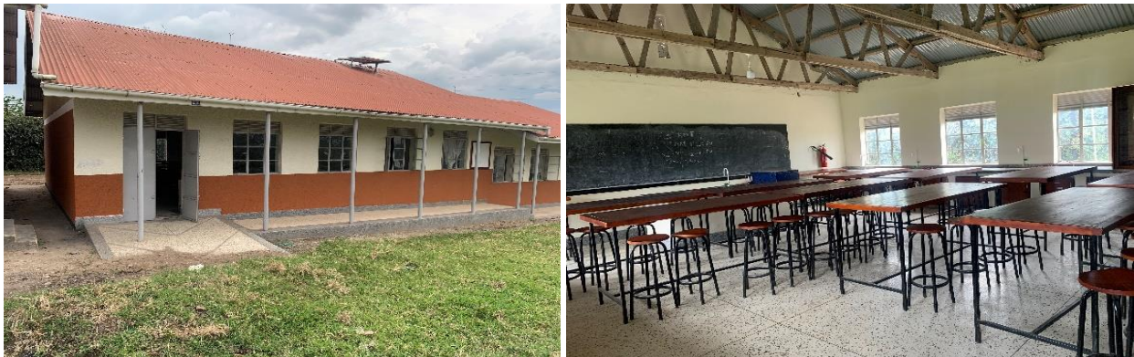
Left: A completed science laboratory block, right: Furniture inside the completed science laboratory block by the UPDF-Engineering Brigade, at Rwantsinga High School, Rubaya S/C, Mbarara District
