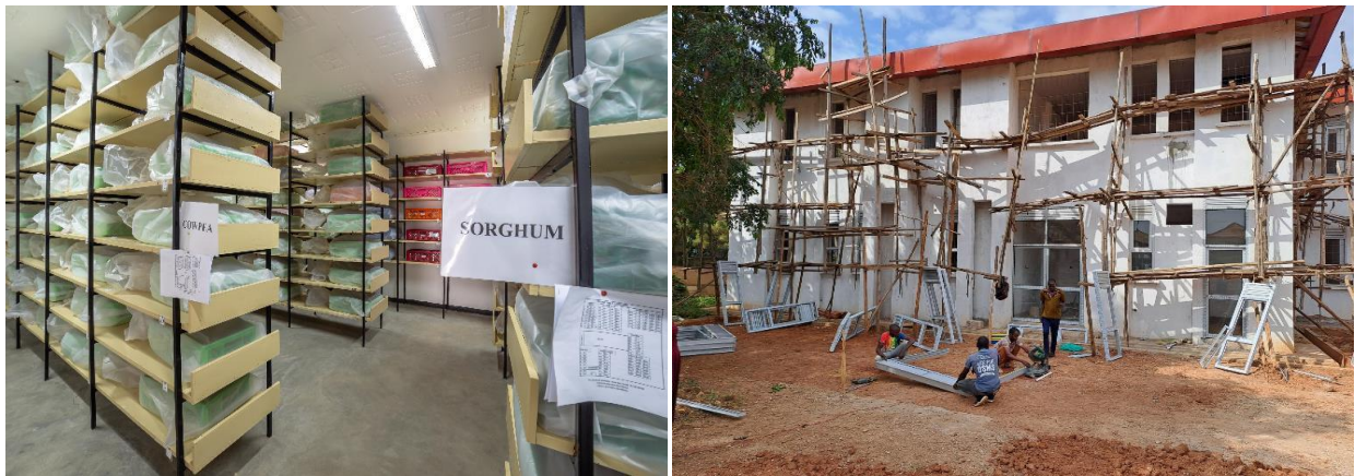
Left-Right: Gene Bank at MaRCCI: Germplasm conservation with over 7,000 local, regional and international accession of cowpea & sorghum; on-going construction of office block and classrooms at MaRCCI
