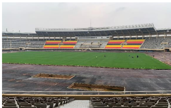
Ongoing renovation of Mandela National Sports Stadium
