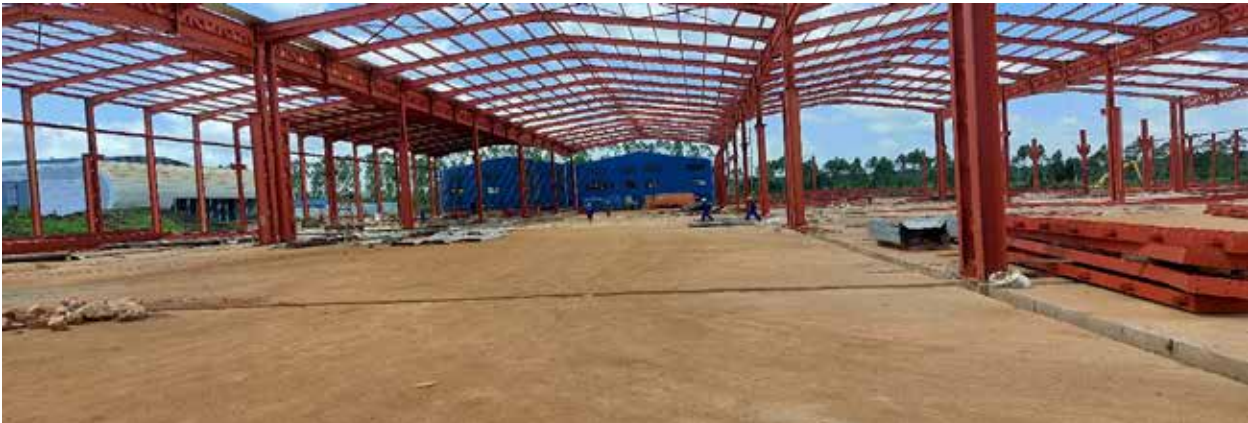
Ongoing construction of electro-coating shop at Kiira Vehicle Plant, Jinja
