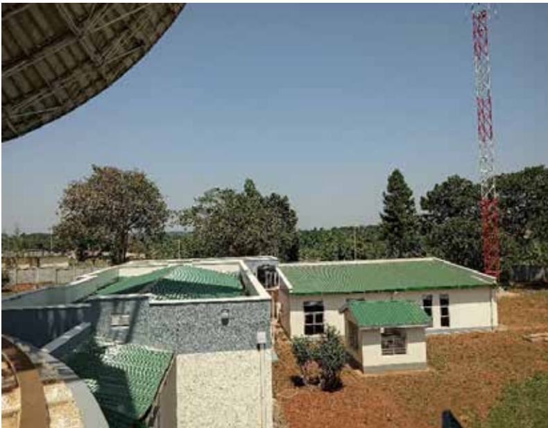
Renovated infrastructure at Mpooma Satellite Station
