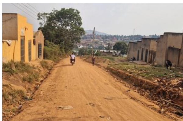
Mbarara City: A section of Lubiri-Kakoba Central Road after routine mechanized maintenance
