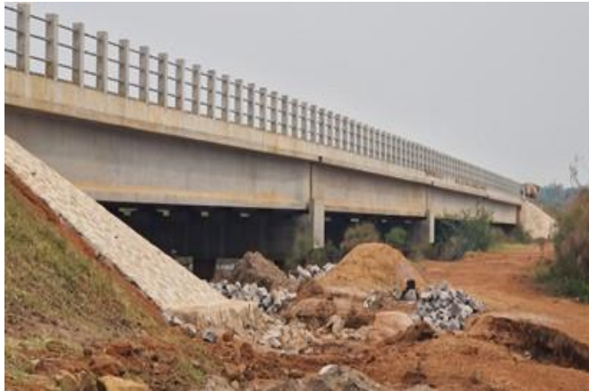
Completed Bridge at Lugogo Swamp Crossing in Nakasongola District
