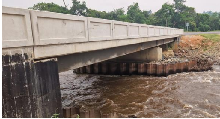
Ntungu Bridge constructed along Rukungiri-Kihihi Road
