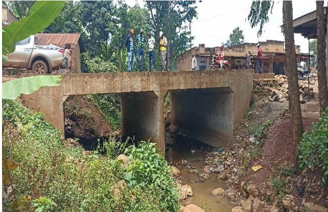
Completed Sahana bridge along the Kufu-Magale Road in Namisindwa District
