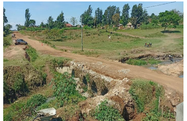
Ongoing Anderema Bridge works in Tororo District of a triple 4m by 4m, 3 cell box culvert: Left - the bridge structure works; Right: the diversion provided to keep the road accessible
