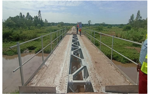
Rehabilitated Truss Bridge at Km 16+500 at Magodesi in Tororo District
