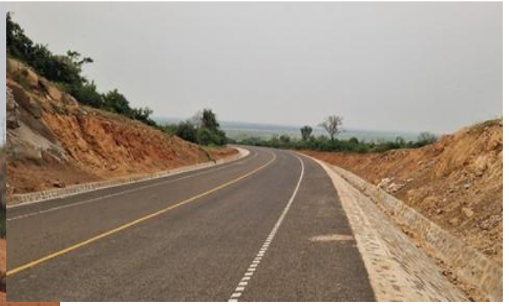
Tarmaked approach road section at Lugogo Swamp crossing in Nakasongola District
