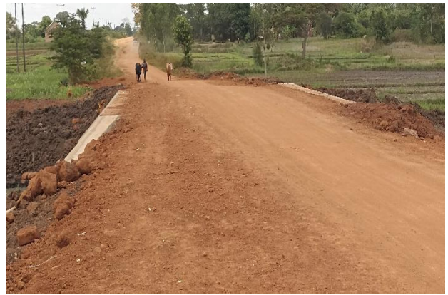
Substantially complete restoration of the Kaboloi bridge in Pallisa District along the Pliisa-Agule Road at Km 8+000 from Pallisa with 4 cells of 2.1m diameter armco culverts
