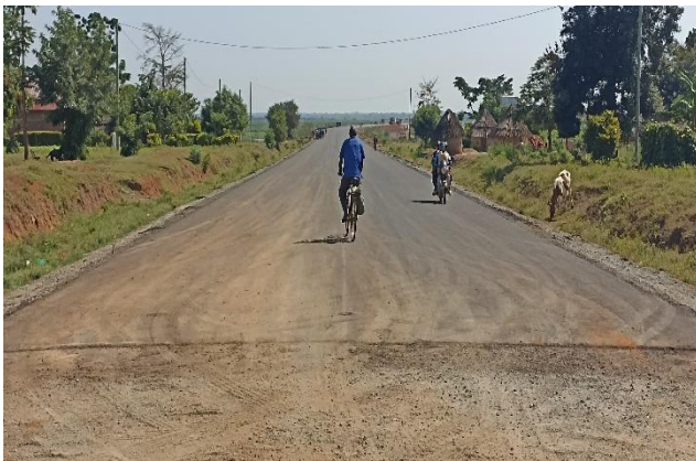
An asphalt paved approach road from Kaliro District side for the Saaka Swamp Crossing
