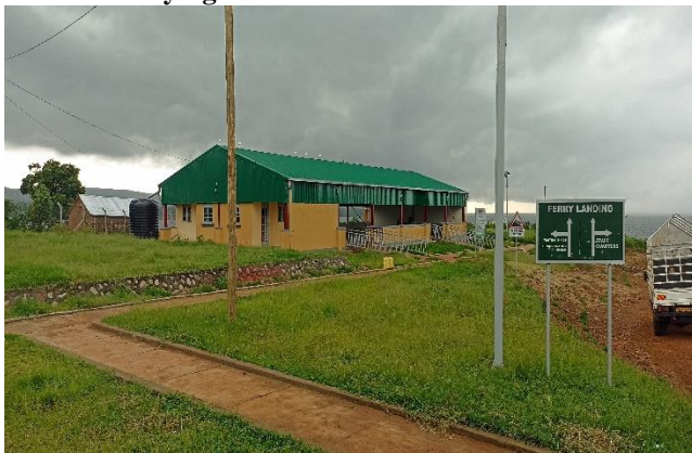
Completed passenger waiting shed at Watega Landing Site in Namayingo District
