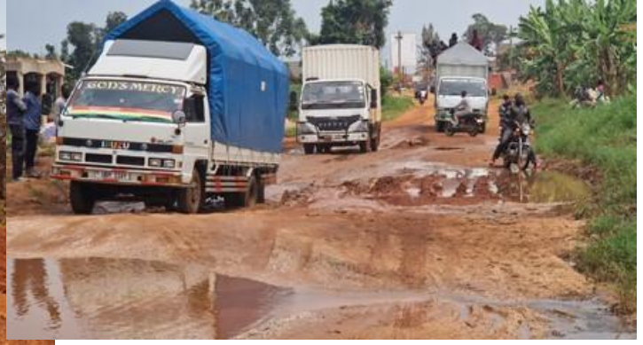
Luwero Station: Kisule-Nakaseke-Kapeeka Road had greatly deteriorated due to the heavy rains in Q1 and Q2
