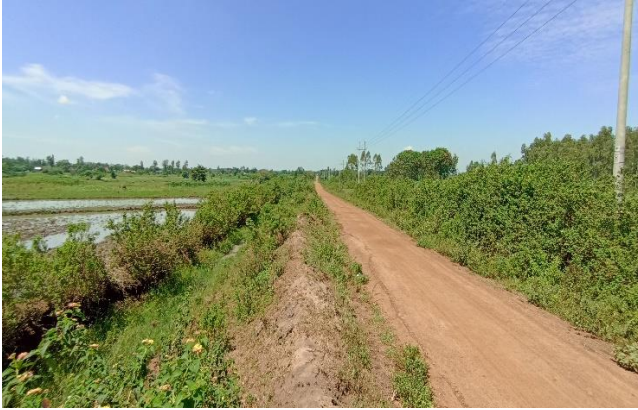
Merikit Nyem Nyem Swamp Crossing in Tororo District: Left - A raised section with a mitre drain; Right – A river-trained section that has been encroached on by the rice growers
