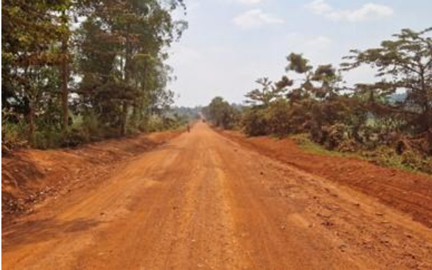
Luwero Station: Kapeeka-Busunju (15km) after mechanised maintenance under a framework contract
