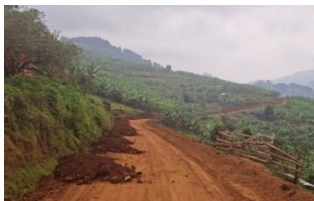
Rukungiri District: Graveling works
