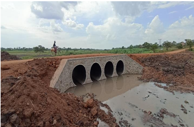
Substantially complete restoration of the Kaboloi bridge in Pallisa District along the Pliisa-Agule Road at Km 8+000 from Pallisa with 4 cells of 2.1m diameter armco culverts
