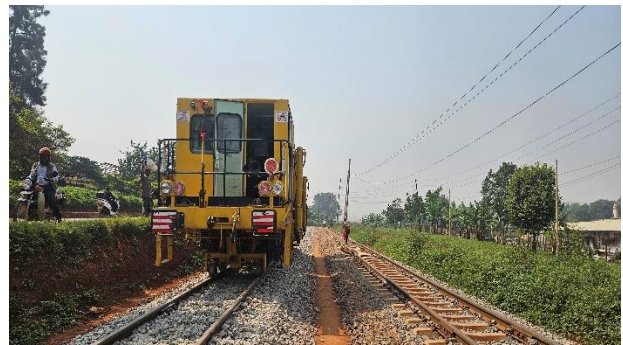
Tamping of ballast ongoing using the tamping machine
