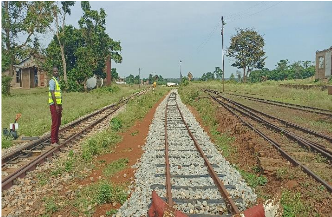
Completed railway track at Km 0 at the Tororo Railway Station
