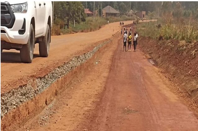
A section undergoing benching at Km 60+000 along Olwiyo-Packwach Road
