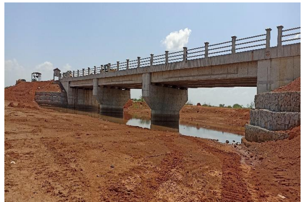
The completed bridge structure at Saaka Swamp Crossing
