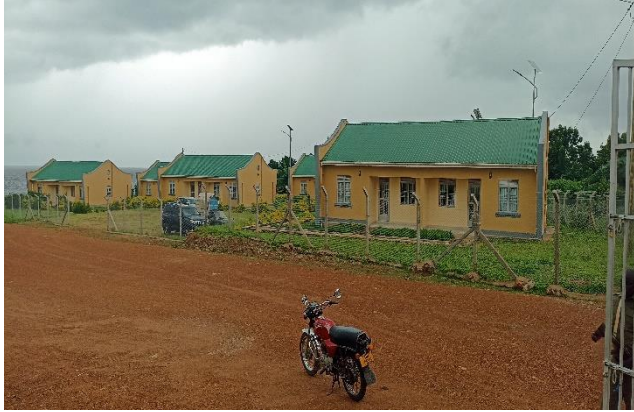
Completed twin unit staff houses at Watega Landing Site in Namayingo District
