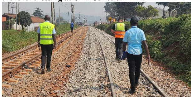
Completed track awaiting ballast tamping
