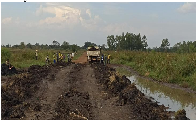
Aleles-Kodike Swamp Crossing in Ngora District: Ongoing swamp-raising works (left) and a completed raised section (right)
