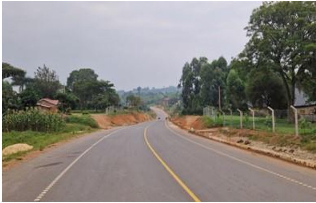
A completed section of Rukungiri-Kihihi-Ishasha Road
