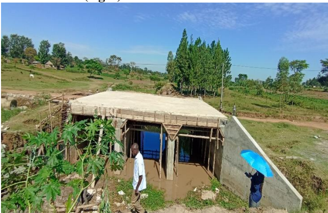
Ongoing Anderema Bridge works in Tororo District of a triple 4m by 4m, 3 cell box culvert: Left - the bridge structure works; Right: the diversion provided to keep the road accessible
