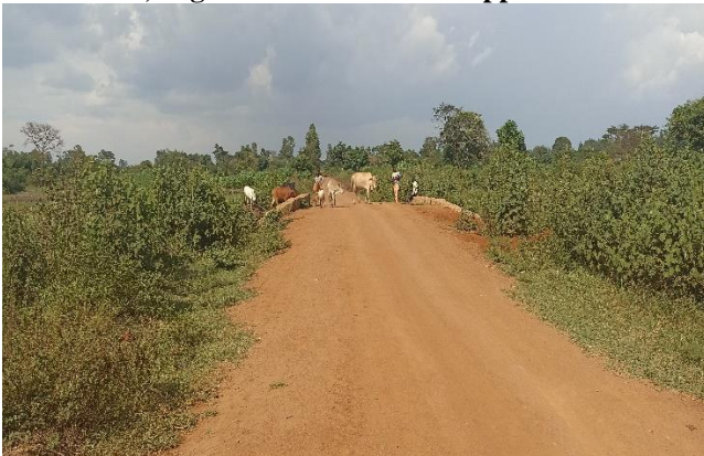
Matawa Swamp Crossing in Tororo District with four swamp crossings: Left – Second swamp crossing at Km 7+900, raised and with culverts installed; Right – Fourth swamp crossing at Km 11+700
