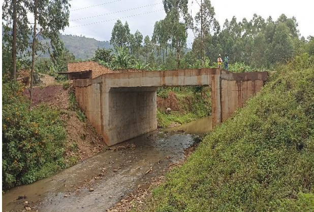
Completed 10m span Nabukuya bridge structure along the Kufu-Magale road in Namisindwa District
