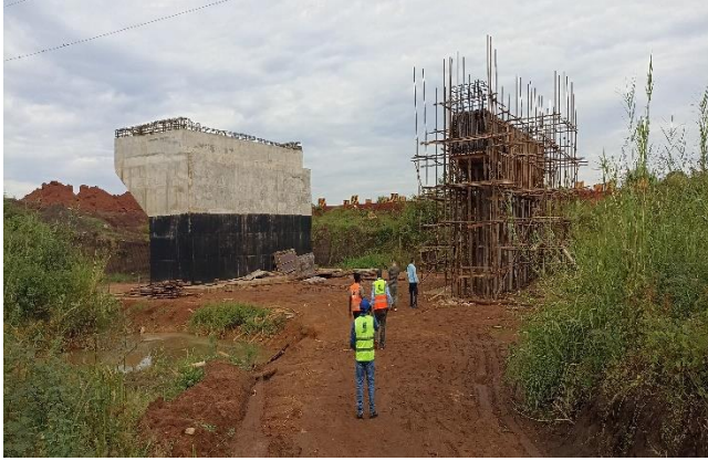
Ongoing River Malaba bridge works at Km 14+320 along the Busia-Malabo Road
