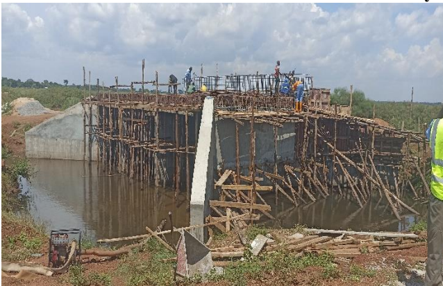
Funguwe-Muwafu Swamp Crossing in Tororo District: Left – Ongoing rebar works for decking of the 3-cell box culvert; Right – A raised section/approach to the box culvert with culverts installed
