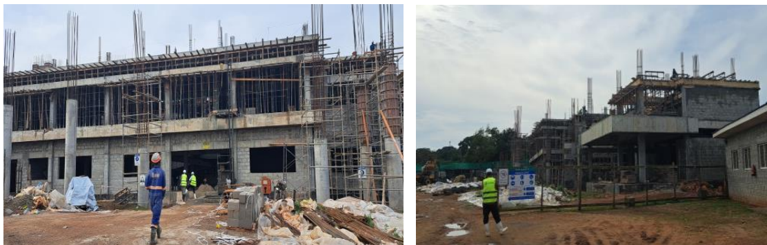
Ongoing construction works at National Water Quality Reference Laboratory in Entebbe
