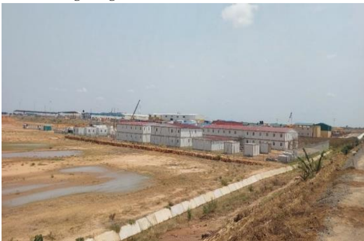
Works at the temporary worker's camp in Buliisa
