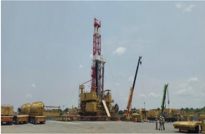
Well drilling at Ngiri 1 Well Pad in Buliisa
