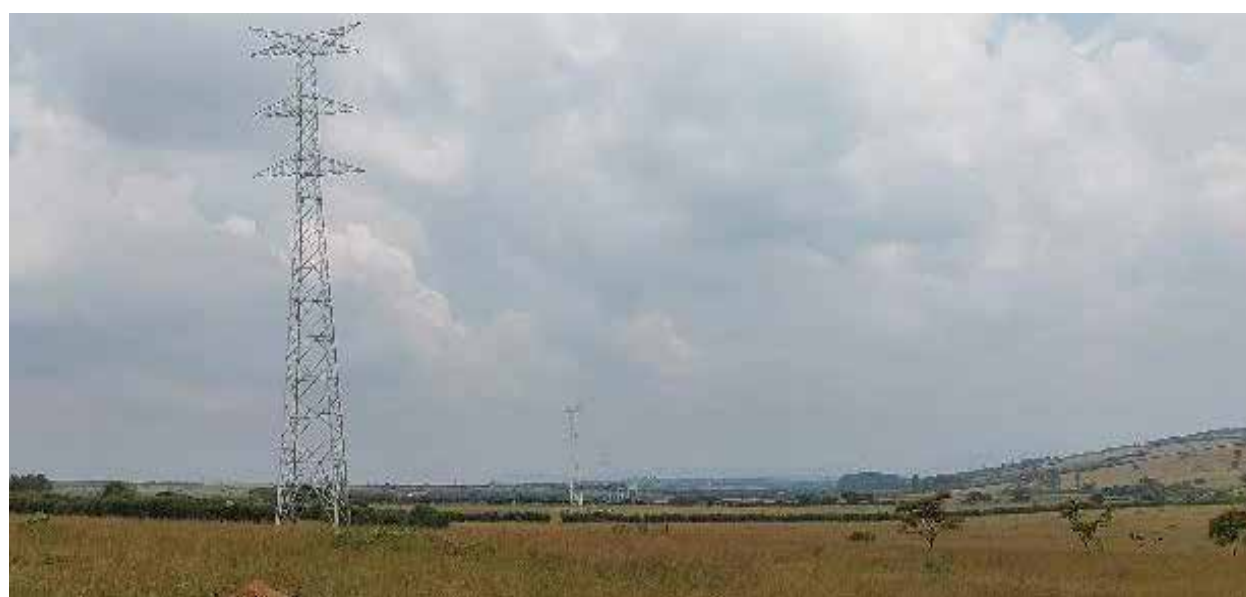
Completed towers on the Mirama-Kabale Transmission Line in Mirama, Ntungamo
