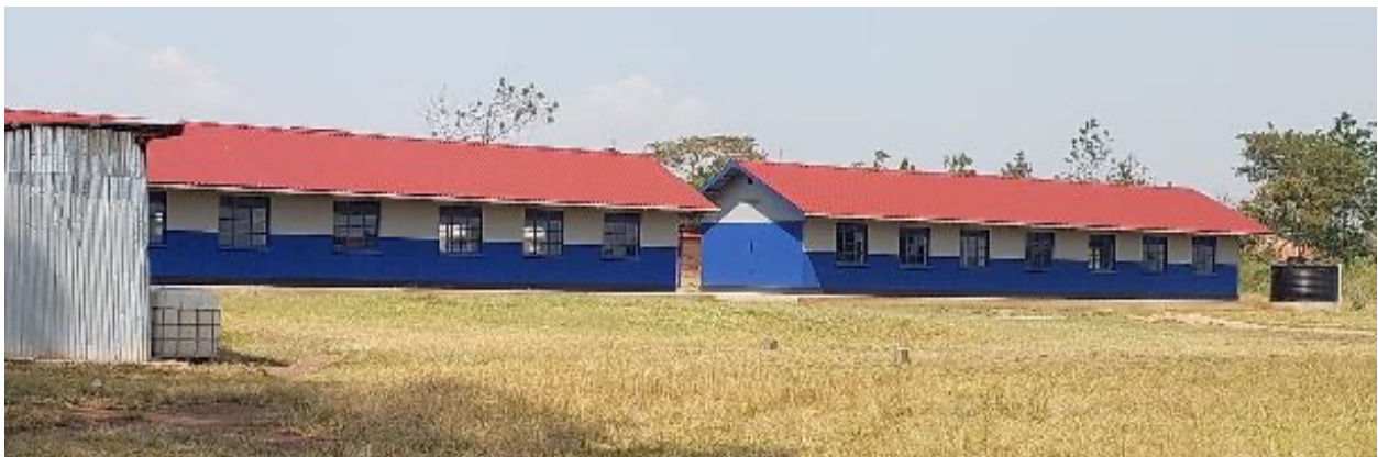
Completed double classroom blocks at Nora Primary School, Oyam District under the Karuma HPP CDAP
