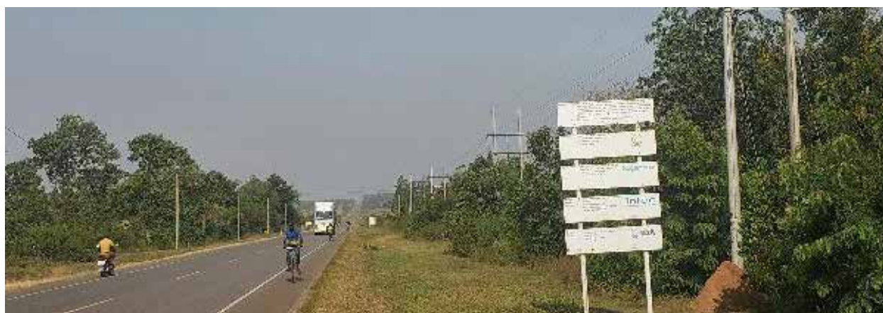
Completed grid extension scheme (Line 21) under ERT III on the Dokolo-Soroti road in Kalaki
