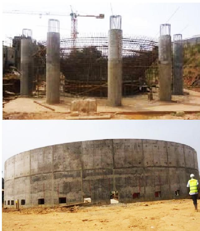
Up - Down: Reinforcement bars and columns of the sludge digester; Trickling filter at Bugolobi for the NWWTP in Kampala district
