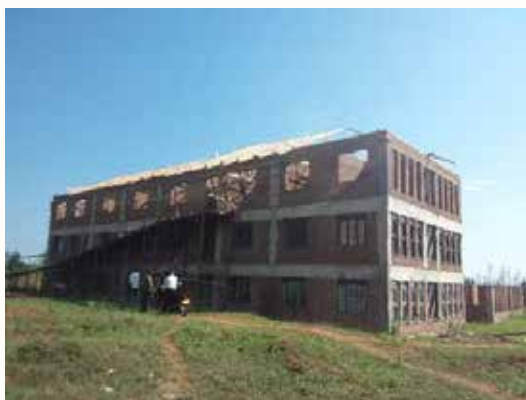
Construction (new) office block
