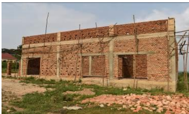
Sub-structure for the warehouse in Ibanda District
