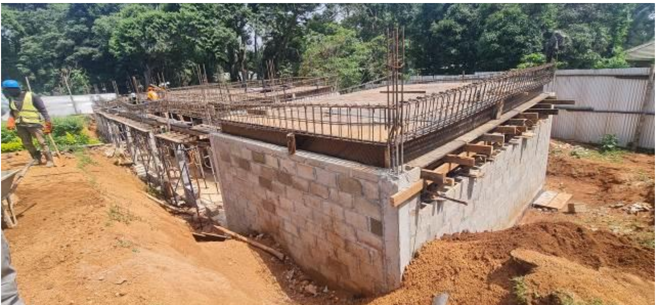
Ongoing construction of the Animal Hospital at UWEC Entebbe
