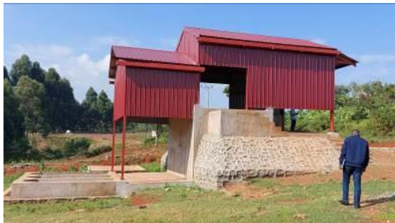
Incomplete coffee washing station at coffee World site in Kween District
