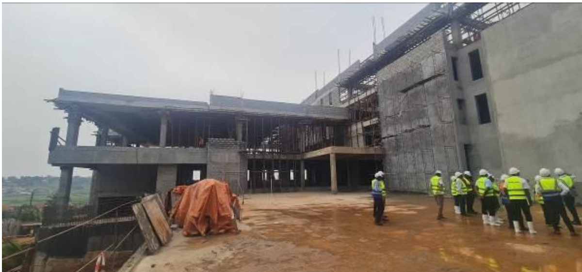
Construction of the BDS superstructure in Butabika
