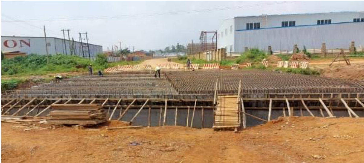
Box culvert construction in South A Estate of KIBP across Namanve River
