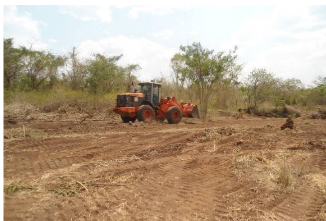
Bush clearing was ongoing at AMFRI FARM in Nakaseke district
