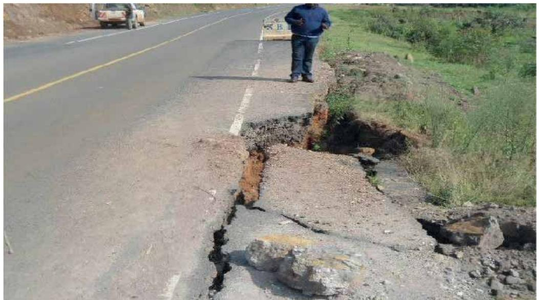
*A section of Kabale- Kisoro road that flaked off after completion of works. This was attributed to the inadequate design tolerances that were adopted.*
