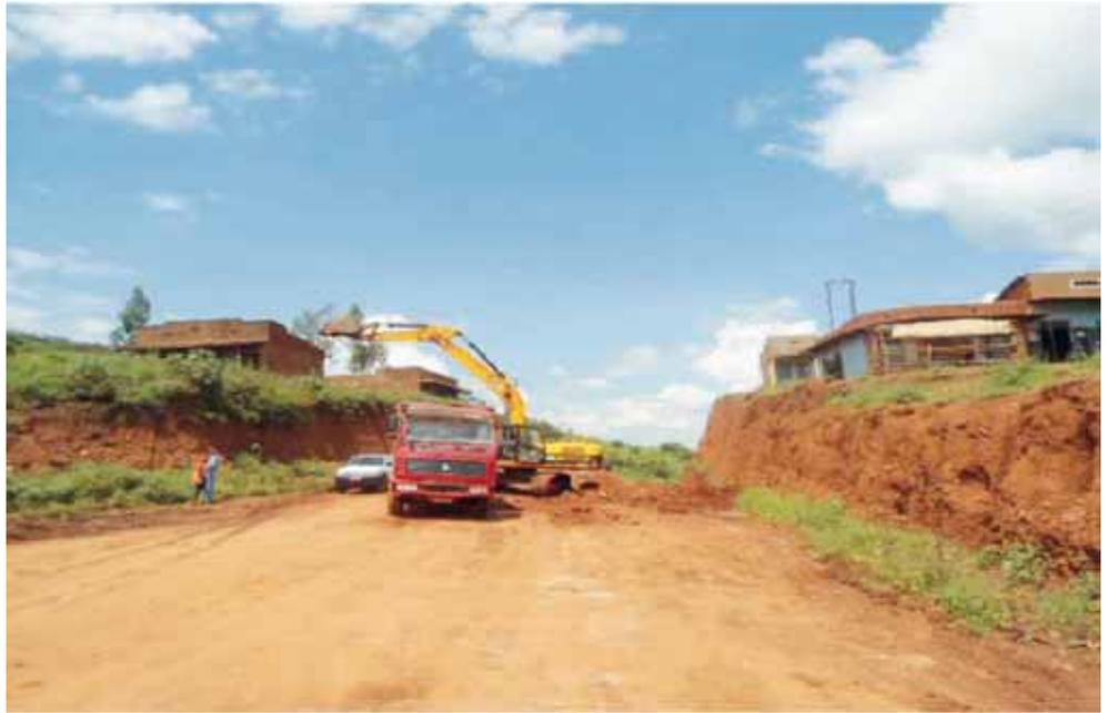
*A section of Ishaka-Kagamba road where the specified road width could not be achieved because of land compensation issues on top of the embankment.*
