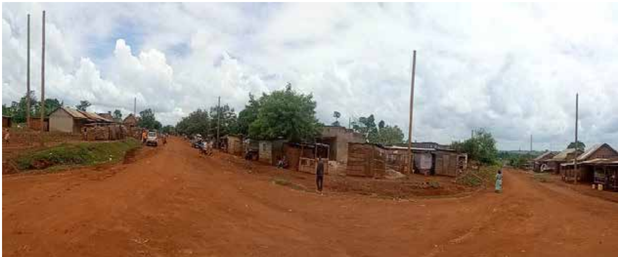
Pole erection works at Bumana trading center, Luuka District
