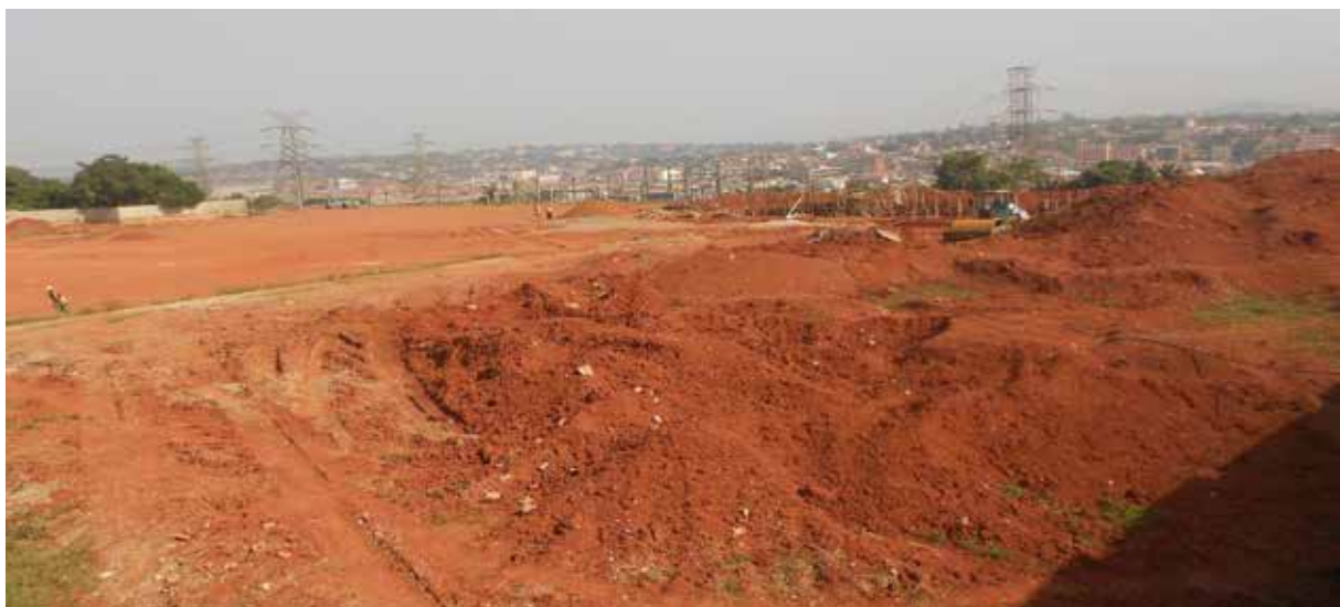
On-going earth works and exaction works at the Mutundwe substation site
