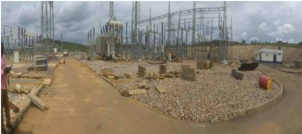
Ongoing Works at Mirama Hills Substation
