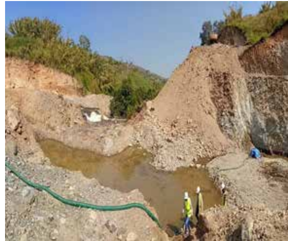
L-R: Completed river diversion channel; On-going dam foundation excavation works
