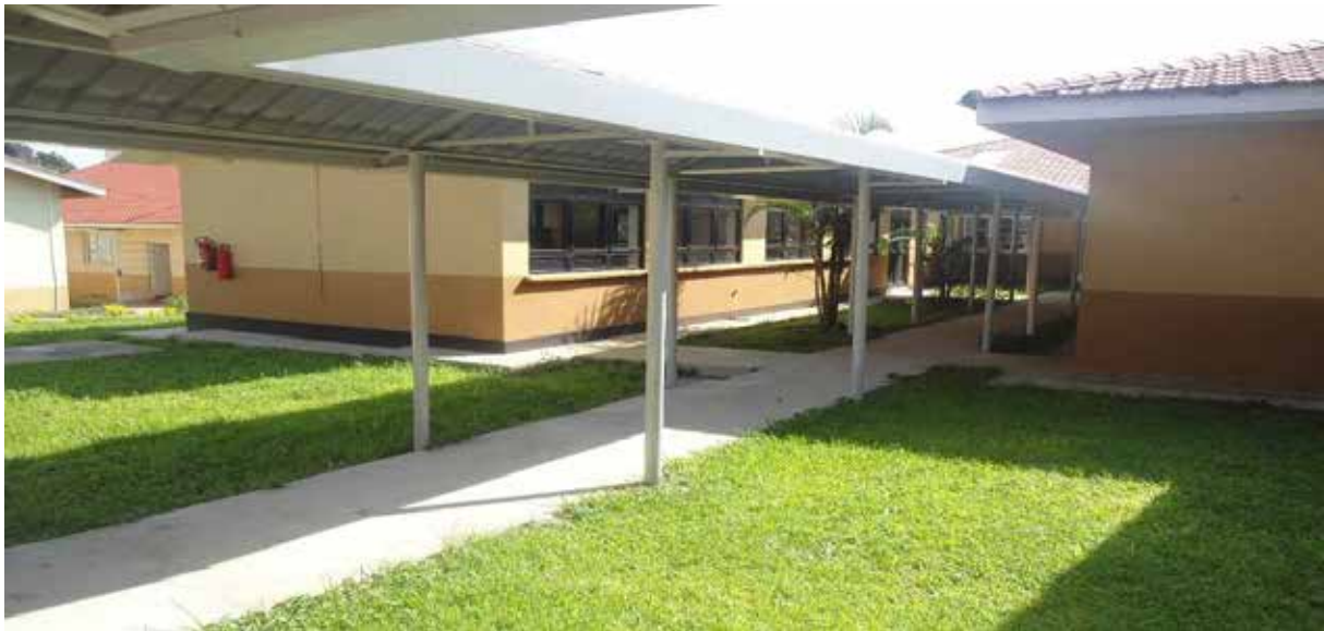
Newly renovated laboratory building to house some of the new laboratory equipment
