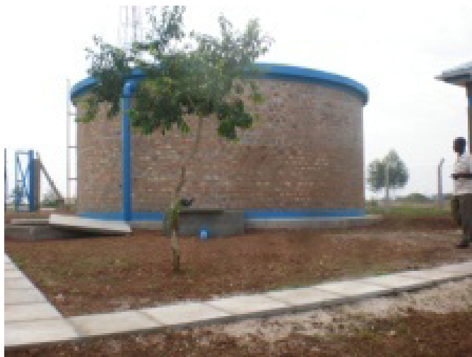
A reservoir tank for Nkoni water supply system constructed on land donated by Buganda Kingdom
