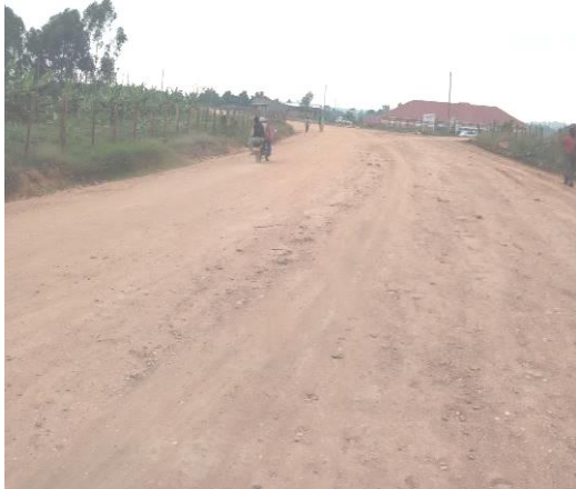
A section of Nyakashambya-Sheema Headquarters Road
