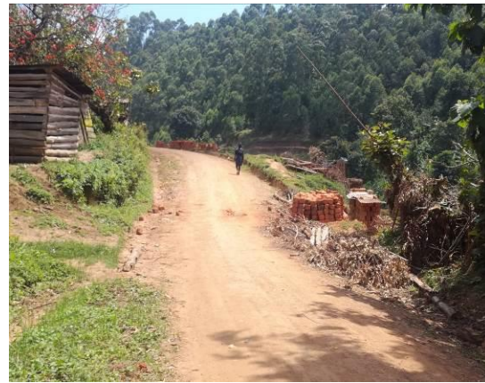
A section of Mwaro-Busenge-Kinawara (17km) where bricks and felled logs are obstructing the road side drain at Km 0+900
