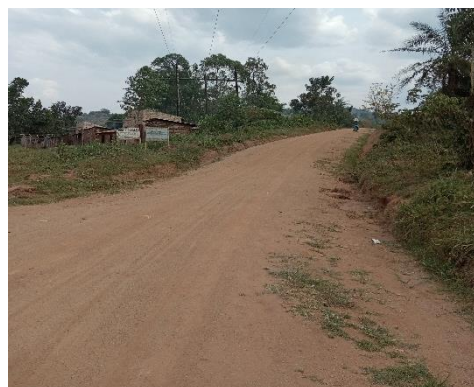
A section of Nalweyo-Kigwerige-Kiryamasasa road at km 0+000
