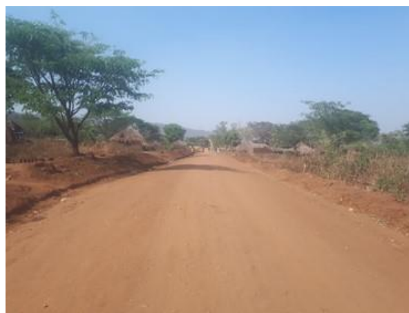
Padel-Pangere Road (12.5km) was in good condition after RMeM carried out in Q2
