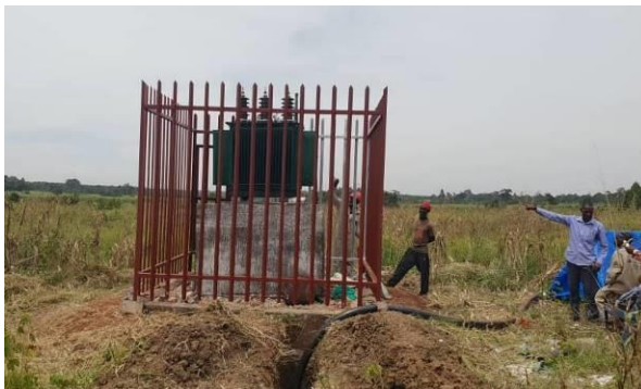
Mounted transformer and ongoing site opening at KMC-Jinja
