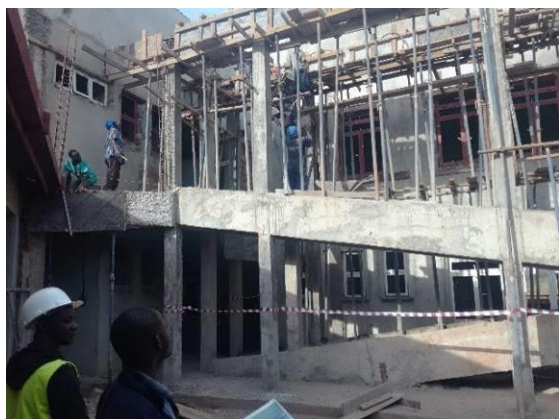
Construction works on the ramp at the Katuna OSBP – Phase 1 works
