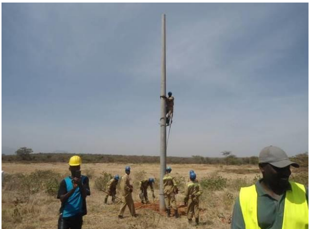
L-R: Ongoing erection of concrete poles in Lorengdwat-Moroto under IDB I funding, Grid extension
