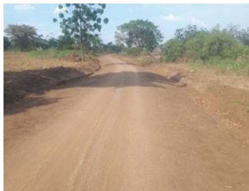
Petete-Kachooha-Radio Road (6.8km) worked on under RMeM
