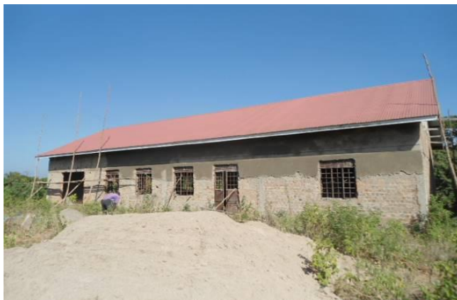
Civil works on all structures at Bamunanika Technical Institute resumed after 2 years' stallment. Plastering was ongoing on a 2 classroom block and a workshop block
