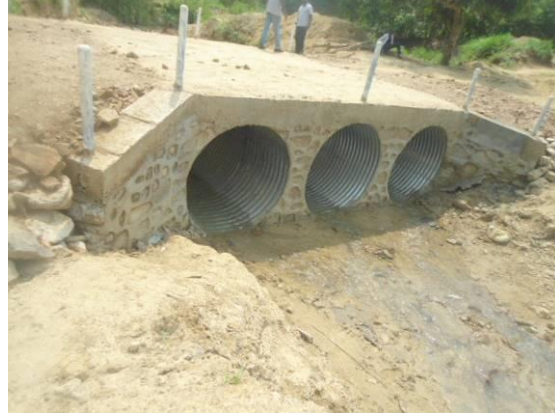
A bridge drift along Hakitenngya-Buhamba Road at 3+500
