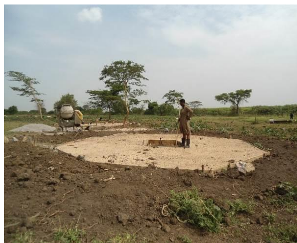
Foundation of water trough constructed at Maruzi Ranch in Apac District
