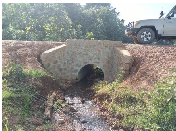
A culvert at Km 13+000 on Masaka-Kidda-Lusakalwamese
