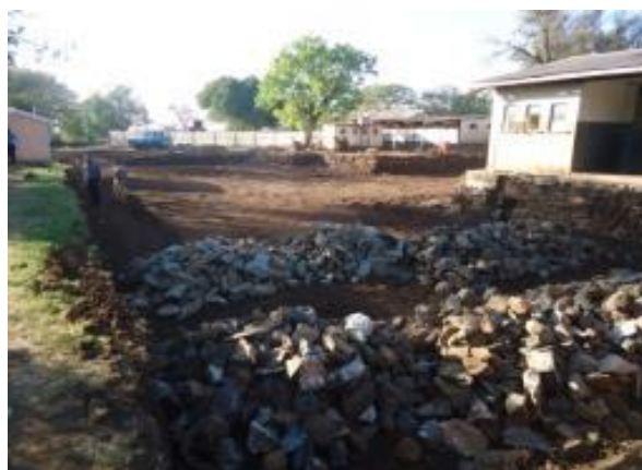
L-R: Staff quarters under construction and excavated foundation for the maternity ward
