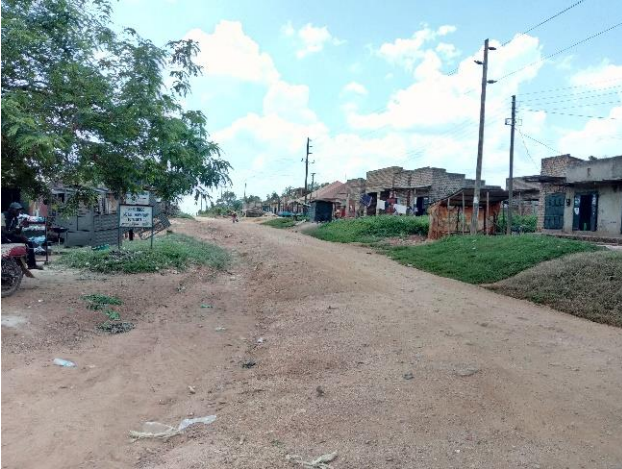
A section of Mawale-Danza-Kakiri Road at 0+000 from Mawale
