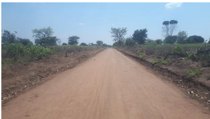
A graded section of Komolo-Aberilela-Eloroberito-Akoromit Road (18km)
