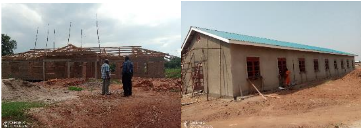
L-R: Construction of administration block at Jinja PTC in Jinja District at roofing stage; Construction of boys Dormitory at Kitgum Core PTC, in Kitgum District at finishes level
