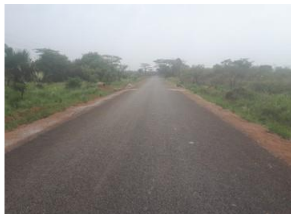
Low cost sealing of 1.5km along Alenga-Kungu road
