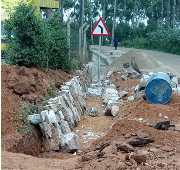
Stone pitching works along State Lodge road
