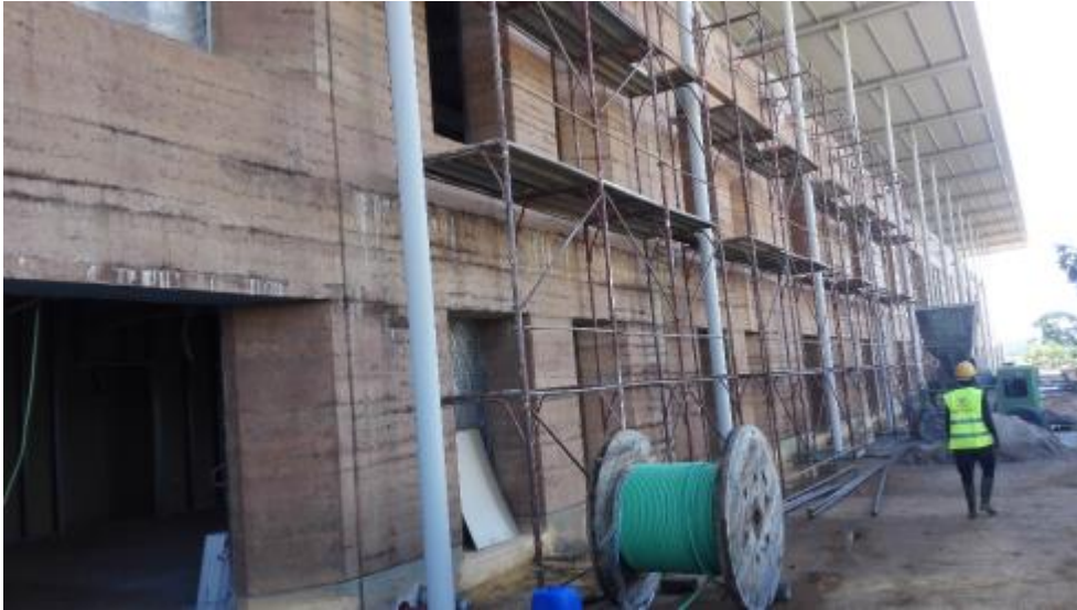
Ongoing works at the Regional Pediatric Surgery Hospital in Entebbe
