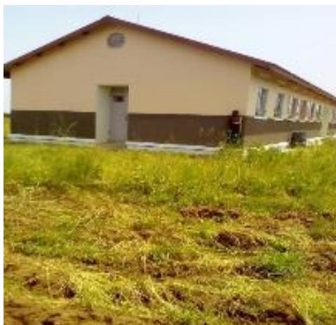
Completed Girls' dormitory at Lolachat Primary School in Nakapiripirit district as at January 2019
