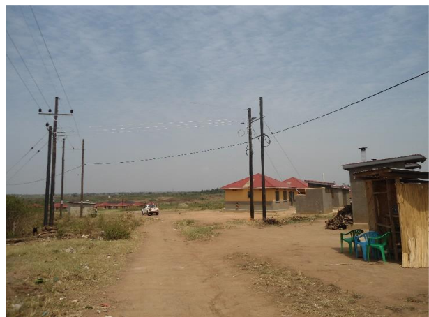
L-R: Ongoing erection of concrete poles in Lorengdwat-Moroto under IDB I funding, Grid extension
