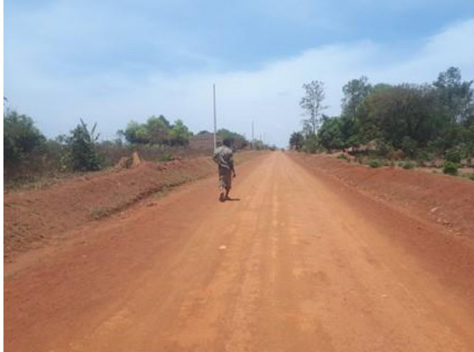
Agweng-Aromo Road (18km) after Routine mechanized maintenance in Q2 FY 2018/19
