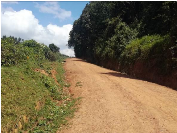
A well compacted section of Kanaba-Kateriteri-Kabahunde road (16km) at km 5+500
