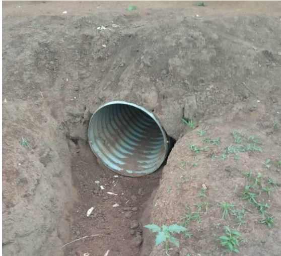
A culvert installed on Nyakashamba Ryamuhunga Road at 0+800
