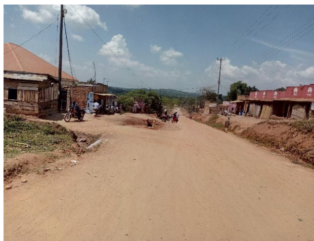
A section of Bombo-Ndejje-Kaalsa road at 0+000
