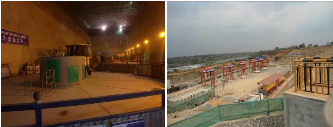
L-R: Electromechanical works in the power house showing a partially completed generator unit, Ongoing works at the power intake
