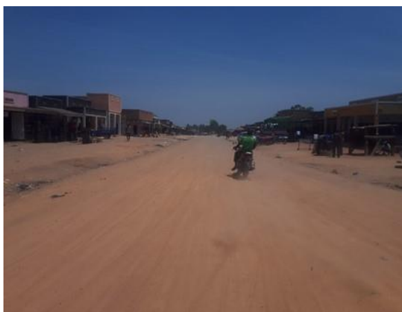
A graded section of Odramacaku-Aroi road (115.4km) at Odramacaku town
