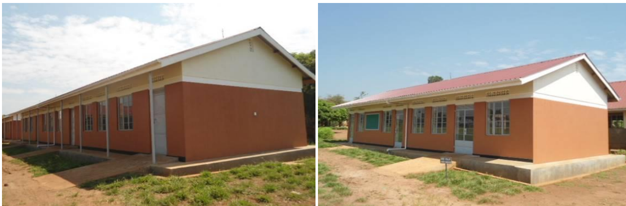
Completed classroom blocks at Bwetyaba UMEA P/S under UTSEP project in Butambala District
