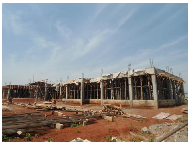
Civil works on the two storied male dormitory at 50% progress at UPIK
