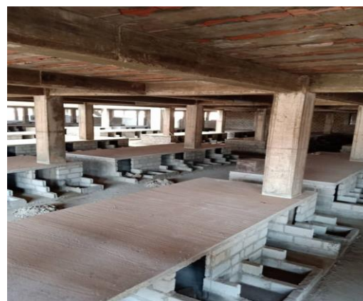
Produce stalls under construction in Busega Market as at February 2019
