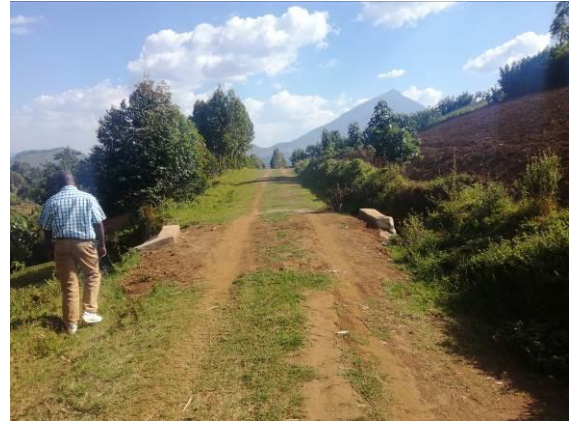
A culvert with end structures on Nyagashinge road (2.3km) at Km 1+800
