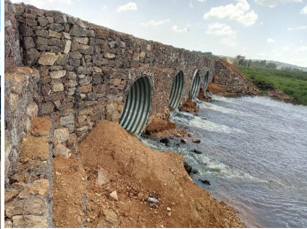
Emergency works of swamp raising along Mawale-Danza-Kakiri Road at 13+800 from Mawale
