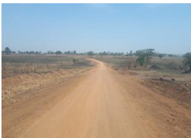
A gravelled section of Palemoderi-Ciforo road (8km) at Km 4+700 during RMeM
