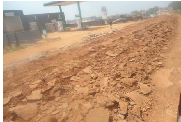
Road bed preparation works on Kampala road in Mityana Municipality
