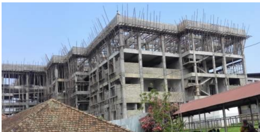
Ongoing works at the Maternity and Children Ward Complex, Masaka RRH
