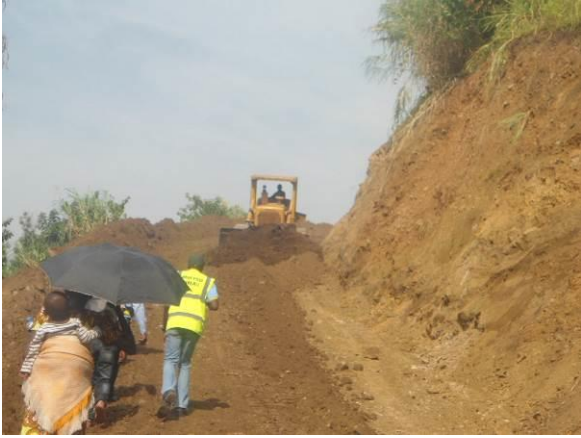
Road opening works on Harugale-Bumpumpoli Road
