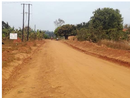
Kyamulibwa-Kinoni-Lusango (15km): A well graded but dusty section at Km 0+000
