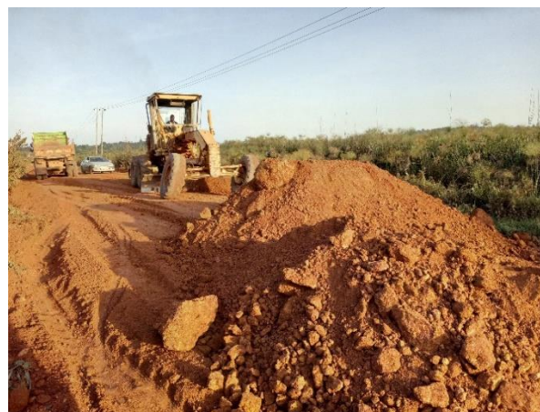
Swamp raising works at Km 12+400 along A section of Kyabakuza-Kiwangala-Ndagwe-Kabale at 13+000
