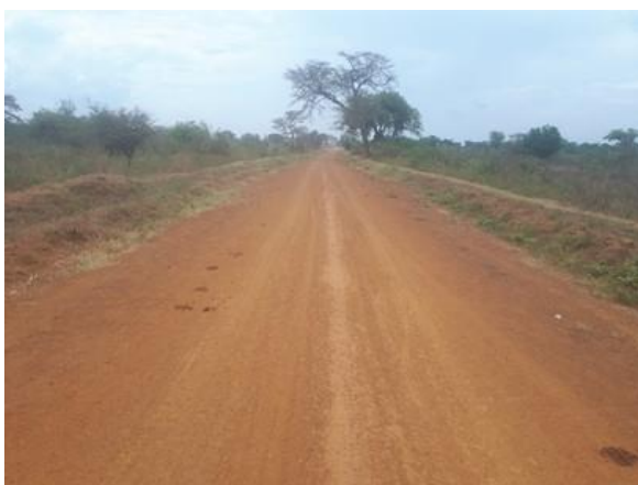
Serere-Kateta-Kyere Road (27.3km) after grading works under RMeM in Q1 FY 2018/19
