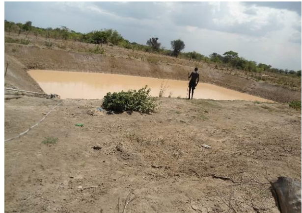
MAAIF excavated community dam with unlevelled soil piles in Buikwe District (left), and valley dam without means of drawing water and troughs in Kaganja village Nakasongola District (right)
