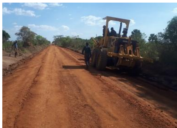
Gravelling works at km 8+400 along Bar junction-Corner Amach Road
