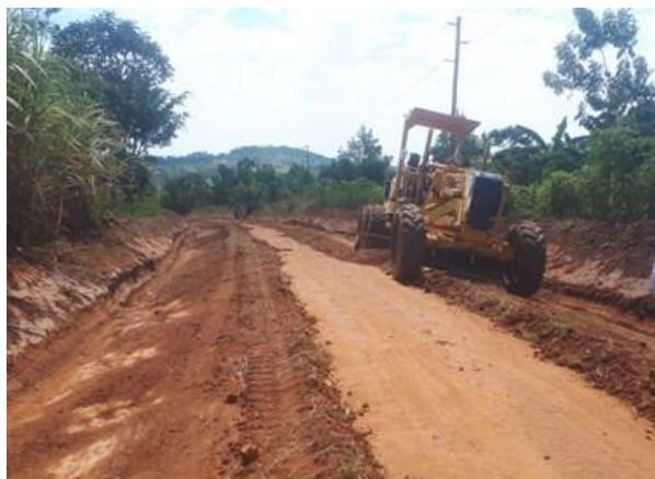
Kabowa-Budiima Road (21.4km): light grading ongoing in preparation for gravelling works
