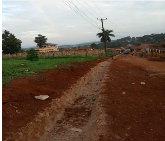
Stone pitching works at Ahamadiya road
