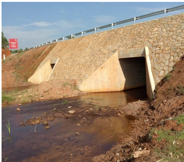
A box culvert at 1+500 on Kashenyi-Mitooma (11.53Km)
