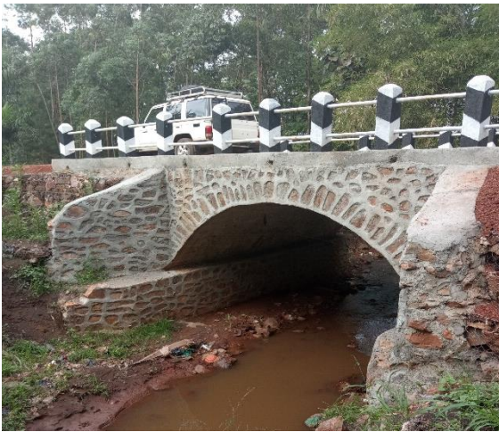
Chris Hanns Arch Bridge
