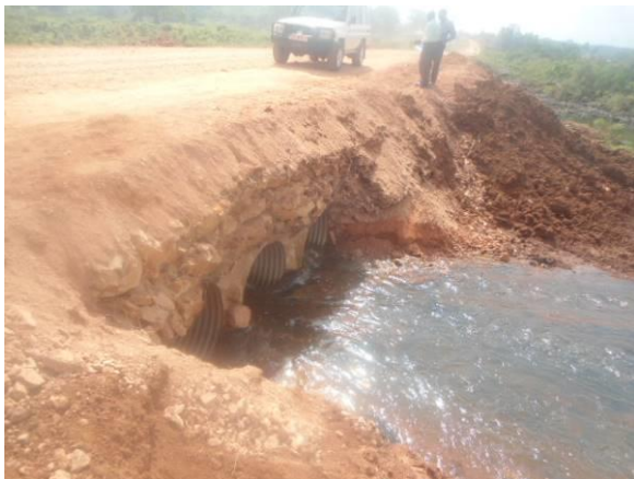
A section of Nakalere 111 swamp along Kiwologoma-Nakwero Road
