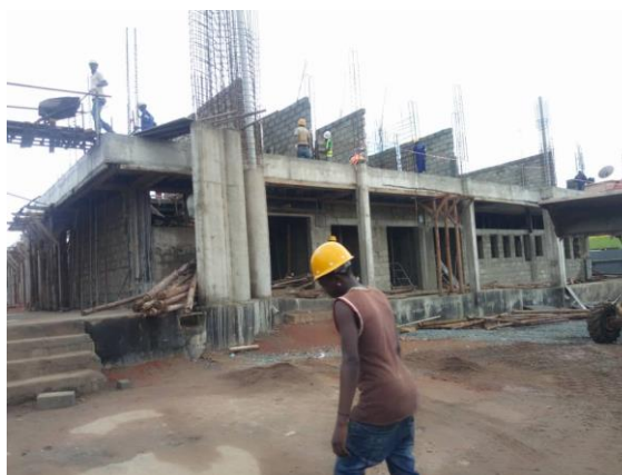
Steel work to columns on first floor for lockups ongoing as well as electro-mechanical works in progress, Kasese main market as at January 2019
