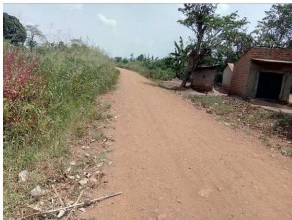
A section of Kyanga-Kamudindi-Kamulama Road
