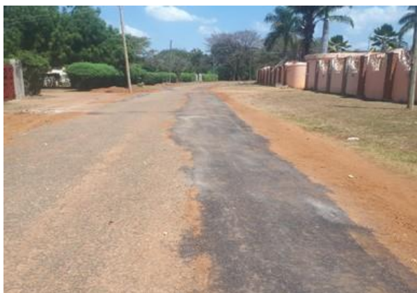
Kyoga Aenue (1.3 km) was undergoing patching works under periodic maintenance
