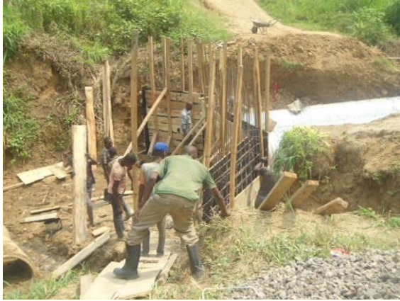
Mamowa Drift Bridge along Bumadu Katumba road
