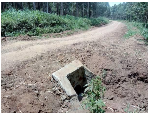
A culvert installed at 9+900 along Butambuka-Guwe-Kitwala Road
