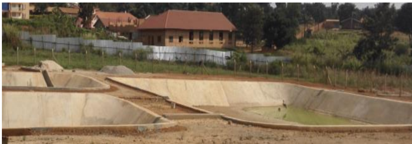
Lagoon at Substantial Completion at Hoima RRH
