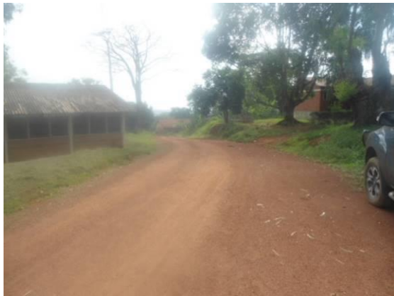
A completed section of Gayaza High School Circular road (1.3km)
