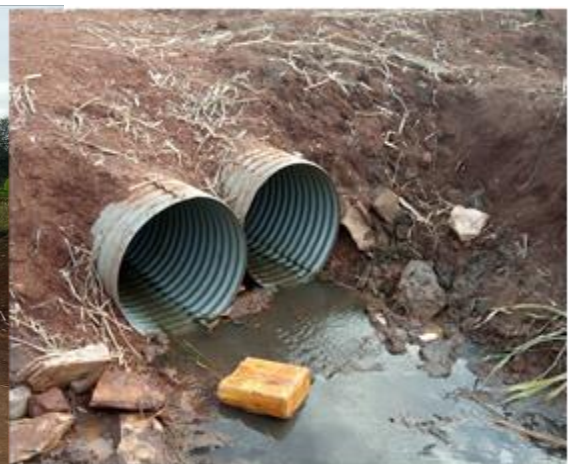
Armco culverts installed at Kinabi-Karim swamp
