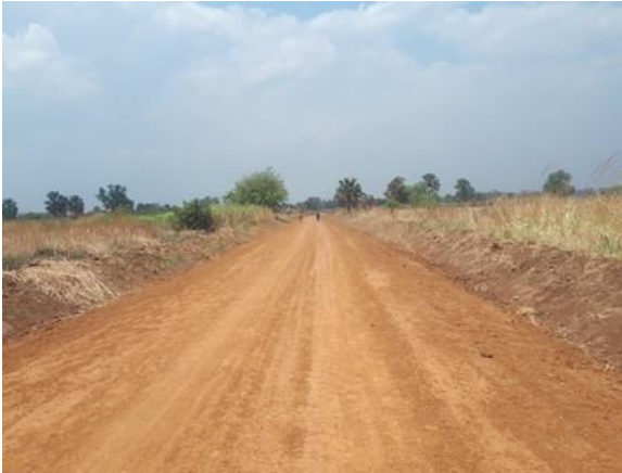
A gravelled section of Gulu-Onyama-Pabbo Road (20km) at km 5+750 worked on under RMeM in Q2
