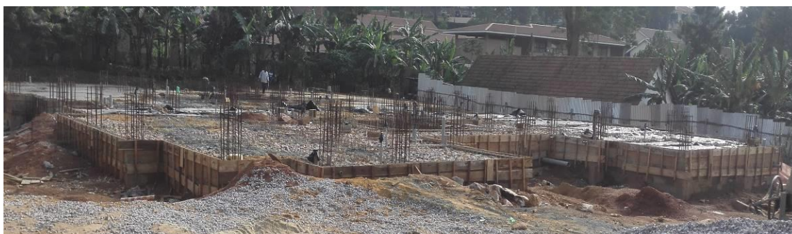
Ongoing foundation works at the 40Unit staff quarters at Masaka RRH
