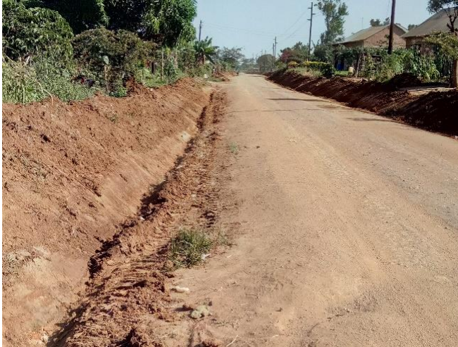
A section of Taba-Kyesiga-Dimo Road at km 0+000
