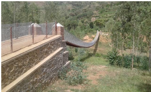
Finished cable bridge in Bubulo – Manafwa District
