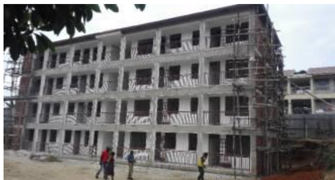
Staff hostel at substantial completion at Fort Portal RRH
