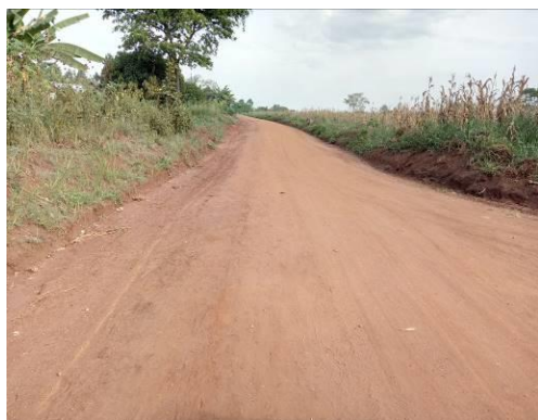
A section of Munsu- nkondo Road at km 6+000
