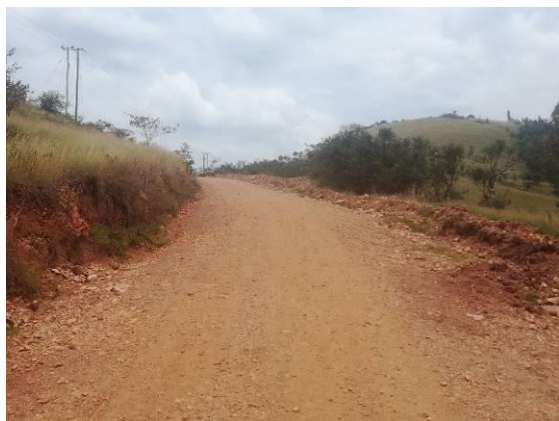
Katinda-Kagarama road (14.3km): A well compacted spot gravelled section at Km 4+100
