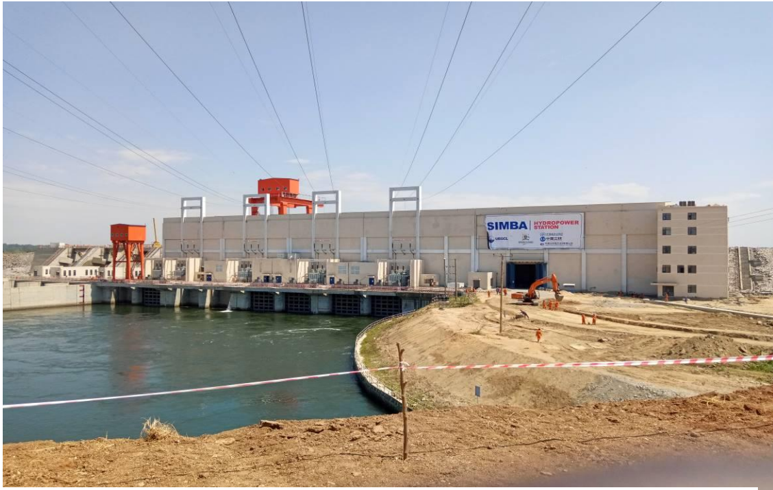
Downstream view of the completed Isimba HPP power house showing the evacuation lines
