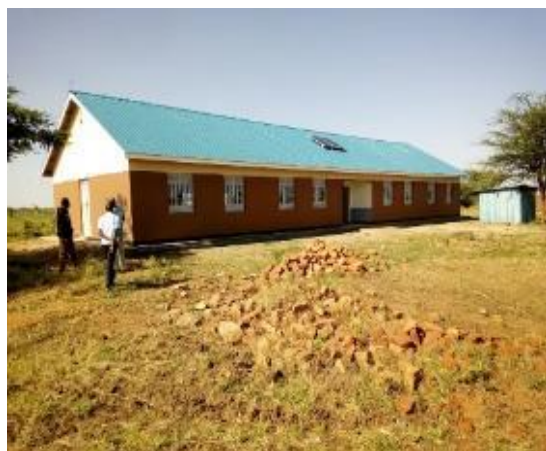
Completed Dormitory at Nadunget Primary School in Nadunget Sub-County, Moroto District as at January 2019
