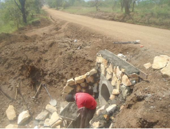
Culvert installation works at Karugutu-Ntoroko road at km 8+400 under Pekasa Enterprises
