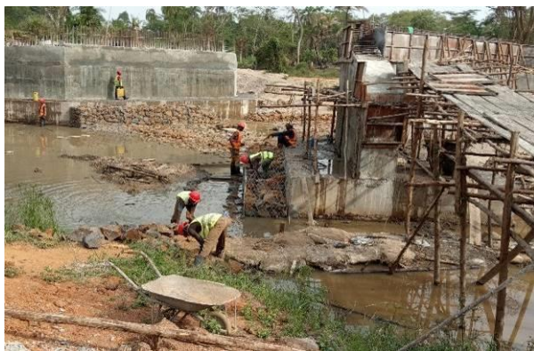
Construction of the abutment walls of Kasaigi bridge in Kakumiro District
