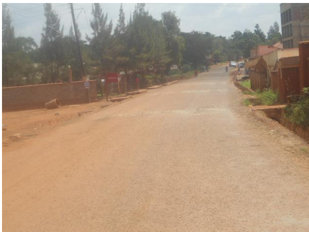
An upgraded section of Najeera-Kungu Road
