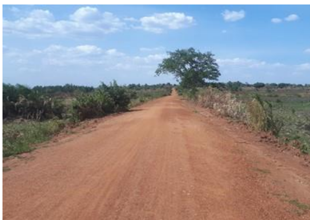
Graded section of junction-Corner Amach Road awaiting gravelling works
