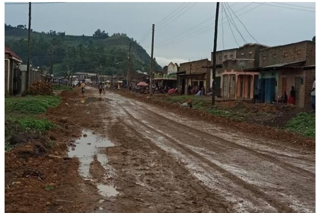
Road bed preparation works of Nyakasharu- Gahire road in Rubirizi TC
