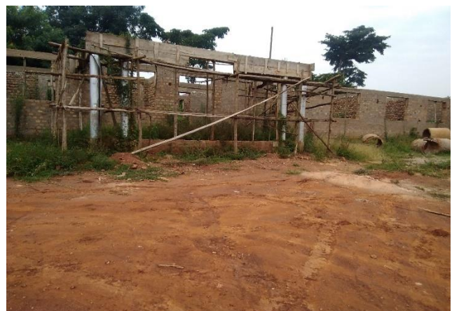
New kagadi town council head offices under construction
