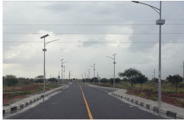
Jubilee Lane (0.567km): One of the completed town roads with solar street lights in Napak District as part of the Akisim-Moroto Road Project
