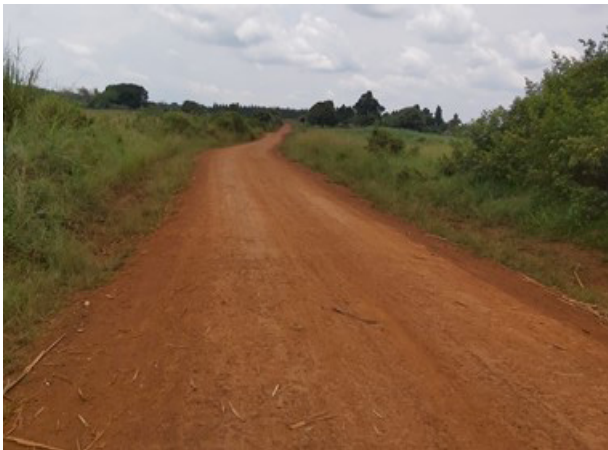
Katagukwa-Kibali-Balyegomba Road (13.6km) underwent routine mechanised maintenance in Q2 FY 2019/20
