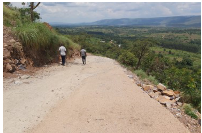
Concreted section of Butta-Kitta Road (0.7km). Works done using emergency funds
