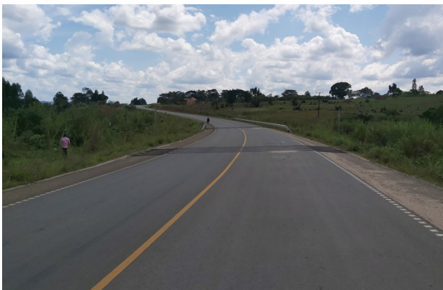
Completed section of Mubende-Kakumiro-Kagadi Road (107km) with rumble strips for speed control
