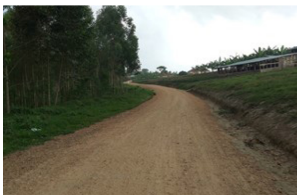
Ntungamo–Rwamukoto Road (1.7km) after rehabilitation in FY2019/20
