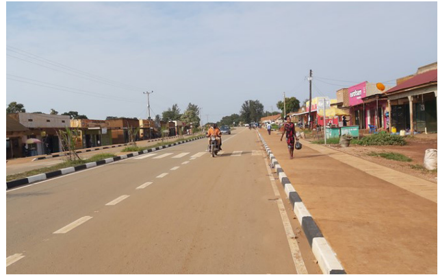
Kigolobya Town along Hoima- Wanseko Road. There is provision for pedestrian walkways, speed bumps, covered side drains, and zebra crossings
