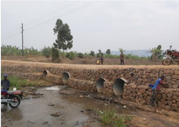
Armco culverts and gabions works installed on Mwizi-Kikagati Road at km 21+700
