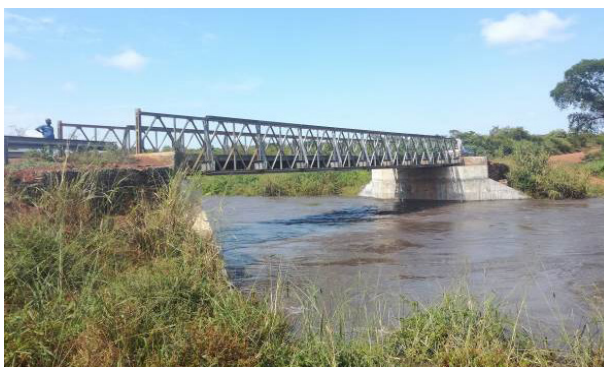
The 30.4m Gem Farm Bailey Bridge in Atiak, Amuru District
