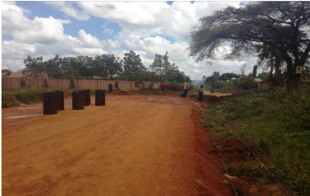
Ekayu Road: Preparation of priming for the road base and excavation
