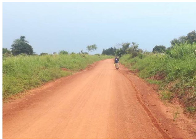
A well graded and graveled section of Katikati-Tenamu-Nwoya Road at Km 29+200
