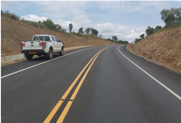
Part of the completed priority section of Masindi-Park Junction Road
