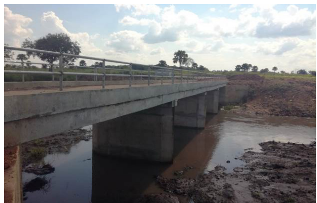
Cetkana-Palyec (5.7km): The 50m – 3 Span bridge at Km 3+000
