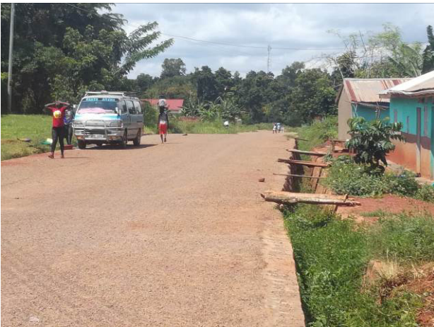
Gulu Gulu Road: The rehabilitated road without provision of access to the road side communities
