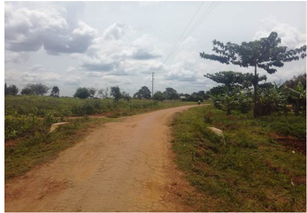
A 600mm culvert line complete with head and wing walls at Km 2+400 along Kameruka-Namirembe-Kakule Road
