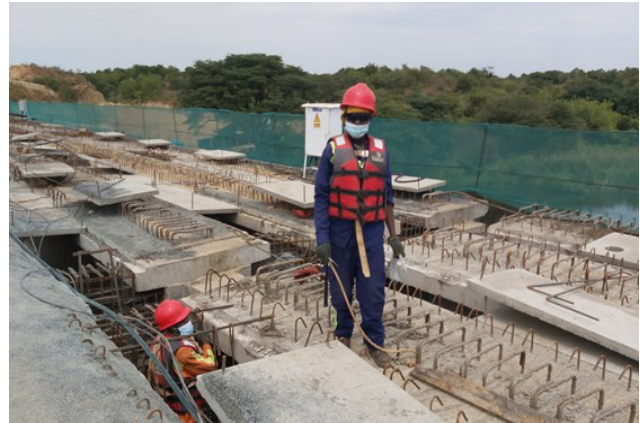
A female steel bender working on Paraa Bridge on Junction-Paraa-Buliisa Road
