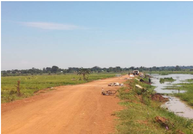
A raised section of the Nsokwe swamp crossing at the border of Bugiri and Bugweri District
