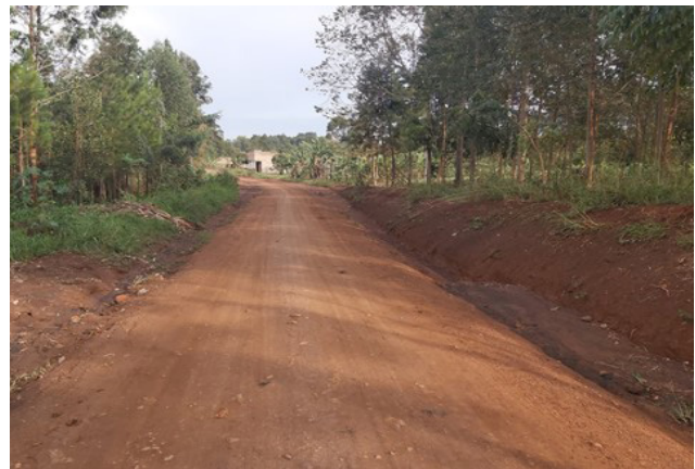
Kirungi-Kachwampale Road (9km) after routine mechanised maintenance in Q3
