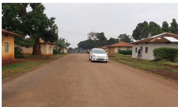
Double surface dressing done on Busambaga Road (0.8km) under periodic maintenance
