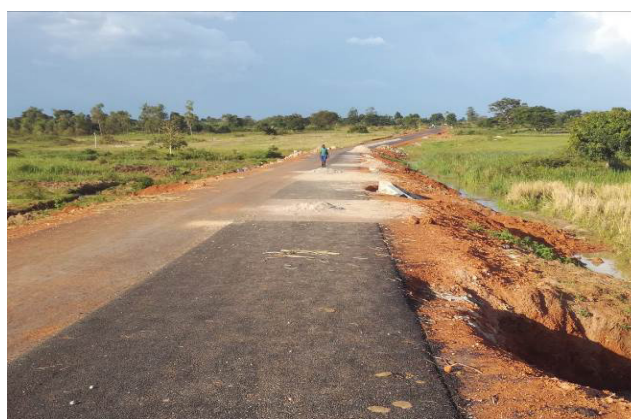
Kayumu-Atatur-Malera Road Section G undergoing LCS works using premix technology
