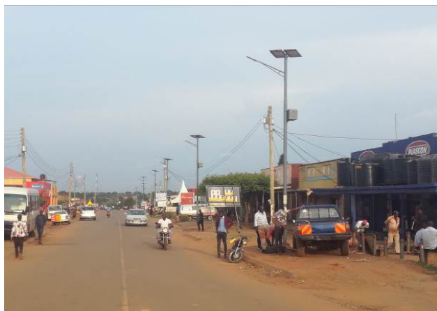
Solar lighting installed on the RHS of Gabula Road
