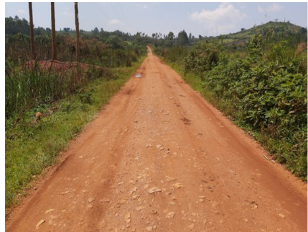
Kyakasura-Nyabaganga-Nyabuharwa Road (4.5km) underwent periodic maintenance in Q2
