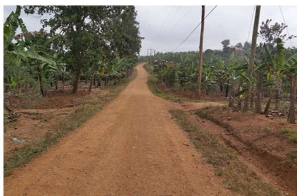
Runyinya-Kyeizooba Road (5.3km) received routine mechanised maintenance in Q2
