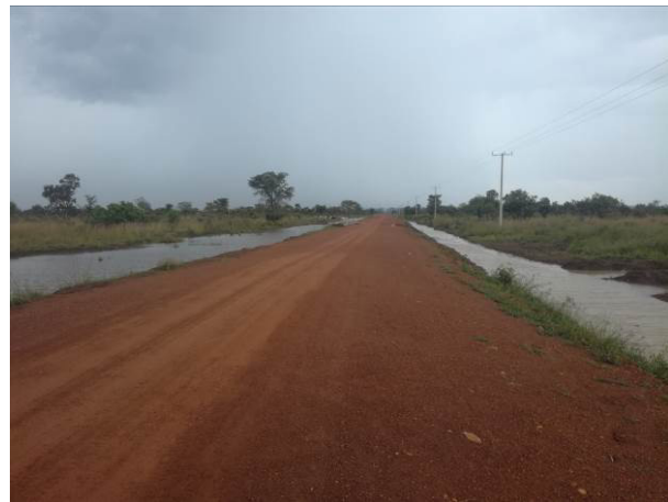
A well graded and graveled swamp raised section at km 7+600 on Usuk-Ngongoja road in Katakwi District
