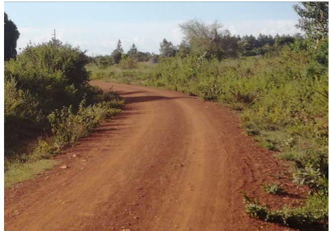
Atatur-Ongoopo-Kannaca Road (13km): Part of the 4 km section that underwent emergency intervention at Km 3+800 – Well graded but with over grown grass on the road side
