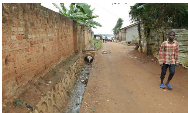
Stone pitching works for side drain on Wuma Road (0.43km)
