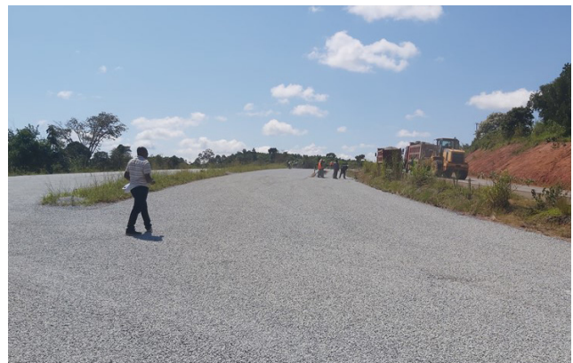
Construction of a resting area along Mubende-Kagadi Road at km 69+
