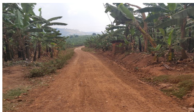
Kaguhanzya-Kyamatambirire Road (4km) received routine mechanised maintenance in Q2
