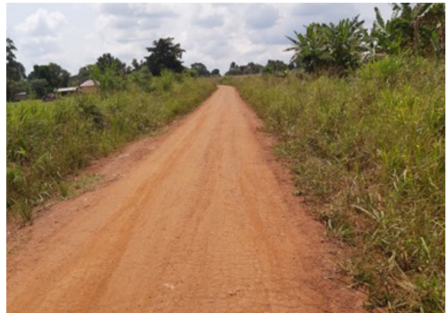
Kihaguzi-Kyakamese Road (10.1km) after routine mechanised maintenance in Q2 FY2019/20
