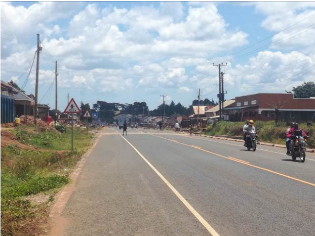
A completed section at Km 7+500 along the Busia-Majanji section of the Musita-Lumino/Busia-Majanji Road
