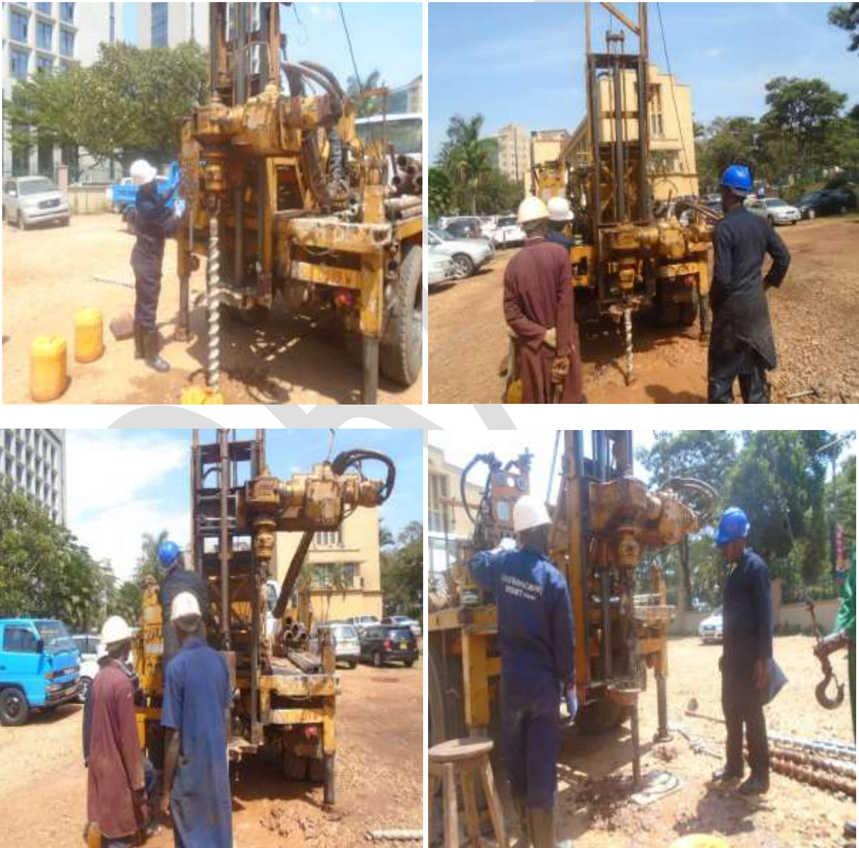
Figure 1: 1.0 – 4.0: Conducting drilling operations
