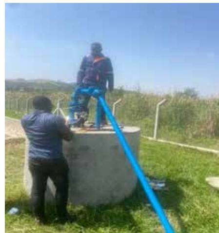
L: Intake; R: Ongoing repair works at the suction pipeline at Kabayanda SSI in Kabayanda Village, Kyewanula Parish, Lyantonde District.
