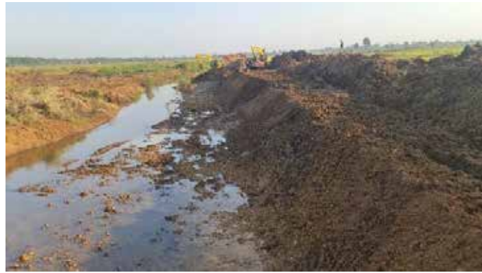
Dredging of River Tochi in Oyam District
