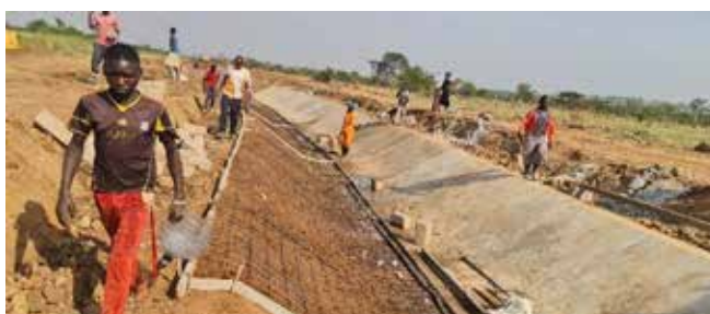
Casting a section of the main canal in Ragem, Packwach District
