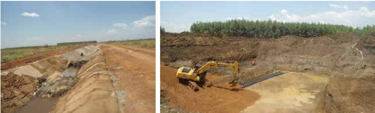
L-R: Ongoing excavation of head works and the secondary canal under construction at Acomai irrigation scheme
