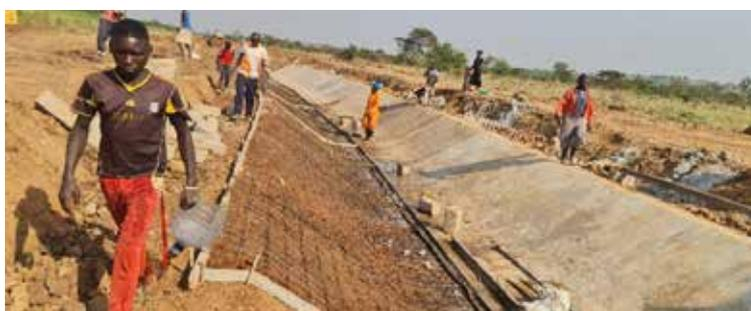
Casting a section of the main canal in Ragem, Packwach District
