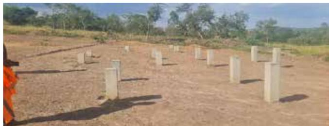
**Column studs for installation of solar array for Orutooma SSI system in Kiruhura District; and for installation of reservoir tank for Miti-Ebiri SSI systems in Kyotera District**
