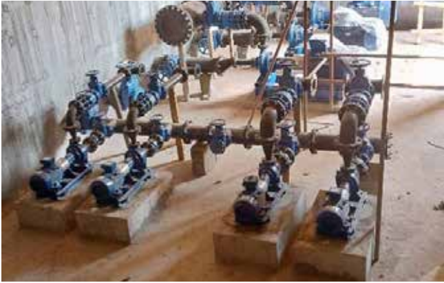
L-R: Pipe laying of the Karuma-Gulu Transmission Mains; Installed uplift pumps of Karuma Water Treatment Plant in Nwoya District
