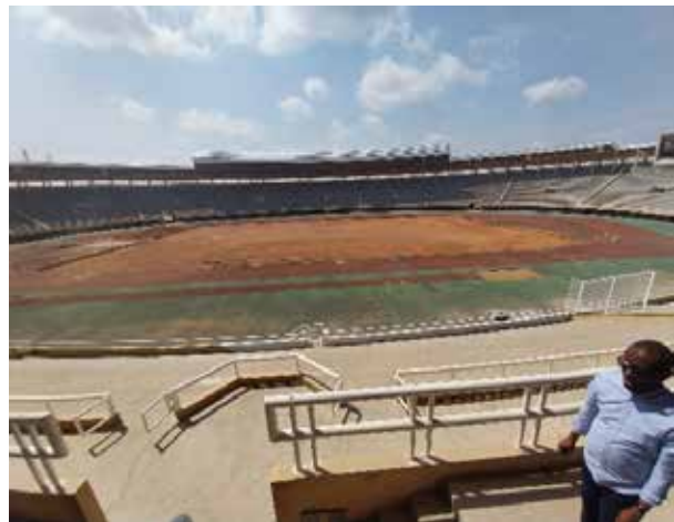
Status of ongoing renovation of the pitch at Namboole Stadium
