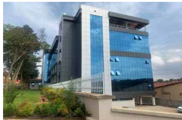
The six-floor UNEB Storage Facility completed and commissioned and in use
