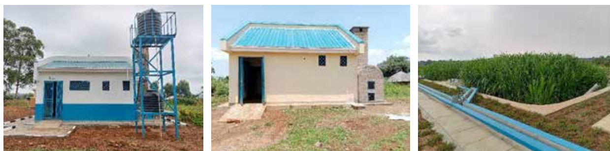
A section of the Yumbe Faecal Sludge Treatment Facility; Institutional toilets in Lawiadul P/S in Pader District, and Oriba P/S in Maracha District
