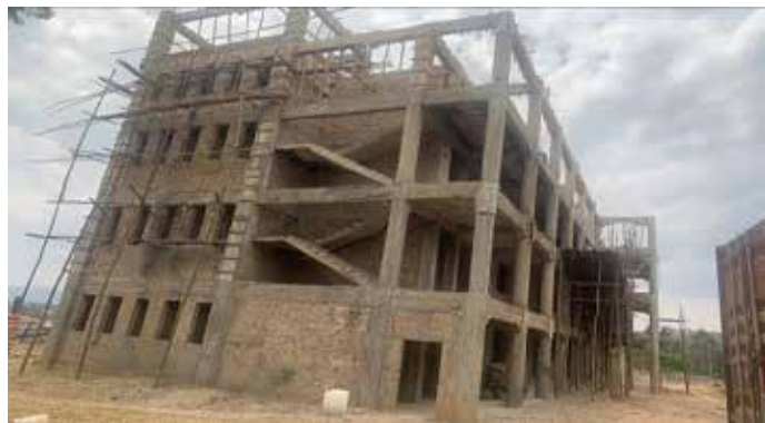
Construction of the Science Laboratory Block at Bishop Stuart University-Mbarara
