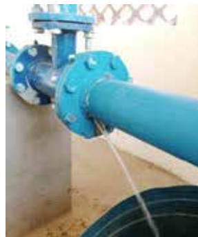
L-R: A PSP of Atiak WSS in Atiak Town Council in Amuru District; Stud columns for the reservoir tank; and a leaking flange of Bulangira WSS in Kibuku District
