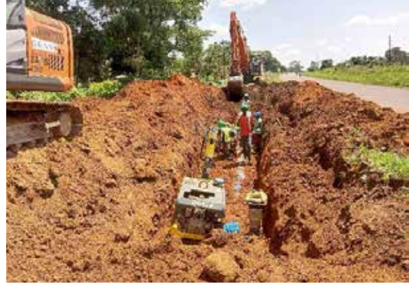
L-R: Pipe laying of the Karuma-Gulu Transmission Mains; Installed uplift pumps of Karuma Water Treatment Plant in Nwoya District
