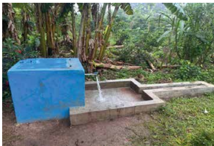
A functional yard tap for Nongo Rural Water Supply System in Busaale Parish, Luweero District.
