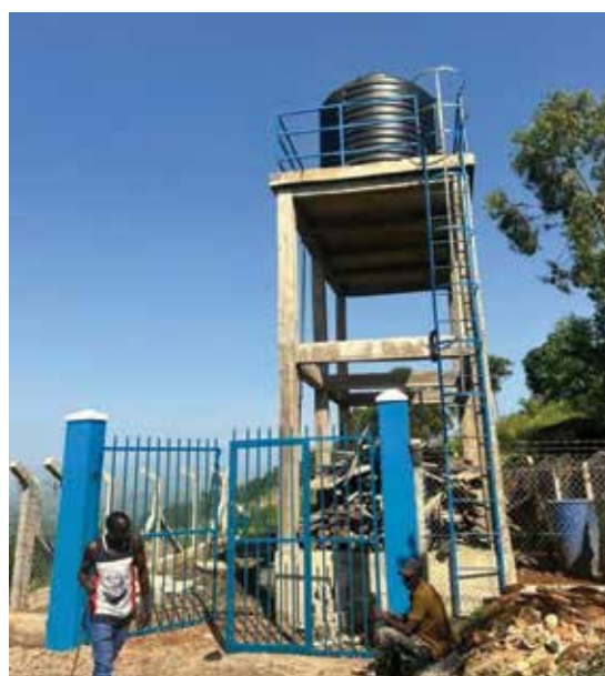
Two 10m 3 reservoir tanks for Iruhura Solar-powered Water Supply Scheme in Rweraza village, Rweraza Parish in Kabarole District.
