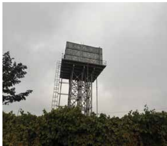
L: Functional PSP; R: 200m 3 reservoir tank at Masulita Urban Water Supply System in Masulita Town Council, Wakiso District.
