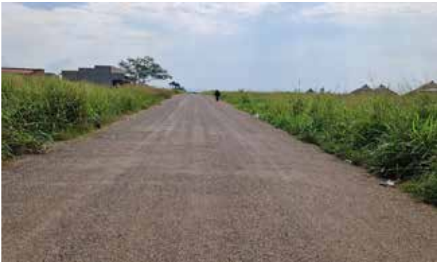
Amuru District: Market Street in Pabbo TC was upgraded using low-cost seal technology
