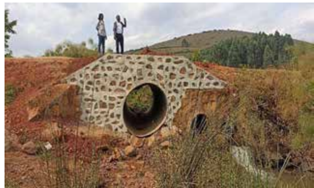
Ntungamo District: The 1800mm diameter Armcoculvert along the Katinda-Kagrama Road at kms 1+000
