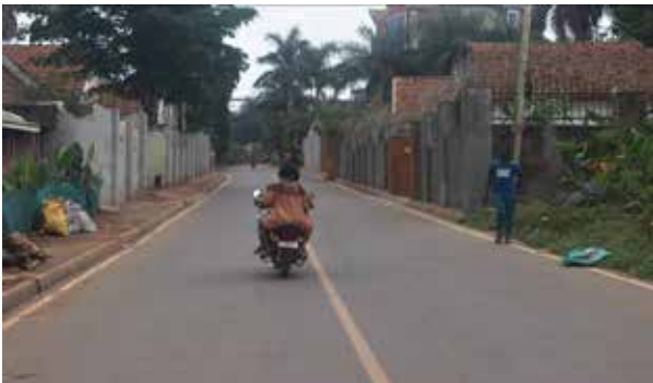
A marked Katuramu Lane in Bukasa – Makindye Division pending completion of paving the walkways
