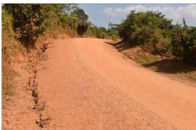
Mubende UNRA Station: A section of Kasambya-Nabakazi Road at the start (0+000)
