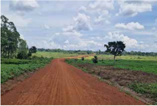
DRRU-Jinja: Bubinga-Buyebe-Buwabe Road (6.5kms) in Bugweri District after the rehabilitation works. The swamp section was raised
