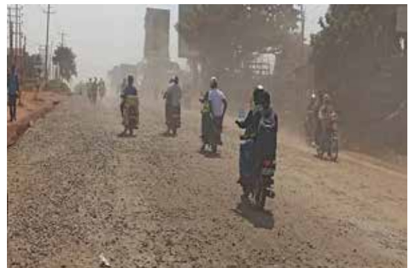
Kampala-Jinja Road: CRR works at the start of the project at Nakawa
