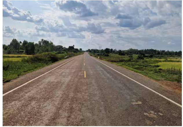
Tororo UNRA Station: Nagongera–Busolwe– Busaba after (kms) was upgraded from Gravel to Bituminous Low Volume Seal Road
