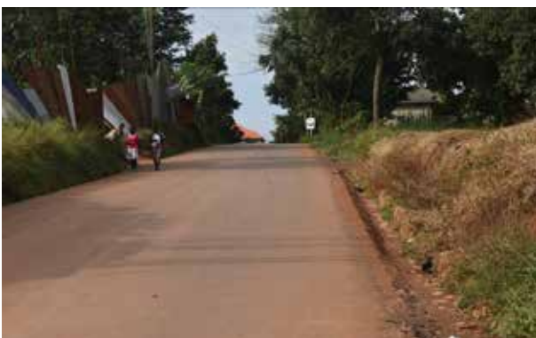
Blaire Road in Kira Municipality paved with asphalt pending road marking
