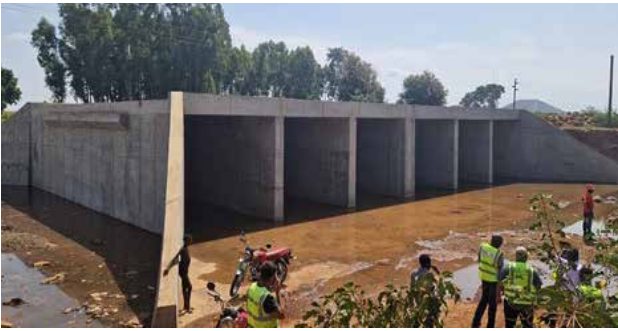
Six cell box culverts constructed along Muyembe-Nakapiripiriti Road
