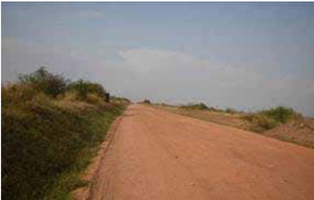
Kasese UNRA Station: A well-graded and shaped section of L.Rwentare-L.George Road at the start (kms 0+000)
