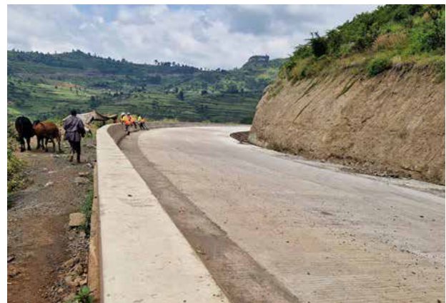
Completed section of rigid pavement along Kapchorwa- Swam Road Project
