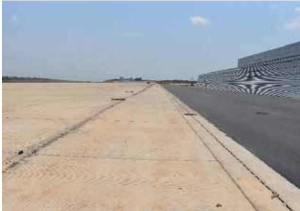
Kabaale International Airport: The parking apron in front of the terminal building
