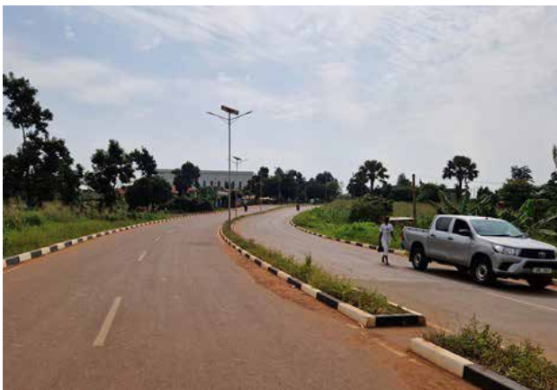
Gulu Logistics Hub Access Road – the project was substantially complete
