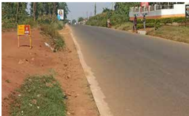
A completed paved section with a concrete edge beam in Kayunga Town on the Kayunga-Nabuganyi Road in Kayunga District using the Probase Technology
