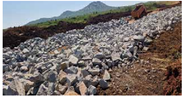
Rockfilling of a swamp section along the Rwenkanye-Apac Road Project
