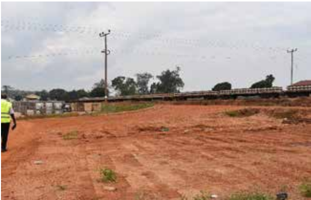
Assembled rail tracks loaded on a train at Kawolo-Lugazi for transportation to Kampala-Namanve section works
