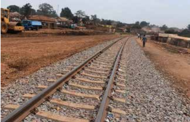
A completed section of the railway line at Namanve Station
