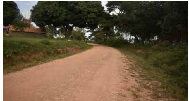
One of the opened, graded and graveled roads in Ndejje University, done in preparation for the hosting of the East African University games in December 2022
