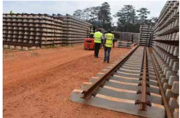
Assembled rail tracks at the Kawolo-Lugazi
