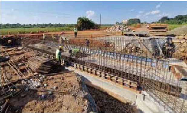
Construction of a box culvert along the Apac-Lira Road section
