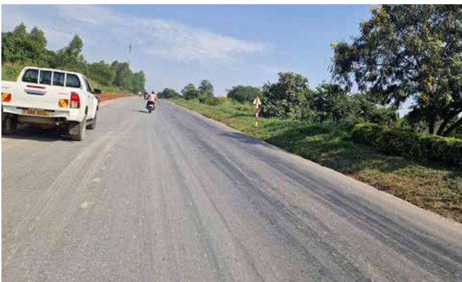
Rehabilitated section of Lira – Kamudini Road section
