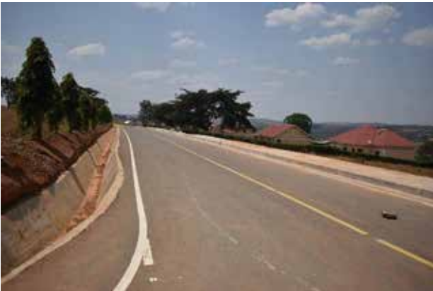
One of the completed Rushere Town roads with a pedestrian walkway, concrete line drain, and road markings
