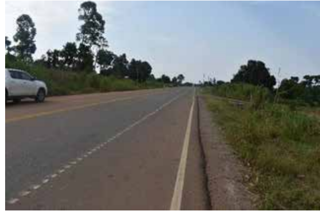
A completed section at Kms 19+000 along the Hohwa-Nyairongo-Kyarushesha Road Project on Oil Road Package 5
