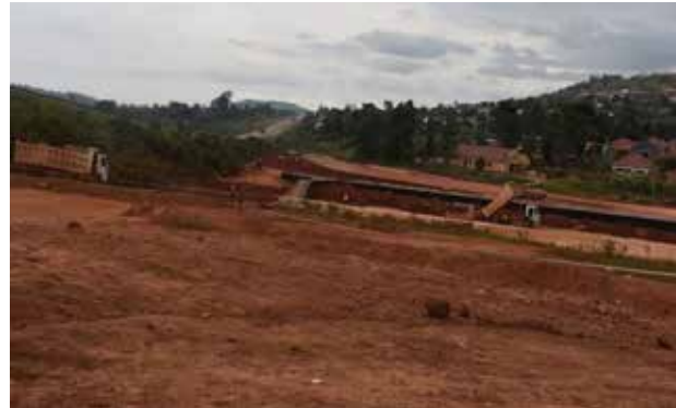
Bridge construction at interchange No.3 (kms 12+500) on the Busega-Mpigi Expressway Road
