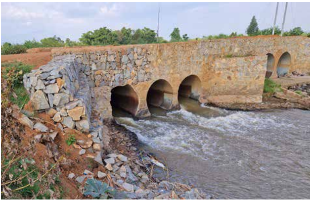
Tororo UNRA Station: Emergency works on Kachonga-Kidoko-Magodes Road
