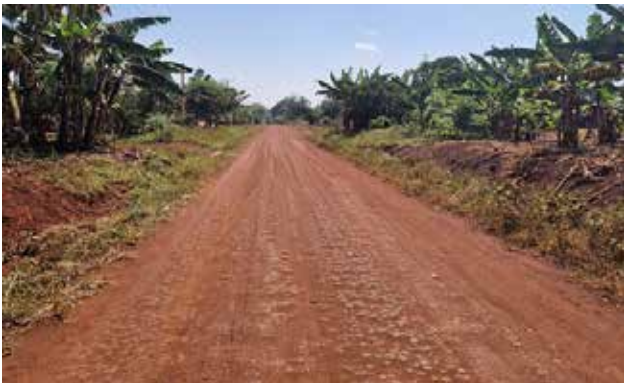
Bugiri District: A section of Muterere-Kimbale after routine mechanized maintenance
