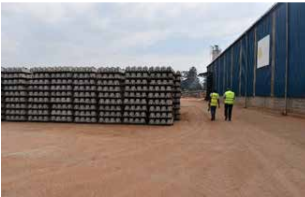
The Concrete Railway Sleepers in the factory yard at Kawolo-Lugazi
