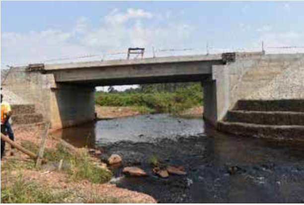
Completed Fjumangabo bridge at Kms 17+163 along the Kabaale-Kiziranfumbi (25kms) Road Project on Oil Road Package 5
