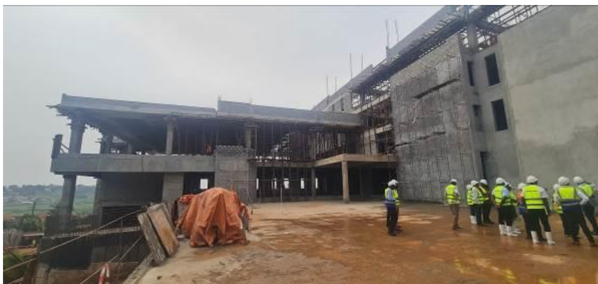
Construction of the BDS superstructure in Butabika
