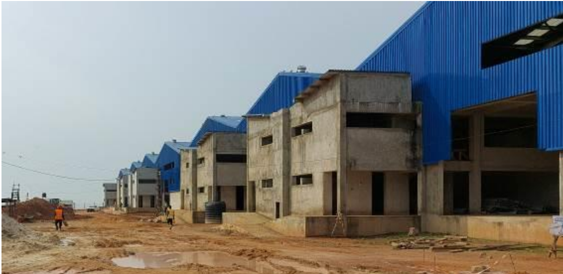
Substantially complete production units at the Airport Free Zone, Entebbe
