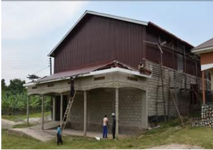
Renovated coffee processing house at Rwandaro
