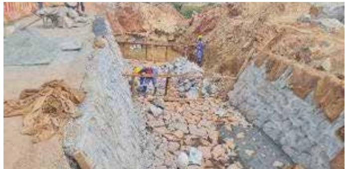
L-R: Stone pitching along a road in the North Estate. A levelled A2 road ready for paving in South A Estate of the Kampala Industrial and Business Park
