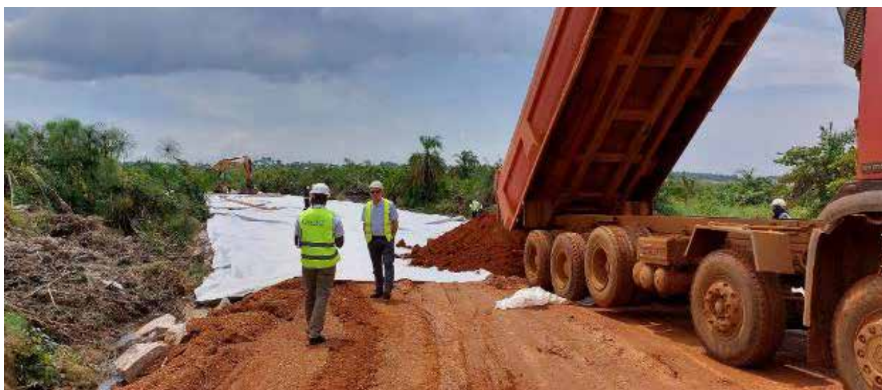
Ongoing works in South C estate at KIBP
