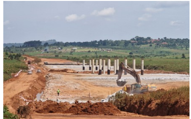
Busega -Mpigi Express: Ongoing bridge construction at km 25+500
