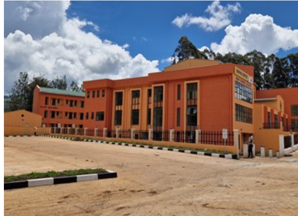
One Stop Border Post constructed at Suam
