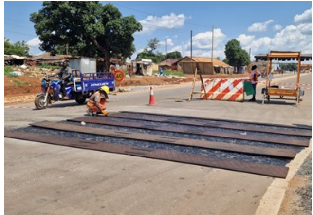
Installation of rumble strip in Adjumani Town along Atiak – Laropi Road
