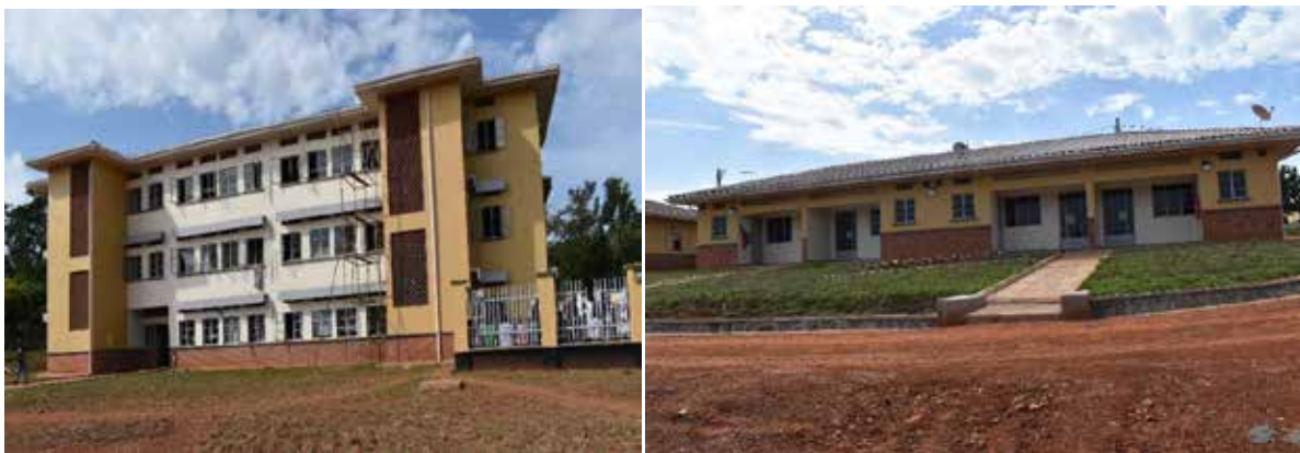
Left: Completed 3- level, 86 Bed capacity boys' dormitory; Right: 4-Unit one Bed room Staff House at Nawanyago Technical Institute in Kamuli District.
