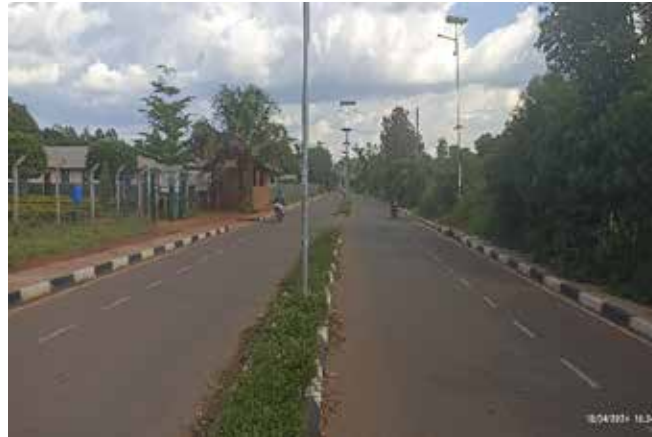
Completed Nelson Mandela Road in Gulu City
