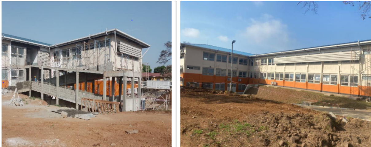
L-R: Ramp under construction on the existing wards, and compound leveling
