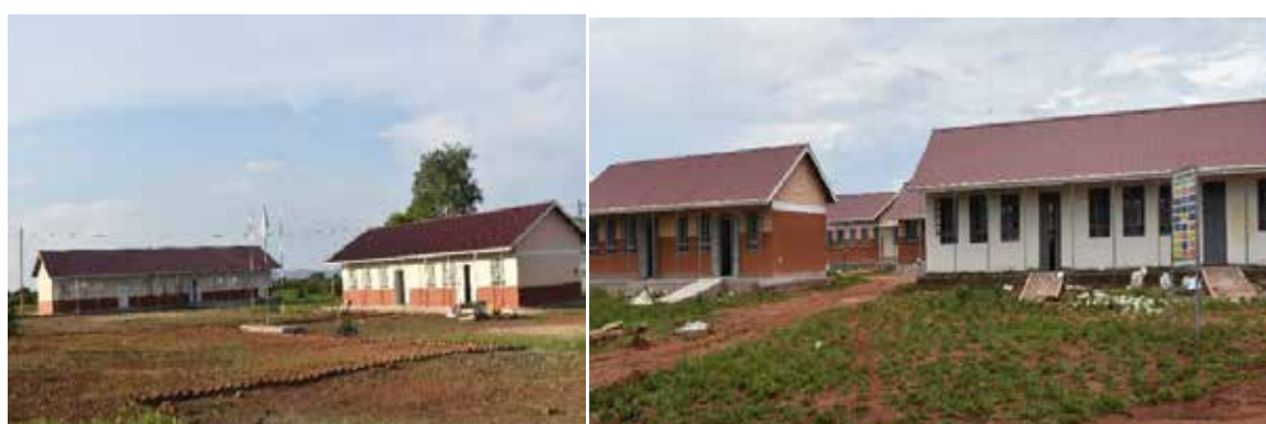
Left: Phase II Substantially complete structures at Arinyapi Seed S.S in Adjumani District; Right: substantially complete structures at Nsambya Seed S.S in Kyankwanzi District.
