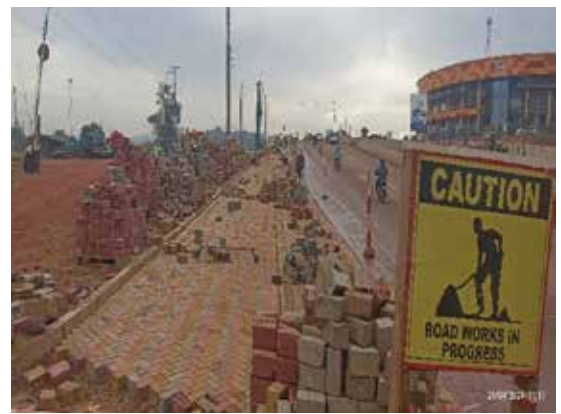
Ongoing pedestrian walkway paving works at Nsambya Junction
