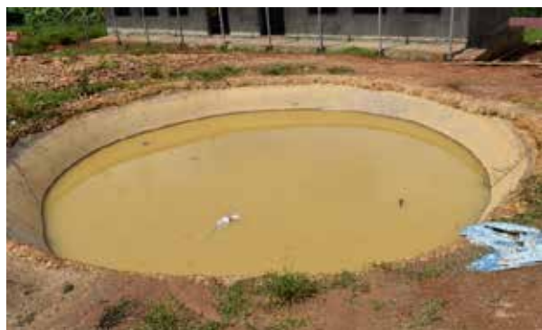
Un covered/unprotected water storage facility/pond at Kitojo Seed S.S-Mitooma district
