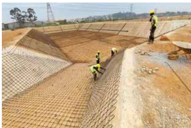
L-R: Setting out and concrete casting for the Sludge dumping and pre-treatment area and Casting of concrete for the side wall anaerobic ponds for Nalukolongo fecal sludge
