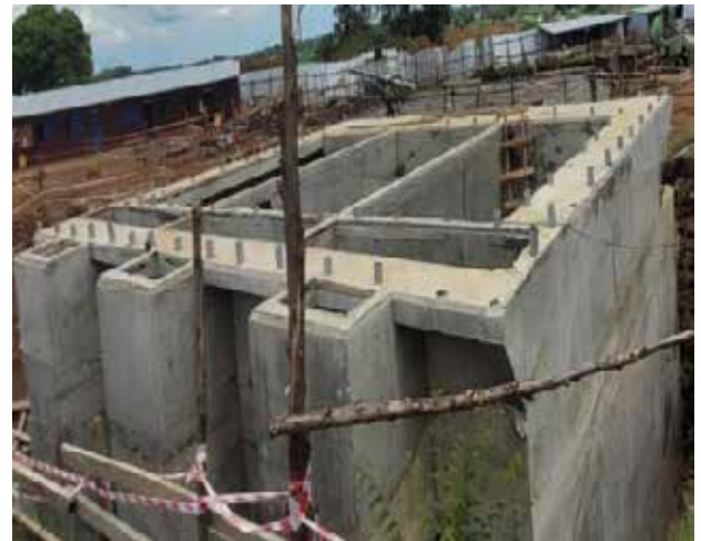
L-R: Surface water pumps at Buikwe WSS and Rapid sand filter at Water treatment plant at Kamuli WSS
