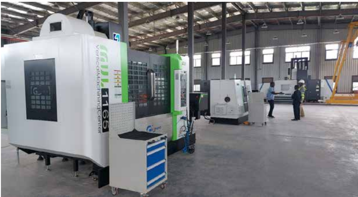
Vertical CNC machines installed in production workshop at Rwebiteete and tested
