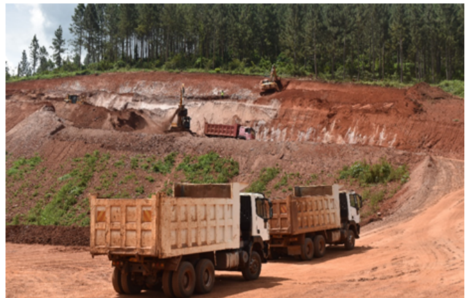
Construction of Kabuyanda Earth Dam in Kanyimizi Parish Isingiro district
