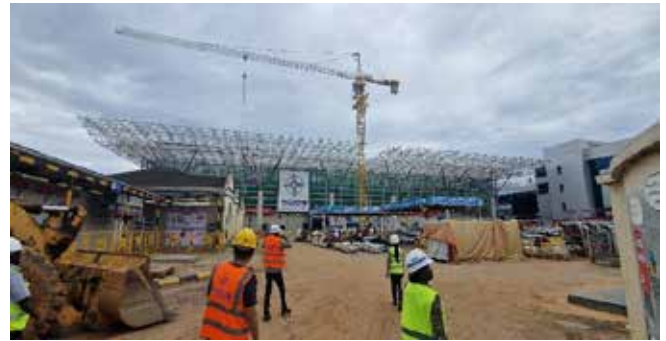
New Passenger Terminal Building that was still under construction
