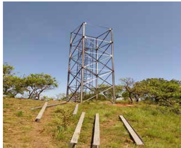
L-R: A Public Stand Post at Nkandwa Solar powered WSS in Kyankwanzi district. Tower erection for the water reservoir tank at Lakwa in Agago district
