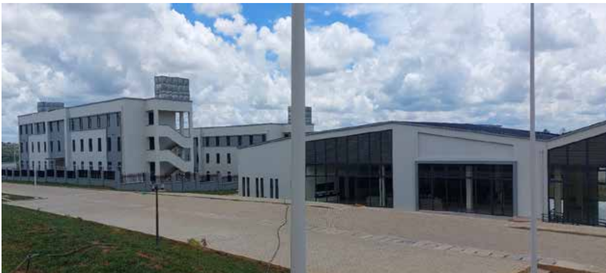
L-R: Completed hostel block and main dining and library blocks at Rwebitete, Kiruhura District
