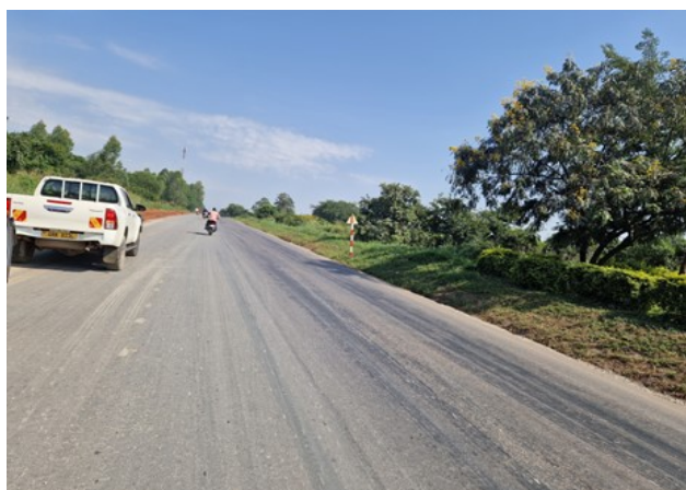
Rehabilitated section of Lira-Kamudini with new asphalt surfacing
