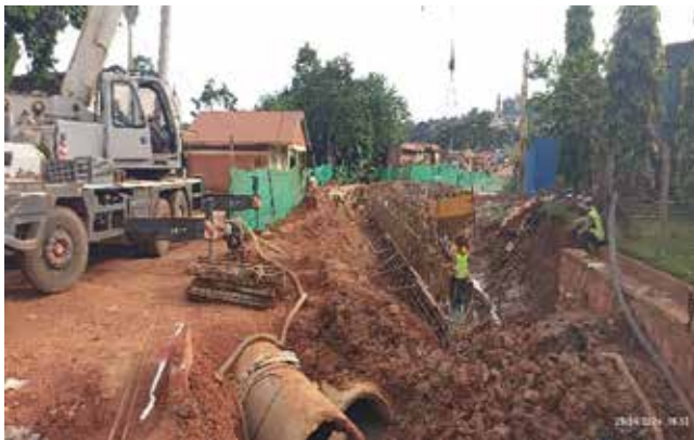
Ongoing box culvert works along Wamala road in Rubaga Division
