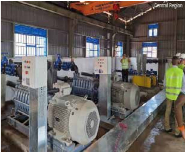
L-R: Surface water pumps at Buikwe WSS and Rapid sand filter at Water treatment plant at Kamuli WSS
