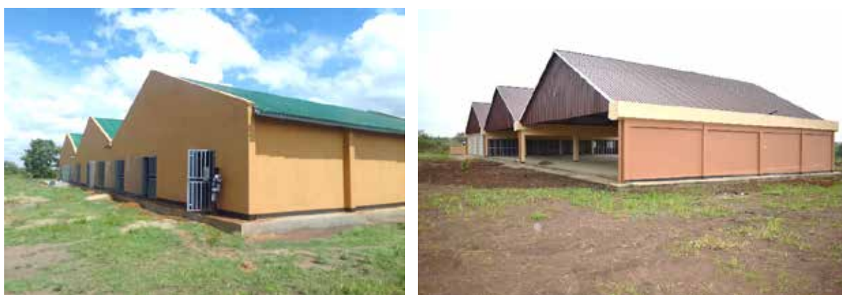
L-R: Completed Lokole satellite market in Agago District and , Opit satellite market in Omoro
