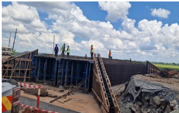
Construction of box culvert long Apac -Lira road section
