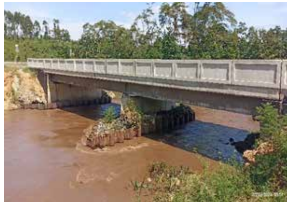
The completed bridge Ntungu bridge bordering Rukungiri and Kanugu district
