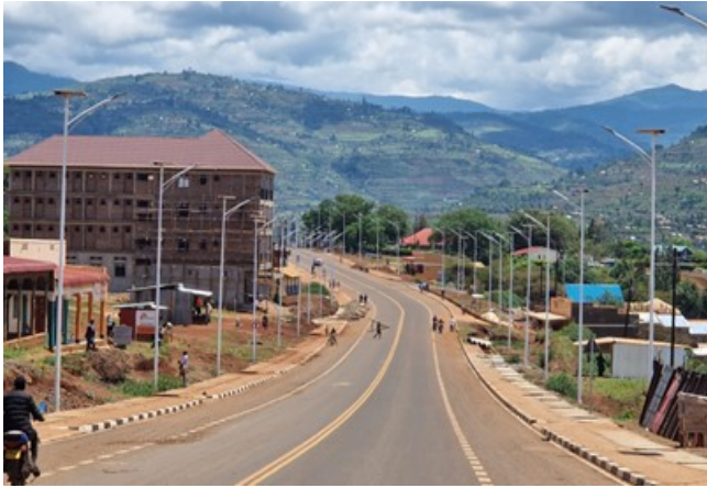
A completed section of the Kapchorwa-Suam Road in Buko Town, featuring pedestrian walkways and street lighting on both sides.
