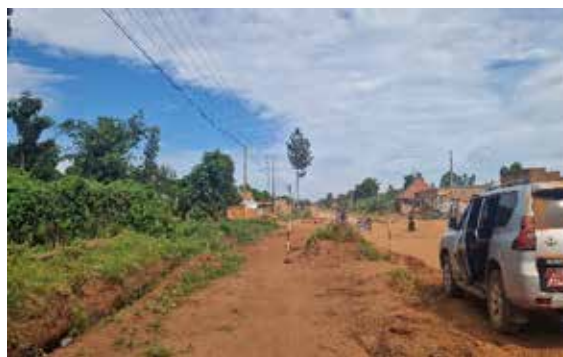
Earth works on Luwero-Butalangu road
