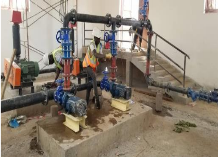
L-R: Pipe fitting and mechanical installations in the pumphouse for Kapchorwa WSS and Chemical mixing equipment in Bundibugvo WSS
