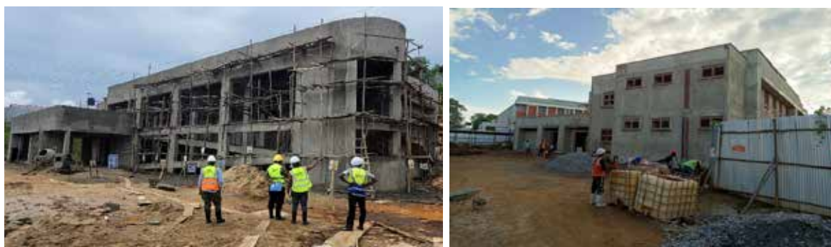
L-R: Biosafety laboratory under construction at Fortportal RRH and Lira RRH
