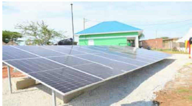
Completed shared solar mini-grid system at Tisai in Kumi District
