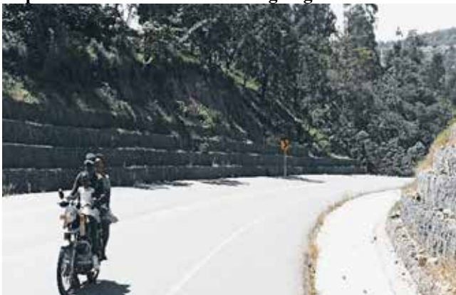
Gabion protection works of the embankment at Km 39+200
