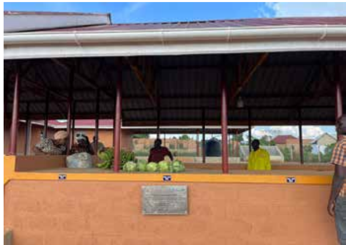
Functional Katakamese Market Shed in Nakaseke District
