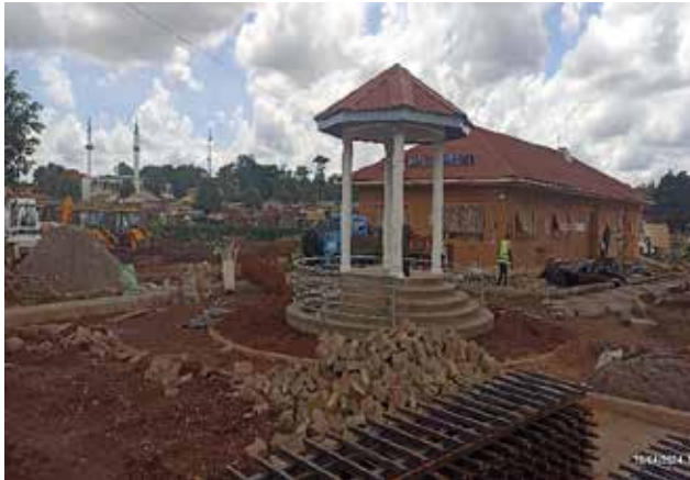
Ongoing works at the Coronation Park in Lira City Council
