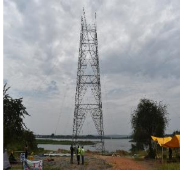
Left: Works on plant house and switchyard at Nebbi substation
