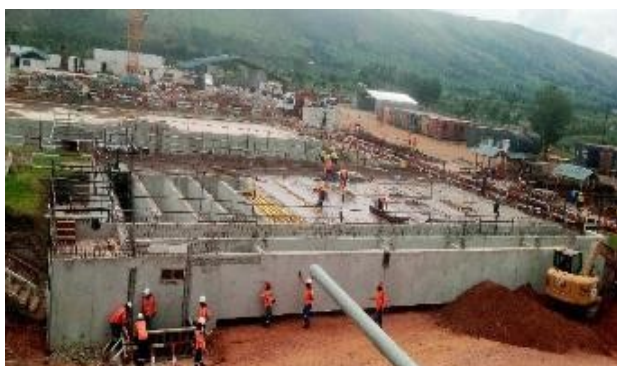
Left: Ongoing construction at the Sand filter tanks. Right: Ongoing foundation works for the administration block for Kagera water works
