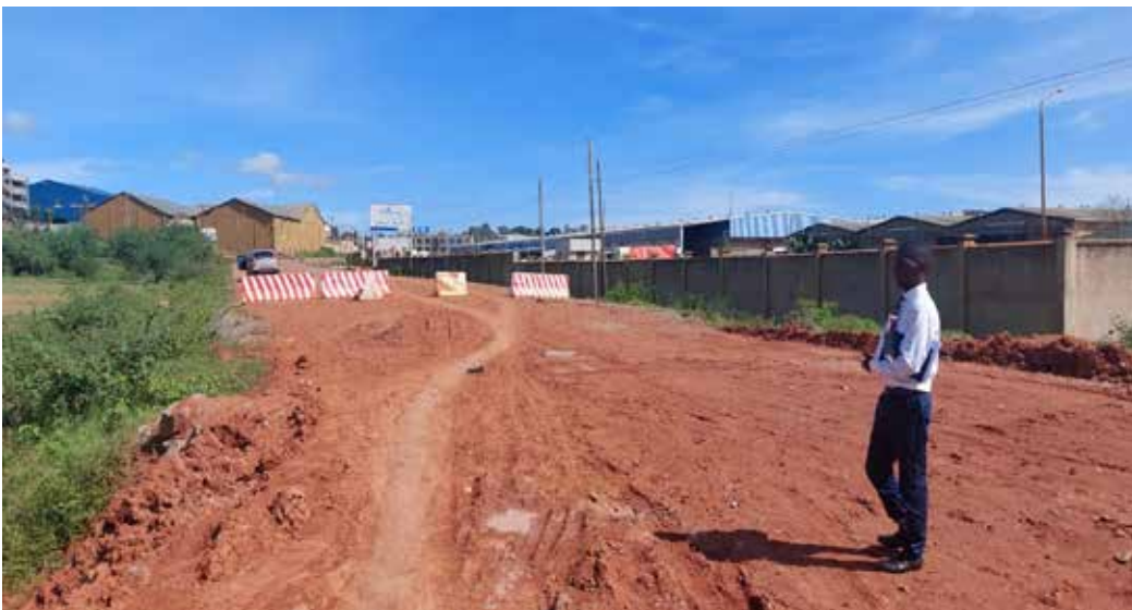
Up: A section of Paved circular road in South C Estate
