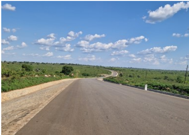
Completed road section of Atiak-Laropi Road Project
