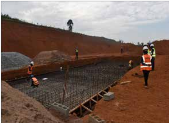
L-R: On-going foundation works at the 132kV substation; A completed resettlement house on the Kabale-Mirama transmission project at Muyumbu village, Kabale.
