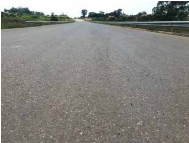
Paved section on Masindi – Biiso Road
