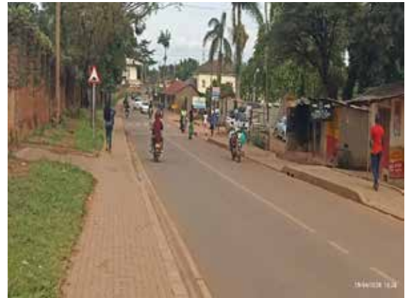
A completed section of Kabega Road in Makindye Division
