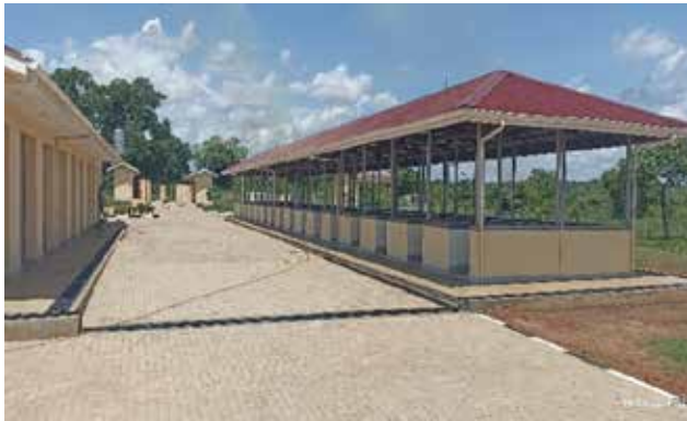
A completed market facility at Lagot Opuk in Lamwo District
