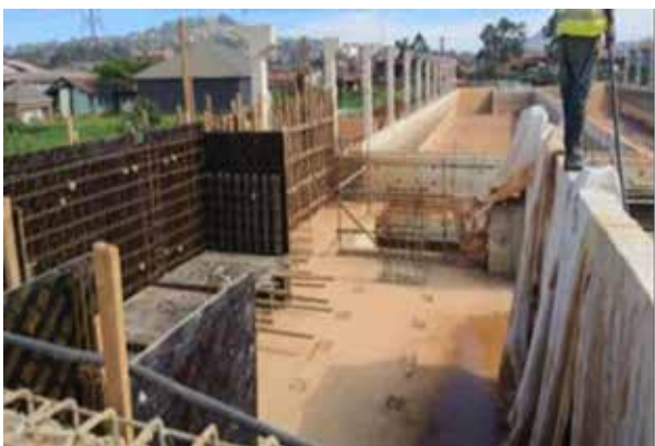
L-R: Setting out and concrete casting for the Sludge dumping and pre-treatment area and Casting of concrete for the side wall anaerobic ponds for Nalukolongo fecal sludge
