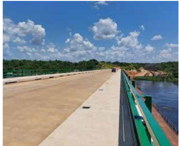
Paara Bridge along the Masindi – Park Junction road
