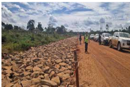
Swamp treatment works on Luwero-Butalangu road
