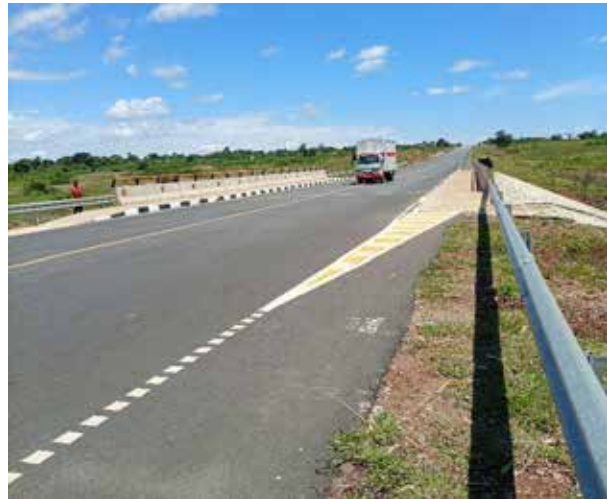
A bridge at 58+700 along Pallisa-Kumi road
