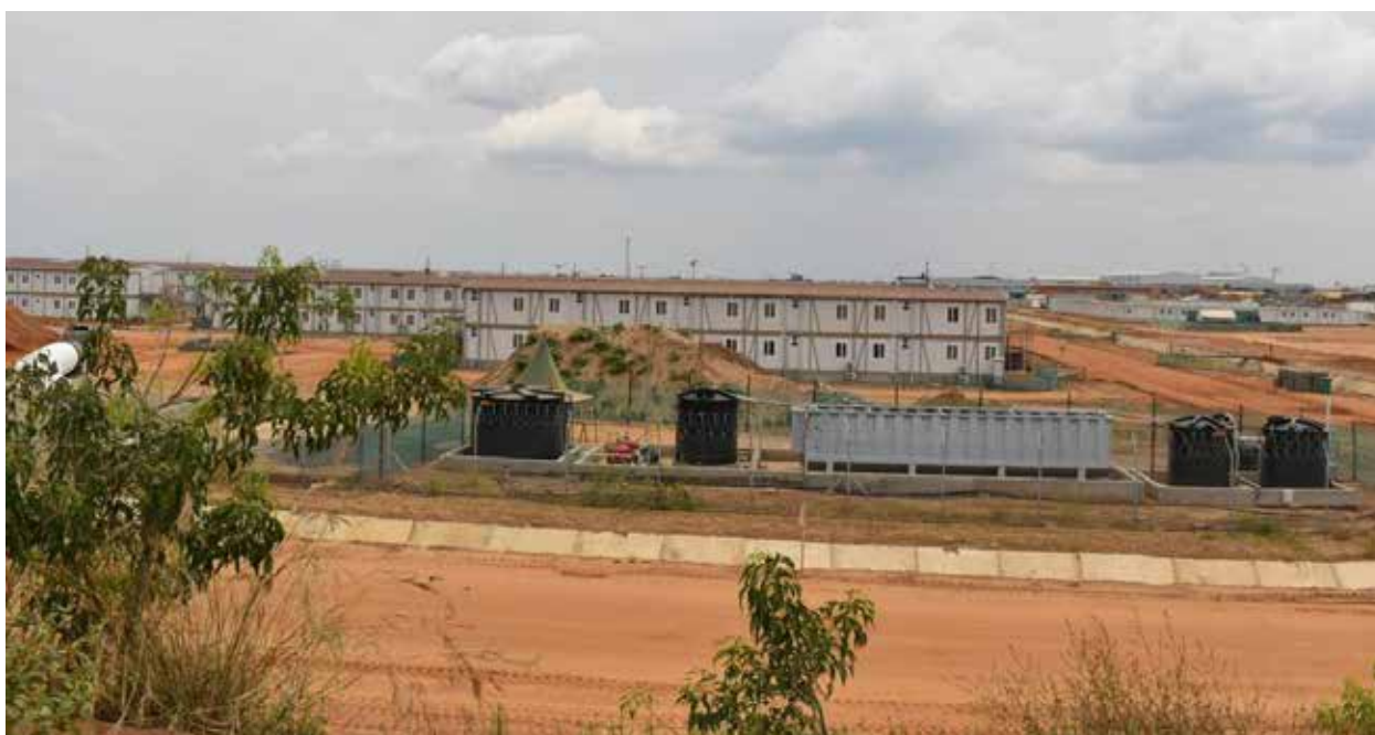
Completed temporary worker's housing units at the Tilenga CPF
