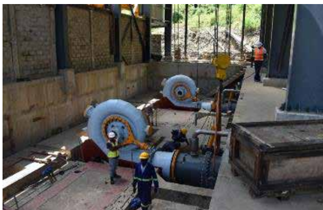
L: Completed penstock and partially completed plant house building at Nyagak III HPP
