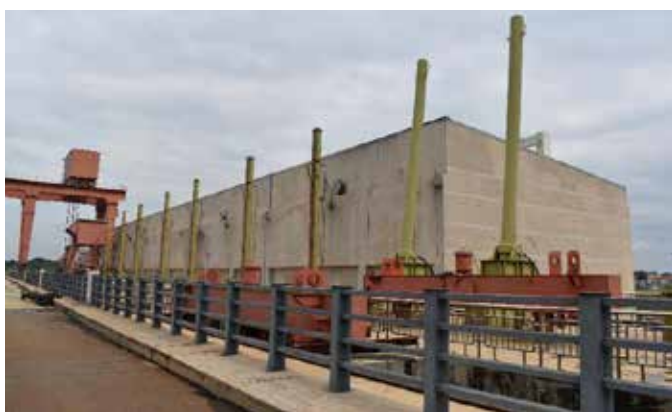
Plant house building and gate lifting hydraulic actuators at the Isimba HPP
