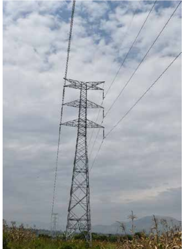
L-R: Completed resettlement house on the Kabale-Mirama Transmission Project; Part of a strung section on the Mirama-Kabale Transmission Project in Ntungamo District
